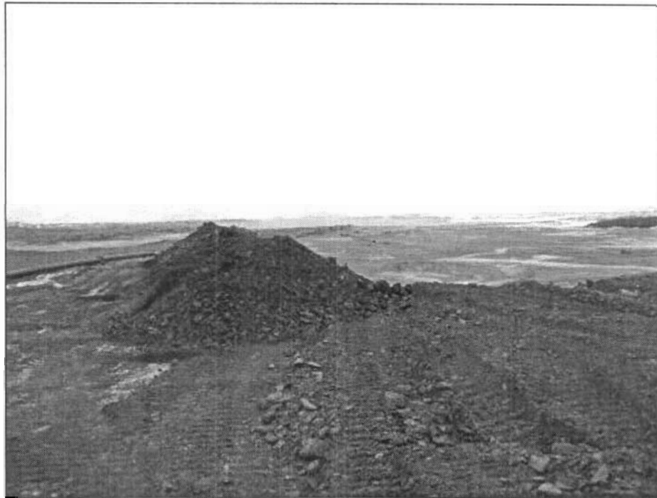
Photo 3 – Stockpiled crushed shale awaiting placement on top of the sub-aerial portion of WTDA
