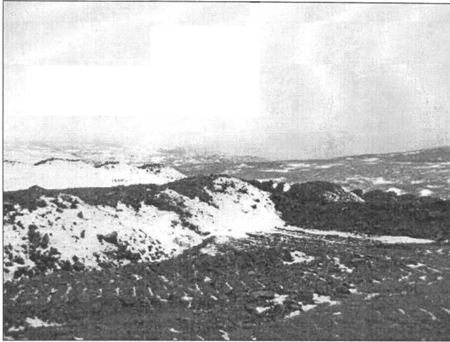
Photo 5 – Shale has been mixed with waste at the landfill and bulldozed into layers
