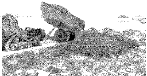
Backfilling basement and broken concrete
