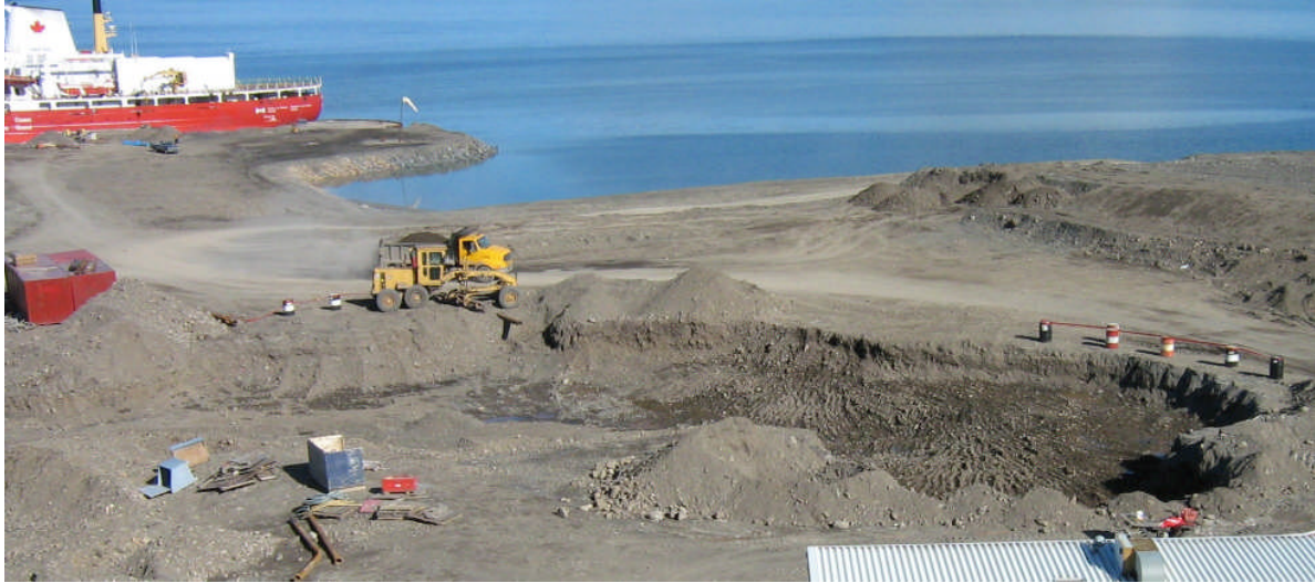
Hydrocarbon Excavation near former refuge station
