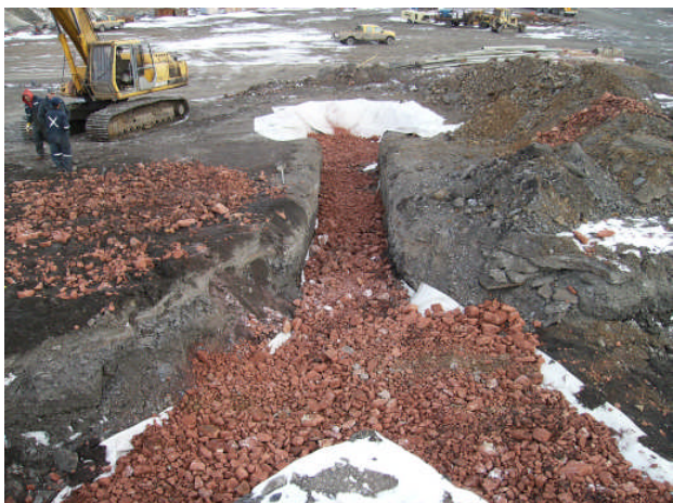
Seepage conduit and sump under construction
