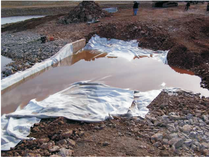
Photo 15 GCL installed upstream of outlet wall to reduce seepage losses. Note embedment of liner in wall abutments.
