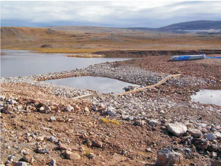
Photo 13 West Twin Outlet Channel prior to GCL installation. Note water level on upstream side of wall approximately 20 cm below crest of wall.
