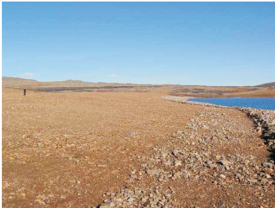
Photo 30 Toe of Test Cell Dike cover along remnant north/south arm of Test Cell Dike.
