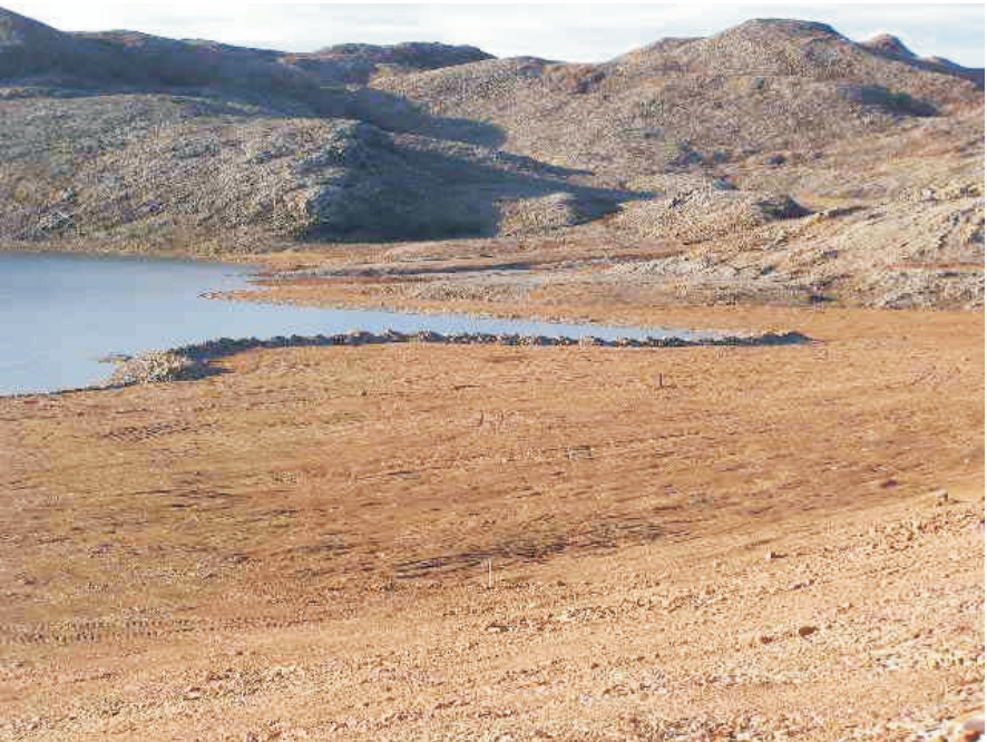
Photo 34 Riprap stockpiled along shoreline of tailings cover at the toe of the West Twin Dike.
