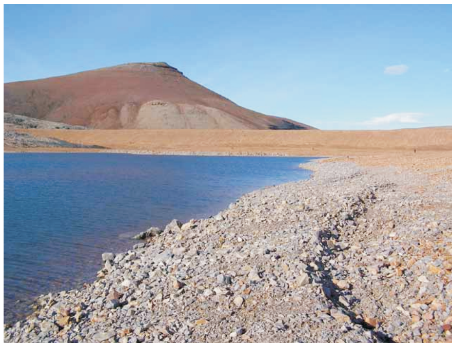
Photo 31 Riprap along shoreline of remnant east/west arm of Test Cell Dike.
