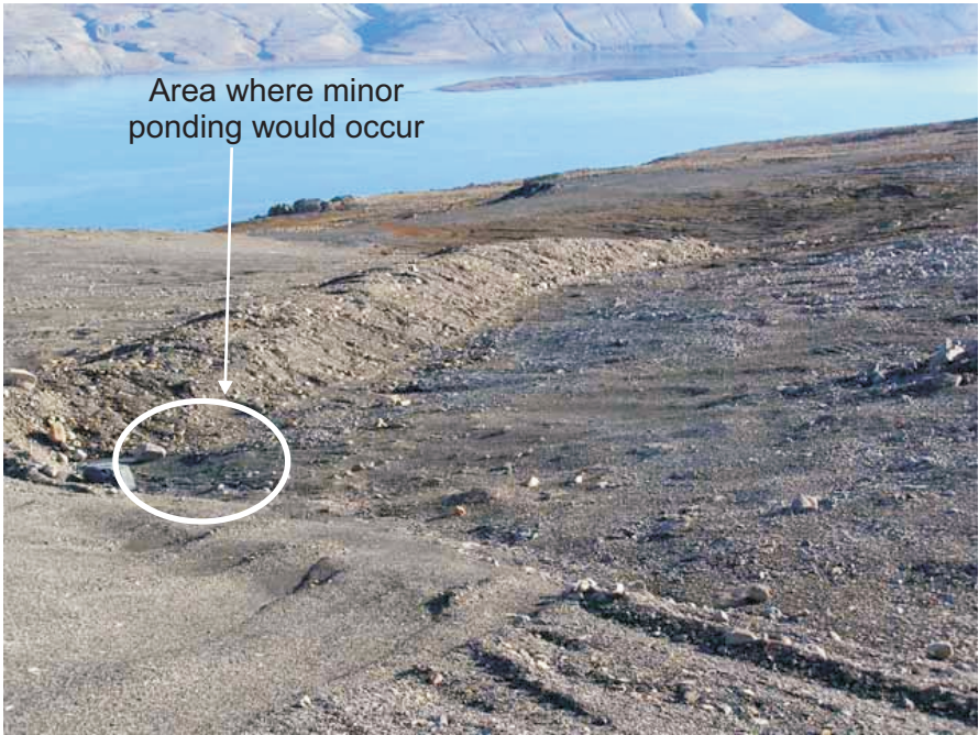
Photo 64 Water deflection berm at the Oceanview Portal cover.
