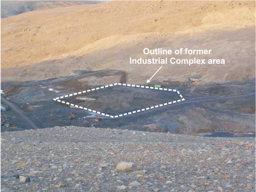
Photo 82 Industrial Complex as seen from Stol Port. Note all infrastructure has been removed and backfilling with metals contaminated soils is ongoing.
