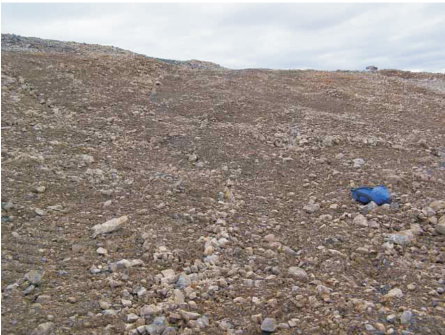
Photo 73 Area 14 Raise Cover. Note armour material applied to surface but no mound constructed.
