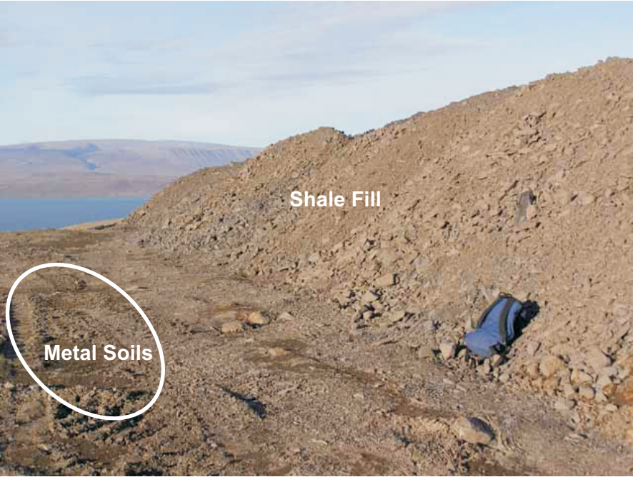
Photo 83 Stockpiled shale fill on top of metals contaminated soils in Industrial Complex foundation.
