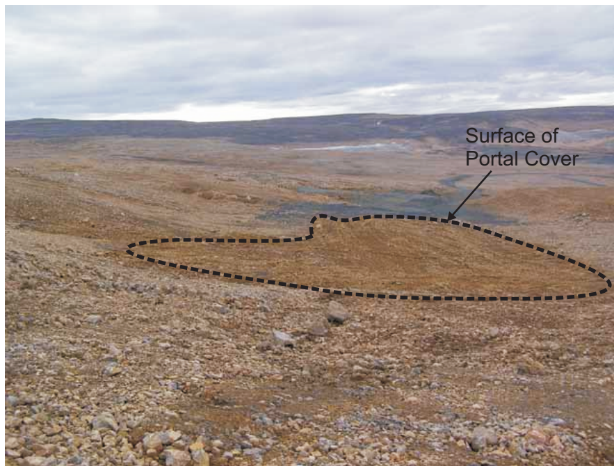
Photo 68 Armoured surface of Area 14 Portal Plug.
