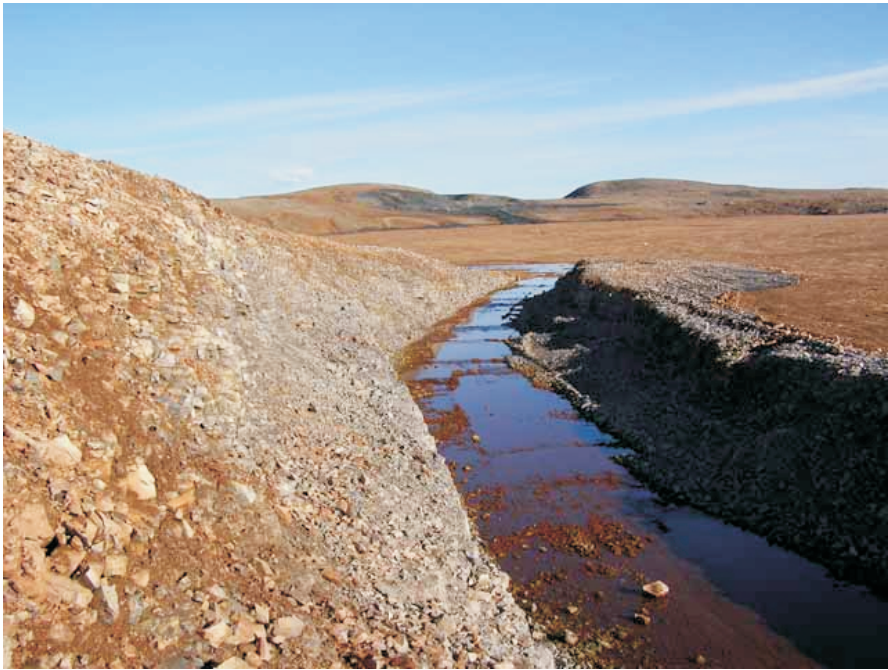
Photo 9 Flow through entrance area of West Twin Dike Spillway.
