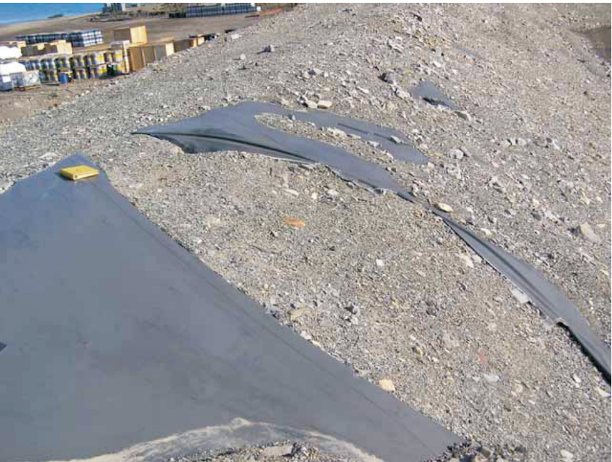
Photo 7 Exposures and tears of the internal liner.
