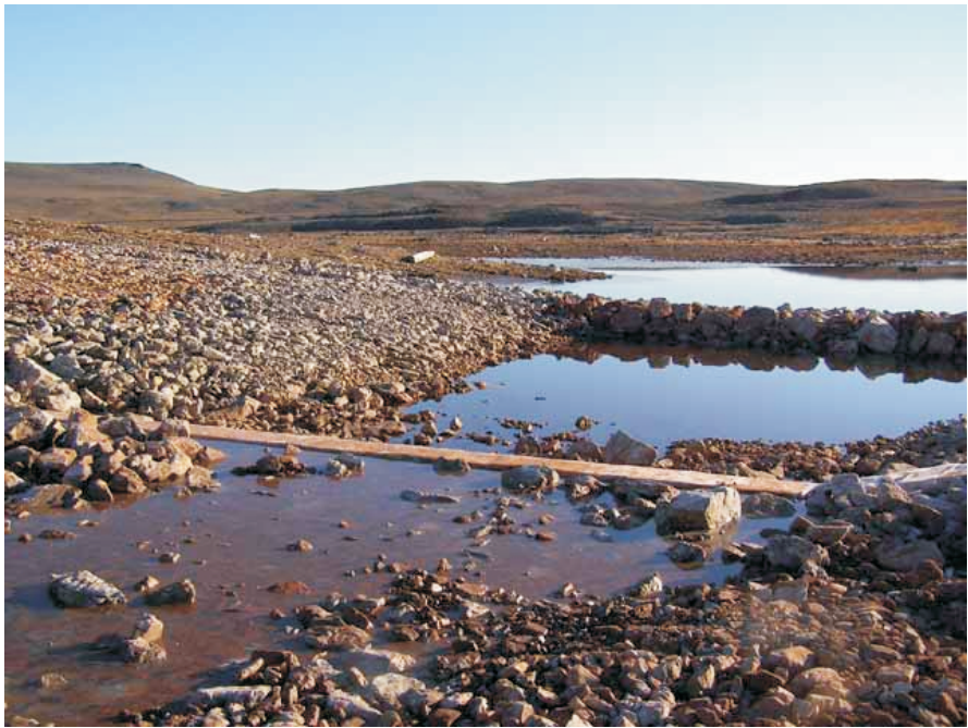
Photo 16 West Twin Outlet Channel after GCL installation. Note rising water level upstream of wall.
