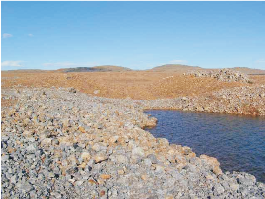
Photo 26 Rip rapped Test Cell outlet. Note riprap only applied to edge of water.
