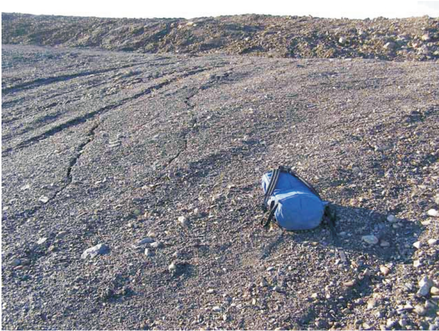
Photo 51 Cracking in southwest corner of Oceanview Open Pit cover.
