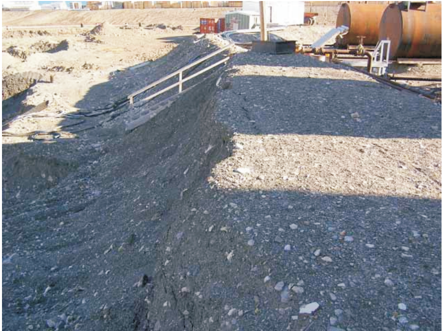
Photo 8 Affected area of Main Tank Farm berm which was partially excavated during reclamation of contaminated soils.
