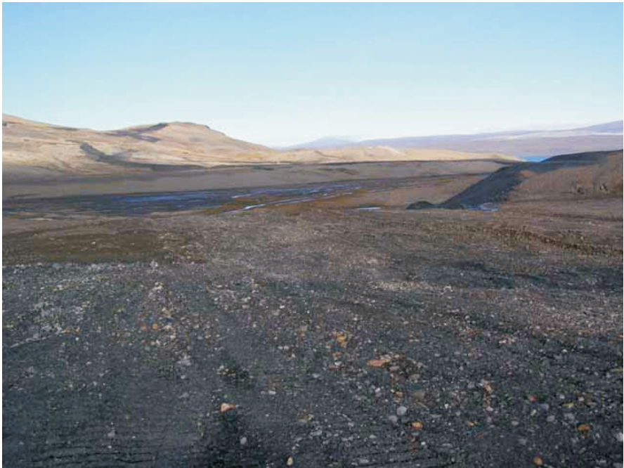
Photo 81 Kuhulu Lake Road armour material borrow area. Note floor of borrow area has been regraded.
