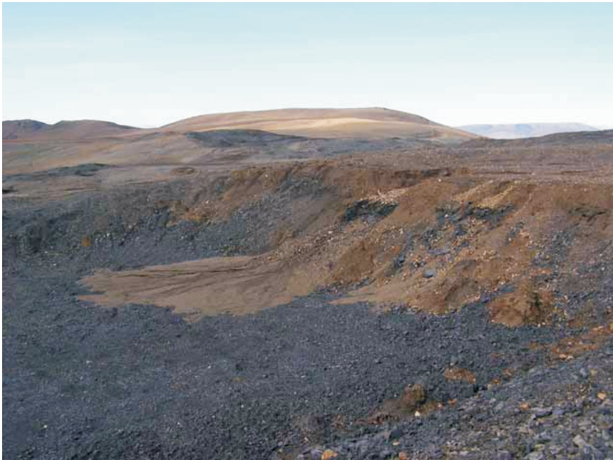
Photo 75 Area 14 Shale borrow area. Note erosion and subsequent deposition of overburden into bottom of pit. Similar to conditions observed in 2006.
