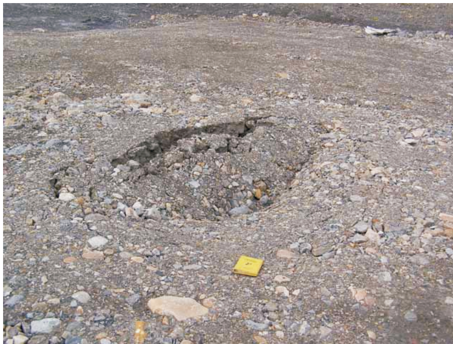
Photo 61 Thermokarst feature in 17N Portal Cover.
