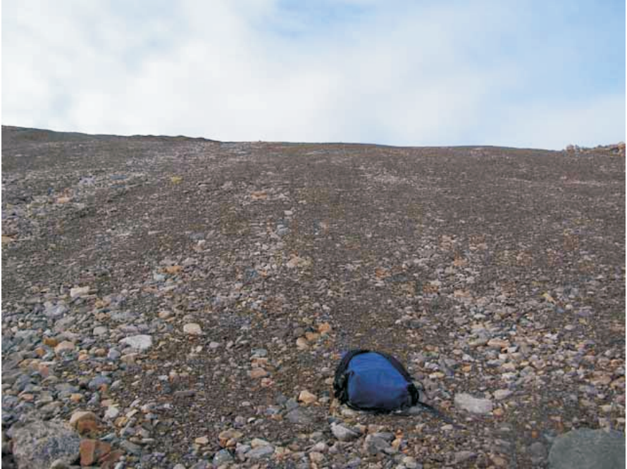
Photo 46 Looking upslope along steepest area of East Open Pit cover. Note no surface erosion observed.
