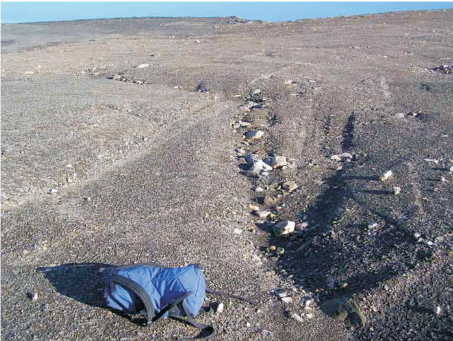
Photo 65 Minor erosion downslope of the upper corner of the surface water deflection berm.
