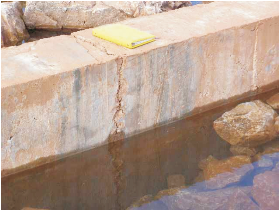
Photo 14 Crack in West Twin Outlet wall. View looking at downstream face of the concrete wall.
