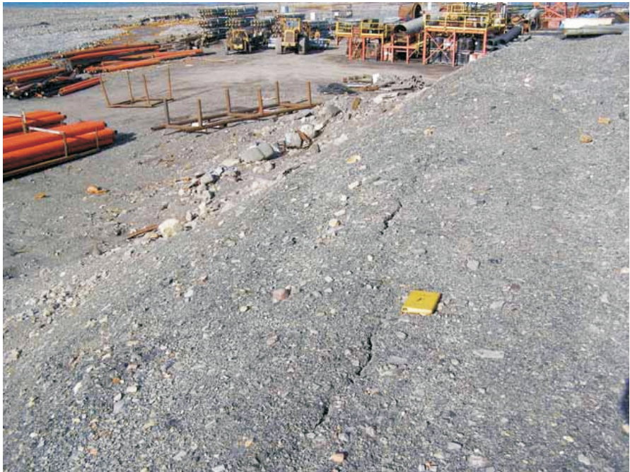
Photo 6 Cracking in crest of containment berm along west side of containment area.
