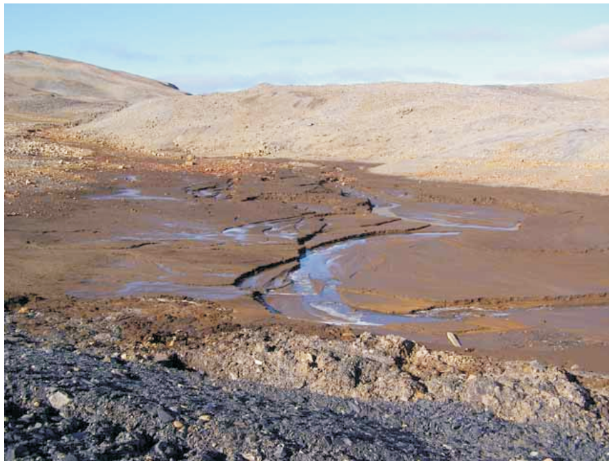
Photo 2 East Adit Treatment Pond. Note channelization of remnant sediments upstream of breach.
