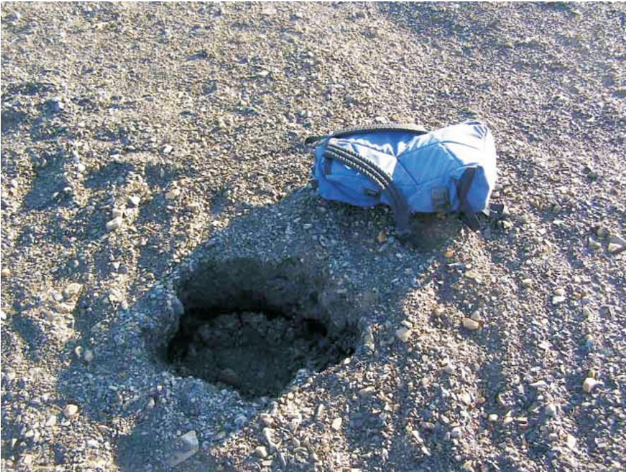
Photo 53 Small thermokarst feature in southeast corner of Oceanview Open Pit cover.
