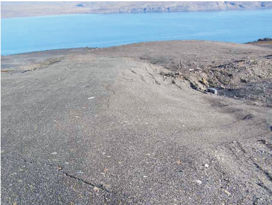
Photo 63 Oceanview Portal cover as seen from the upslope edge of the cover. Note minor cracking along the right (east) edge of the cover.
