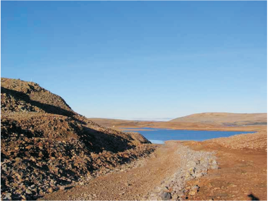
Photo 10 Bottom of spillway looking downslope. Note left (north) side of spillway has been riprapped as recommended in 2006.
