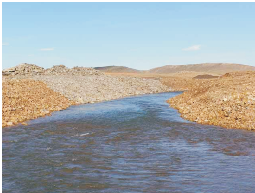
Photo 18 Flow through East Twin Creek Diversion Channel. Note area of channel rehab where light coloured armour rock was placed.
