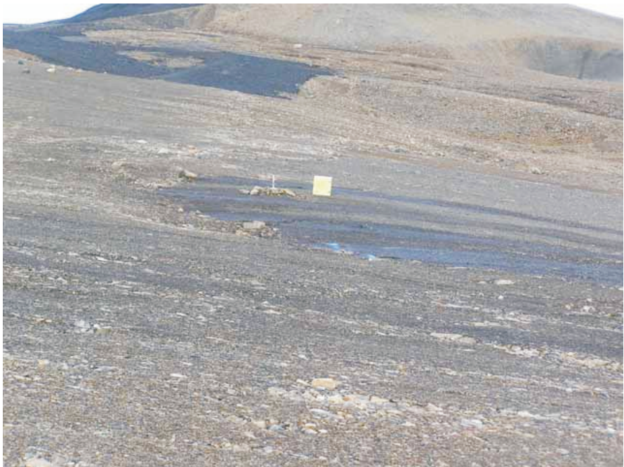
Photo 47 Intermediate level of East Open Pit Cover. Note dark area where seepage exits on face of cover.
