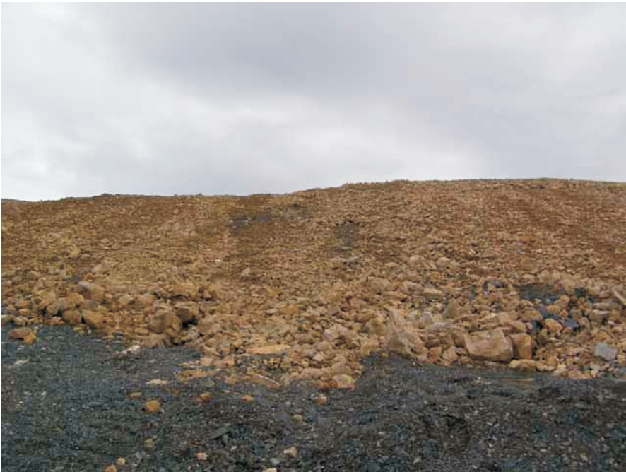
Photo 55 Armour placed at north edge of Area 14 waste rock cover.
