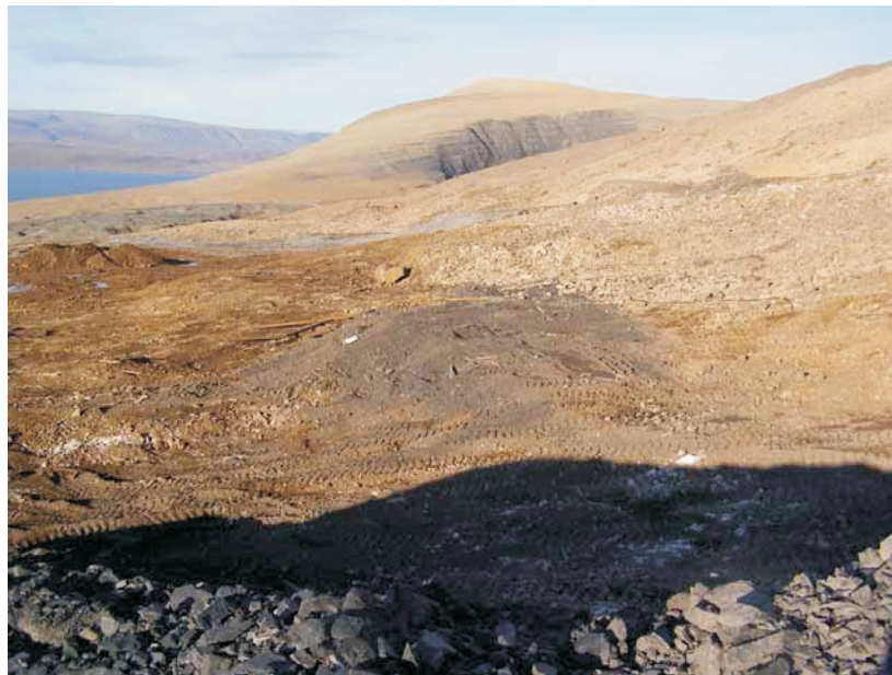
Photo 4 Former location of Day Tank Farm. Note berms have been excavated and liner and tanks have been removed.
