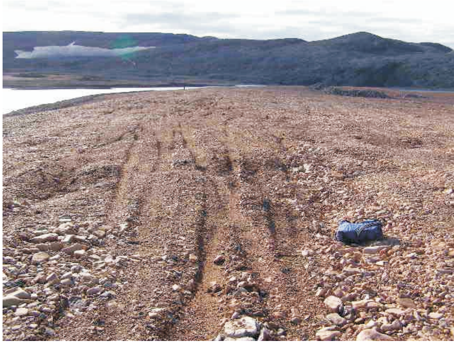
Photo 29 Surface of north/south arm of Test Cell dike. Note un-evenness and settlement of surface.
