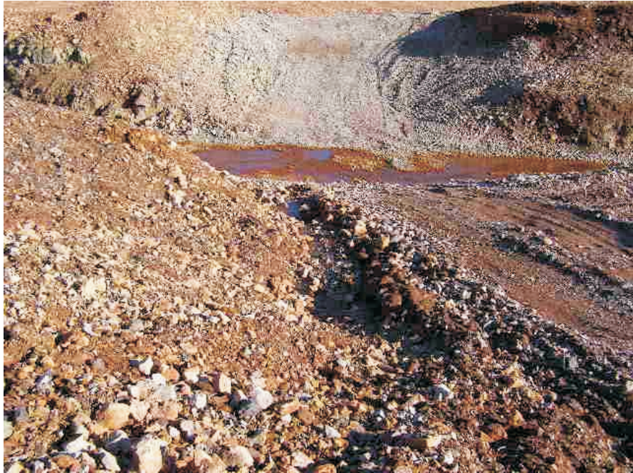
Photo 12 Access ramp into spillway. Note drainage path along edge of access ramp where flow enters the spillway.
