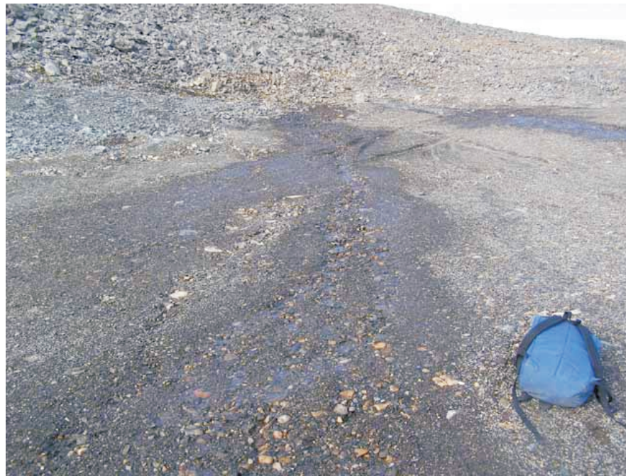
Photo 49 Very minor rill erosion on surface of East Trench cover.
