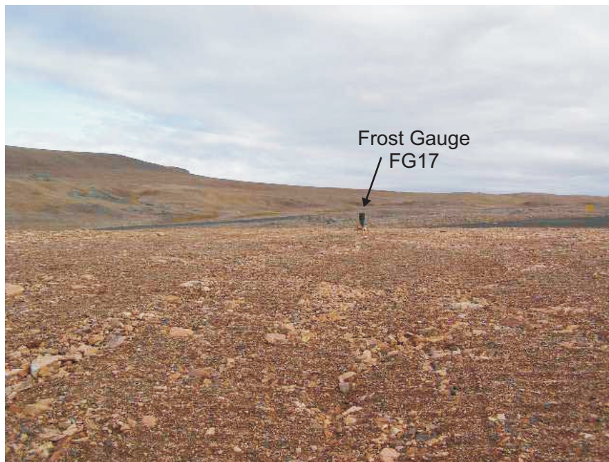
Photo 59 Surface of Upper Dump Pond tailings cover. Note frost gauge FG17 on surface of cover.
