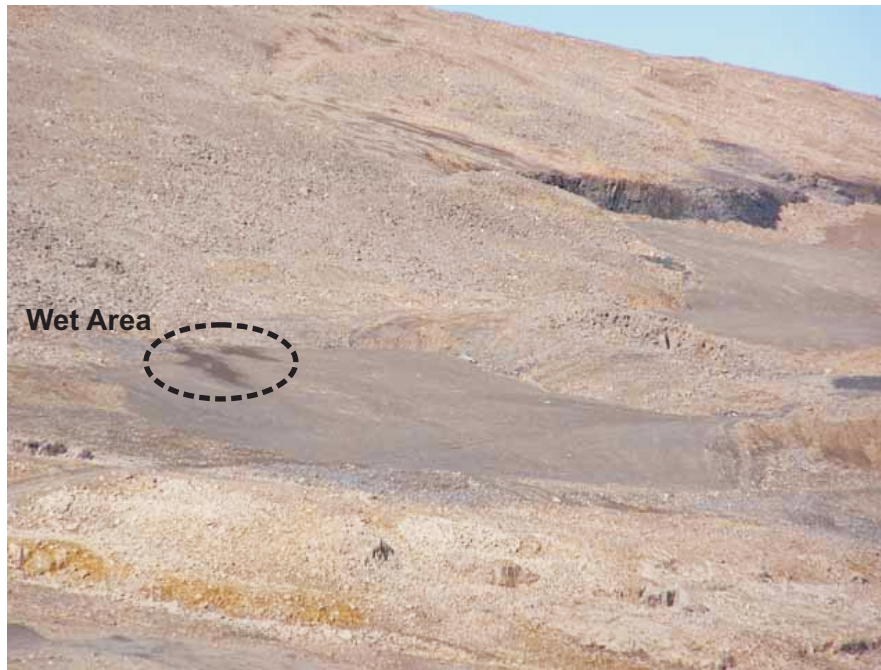
Photo 48 East Trench cover as seen from Kuhulu Lake road. Note the wet area near the top of the cover indicating some minor surface flow.
