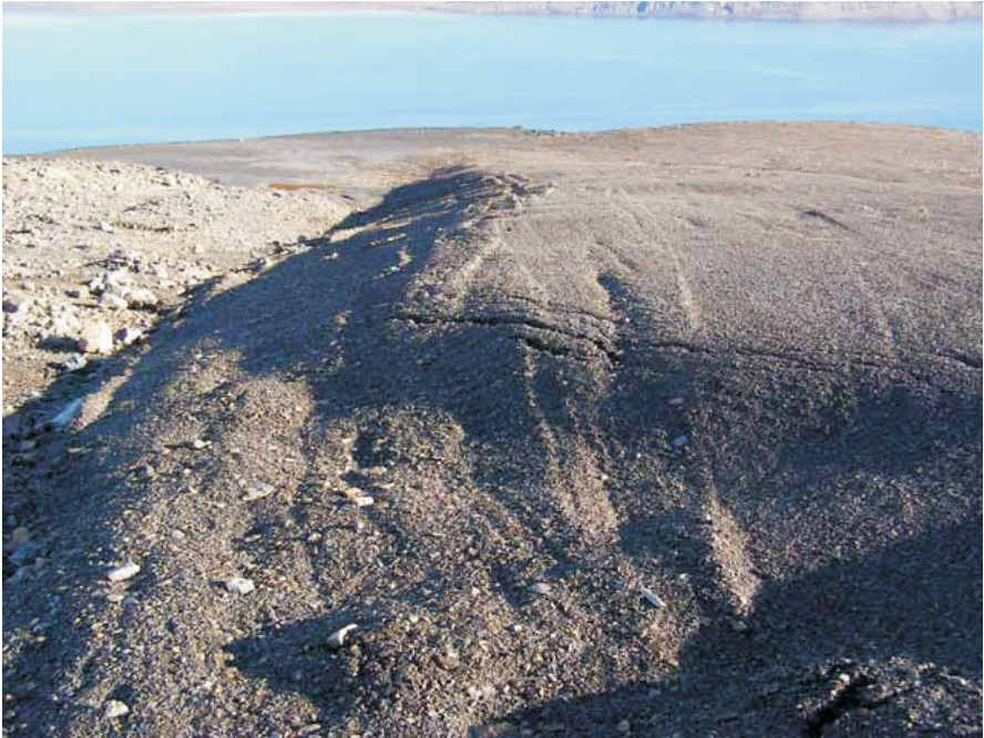
Photo 62 Settlement depression at the southwest corner of the Oceanview Portal cover.
