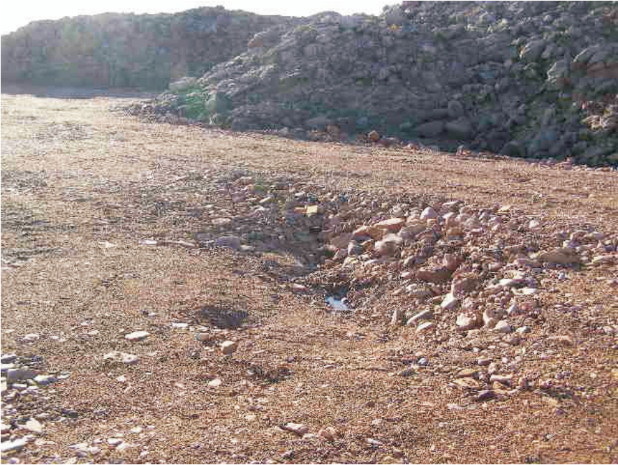
Photo 20 Thermokarst feature at south edge of Surface Cell cover.
