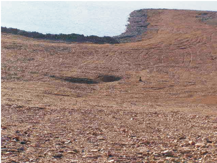
Photo 32 Thermokarst features adjacent to Thermistor 05-26 at toe of West Twin Dike. Note this was an area of excessive shale fill thickness.
