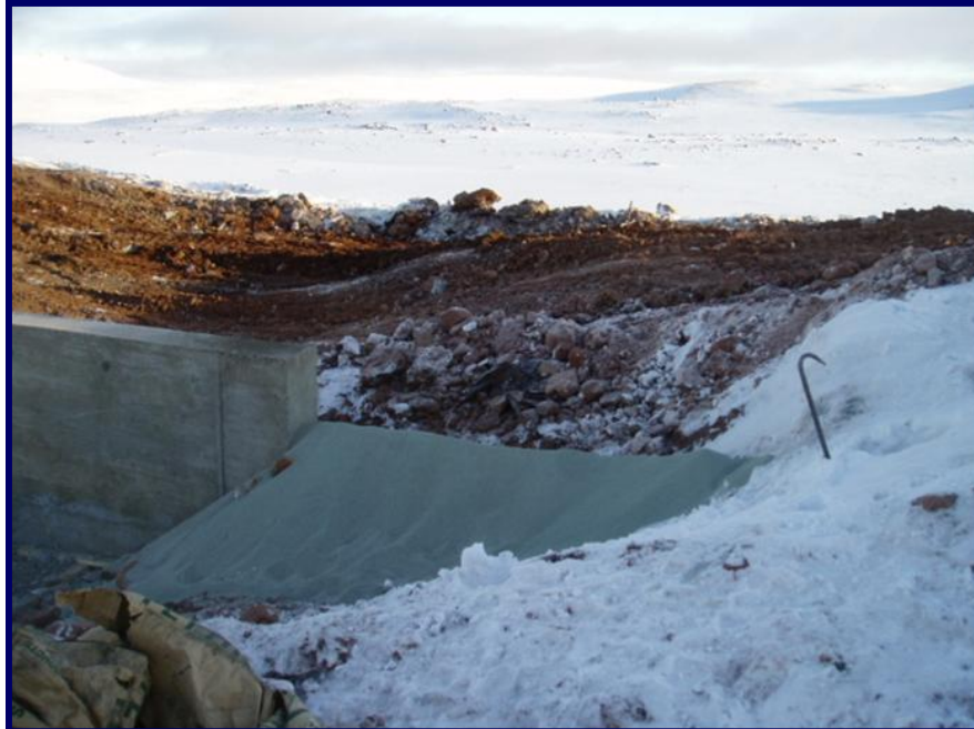
Photo 26 - October 7, 2005 Bentonite powder placed at the south abutment to 370.2 m elevation.
