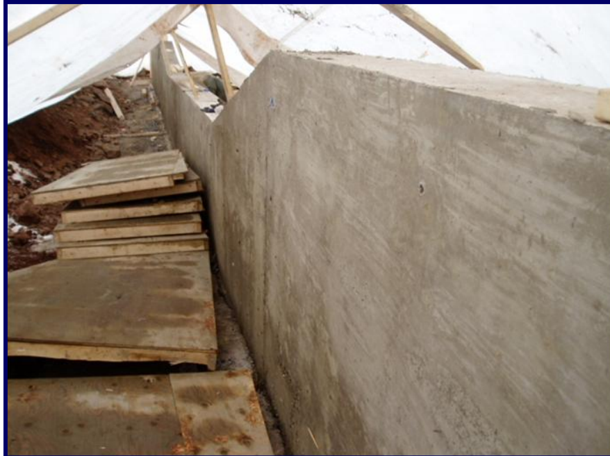
Photo 24 - October 3, 2005 Cut-off wall following the removal of the forms.
