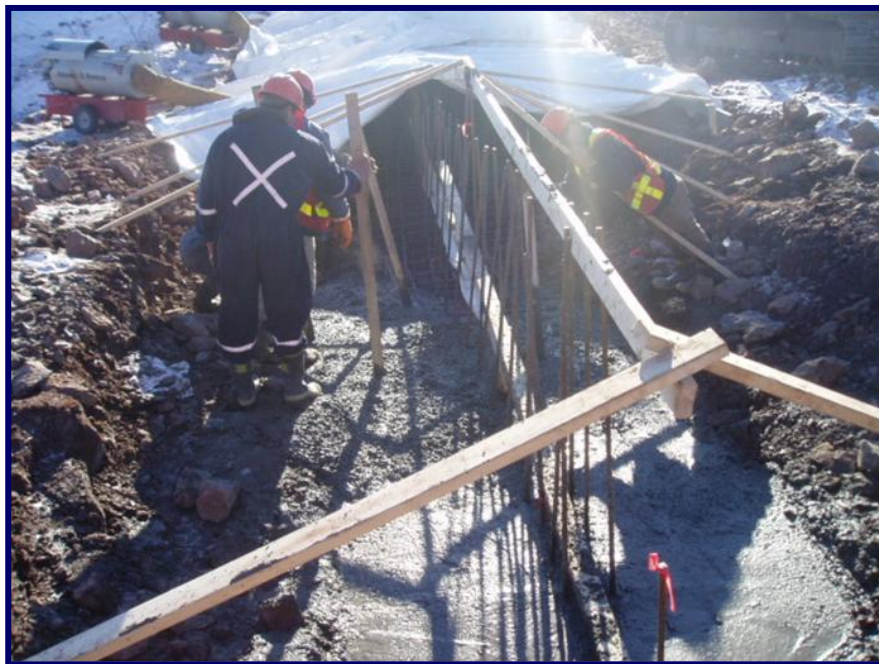
Photo 12 - September 20, 2005 Manually agitating concrete placed in foundation trench excavation.
