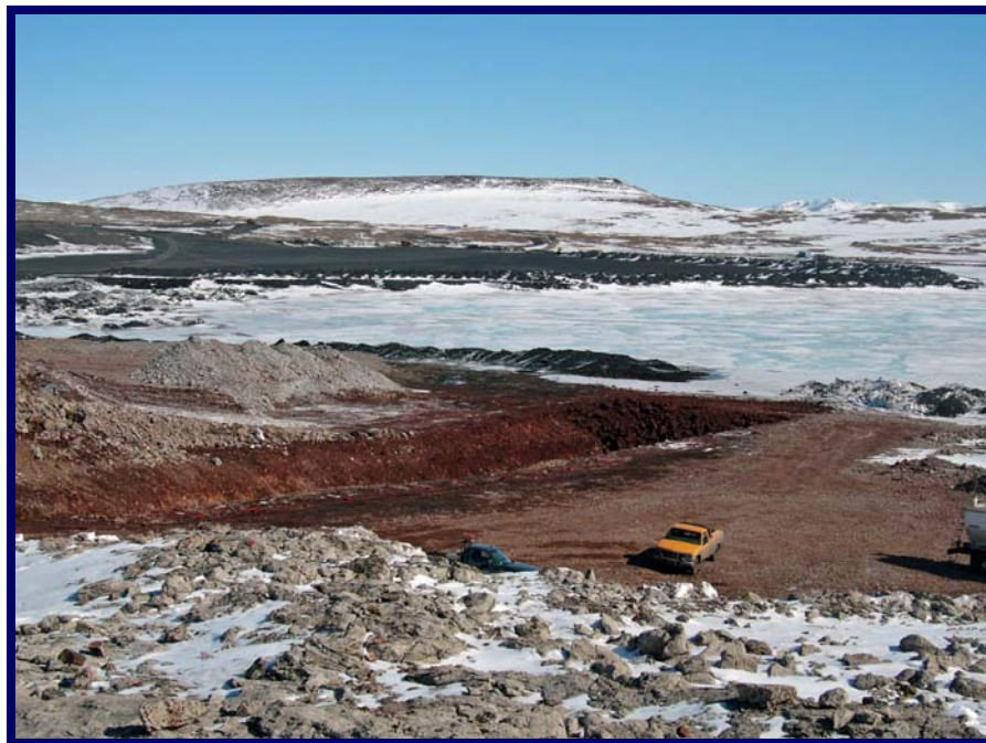
Photo 4 May 21, 2005 Stockpiling Type 1 riprap adjacent to spillway outlet.
