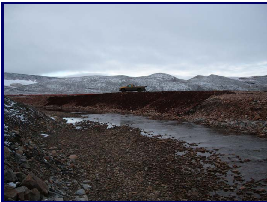
Photo 4 - September 2005 Regraded portion of East Twin Creek Diversion Channel Dike.
