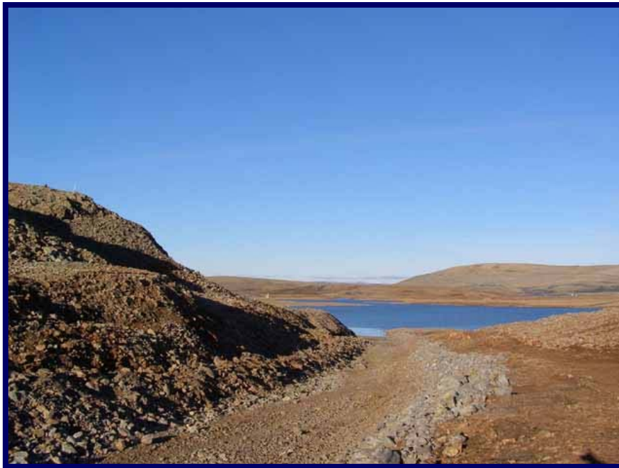
Photo 32 August 31, 2007 Bottom of Spillway looking downslope. Note riprap applied to left side of spillway.
