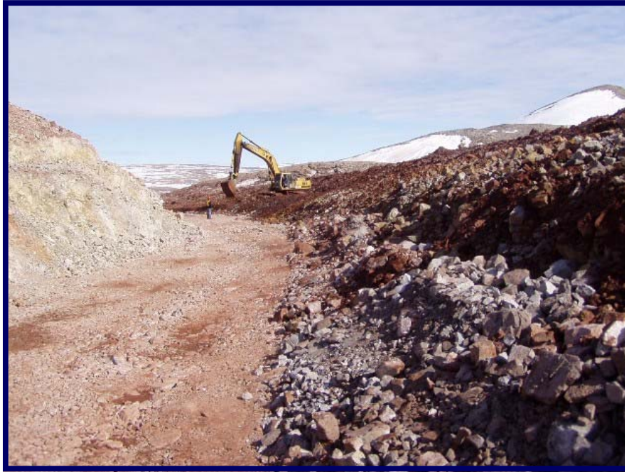
Photo 31 Applying Type 1 riprap to right hand side of spillway channel through chute section.
