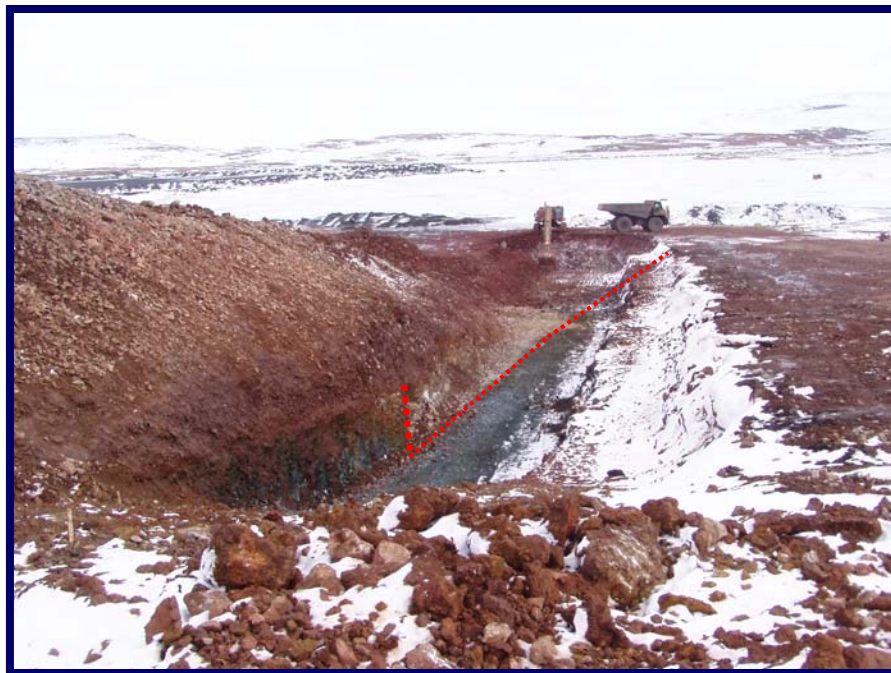
Photo 16 May 19, 2005 Initial excavation of lower portion of spillway chute. Note transition between dark green diabase and grey dolostone in sidewall and base of spillway.
