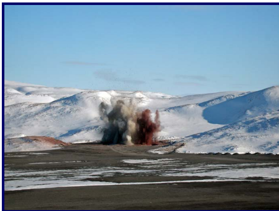
Photo 2 May 14, 2005 Blast at spillway.
