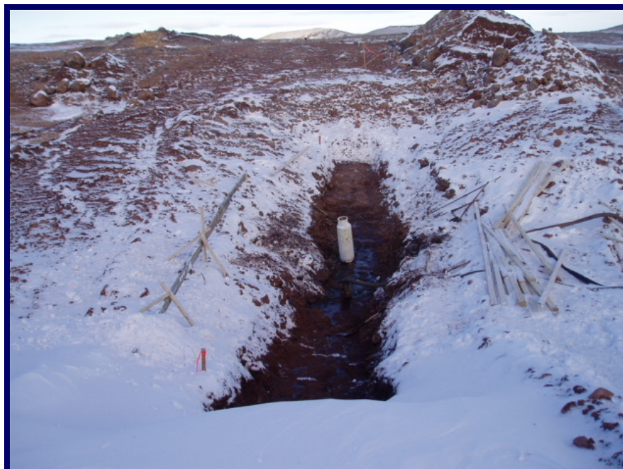
Photo 4 - September 2005 De-watered outlet trench.
