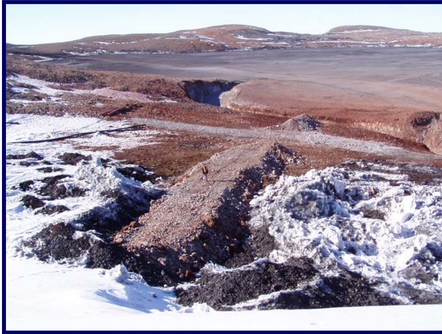
Photo 33 May 27, 2005 Water deflection berm near spillway access ramp. Note person on berm for scale.
