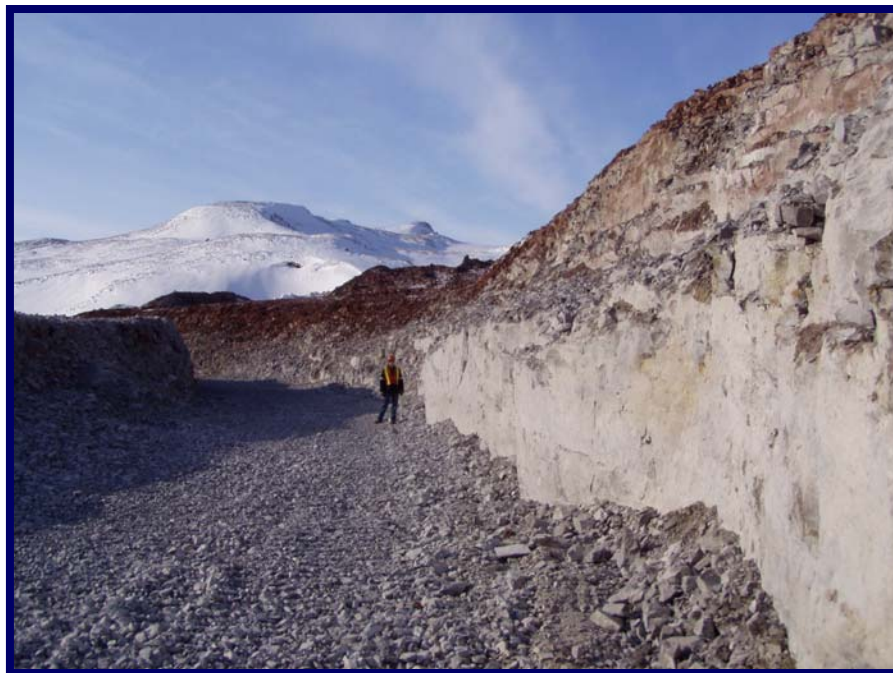
Photo 8 May 18, 2005 Excavated spillway channel near inlet Note near vertical intact bedrock on right side of photo. Also note bench constructed near mid-point of slope on right side of photo.
