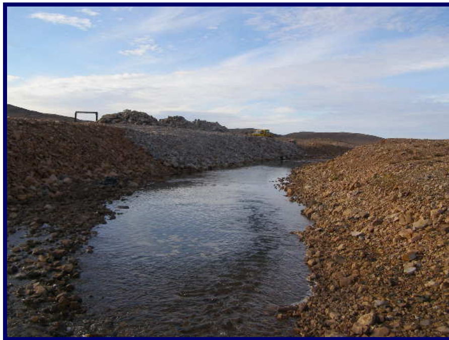
Photo 6 - August 2006 View looking downstream. Armoured section of diversion dike.
