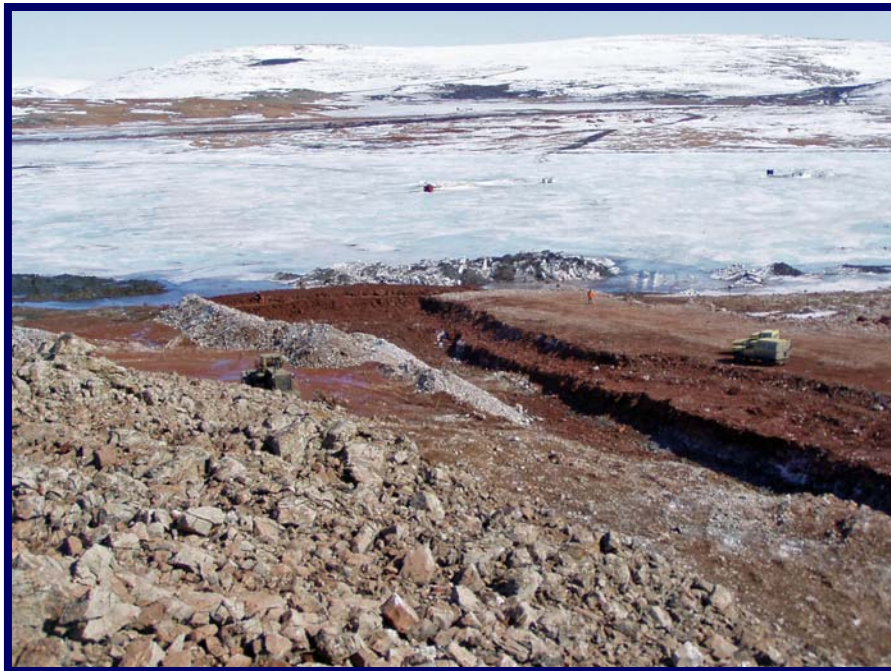
Photo 28 May 25, 2005 Excavated spillway outlet channel. Note plug left at outlet to keep area from backflooding.
