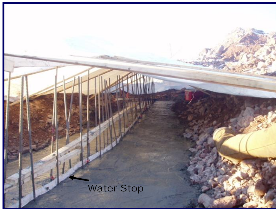
Photo 15 - September 20, 2005 Completed concrete pour in foundation trench. Note the water stop placed into the foundation.
