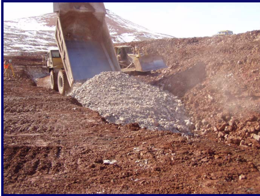
Photo 21 Type 2 May 27, 2005 Backfilling spillway chute with Type 1 riprap.
