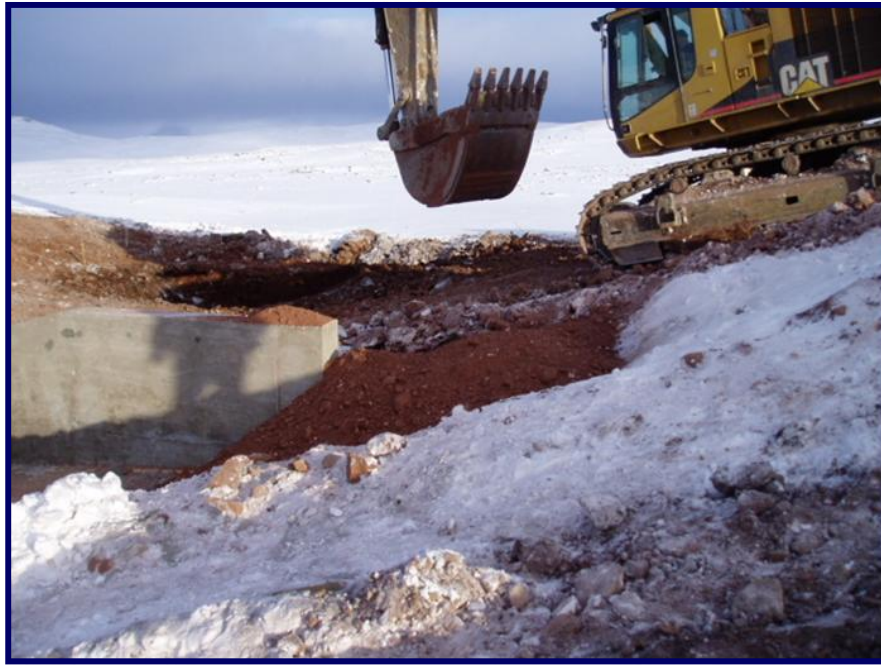
Photo 27 - October 7, 2005 Screened sand and gravel placed at the south abutment on top of the bentonite powder.
