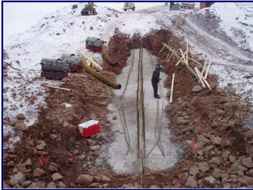
Photo 17 - September 23, 2005 Cured concrete in foundation trench. Preparing to construct rebar mesh for cut-off wall.
