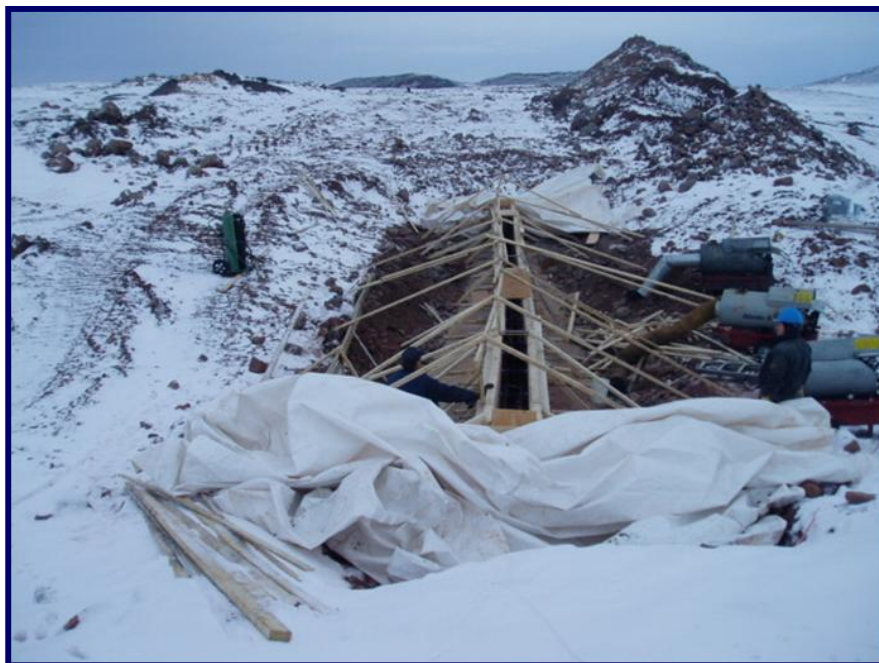
Photo 20 - September 29, 2005 The form constructed for the cut-off wall.
