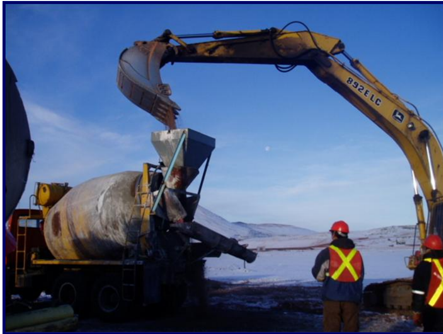
Photo 9 - September 20, 2005 Excavator adding aggregate to the concrete mixer.
