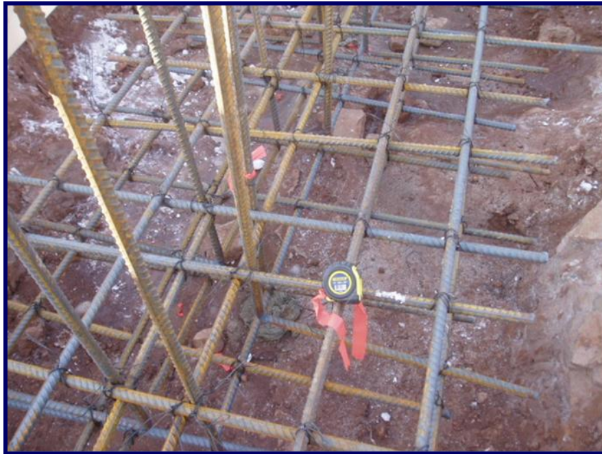
Photo 7 - September 17, 2005 Close up view of the rebar mesh constructed for the foundation trench.
