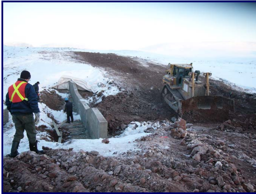
Photo 31 - October 7, 2005 D8 dozer further removing materials downstream of cut-off wall down to bedrock.
