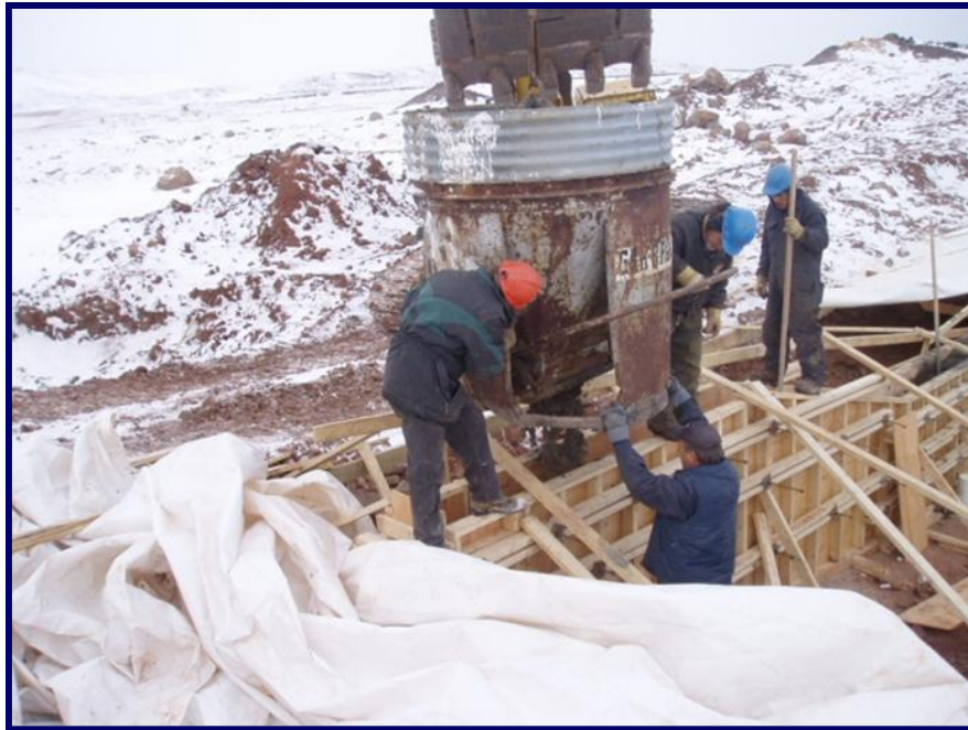
Photo 21 - September 29, 2005 Placing concrete into forms to construct the cut-off wall.
