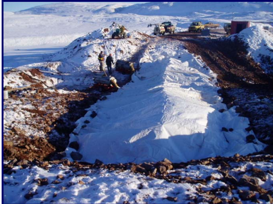
Photo 16 - September 20, 2005 Tarps and heaters used to allow the concrete to cure after the concrete pour in foundation trench.
