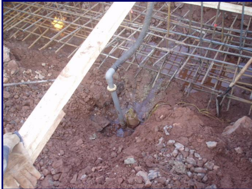
Photo 8 - September 19, 2005 Sump area and submersible pump used to de-water the foundation trench excavation .
