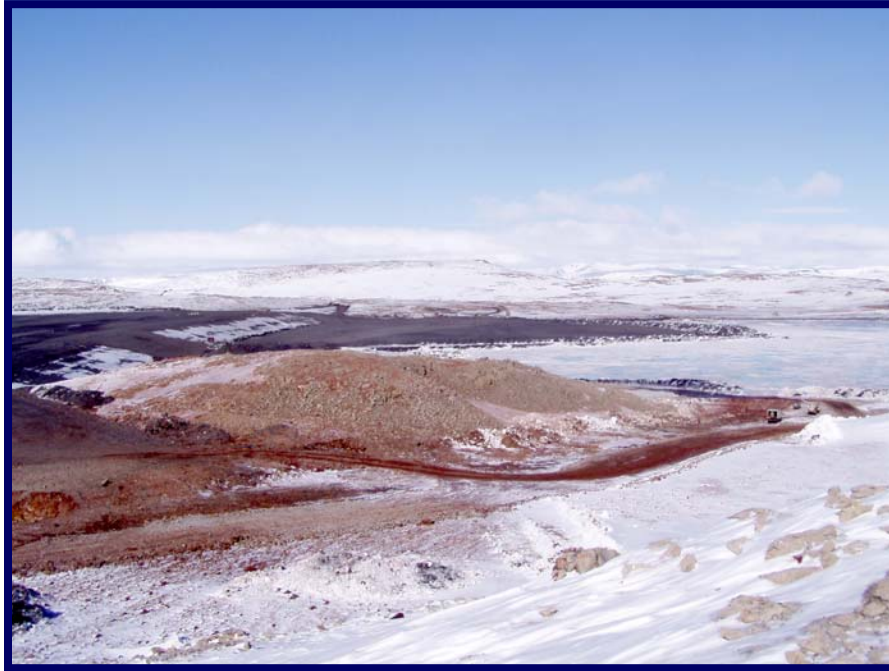
Photo 25 May 17, 2005 Dolostone outcrop on left hand side of spillway excavation prior to benching.
