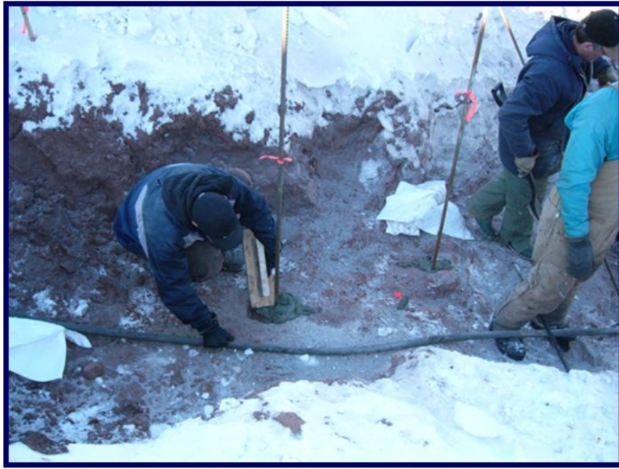
Photo 5 - September 12, 2005 Grouting of the dowels into competent bedrock in foundation trench.
