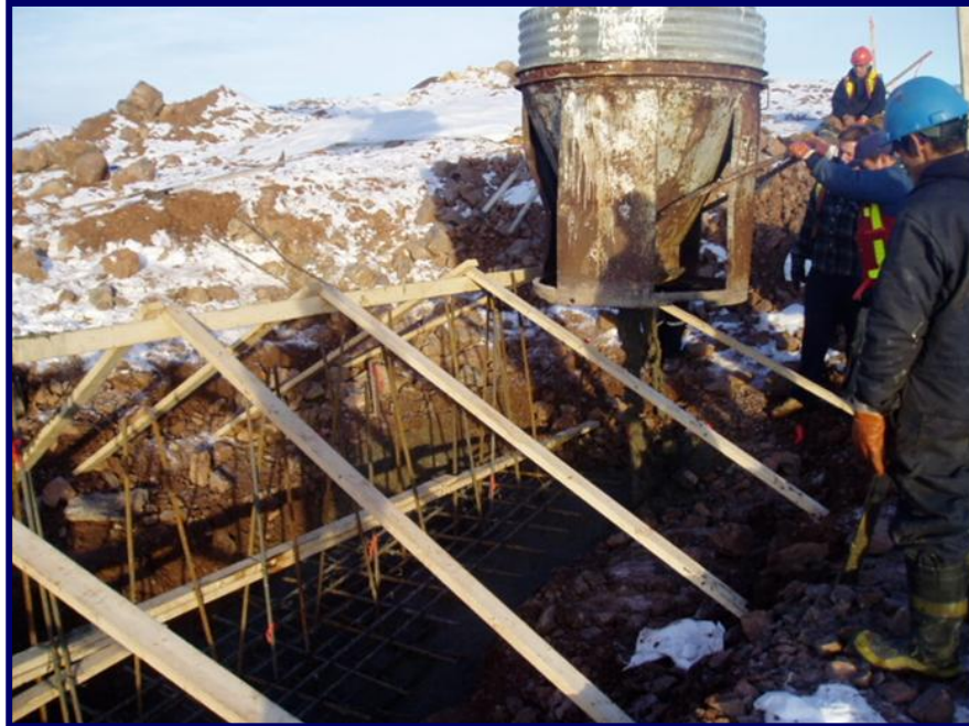
Photo 10 - September 20, 2005 Concrete hopper used to place the concrete in the foundation trench excavation.
