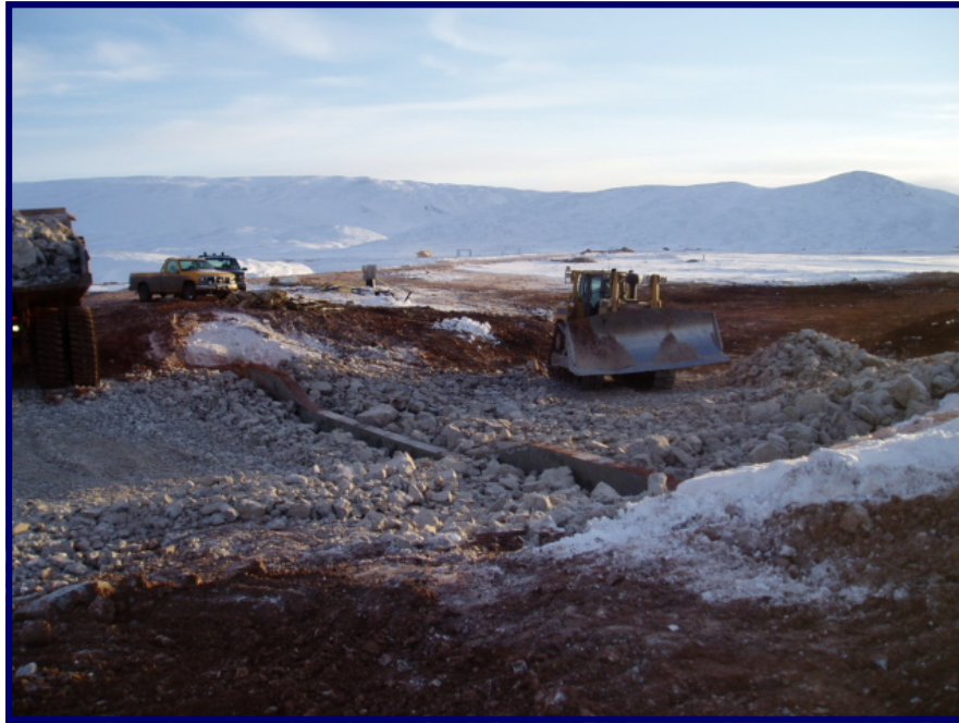
Photo 33 - October 8, 2005 Placement of riprap upstream of cut-off wall.
