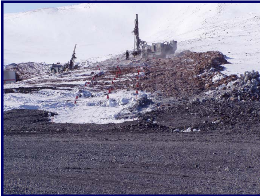
Photo 1 May 15, 2005 Drilling for subsequent blast at spillway inlet. Note cones identifying drill holes.
