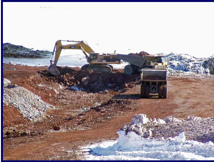
Photo 27 May 25, 2005 Excavation of spillway outlet channel.
