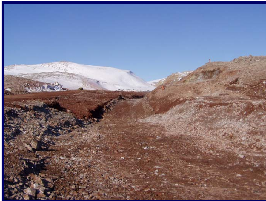
Photo 20 May 26, 2005 Backfilled spillway excavation with Type 2 riprap.
