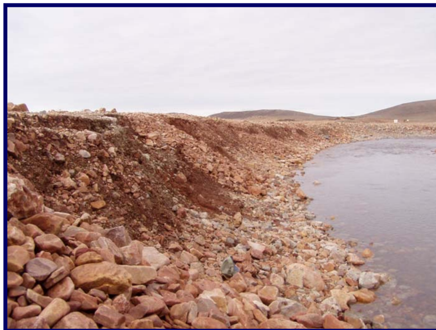
Photo 2 - July 2004 East Twin Diversion Channel prior to reclamation. Close up view of area of erosion on face of dike.
