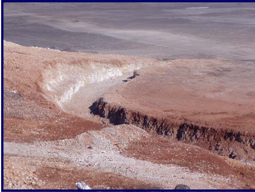
Photo 11 May 25, 2005 View of inlet portion of spillway. Note transition between red stained frost affected bedrock and grey intact bedrock.
