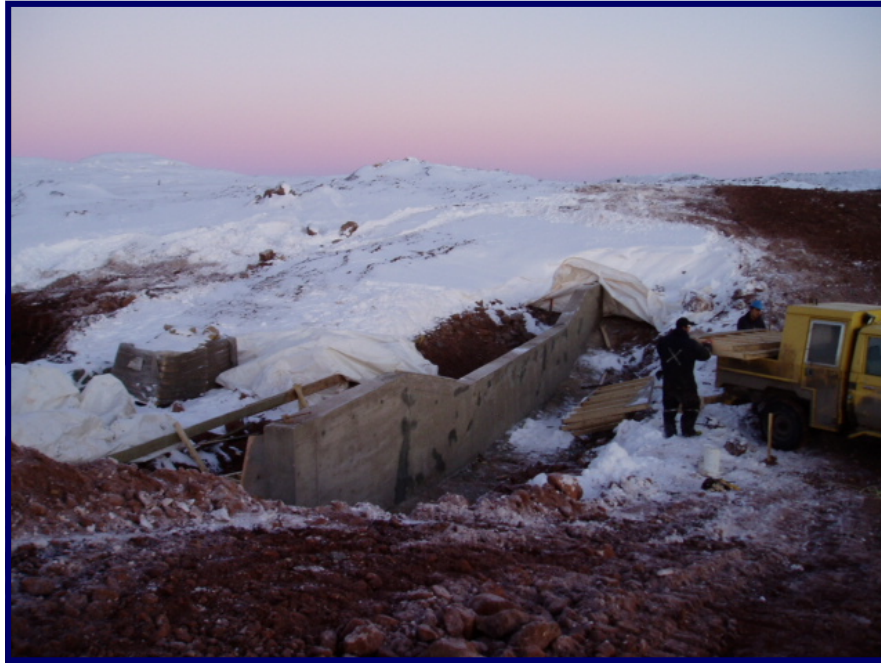
Photo 25 - October 3, 2005 Cut-off wall following the removal of the forms.
