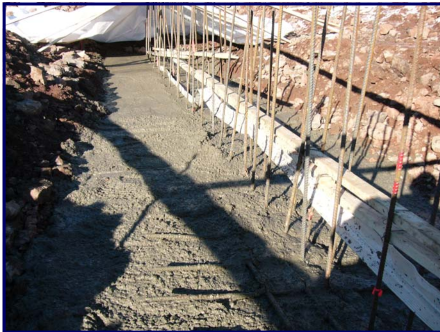
Photo 14 - September 20, 2005 Concrete placed in foundation trench.
