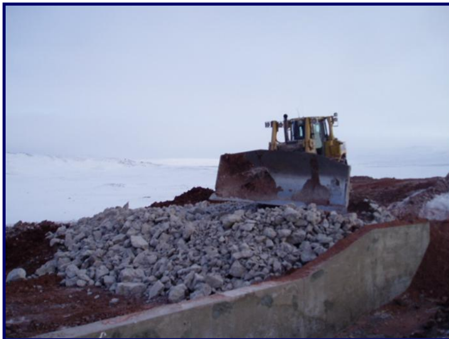
Photo 32 - October 7, 2005 Dozer placing the riprap at the Outlet Channel.
