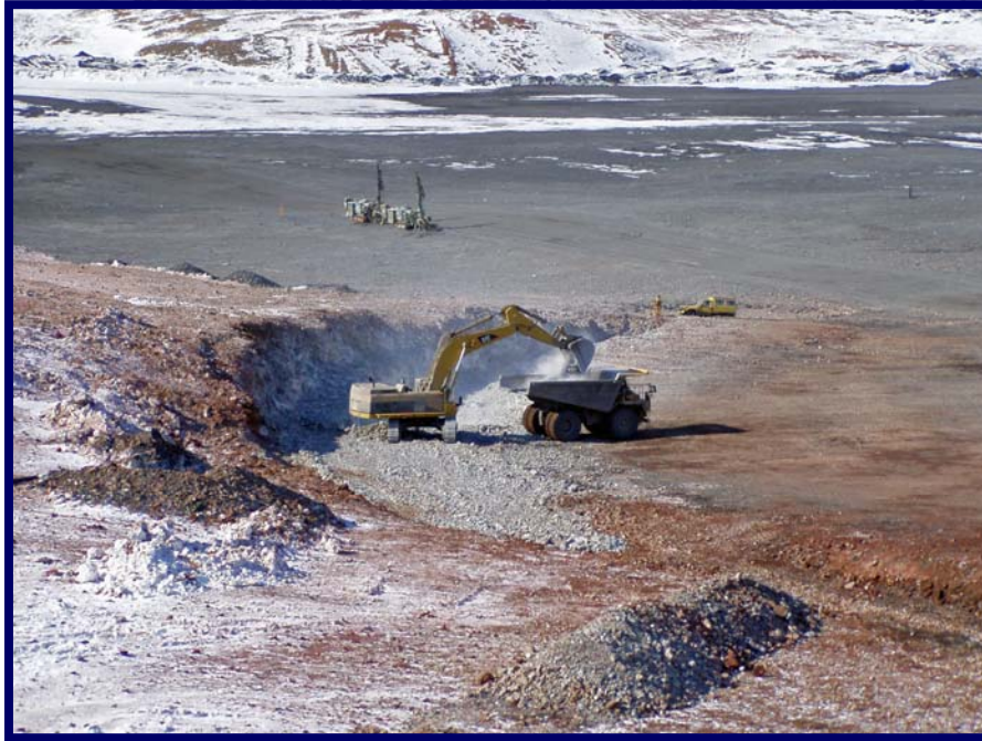
Photo 7 May 17, 2005 Excavating material from inlet portion of spillway.
