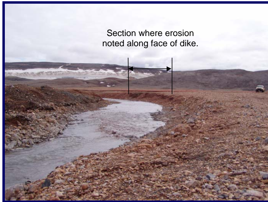
Photo 3 - July 2004 View looking upstream. Note area of erosion on dike.
