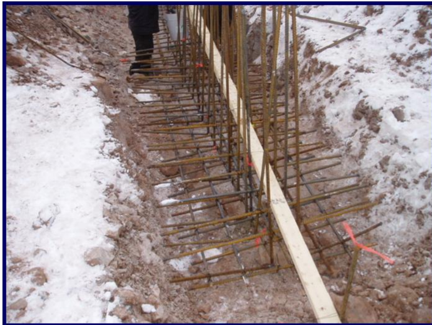
Photo 6 - September 14, 2005 Rebar mesh constructed for the foundation trench.
