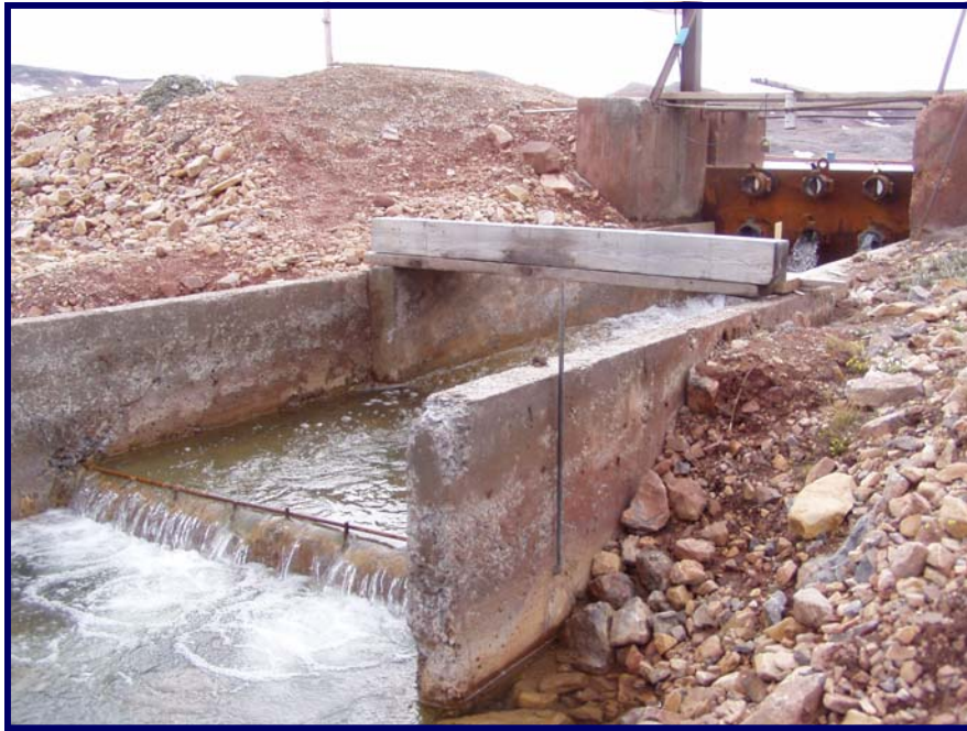
Photo 1 - July 2004 Previous concrete outlet structure.
