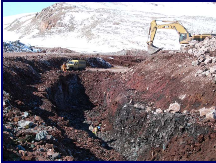
Photo 17 May 21, 2005 Excavation of upper portion of spillway chute. Note poor quality of rock in sidewall of excavation.
