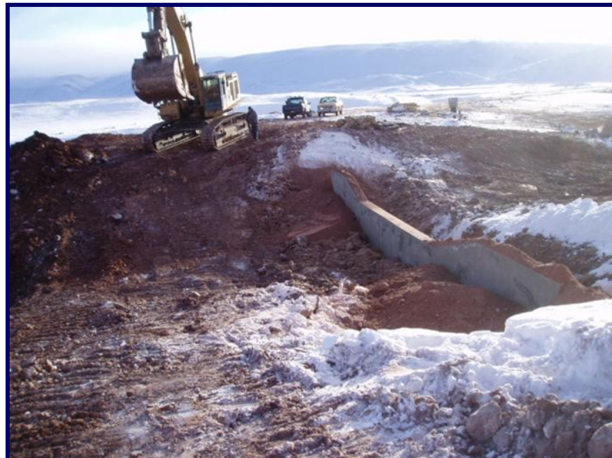
Photo 28 - October 7, 2005 Excavator placing sand and gravel adjacent to the cut-off wall.
