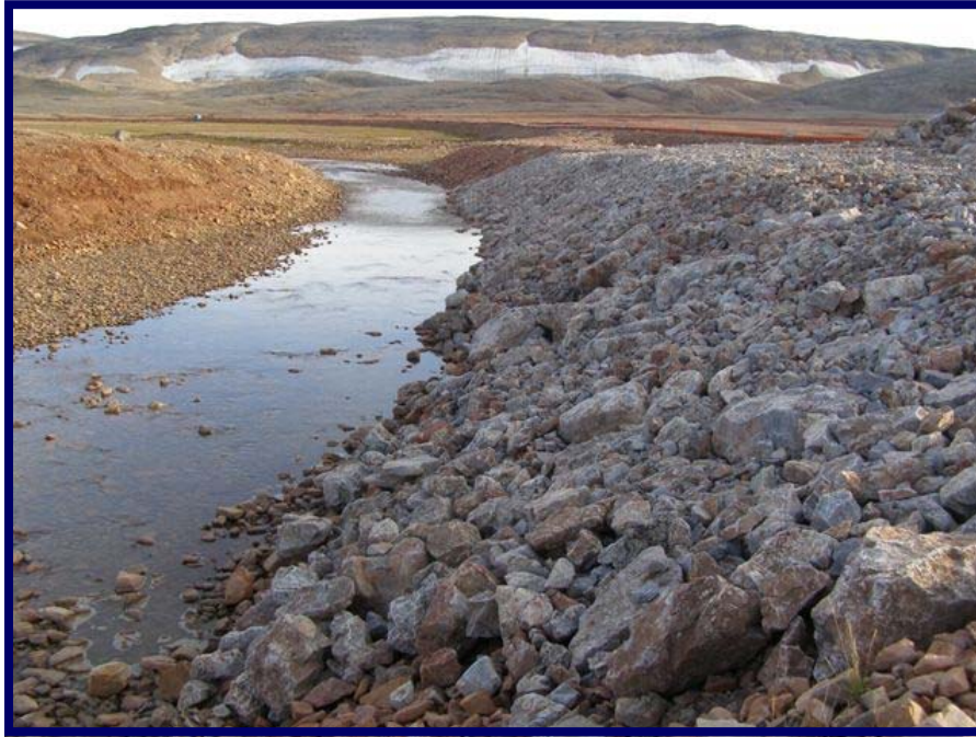
Photo 5 - August 2006 View looking upstream. Armoured section of diversion dike. Note grain size distribution of rockfill.
