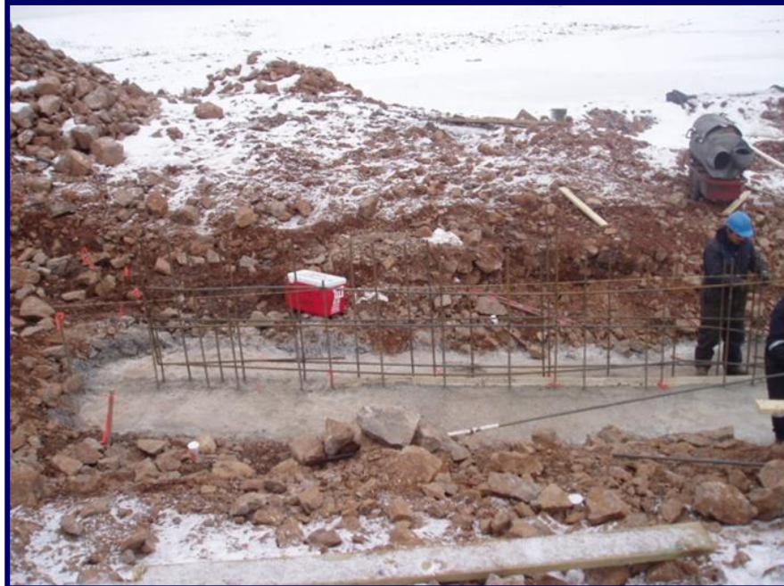
Photo 18 - September 23, 2005 Horizontal rebar constructed for the cut-off wall.
