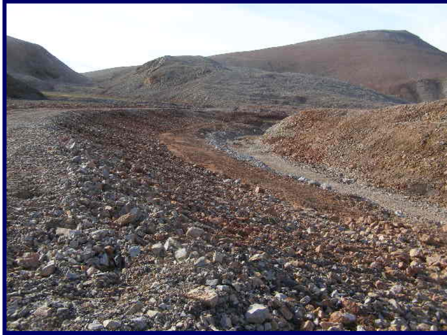
Photo 23 - August 2006 View of overburden bench on right hand side of spillway excavation.
