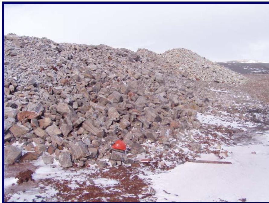
Photo 6 May 20, 2005 Stockpile of Type 1 riprap. Note hard hat for scale.
