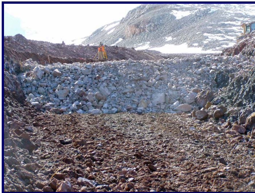
Photo 22 May 27, 2005 Backfilling spillway chute with Type 1 riprap.
