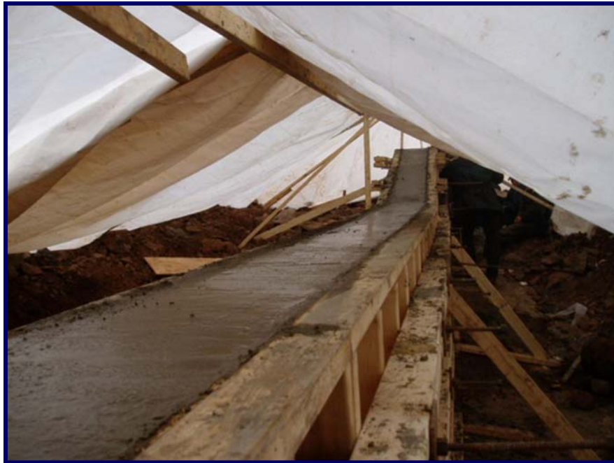
Photo 23 - September 29, 2005 Concrete placed in the cut-off forms.
