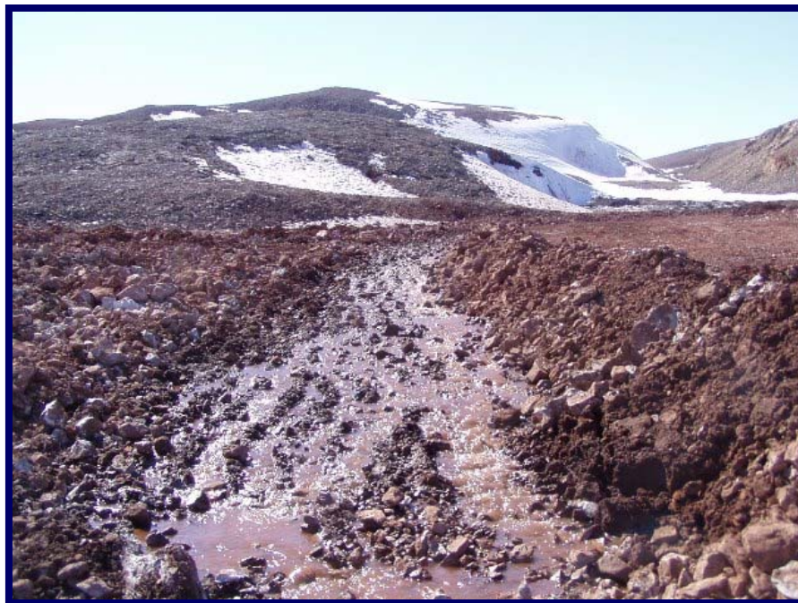
Photo 34 June 10, 2005 Water diversion ditch adjacent to access road.
