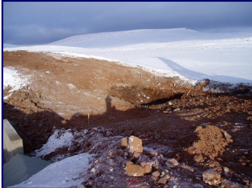
Photo 30 - October 7, 2005 Excavation of the stilling pool downstream of cut-off wall.
