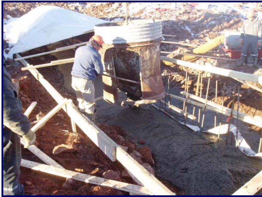
Photo 11 - September 20, 2005 Concrete being placed into the foundation trench excavation.
