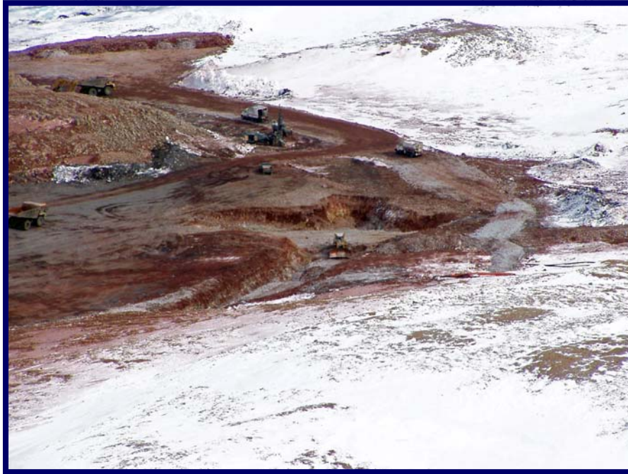
Photo 13 May 18, 2005 Access ramp between inlet and chute portions of spillway.
