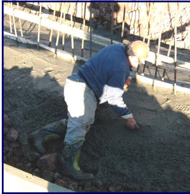
Photo 13 - September 20, 2005 Manually finishing, concrete around rebar in foundation trench.
