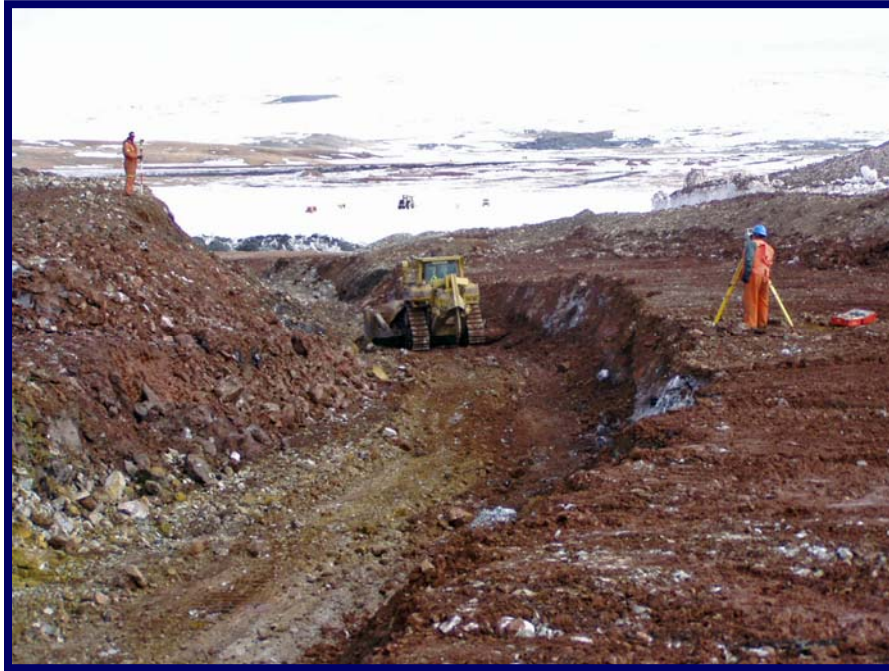
Photo 19 May 26, 2005 Backfilling chute portion of spillway with Type 2 riprap.
