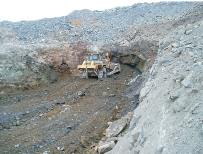
Photo 3 - 88 Portal partially backfilled. Date: August 1, 2005
