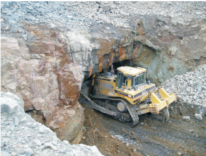
Photo 2 - D8 placing fill inside the 88 Portal. Date: August 1, 2005
