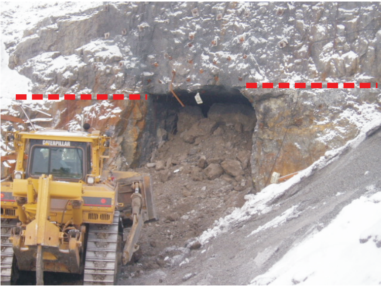
Photo 2 - 00 Portal partially closed. Date: October 2, 2005
