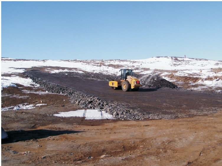
Photo 2 - Compacting initial lift of shale for Oceanview Portal cover. Date: May 28, 2005
