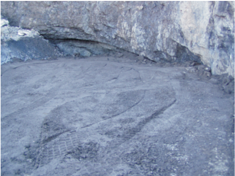
Photo 4 - Coarse fill in 38-11 stope after levelling. Date: July 3, 2005
