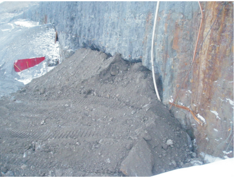
Photo 3 - Backfilled 01 Portal. Date: September 30, 2005
