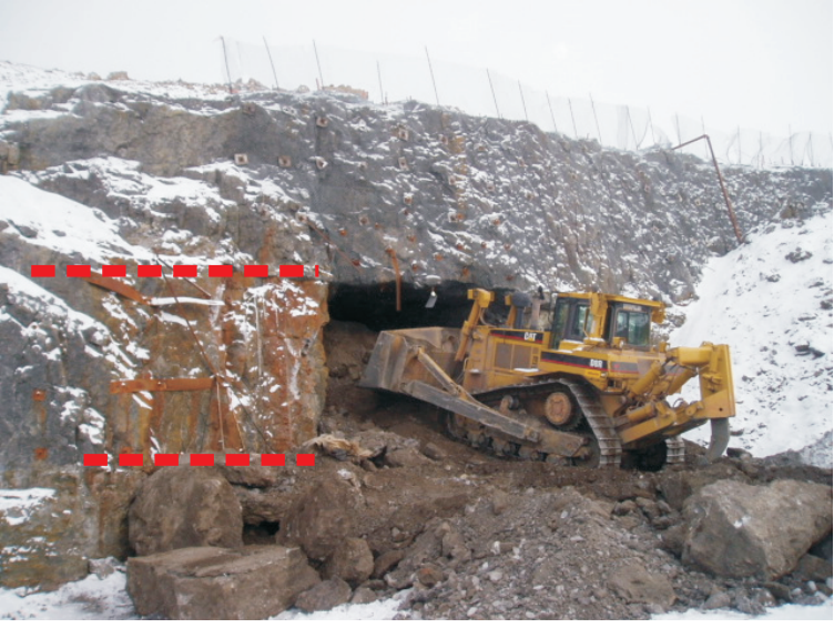
Photo 3 - D8 placing waste rock into the 00 Portal. Date: October 2, 2005
