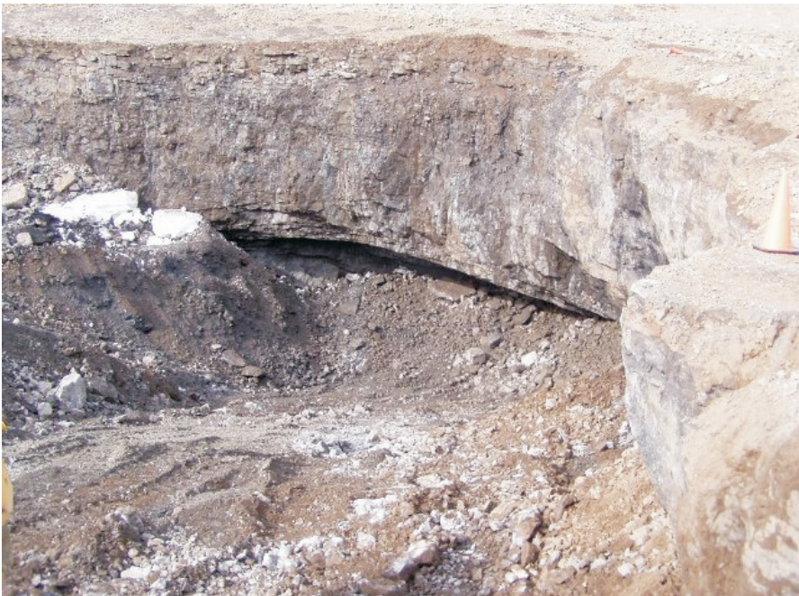
Photo 2 -38-11 stope opening after partial backfilling. Date: June 27, 2005
