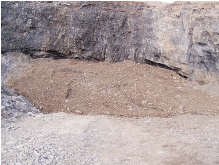
Photo 3 - Backfilling 38-11 stope. Date: July 9, 2005
