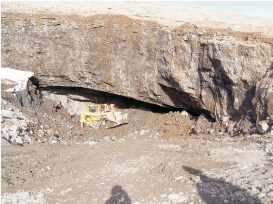
Photo 1 - Backfilling 38-11 stope opening. Date: June 27, 2005
