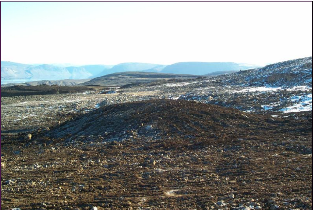
VIEW OF SHALE CAP ON OCEANVIEW EAST RAISE POST-RECLAMATION (SEPTEMBER 2002).
