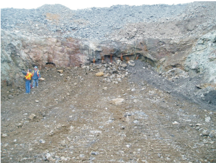
Photo 5 - 88 Portal completely backfilled with waste rock. Date: August 1, 2005
