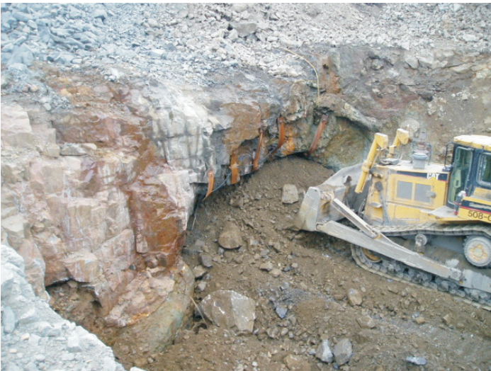
Photo 4 - 88 Portal partially backfilled. Date: August 1, 2005
