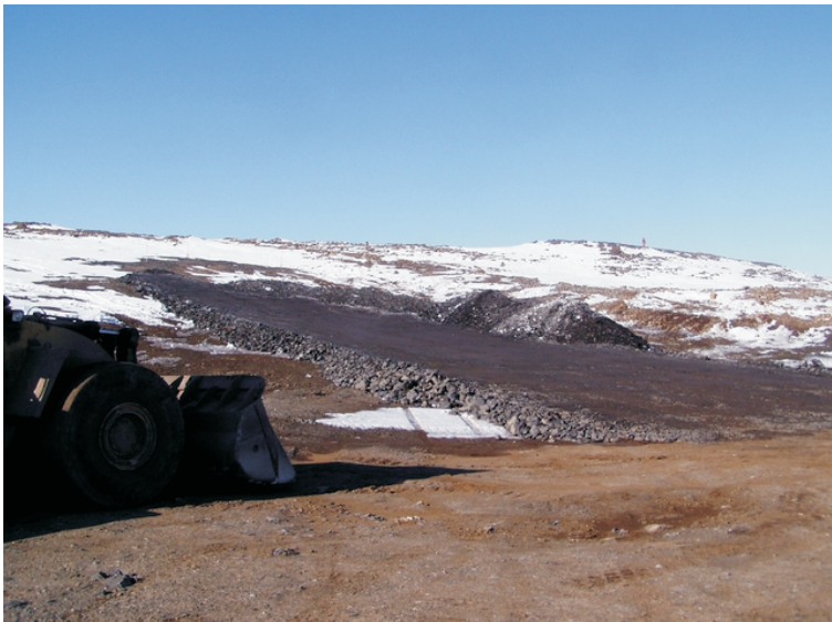
Photo 1 - Initial lift of shale for Oceanview Portal cover. Date: May 28, 2005
