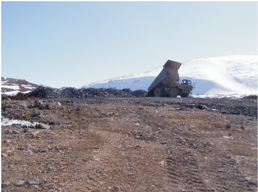
Photo 2 - Constructing thermal cover at K-Baseline Portal. Date: May 28, 2005
