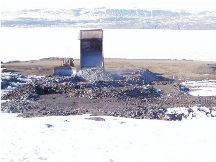
Photo 3 - Constructing second lift of shale for Oceanview Portal cover. Date: May 29, 2005
