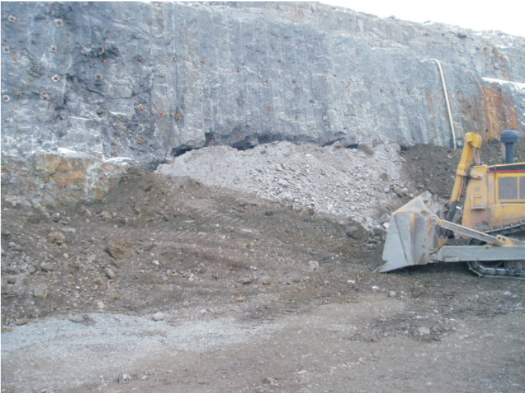
Photo 4 - Backfilled 01 Portal. Date: September 30, 2005
