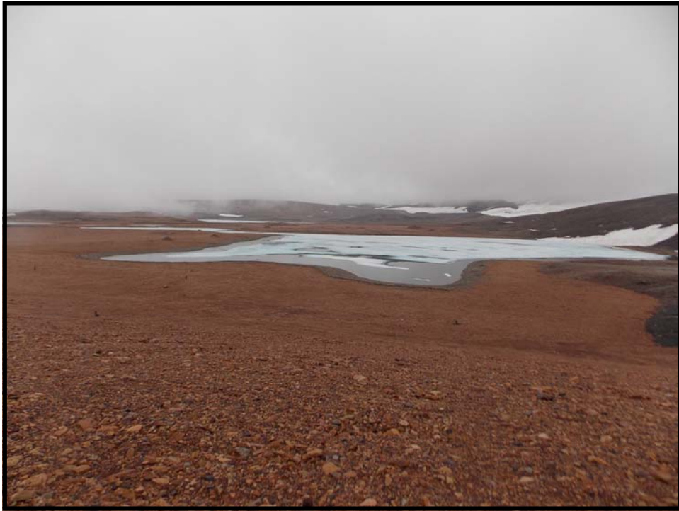
Photo 27. Toe of West Twin Dyke.
