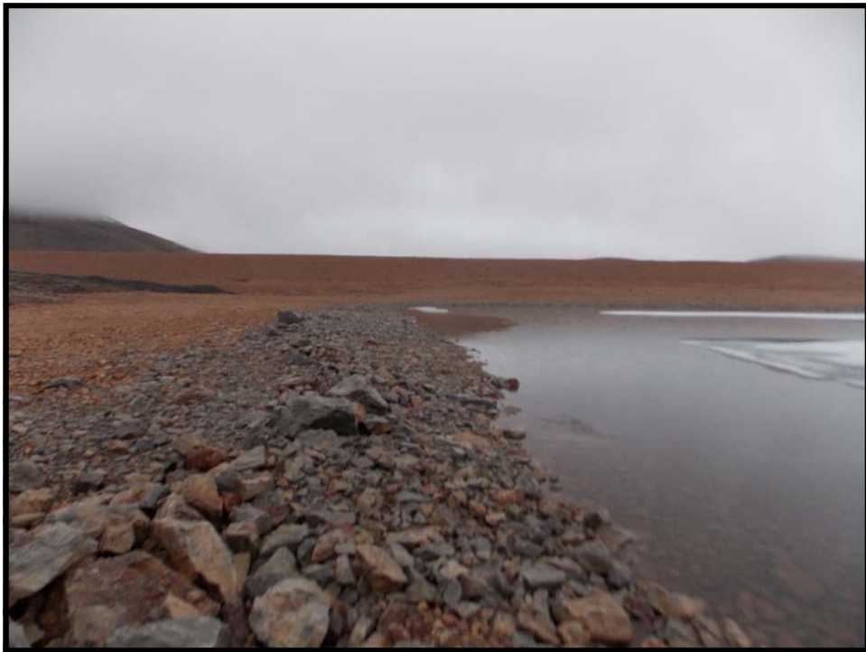
Photo 28. Toe of West Twin Dyke—Armour along shoreline of cover at toe of West Twin Dyke.
