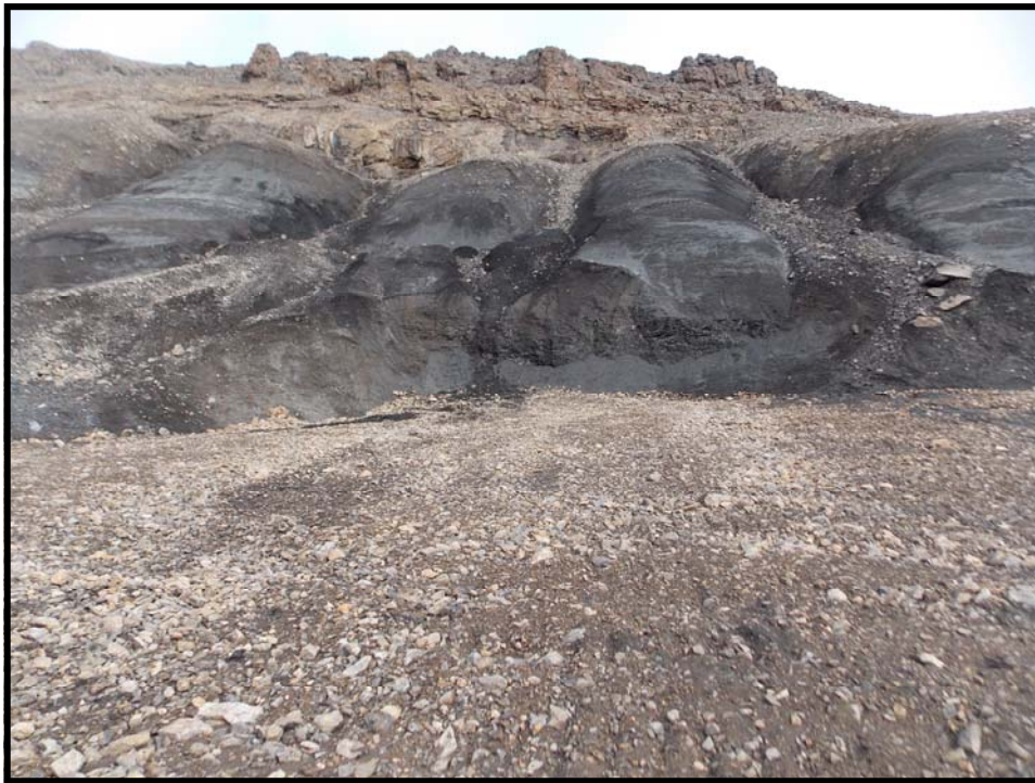
Photo 59. 09S Portal—Looking upslope along surface of cover.
