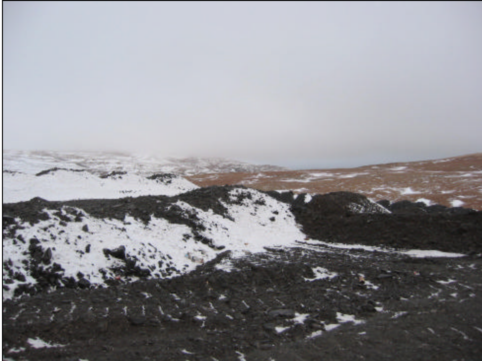
Photo 5 – Shale has been mixed with waste at the landfill and bulldozed into layers
