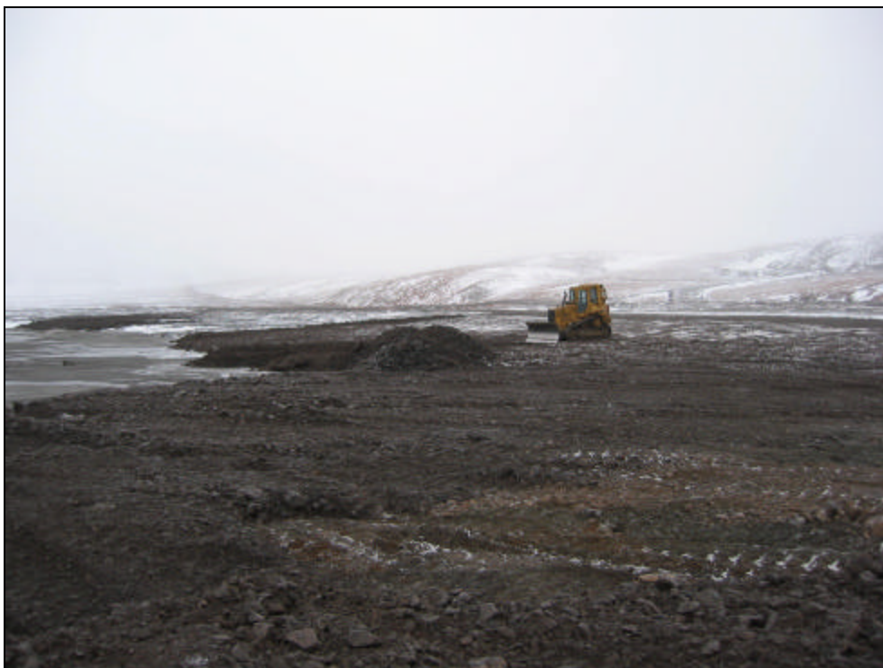
Photo 4 – Heavy machinery was placing crushed shale over WTDA, however due to wet conditions this activity had been temporarily halted.
