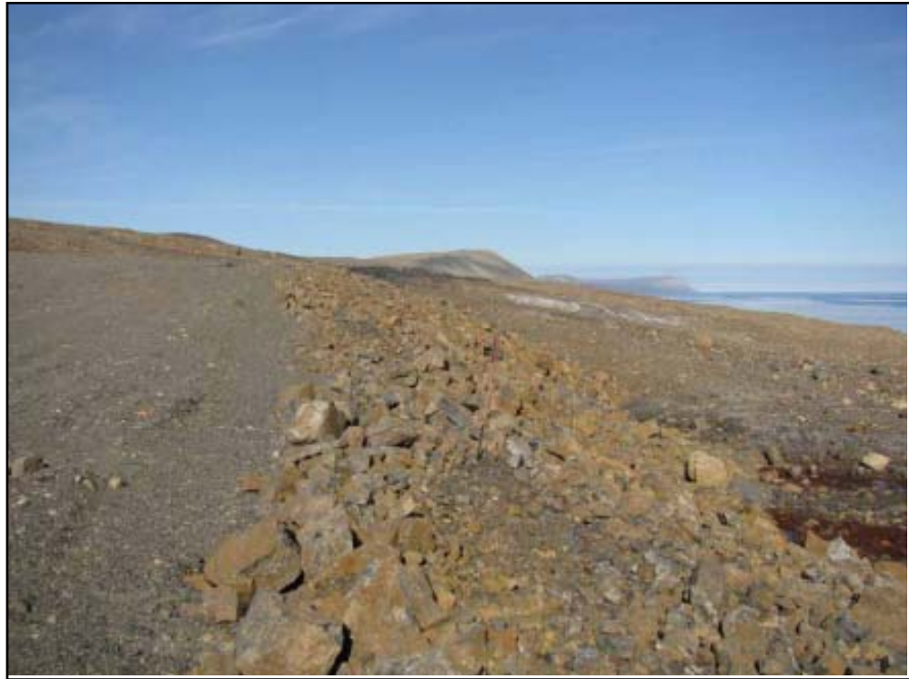
Photo 50 Rockfill placed against the toe of the Oceanview Open Pit cover.
