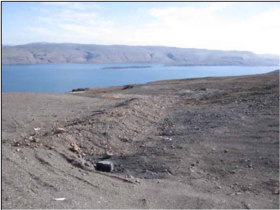
Photo 61 Water deflection berm at the Oceanview Portal cover.
