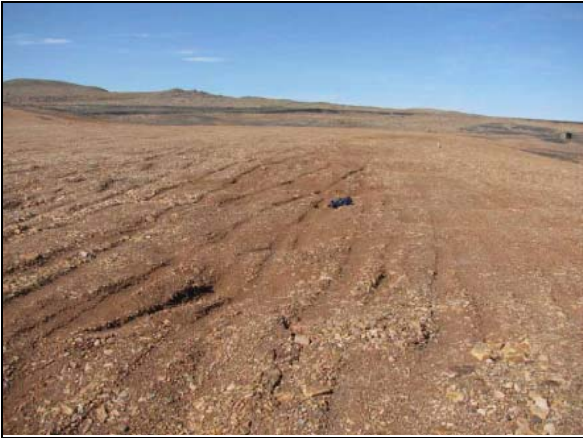
Photo 26 Soft area on the crest of the North/South area of the Test Cell Dike.
