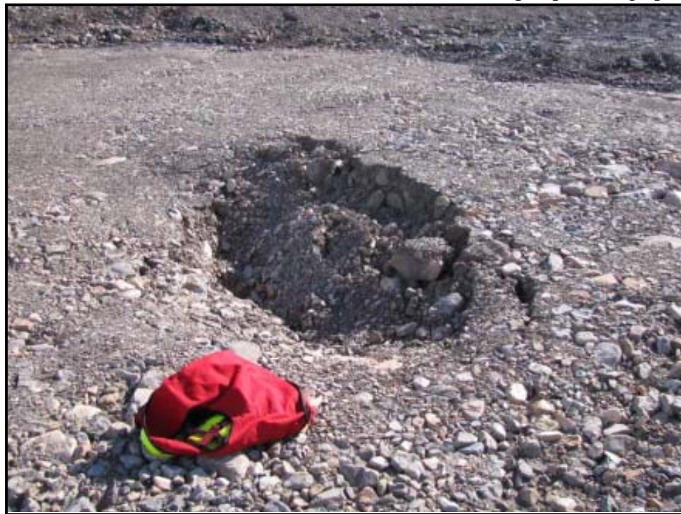
Photo 58 Thermokarst feature in 17N Portal Cover.
