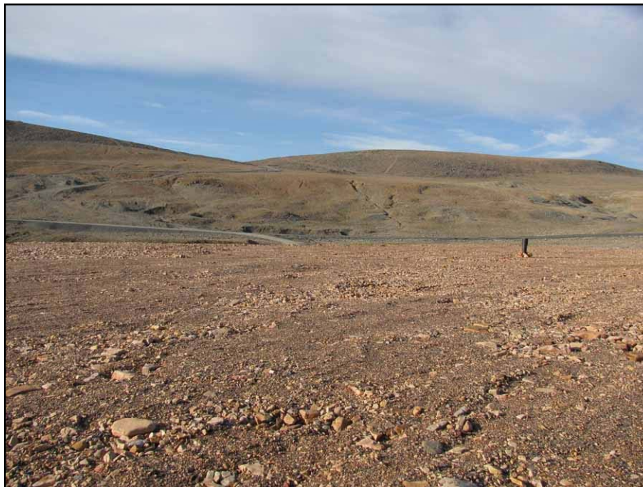
Photo 56 Surface of Upper Dump Pond tailings cover. Note frost gauge FG17 on surface of cover.
