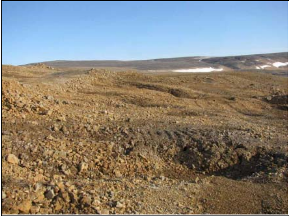
Photo 71 Minor thermokarsting at Area 14 armour borrow area. Note that it does not appear to have progressed since 2007.
