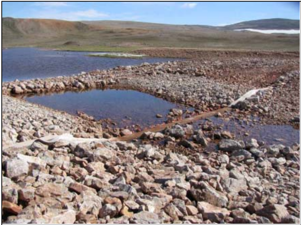
Photo 11 West Twin Outlet Wall. Note water level is approximately 3 cm below invert of wall.
