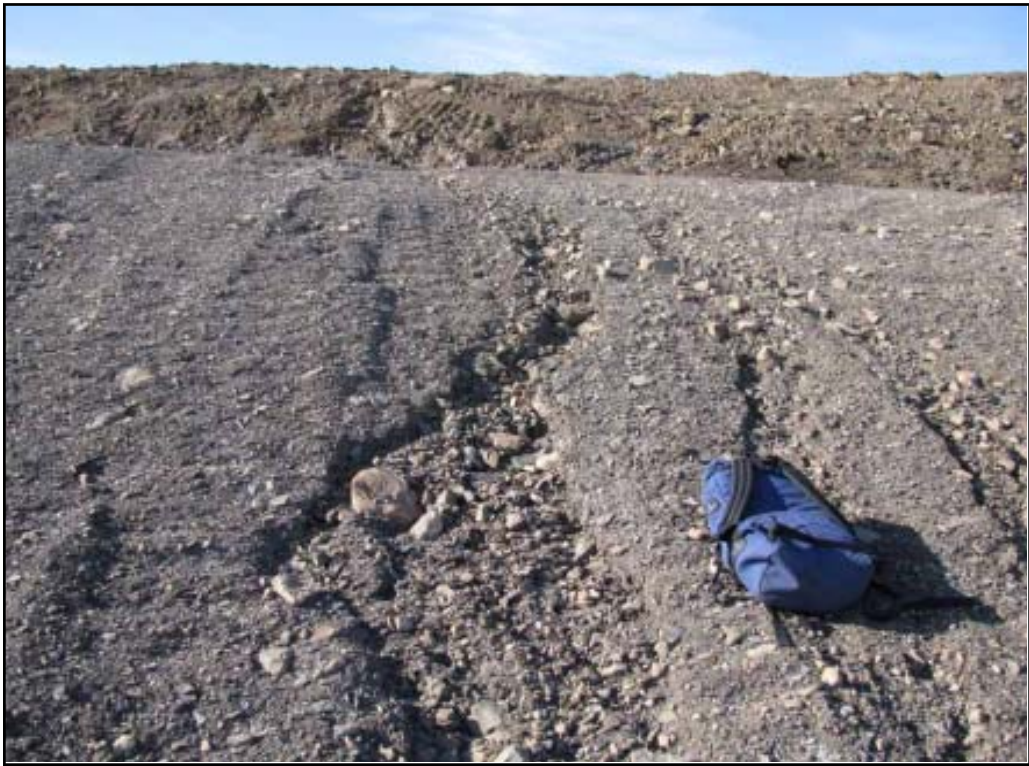
Photo 49 Minor rill erosion in southwest corner of Oceanview Open Pit cover. Note self armouring occurring. Erosion does not appear to have progressed since 2007.
