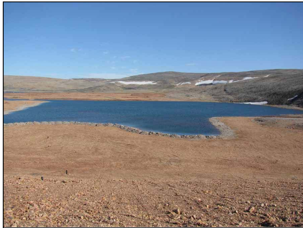
Photo 31 Riprap stockpiled along shoreline of tailings cover at the toe of the West Twin Dike.
