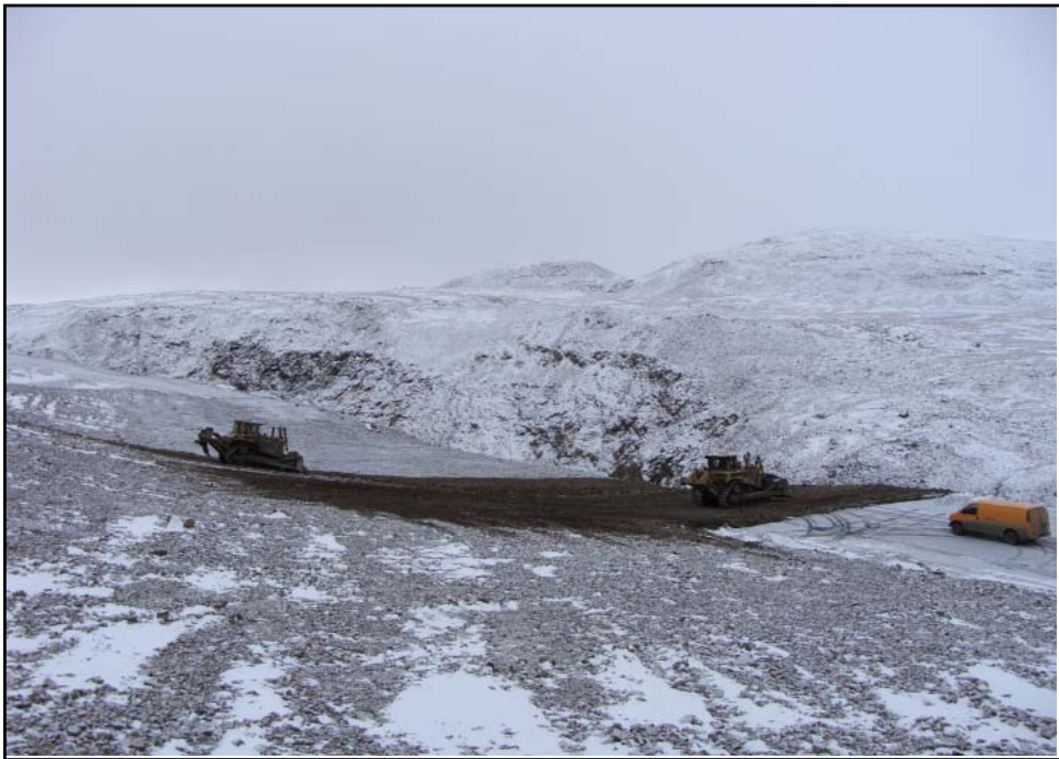
Photo 40 Photo taken in September 2008. Construction photo of the spreading of armour rock over the exposed shale in the road across the toe of the West Open Pit cover.
