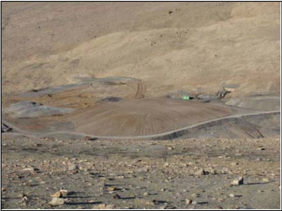
Photo 78 Industrial Complex cover as seen from Stol Port. Note that this cover was completed over metals contaminated soil and the original foundation during the summer of 2008.
