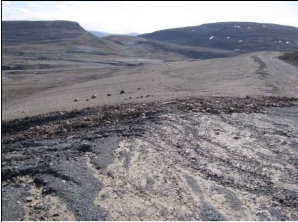
Photo 43 Surface of the East Open Pit cover. Note that minor erosion of exposed shale near the edge of the cover was noted.
