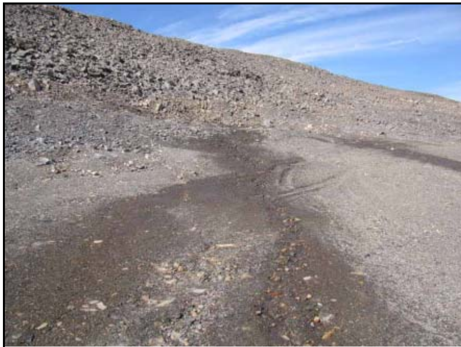
Photo 46 Very minor rill erosion attributed to constant seepage on surface of East Trench cover. Similar to what was observed in 2007.
