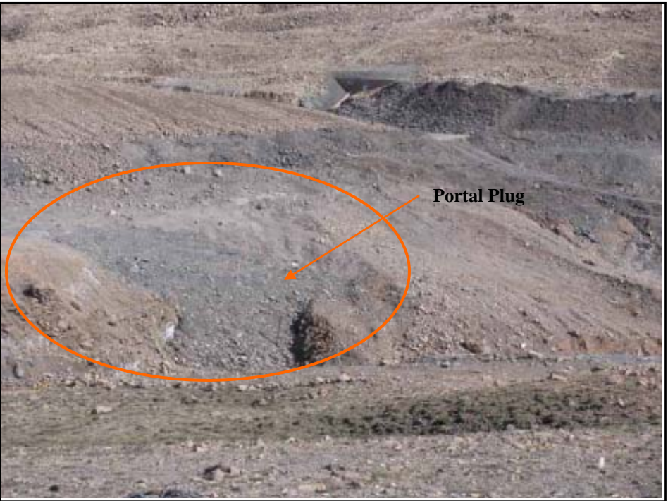
Photo 81 Mill foundation plug. Note no armour material had been applied to the face of the plug at the time of the photo.
