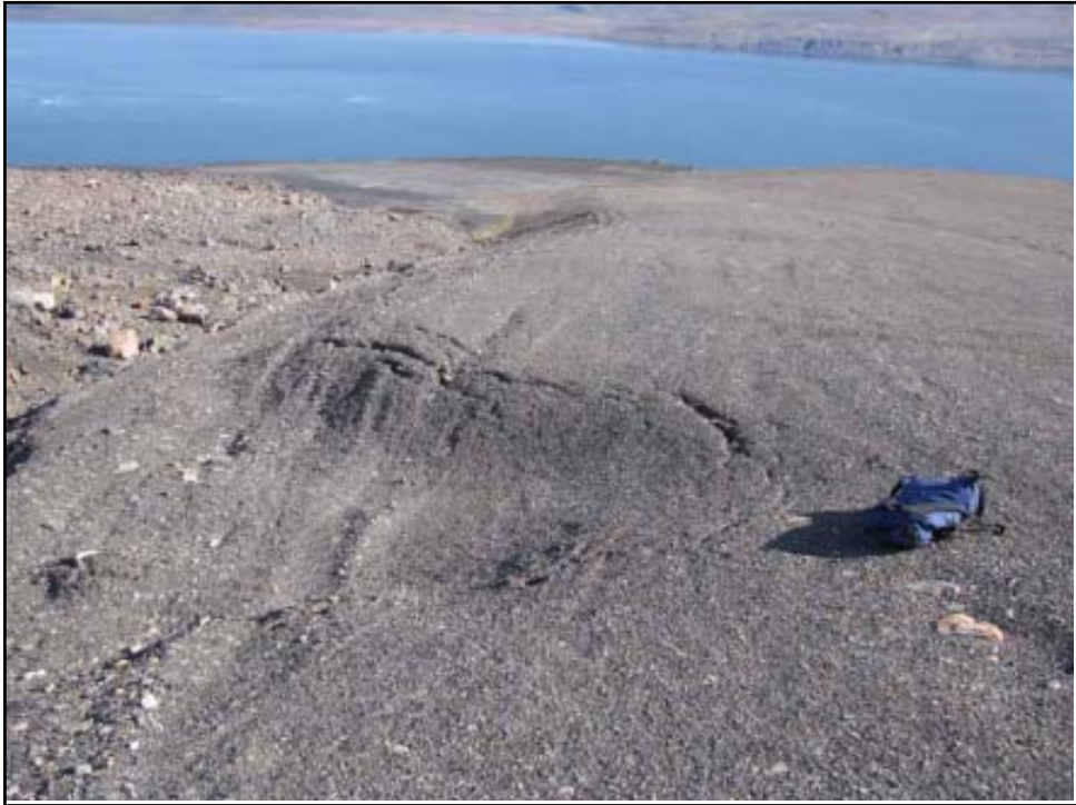
Photo 59 Settlement depression at the southwest corner of the Oceanview Portal cover. Note that the depression does not appear to have progressed since 2007.
