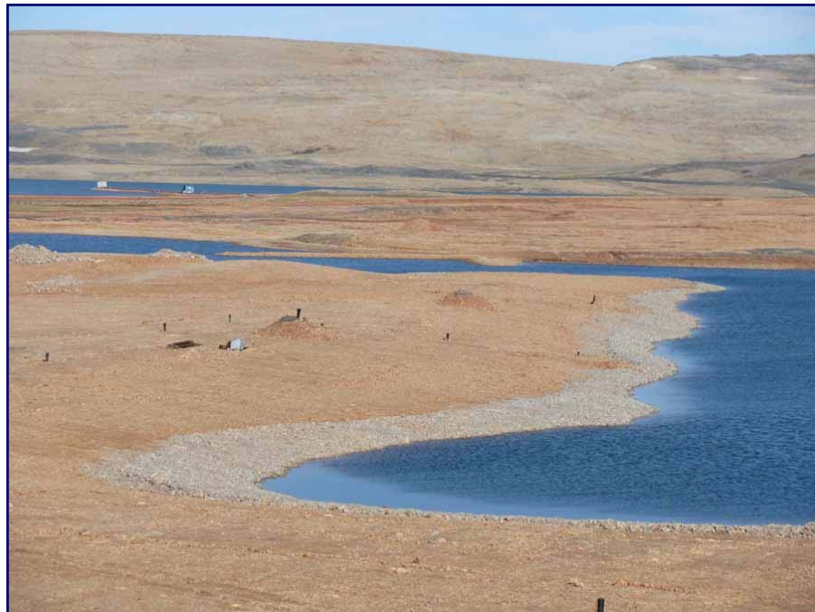
Photo 28 Riprap along toe of East/West arm of Test Cell Dike.
