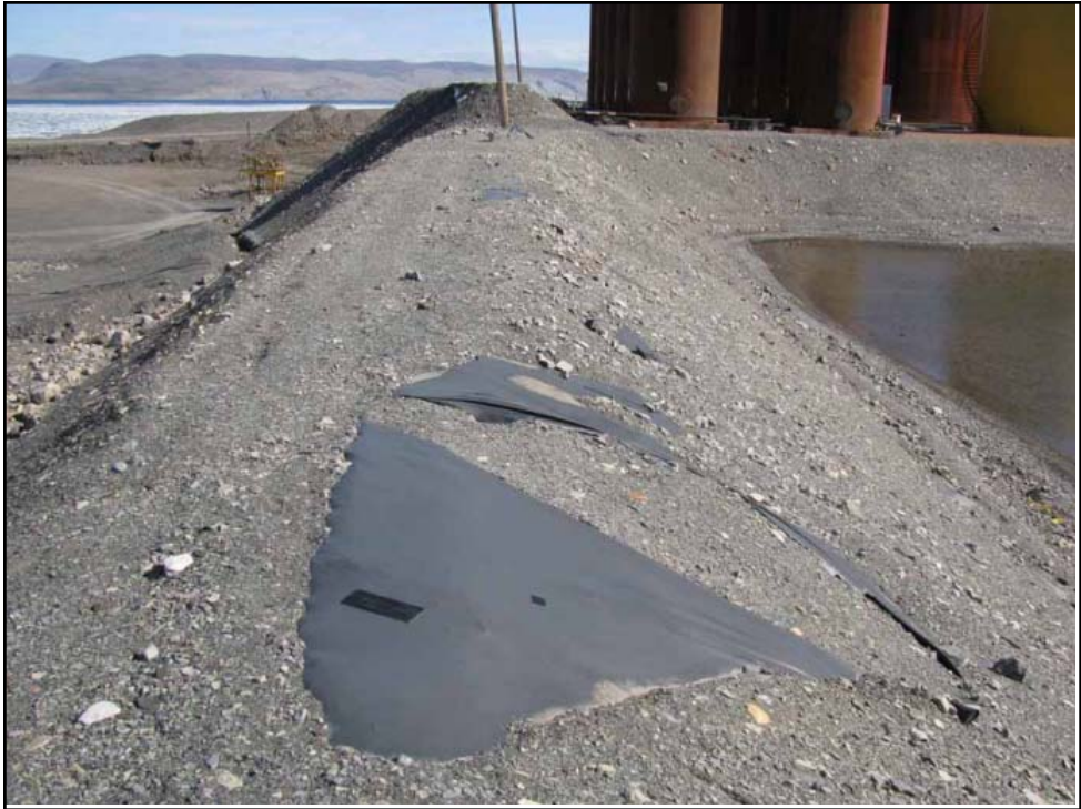
Photo 5 Exposures and tears of internal liner.
