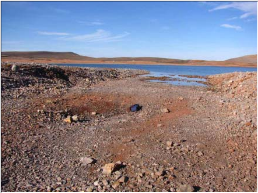
Photo 9 Settlement depression near spillway outlet.
