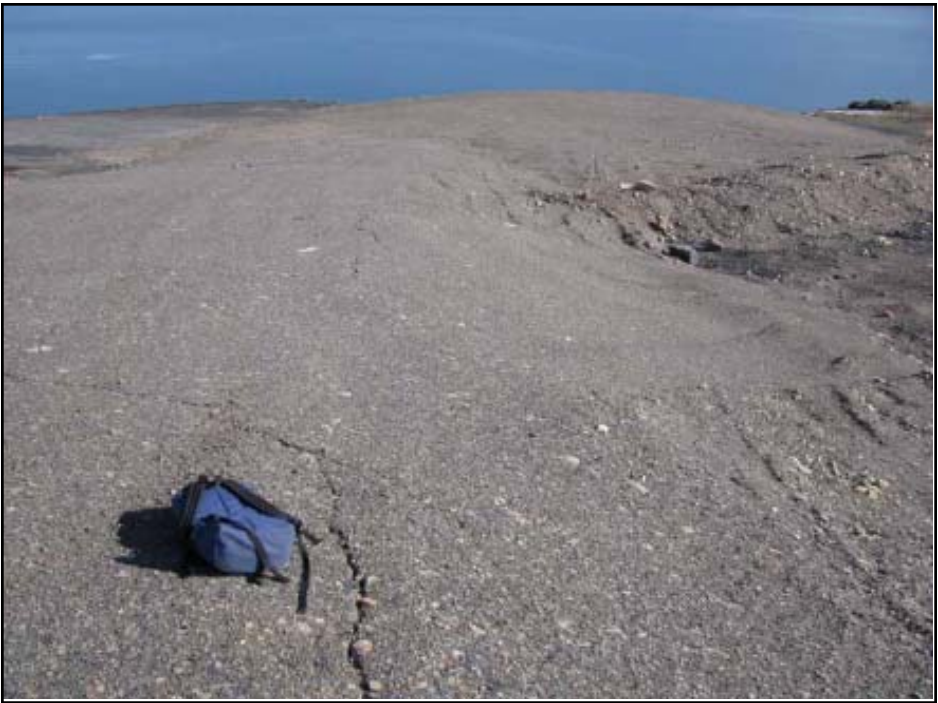
Photo 60 Oceanview Portal cover as seen from the upslope edge of the cover. Note minor cracking along the right (east) edge of the cover.
