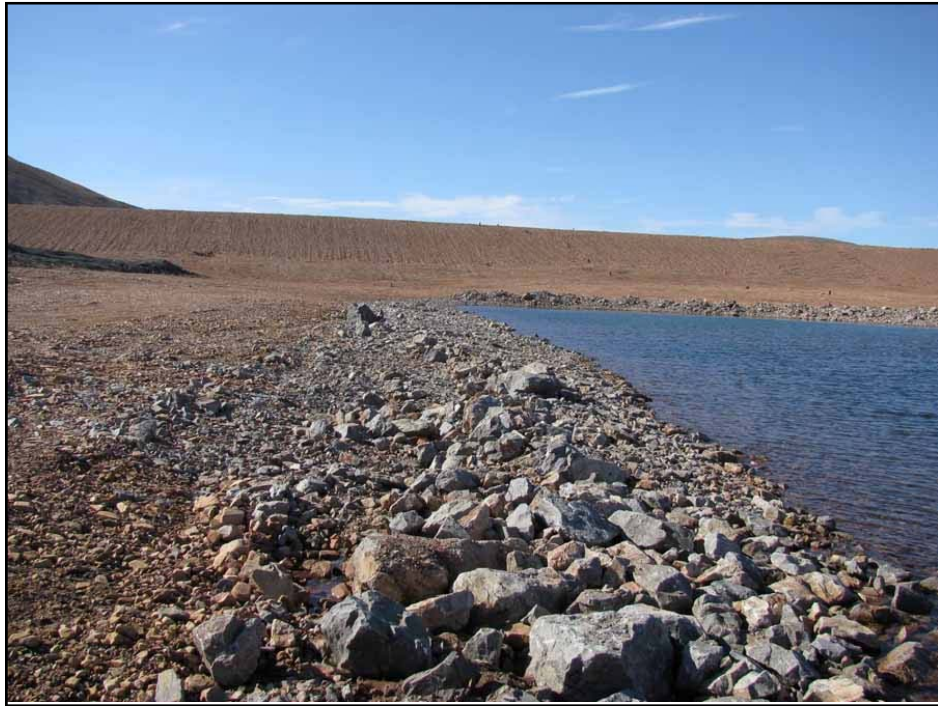
Photo 32 Riprap along shoreline of Toe of West Twin Dike tailings cover.
