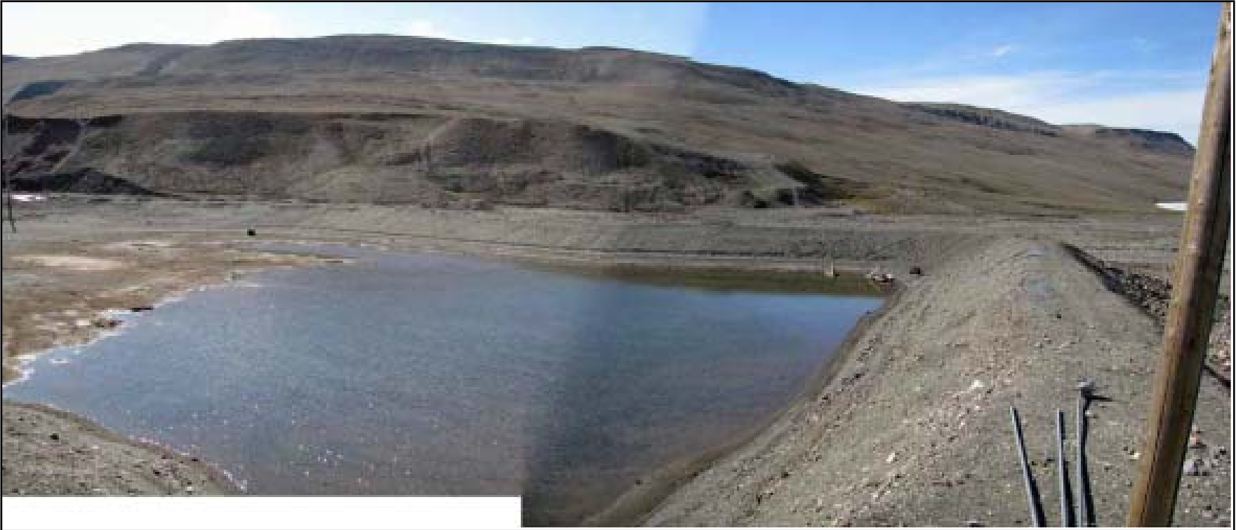
Photo 4 Inside of Main Tank Farm con- tainment berm. Note water retained in retention pond.
