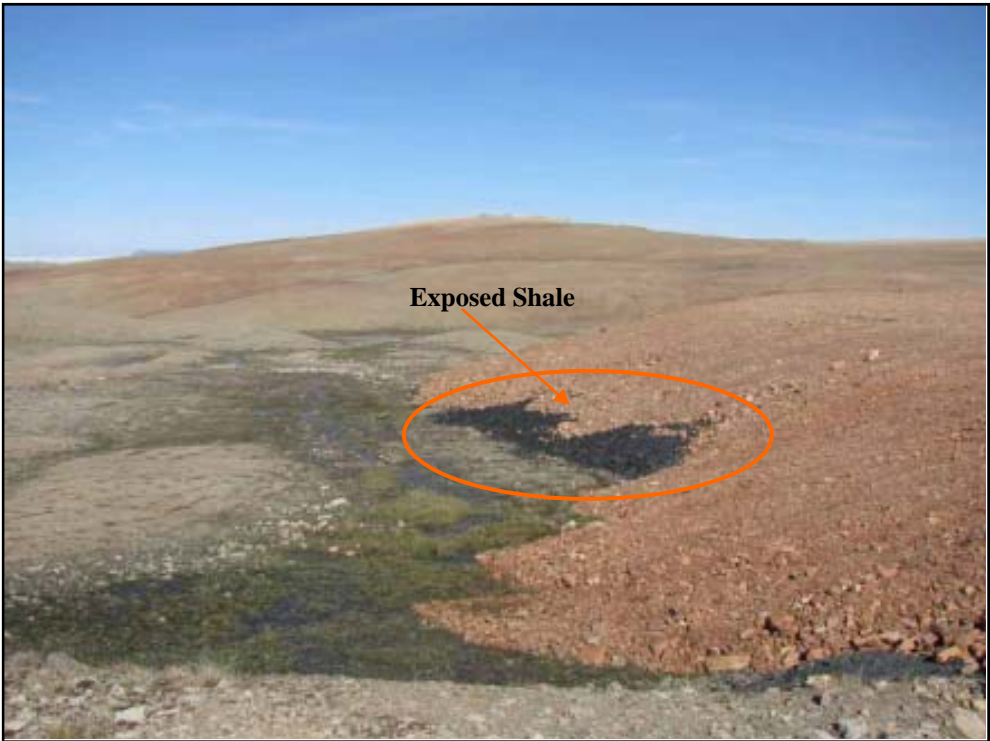
Photo 33 Toe of Landfill cover. Note exposed shale at toe of cover.
