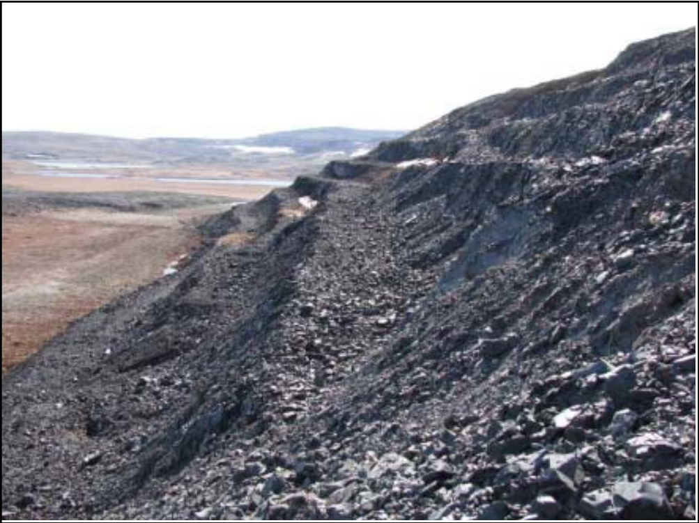
Photo 70 Mt. Fuji shale borrow area. Note that slopes are falling and are naturally reclaiming to the angle of repose.
