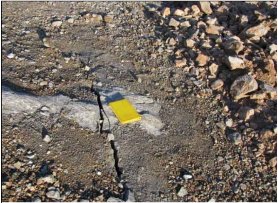
Photo 38 Crack in the West Open Pit crown pillar. Similar condition to what was observed in 2007.
