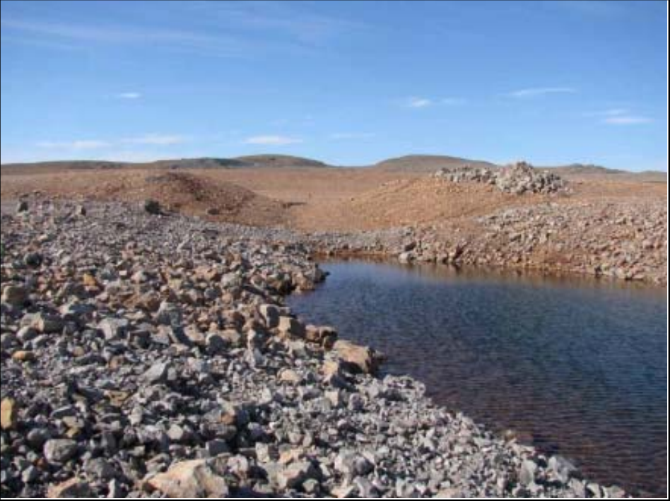
Photo 23 Rip rapped Test Cell outlet. Note riprap only applied to edge of water.
