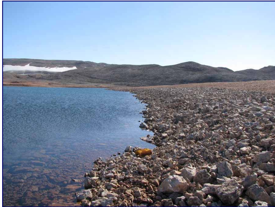
Photo 27 Riprap along toe of North/South arm of Test Cell Dike.
