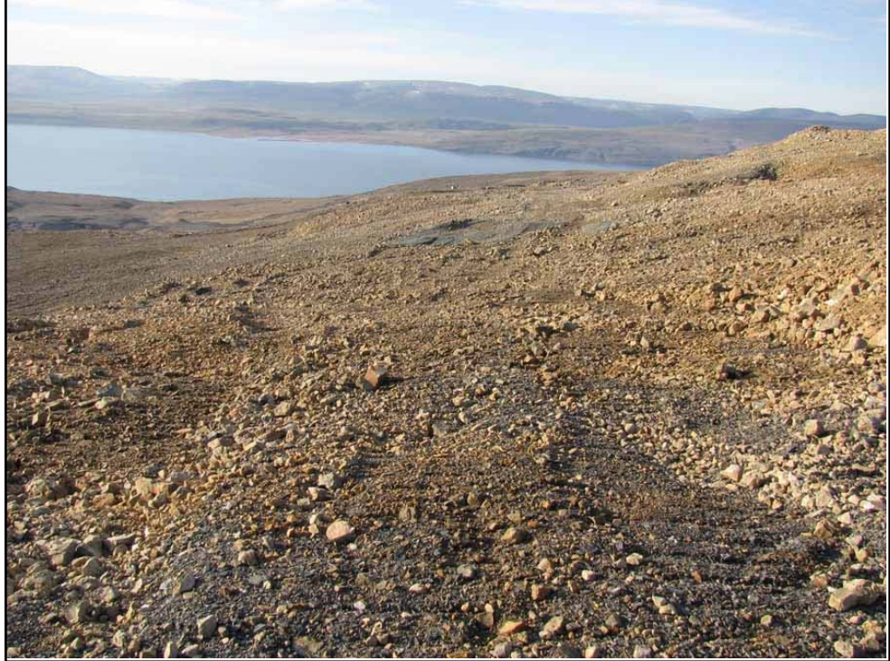
Photo 69 Area 14 Raise Cover. Note armour material applied to surface but no mound constructed.
