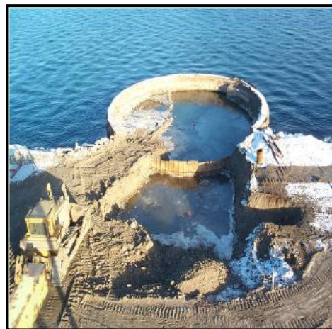
Figure 39 – Excavation of Hydrocarbon Contaminated Soils in Centre Dock Cell (2006)
