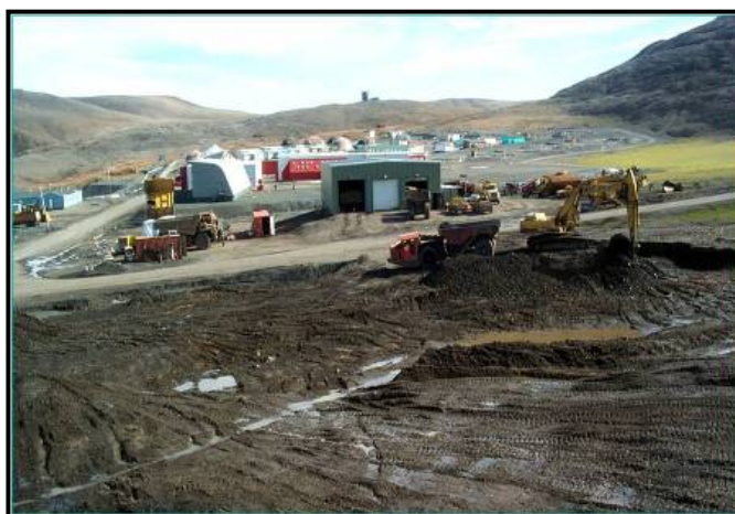
Figure 35 – Reclamation of Hydrocarbon Contaminated Soils, Nanisivik Townsite (2005)
