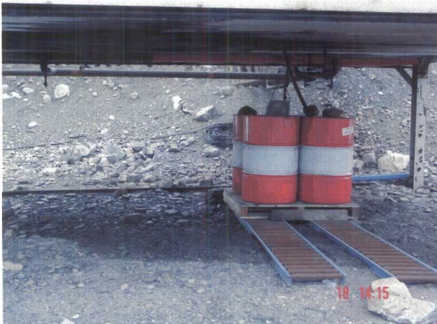
Photo # 10 Tank farm pump house spill. Note hose draining floor to drums below.
