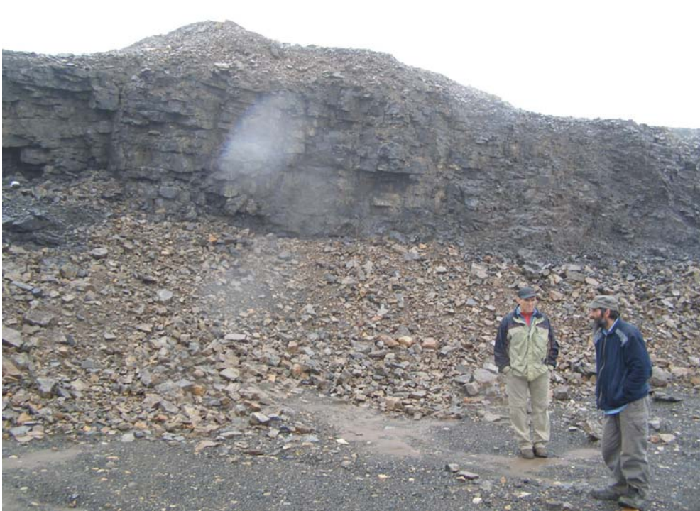
Photo 36 Base of the remnant East Open Pit highwall, some loose rock was noted.
