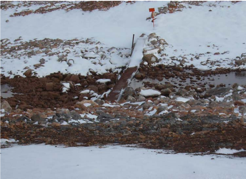
Photo 13 West Twin Outlet Wall in early September. Note reduction in water level upstream of wall.
