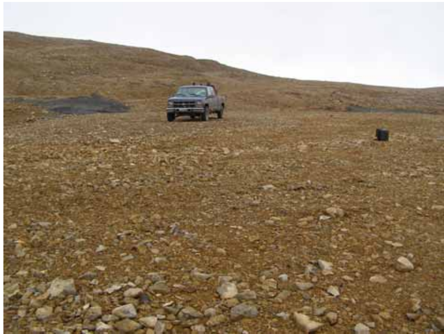
Photo 46 Upper flat surface of the Area 14 waste rock cover.
