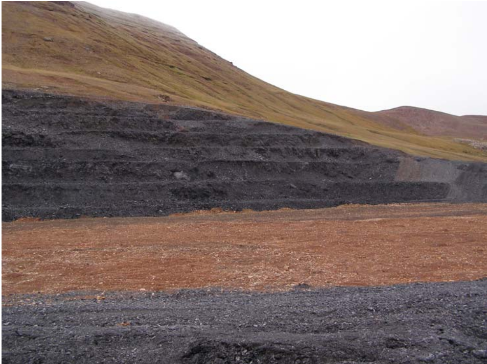
Photo 62 Mt. Fuji shale borrow area. Note that slopes are falling and are naturally reclaiming to the angle of repose.
