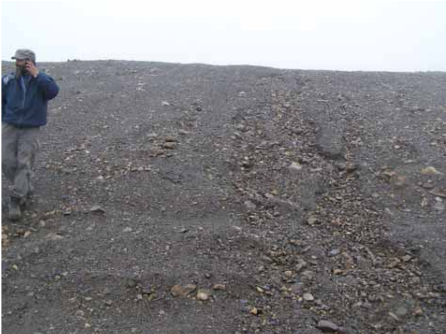
Photo 41 Minor erosion on the south face of the Oceanview Pit Cover.
