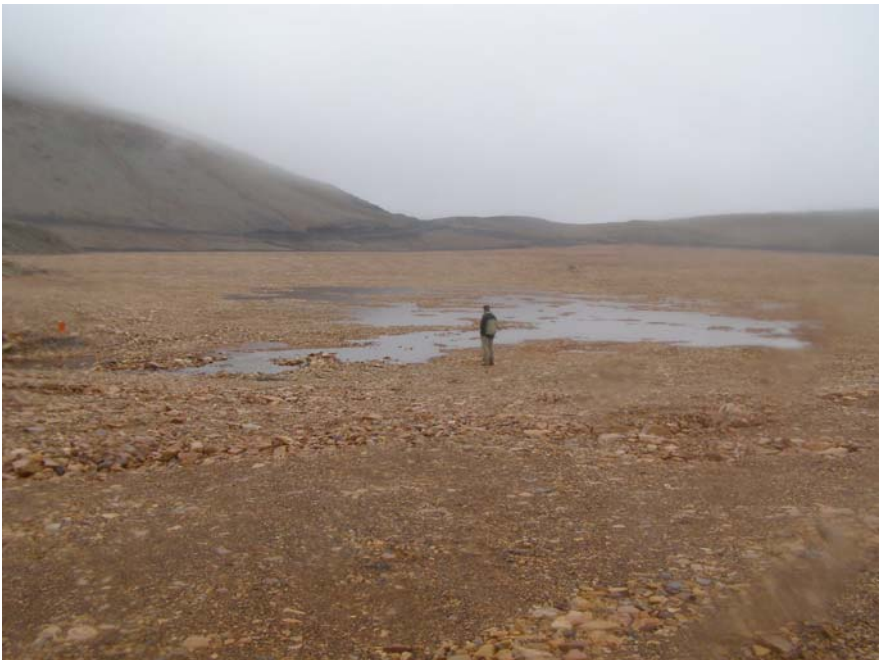
Photo 9 Head pond at spillway entrance. Note presence of exposed armour material in middle of pond which indicates a reduction in the water level of the retained pond.
