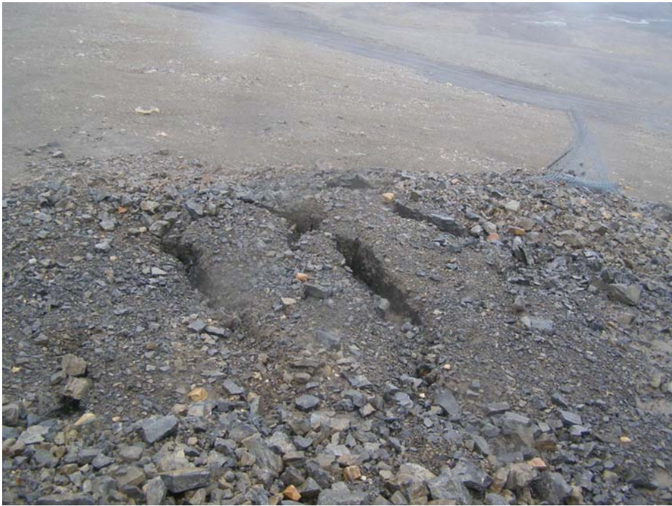
Photo 37 Crack in the crown pillar at the East Open Pit. No changes noted since 2008.
