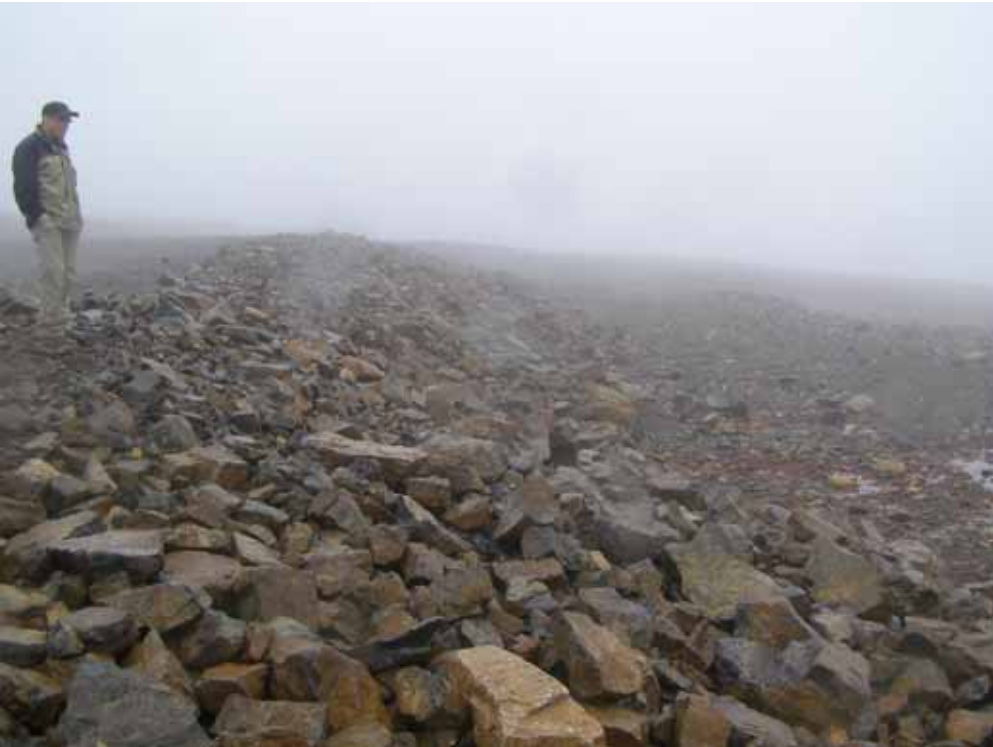
Photo 44 Rockfill placed against the toe of the Oceanview Open Pit cover.
