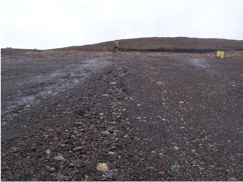
Photo 38 Minor surficial erosion observed on surface of East Open Pit cover.
