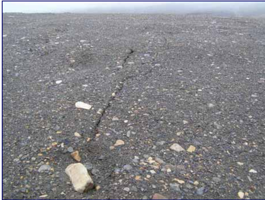
Photo 53 Surface of inclined face of K-Baseline Portal Cover. Note the cracking that is occurring.
