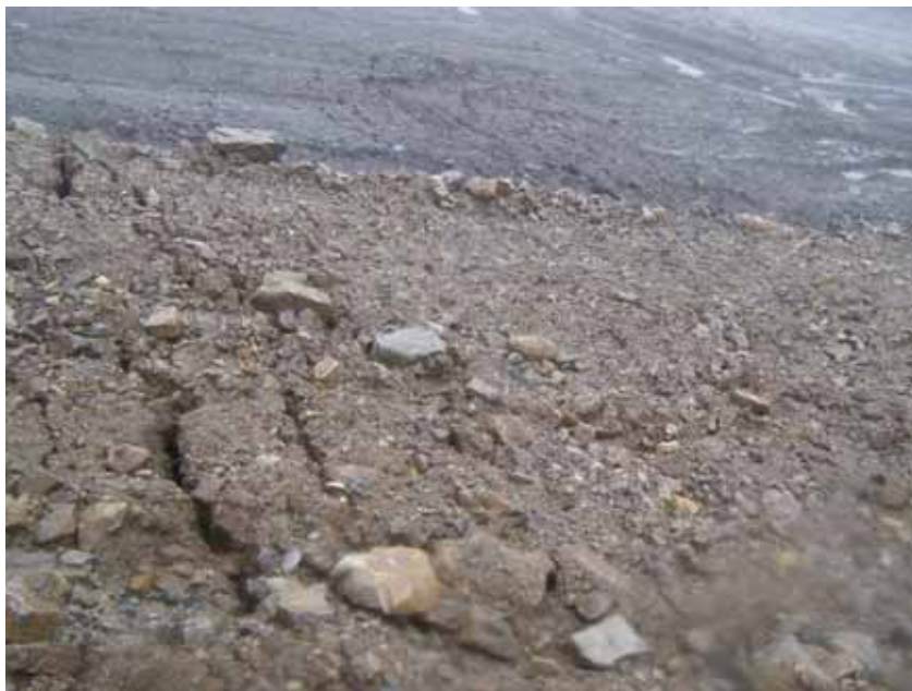
Photo 57 Cracking and deformation noted along east edge of portal cover.
