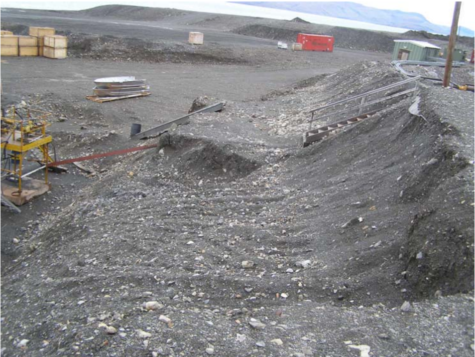
Photo 6 Affected area of Main Tank Farm berm which was partially excavated during reclamation of contaminated soils.
