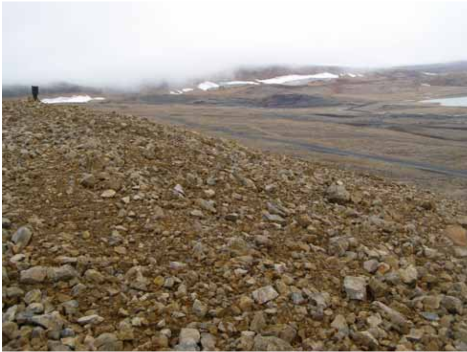
Photo 45 Face of the Area 14 Portal Cover. View looking south. Note frost gauge instrument at the crest of the slope.
