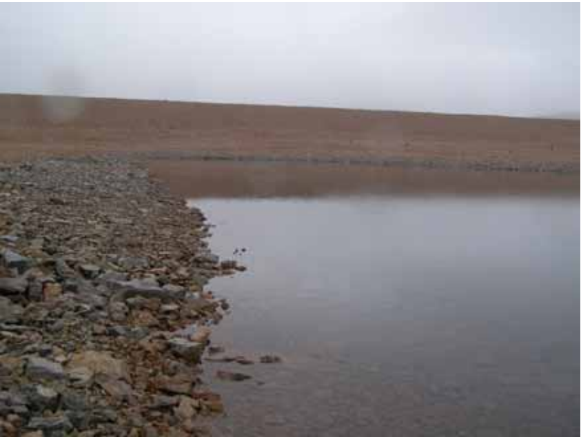
Photo 26 Rip rapped shoreline at Toe of West Twin Dike tailings cover .
