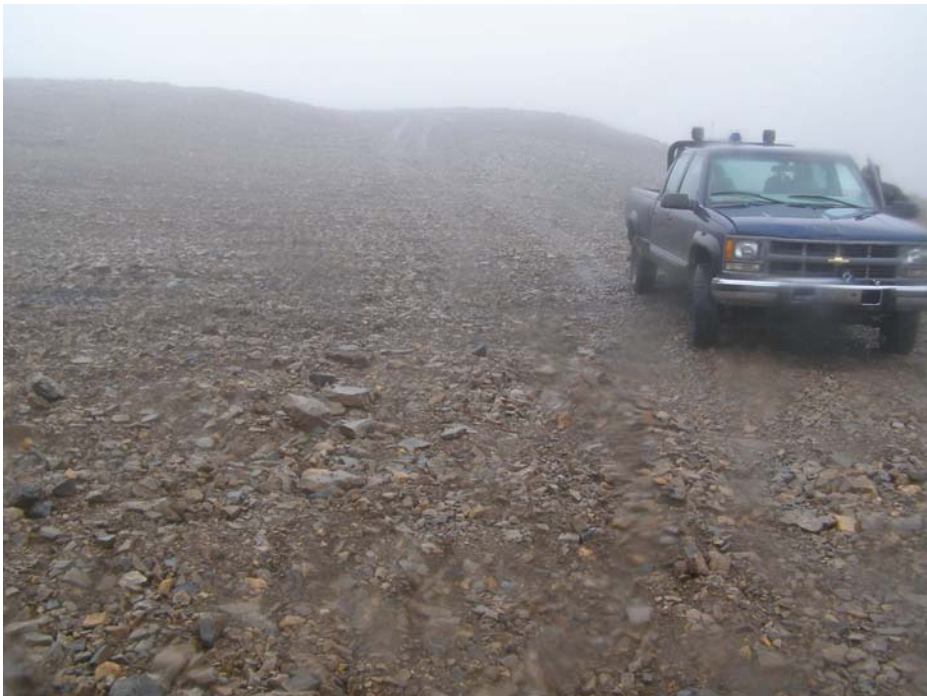
Photo 33 Surface of West Open Pit cover, roadway is armoured as requested in 2008.
