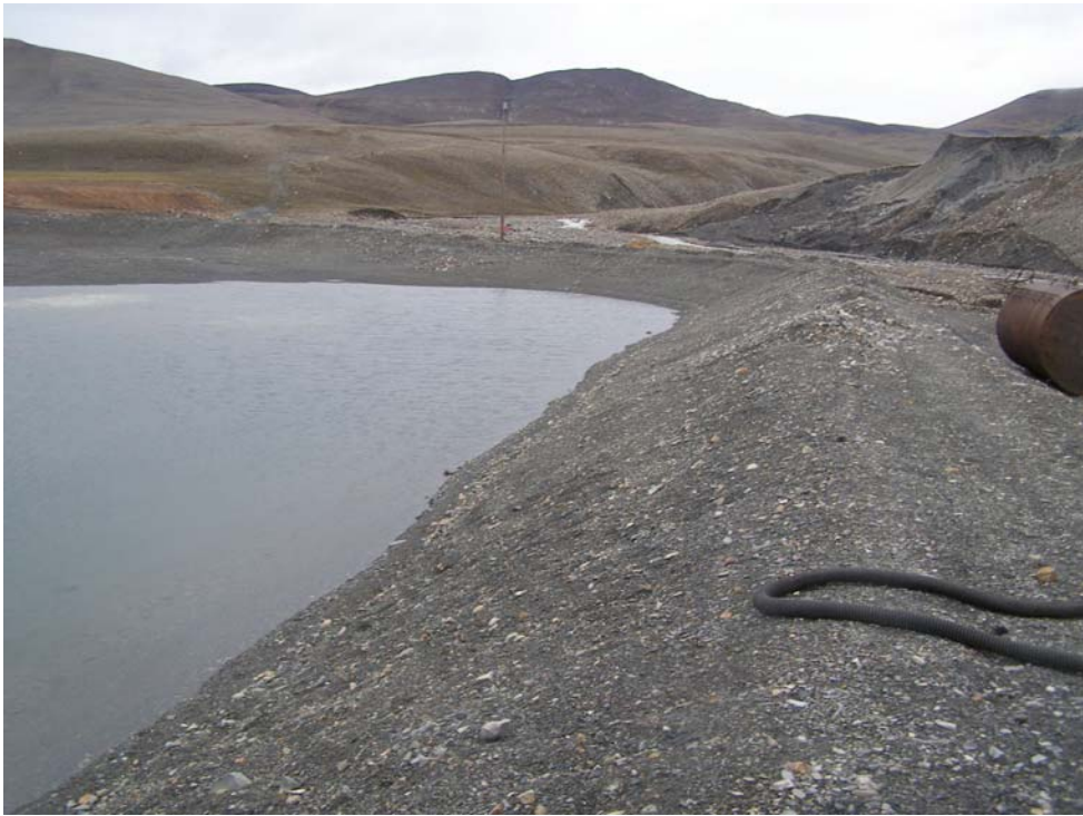
Photo 4 Inside of Main Tank Farm containment berm. Note water retained in retention pond.
