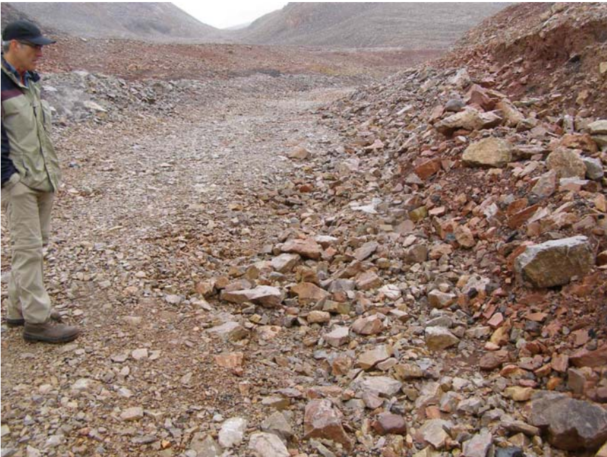
Photo 10 Small section of erosion in base of the spillway.
