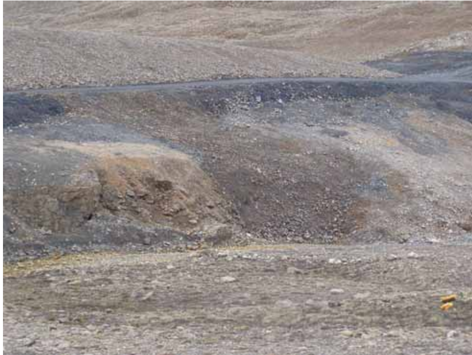
Photo 60 Mill Portal plug. Note that armour material was applied to the surface of the cover as recommended in 2008.
