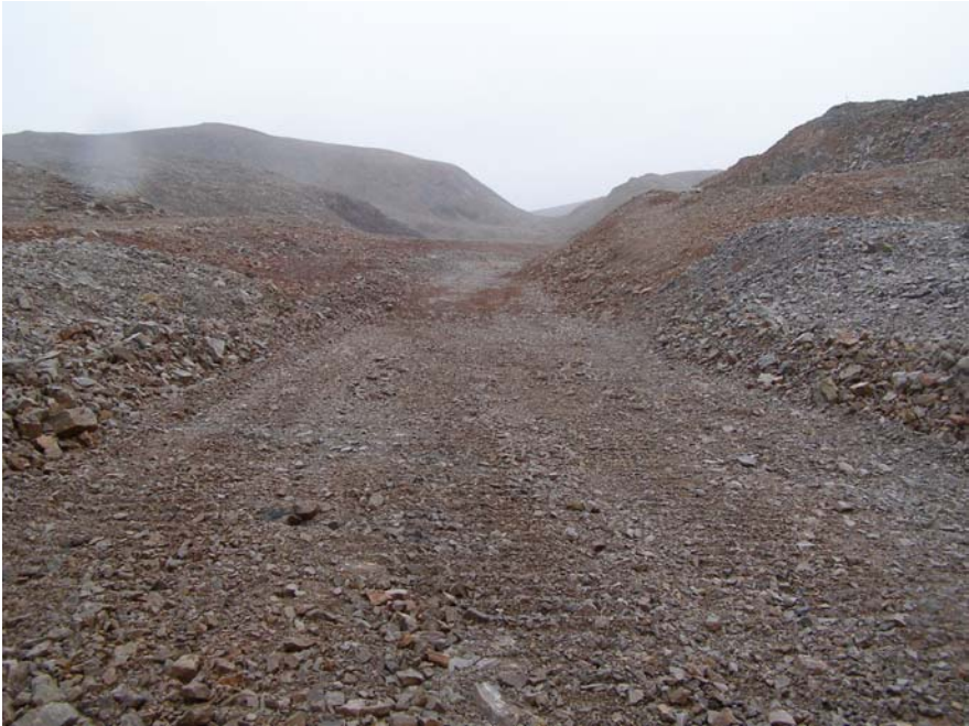
Photo 7 Re-graded bottom of the spillway.
