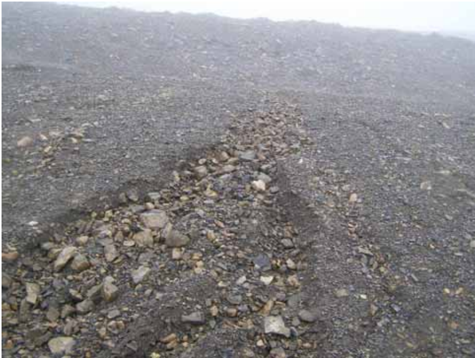
Photo 43 Minor rill erosion in southwest corner of Oceanview Open Pit cover. Note self armouring occurring. Erosion does not appear to have progressed significantly since 2008.
