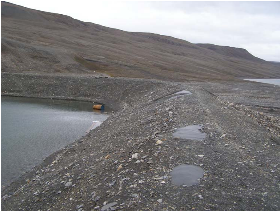
Photo 5 Exposures of internal liner.
