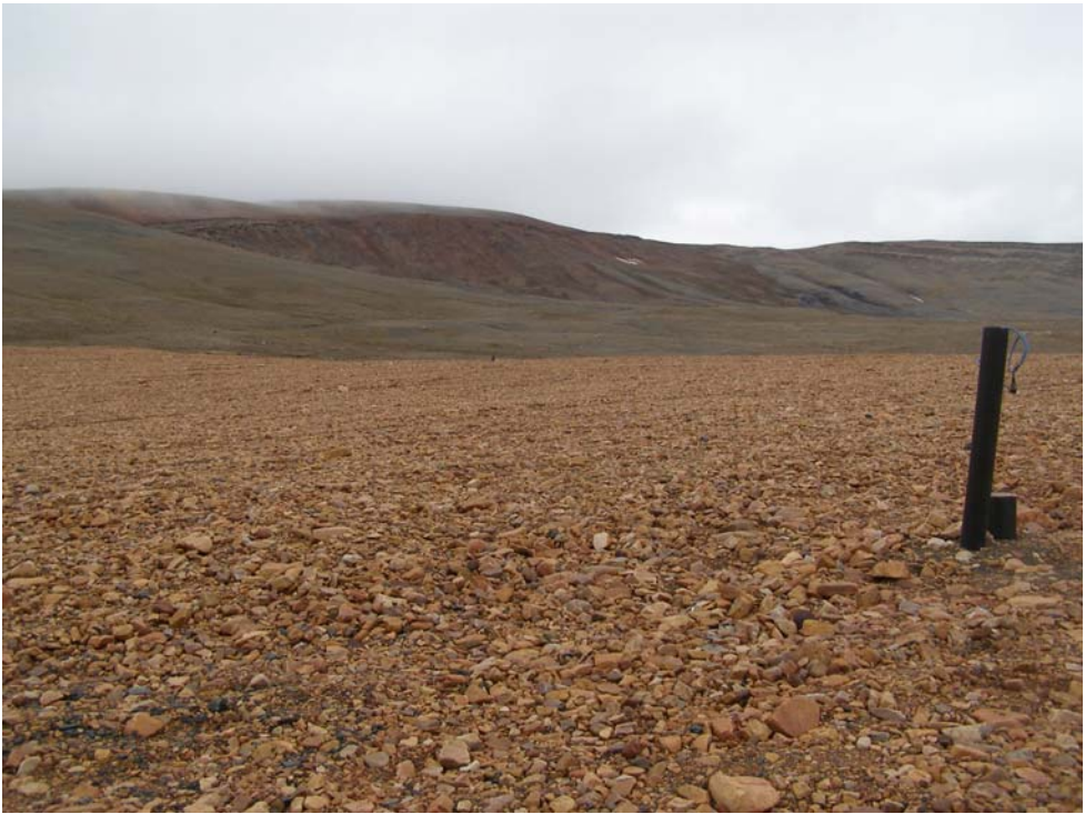
Photo 29 Re-compacted surface of Landfill cover.
