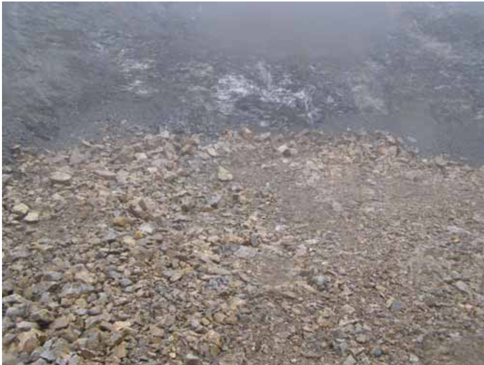
Photo 56 Surface of 09 South Portal Plug where cover butts against crown pillar.
