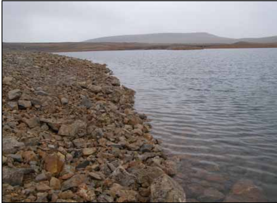
Photo 23 Riprap along toe of North/South arm of Test Cell Dike.
