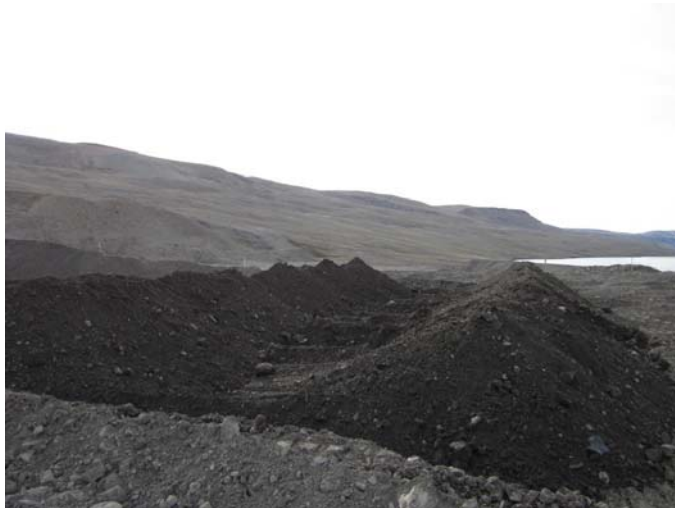
Photo 13: Windrows within in-situ treatment area
