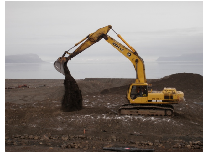
Photo 12: Fertilizer being mixed into the soil at LTA (July 14, 2012)
