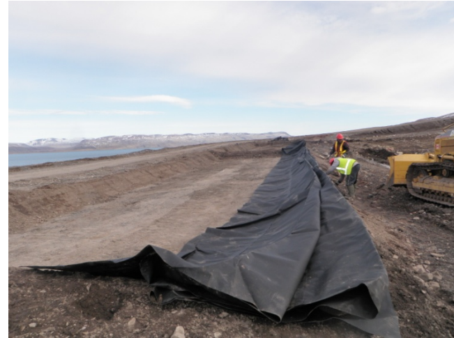
Photo 2: RLLDPE liner placement in UTA-9 (August 20, 2012)
