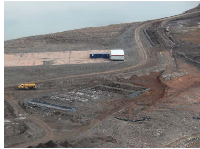
Photo 4: Aerial view of LTA and drainage diversion berm and silt fencing (August 30, 2012) (photo courtesy of Canadian Coast Guard)
