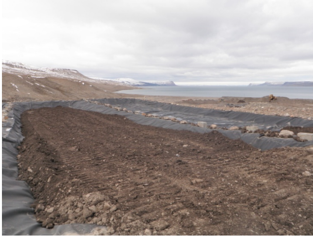
Photo 9: Base and ramp completed in UTA-7 (August 20, 2012)
