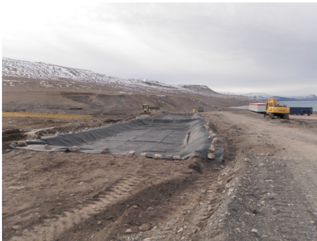
Photo 3: Liner placed and secured in UTA-10 (August 20, 2012)
