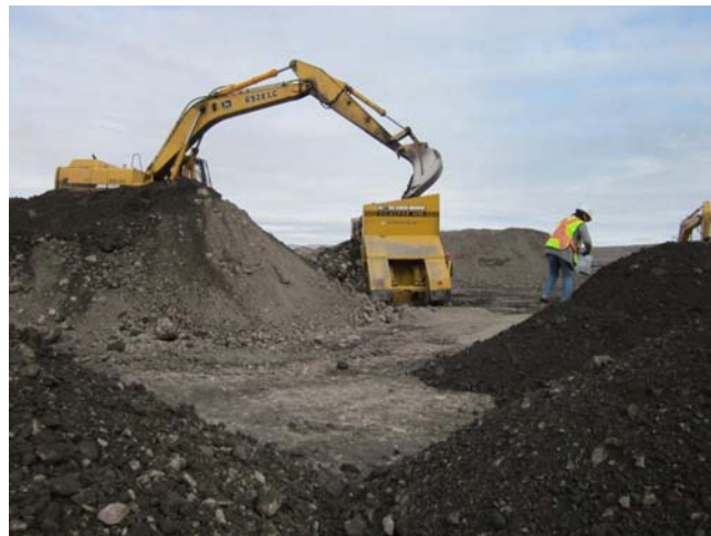
Photo 7: Collecting sample of soil from in-situ area following screening of oversized rock (August 22, 2012)
