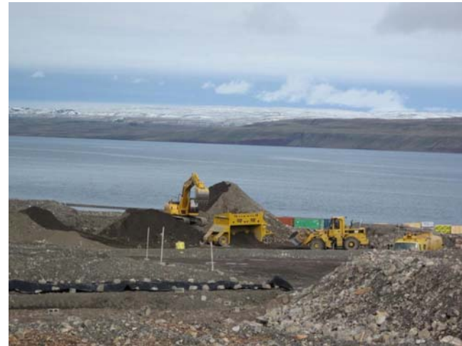
Photo 6: Screening of oversized rock from stockpile in Area 1 (August 18, 2012)
