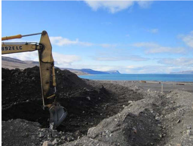
Photo 5: Excavation of Area 1 with exterior berm being maintained (August 12, 2012)
