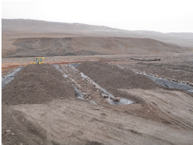
Photo 11: Screened contaminated soil loaded in LTA-5 and LTA-6 (August 24, 2012)
