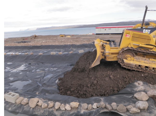
Photo 8: Bulldozer pushes screened low level PHC contaminated soil into UTA-7 to create base layer (August 20, 2012)
