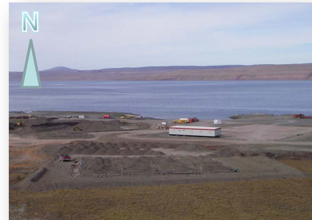
Photo 4: Site overview on August 24, 2011. UTA with water diversion berm in foreground and construction of cells 6, 7, and 8 in progress.
