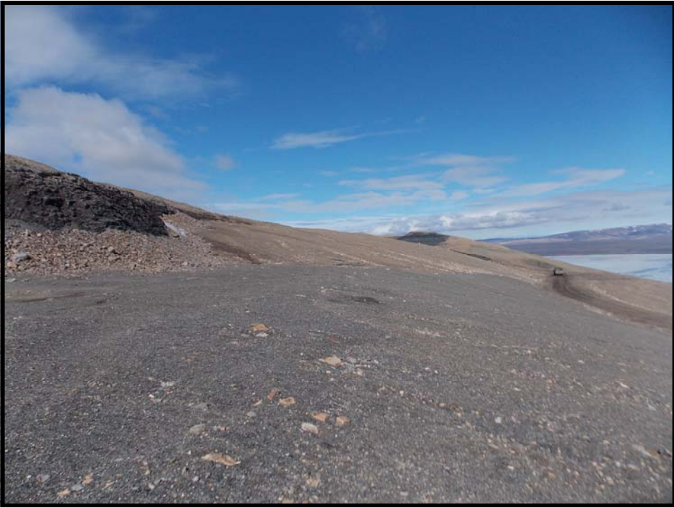
Photo 37. East Open Pit—Sloping upper surface of cover system.
