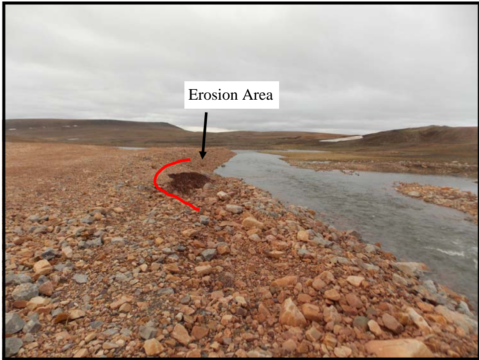
Photo 14. East Twin Creek Diversion Channel– Erosion area noted above seepage discharge point. Erosion is further advanced compared to 2012.
