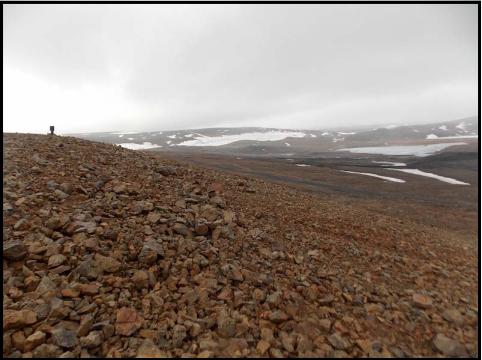
Photo 52. Industrial Complex Cover—Sloping face of cover.
