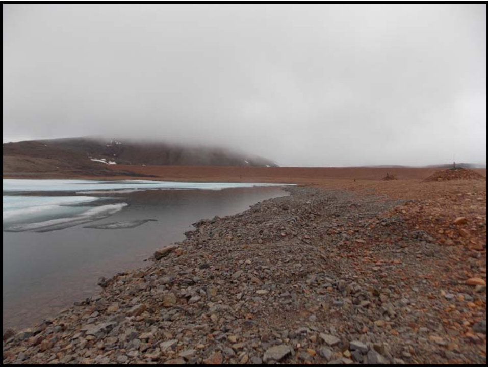
Photo 24. Toe of Test Cell Dyke—Armour along shoreline of cover at toe of Test Cell Dyke. East/West arm, view looking west.
