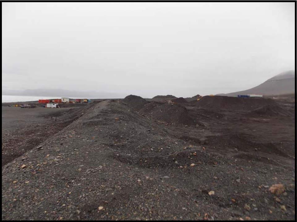
Photo 2. Main Tank Farm—Remnant perimeter dyke in location of old water retention pond.
