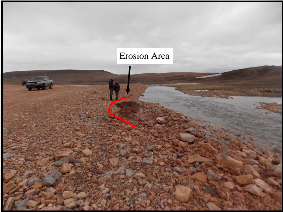
Photo 13. East Twin Creek Diversion Channel– Erosion area noted above seepage discharge point.
