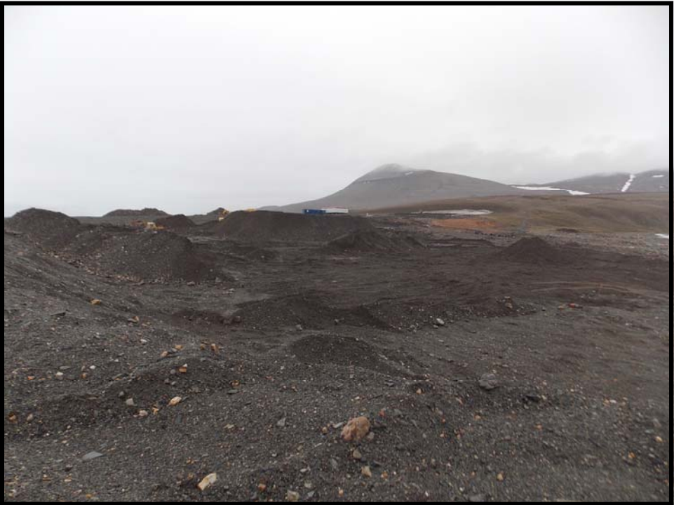
Photo 4. Main Tank Farm—Stockpiles of soil excavated from tank farm foundation.
