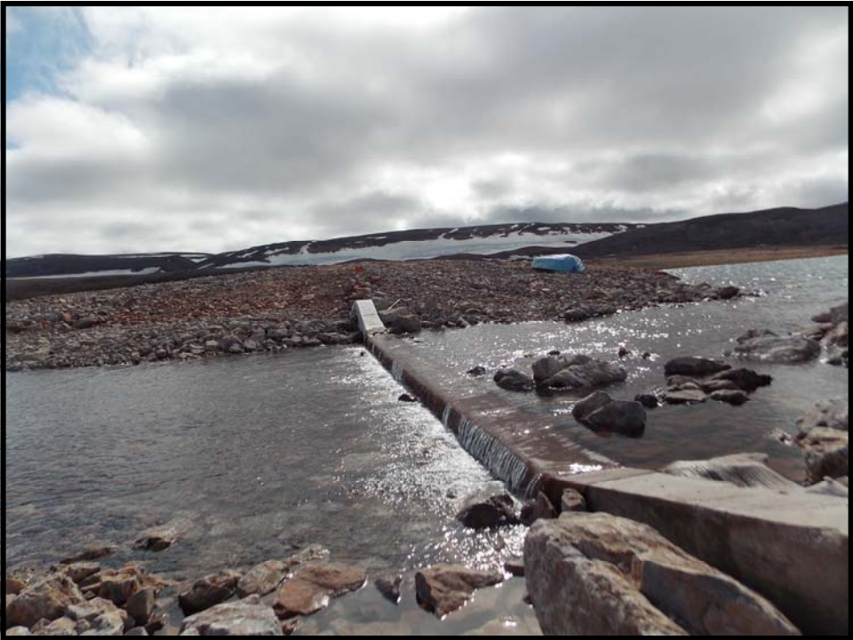
Photo 9. West Twin Outlet Channel—Note water running over wall.
