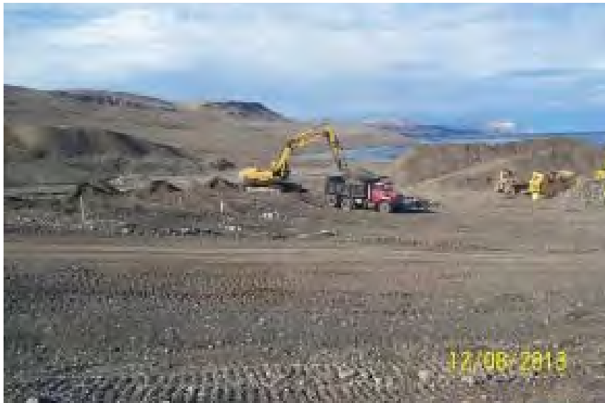
Photo 15: Stockpile of screened fine PHC contaminated soil on right and biopiles being removed from the lower treatment area on left.
