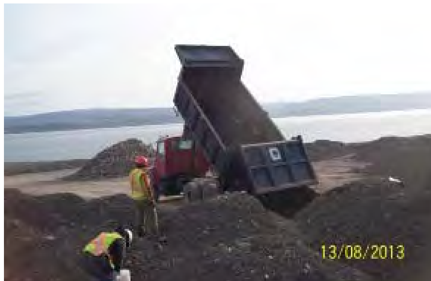
Photo 17: Biopiles from the upper and lower treatment area are relocated to the prepared area of the pad. The remaining stockpile of rock is in front of the truck.
