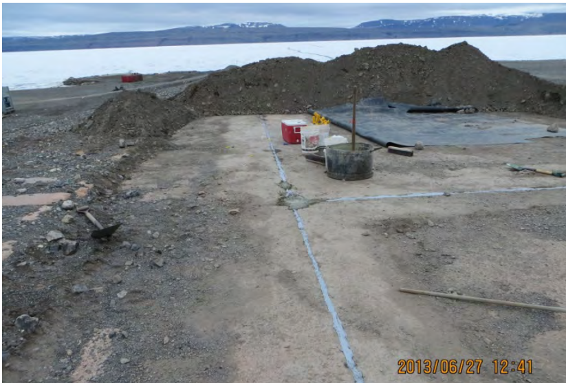
Photo 11: Preparation of the concrete pad for temporary storage of PHC contaminated soil. Cracks were sealed and a sump established
