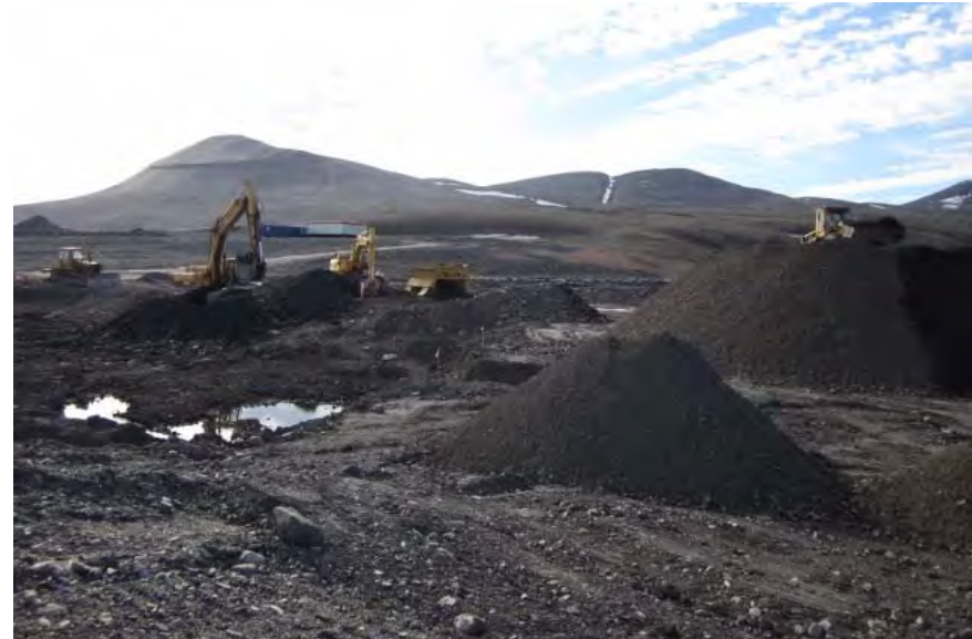
Photo 14: Stockpiles of screened fine PHC contaminated soil on right and excavation and screening plant in Area 1 on left.
