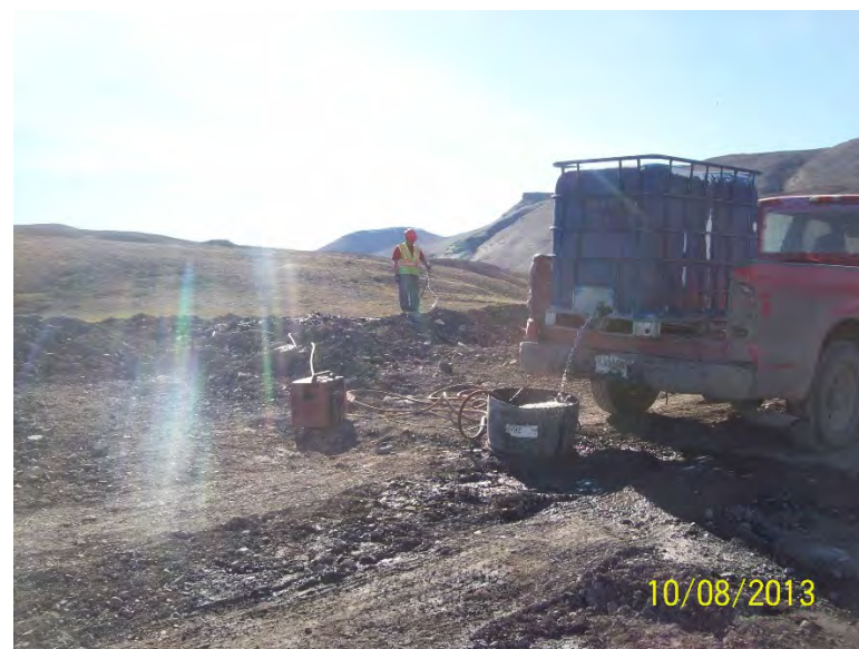
Photo 20: Apply water to the biopiles during an extended dry spell.
