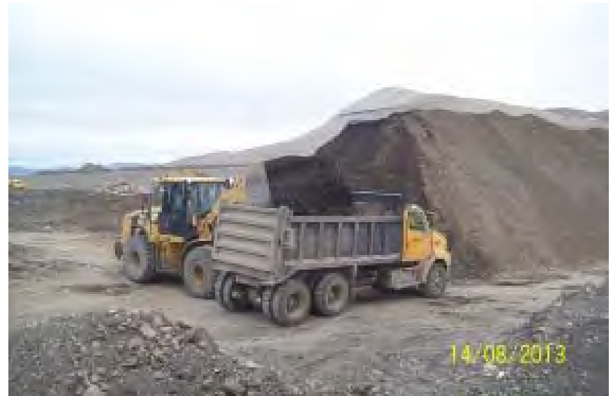
Photo 16: Part of the stockpile of screened fine PHC contaminated soil being relocated to the upper and lower treatment area.
