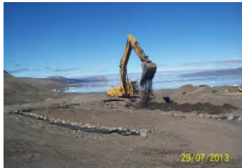
Photo 18: Aeration of a biopile in the upper treatment area.
