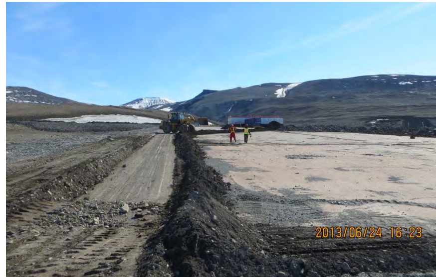
Photo 12: Preparation of the concrete pad for temporary storage of PHC contaminated soil. Berms were placed to divert surface water from the prepared area.
