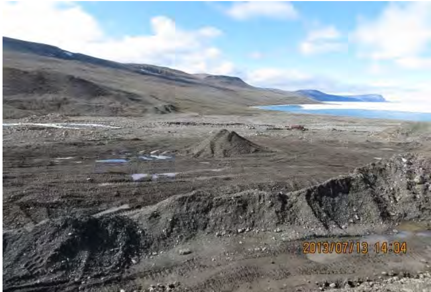
Photo 13: Stockpile of screened fine soil in former secondary containment area. Soil stockpiled here in 2012 was levelled off.
