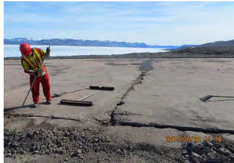
Photo 10: Preparation of the concrete pad for temporary storage of PHC contaminated soil. Soil was removed from the cracks.
