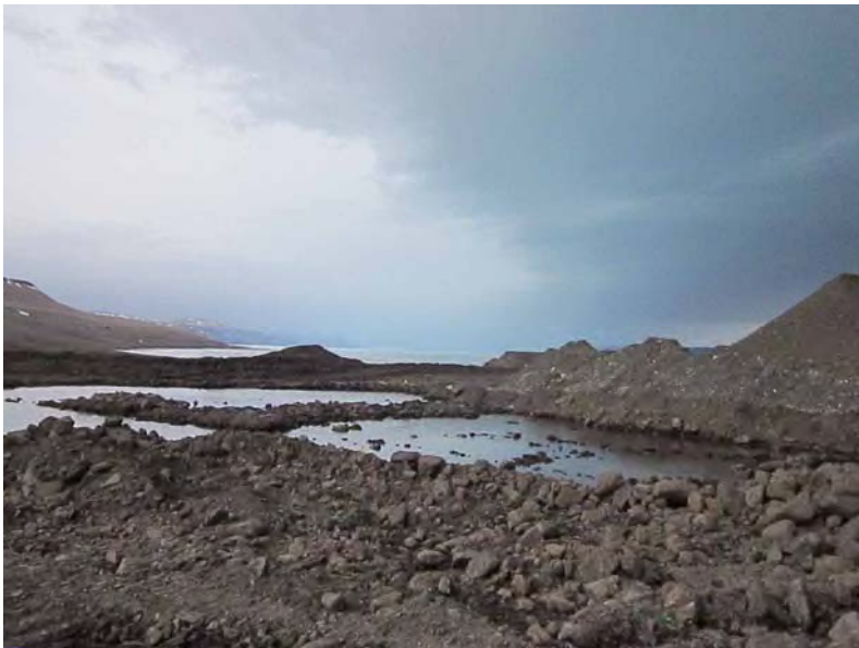
Photo 3: Excavation of Area 4 proceeded with the removal of an overlying layer of non PHC contaminated soil. Frozen ground restricted the risk of excavating into the underlying contaminated soil.
