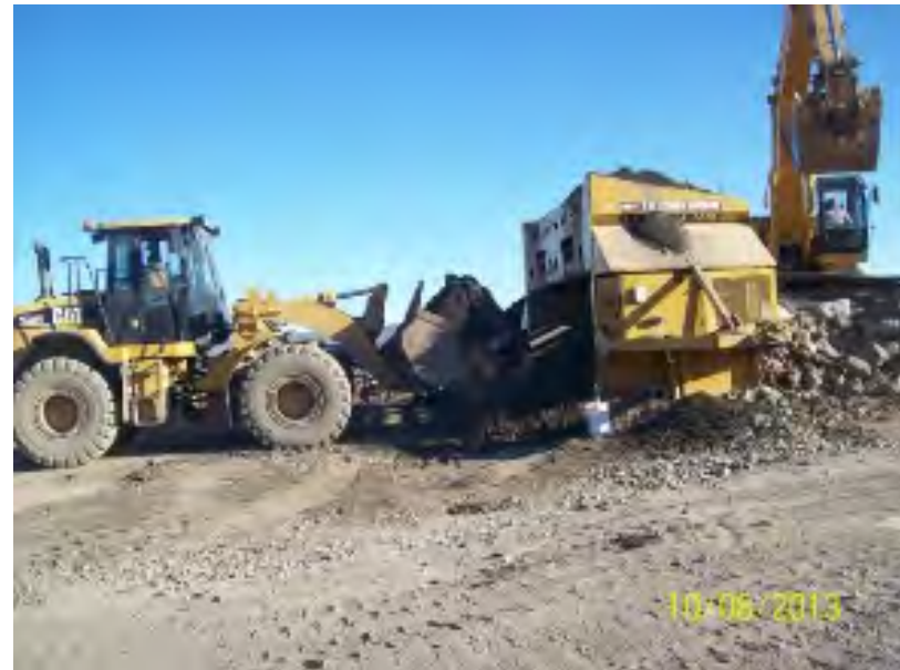
Photo 6: Soil passing through the vibrating screener.
