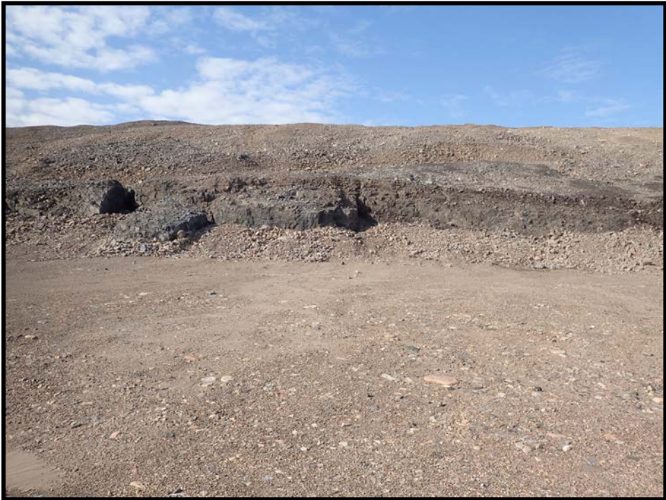
Photo 44. East Open Pit—Face of remnant highwall where cracking of crown pillar has been observed.
