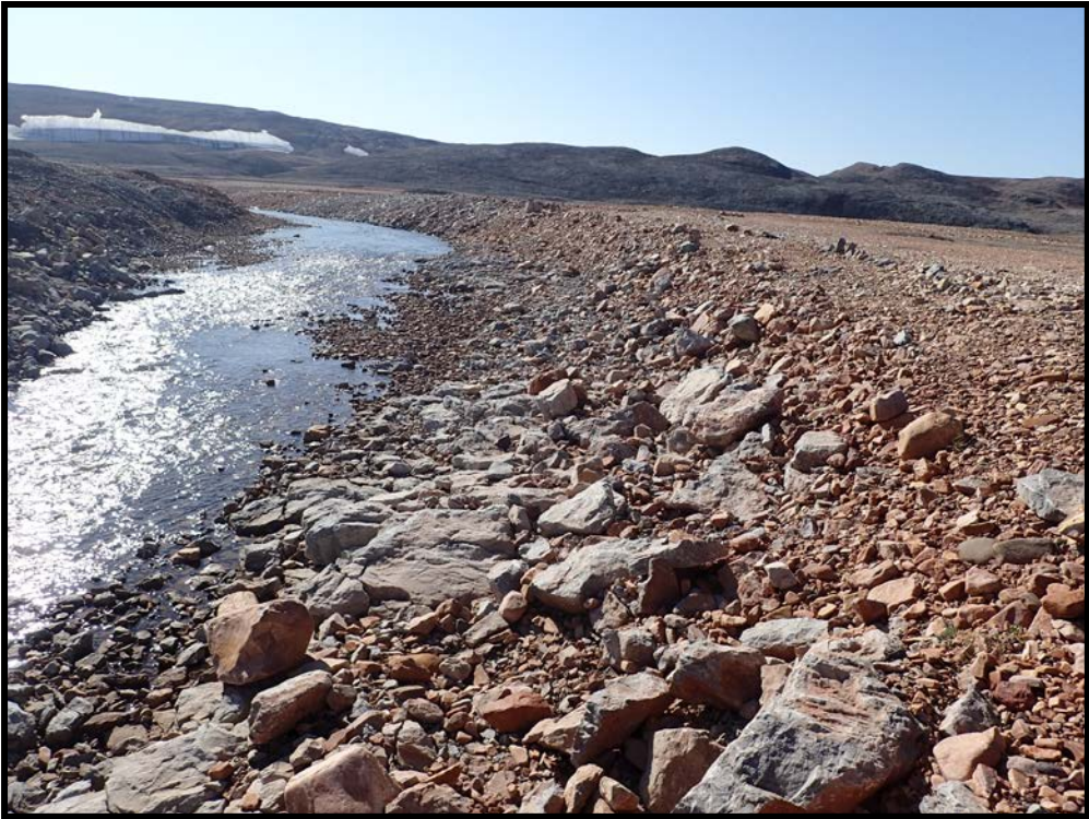
Photo 16. East Twin Creek Diversion Channel– View of area downstream of armoured area. Note bedrock outcrop along face of dyke and in bottom of channel.
