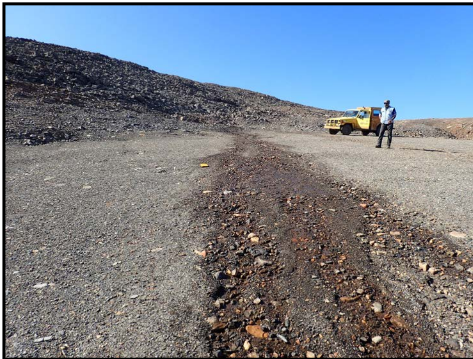
Photo 48. East Trench—Spring water running along surface of cover causing minor rill erosion
