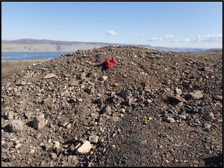
Photo 72. Oceanview East Raise. — Mound over backfilled raise. No settlement has been observed.
