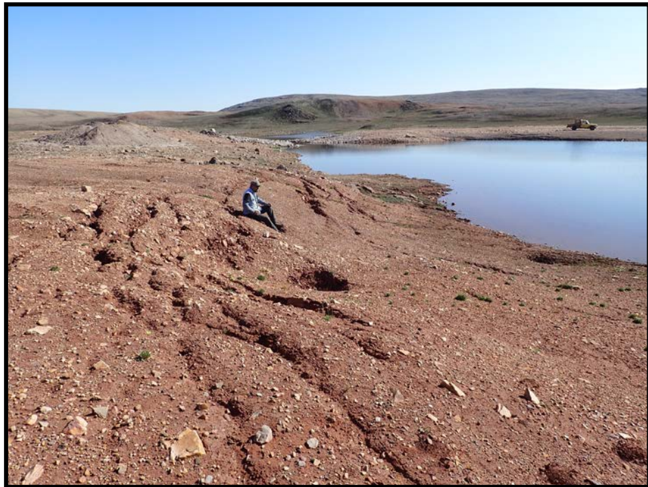
Photo 12. West Twin Outlet Channel—Settlement induced cracking along north edge of polishing pond.
