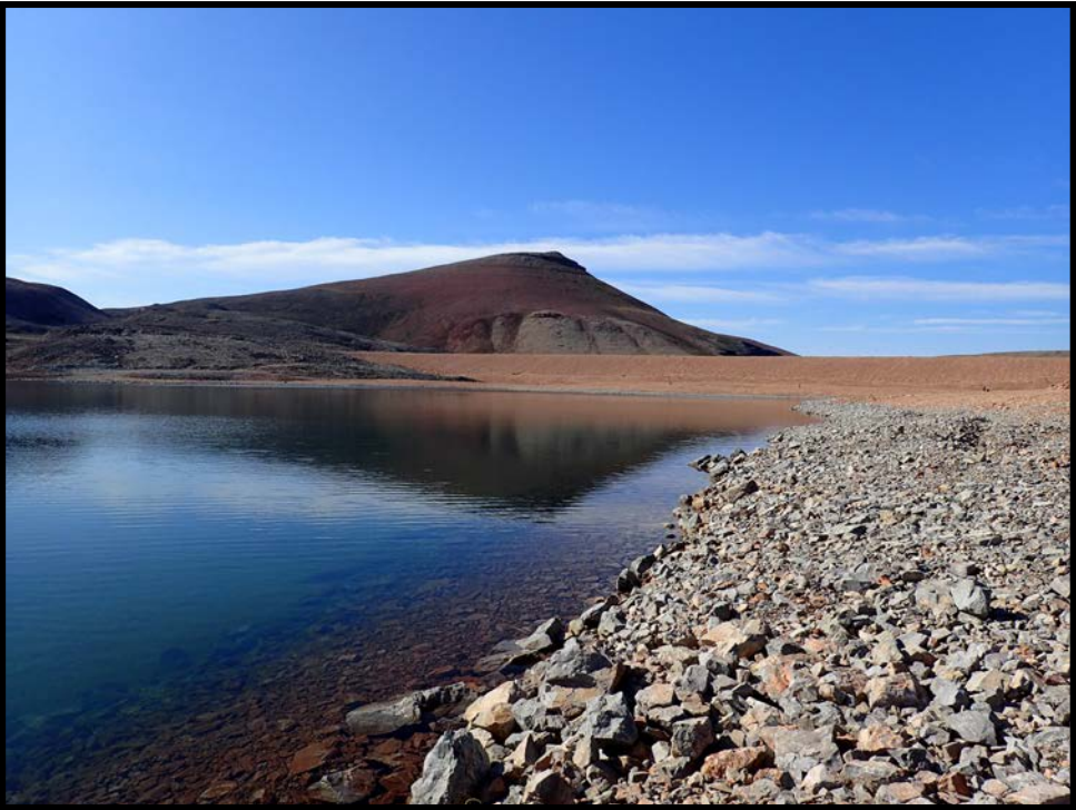
Photo 30. Toe of Test Cell Dyke—Armour along shoreline of cover at toe of Test Cell Dyke. East/West arm, view looking west.
