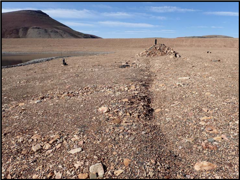
Photo 23. Test Cell—Settlement trough along edge of East/West Test Cell dyke.
