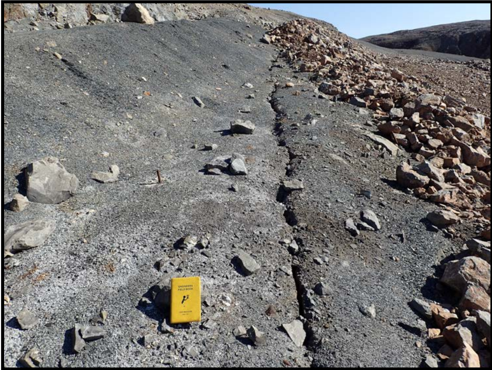
Photo 39. West Open Pit—Crack in crown pillar. Note that there has been no visual change in the 10 years since closure.
