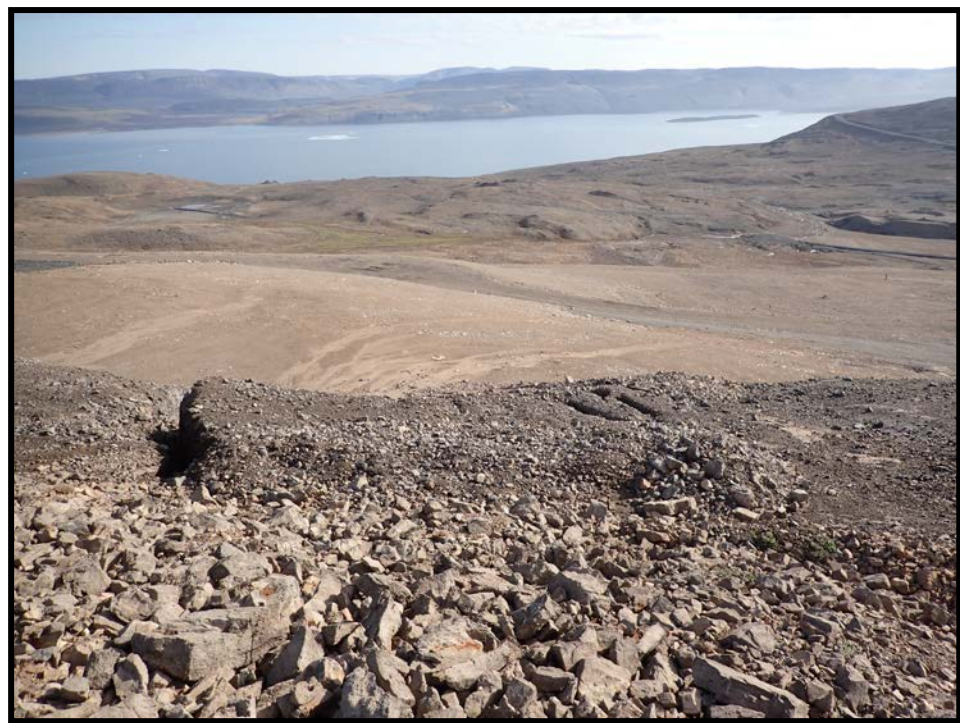
Photo 46. East Open Pit—Cracking in crown pillar. Similar condition to 2014.
