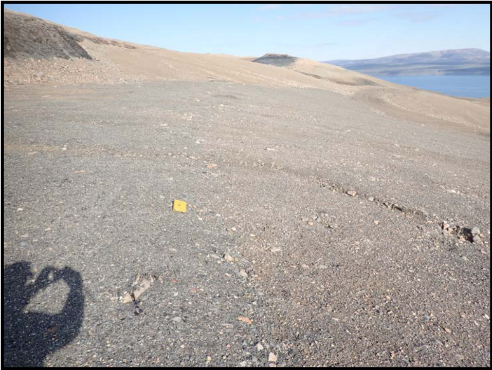
Photo 43. East Open Pit— At transition from flat to sloping upper surface of cover system. Note minor settlement and cracking.
