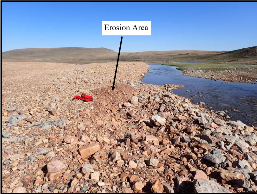
Photo 15. East Twin Creek Diversion Channel– Erosion area noted above seepage discharge point. Erosion is similar to 2013.
