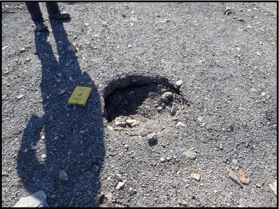
Photo 52. Oceanview Open Pit—Small sinkhole in middle of cover system. Note little visible change since 2014.
