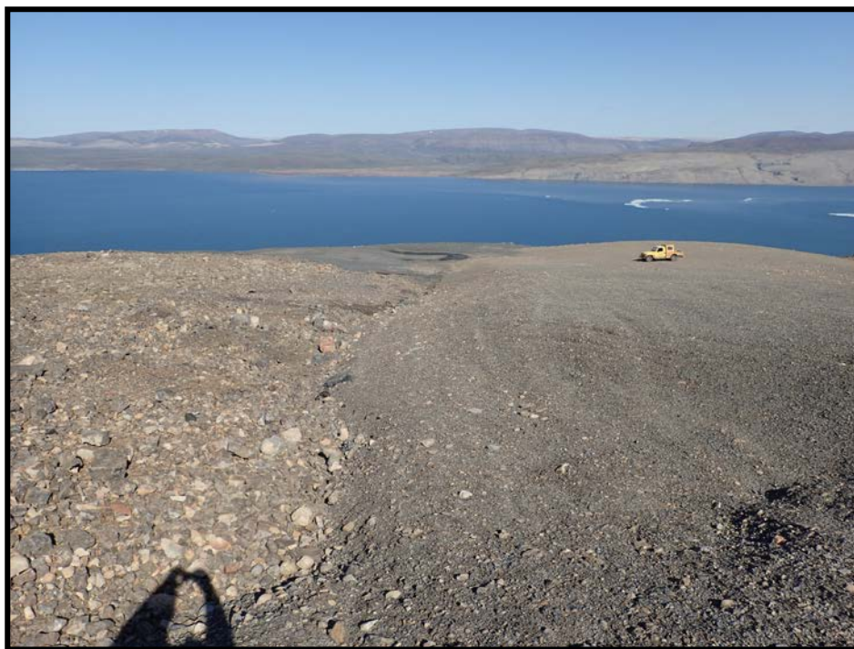
Photo 63. Oceanview Portal—Settlement area along west edge of cover. Note very little to no change in 10 years.
