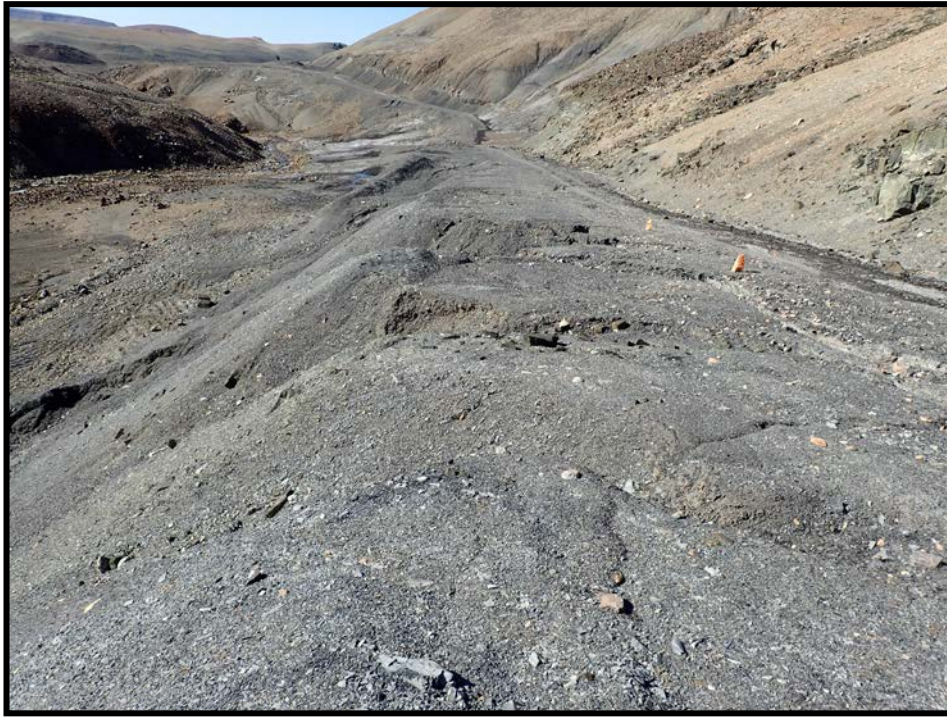
Photo 67. 09S Portal—Eroding road between 09S and 17N portals.
