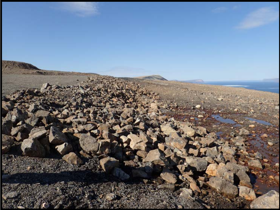
Photo 49. Oceanview Open Pit—Toe of cover system. Note seepage emerging at the bottom of toe.
