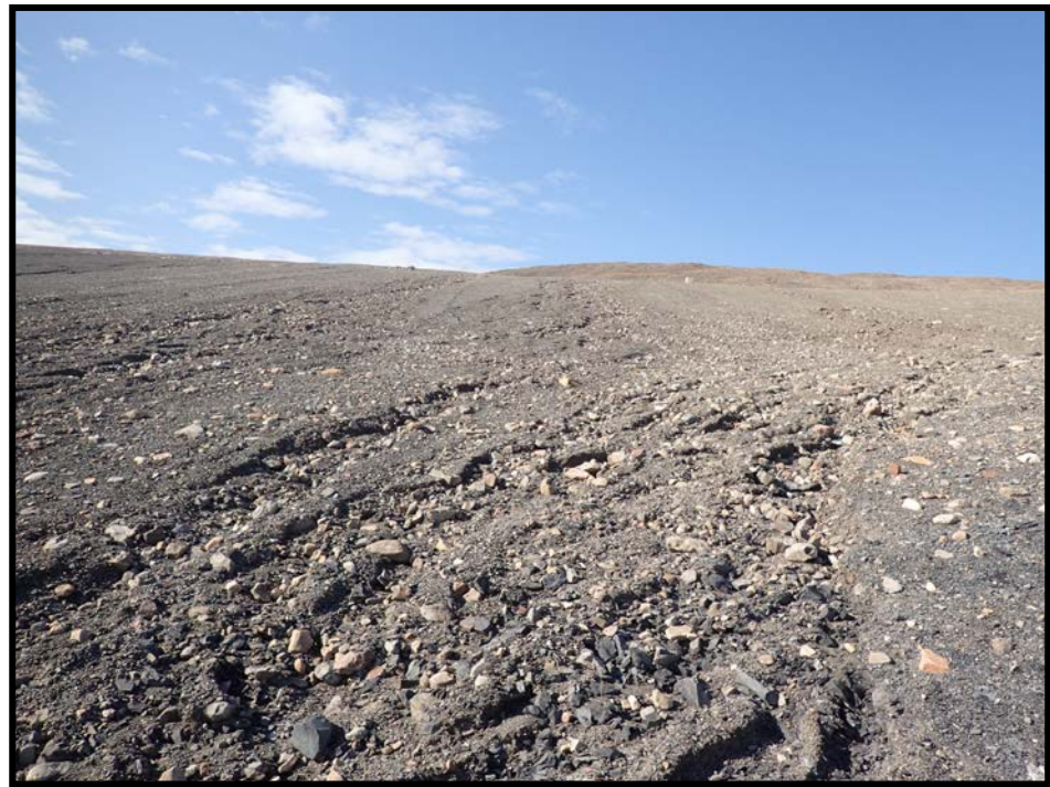
Photo 45. East Open Pit—Looking upslope along lower sloping face of cover. Note rill erosion.
