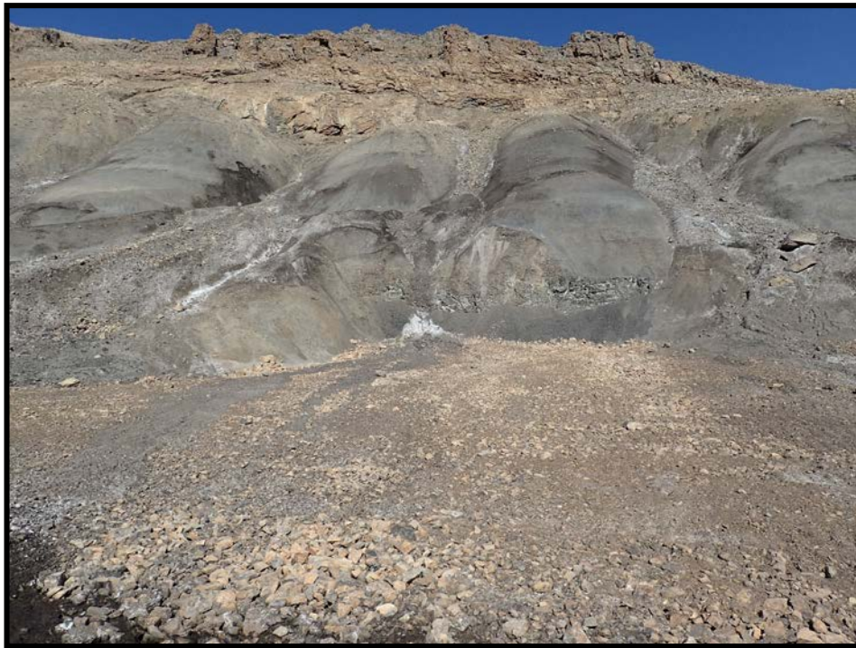
Photo 68. 09S Portal—Looking upslope along surface of cover. Note shale deposited on top of armour from upslope.
