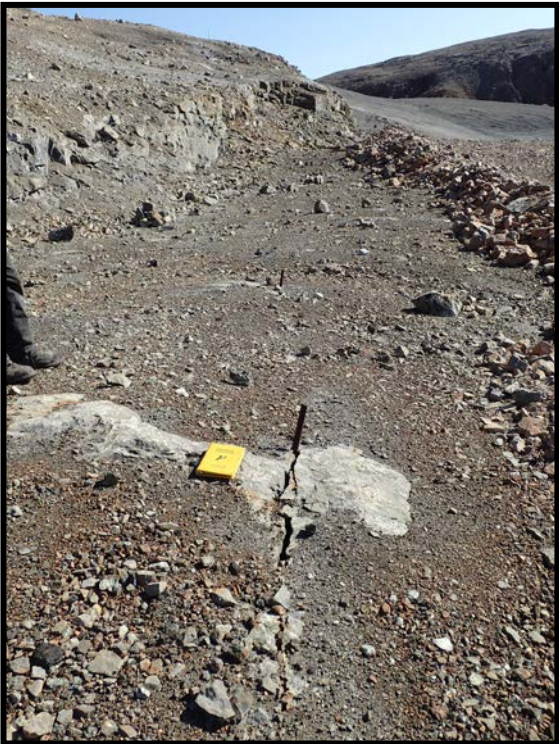
Photo 40. West Open Pit—Crack in crown pillar. Note that there has been very little change in the 10 years since closure.
