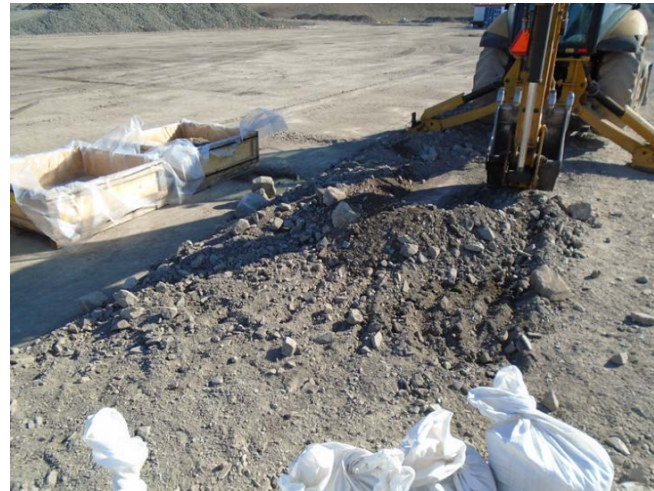
Photo 8: Lead and zinc concentrate contaminated soil was shoveled into bags and then a backhoe used to scrape the underlying soil. The bags and soil were deposited in the wood boxes. Facing southeast.
