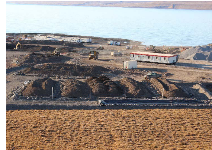
Photo 12: Treatment cells containing PHC contaminated soils. Facing north.
