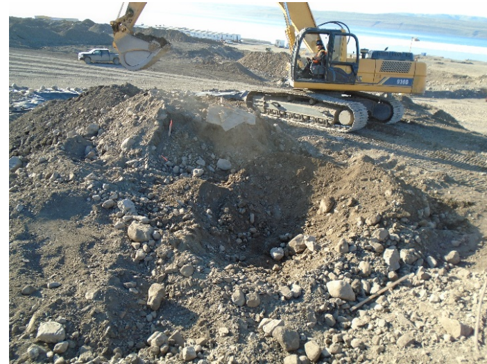
Photo 10: Excavation of waste concentrate contaminated soil from LTA2 and LTA3. Facing northwest.
