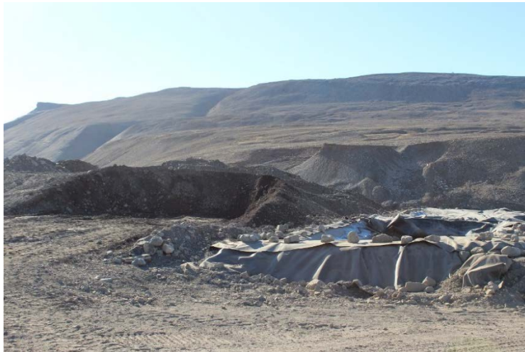
Photo 11: Soil recovered from LTA2 and LTA3 is placed in LTA stormwater retention pond and covered. Facing west.
