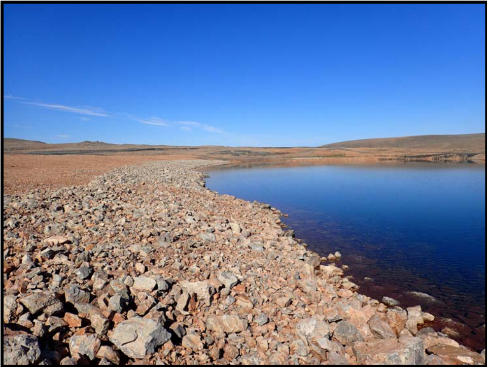
Photo 29. Toe of Test Cell Dyke—Armour along shoreline of cover at toe of Test Cell Dyke. East/West arm, view looking east.
