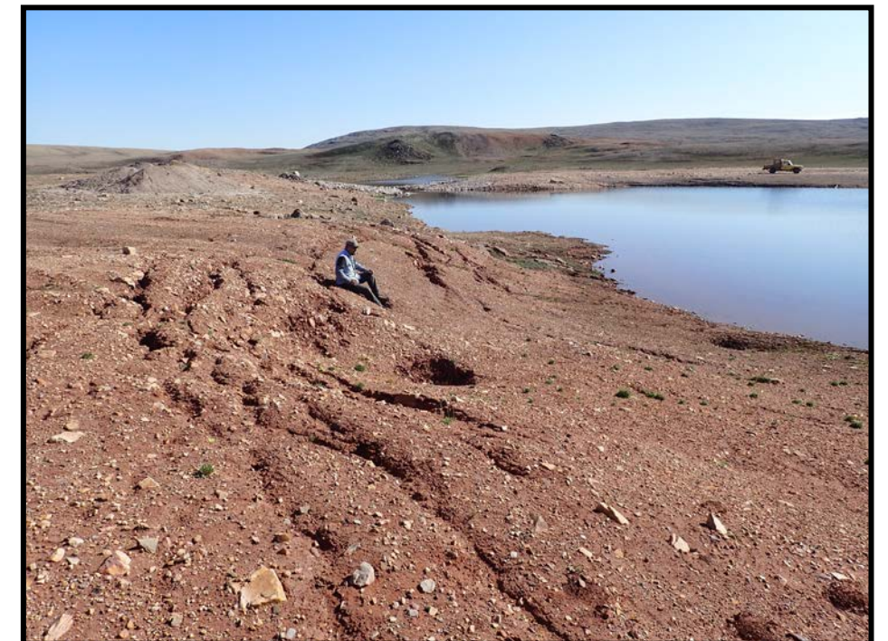
Photo 12. West Twin Outlet Channel—Settlement induced cracking along north edge of polishing pond.
