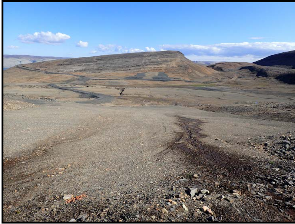
Photo 47. East Trench—Trench cover as seen from upslope edge. Not small flow of water on surface of cover causing minor rill erosion.
