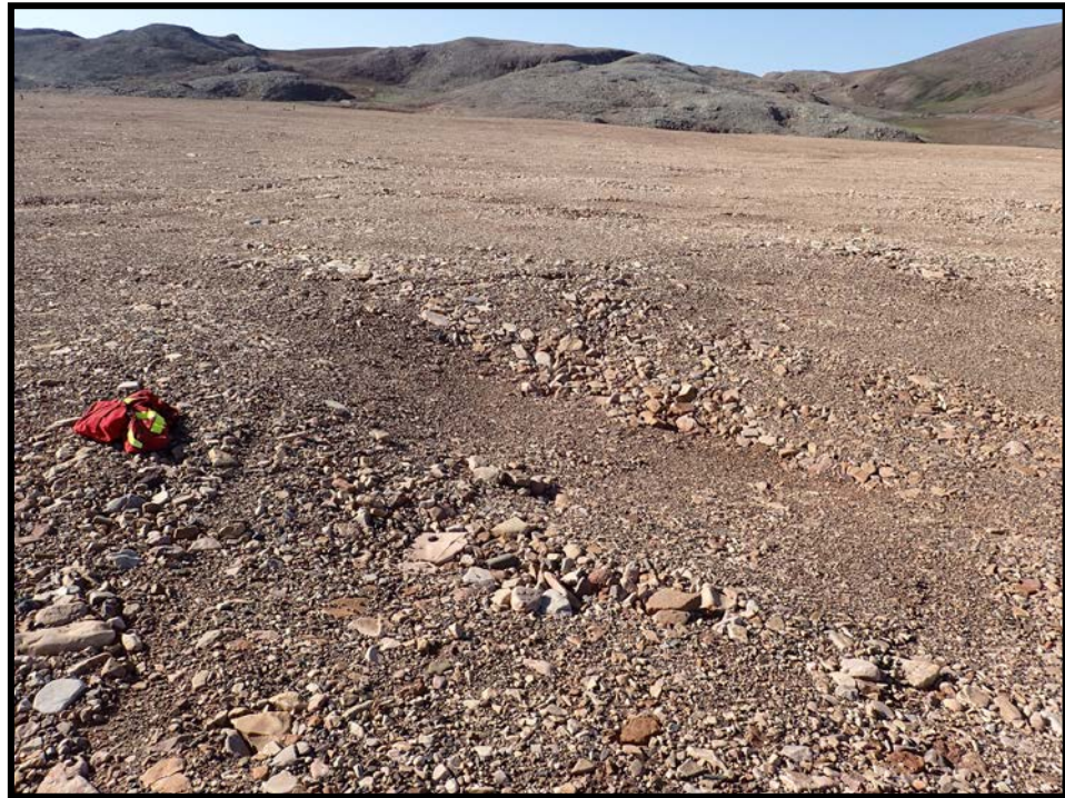
Photo 17. Surface Cell—Thermokarst settlement near E/W drainage channel.
