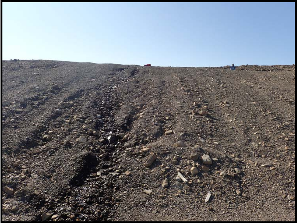
Photo 50. Oceanview Open Pit—Rill erosion along backslope. Note self armouring that is occurring.
