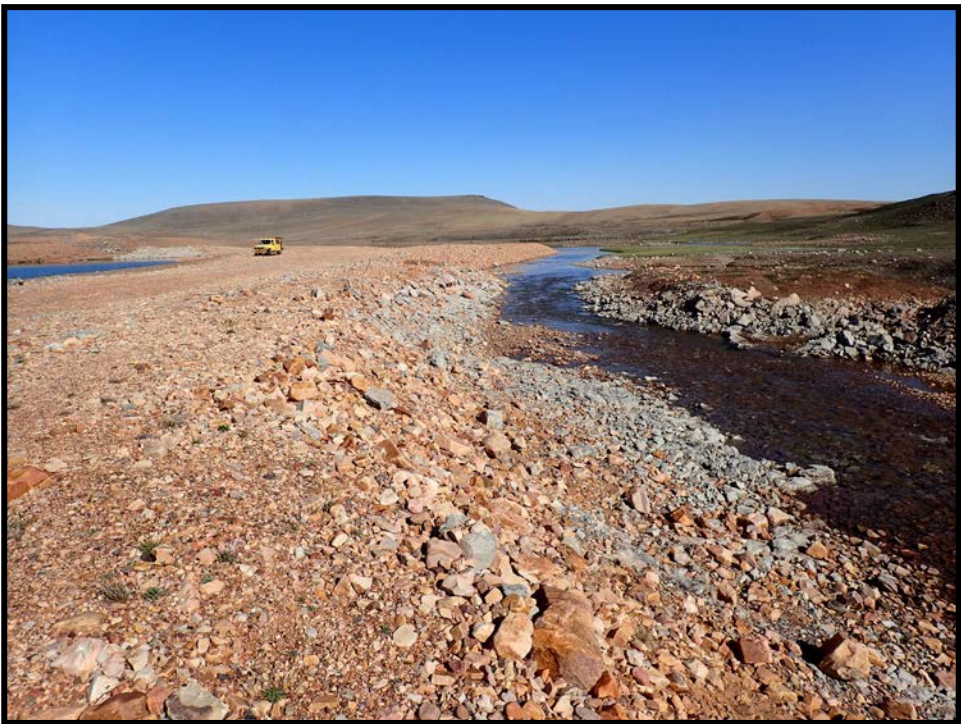
Photo 14. East Twin Creek Diversion Channel– View of area downstream of armoured area. Note bedrock outcrop along face of dyke and in bottom of channel.
