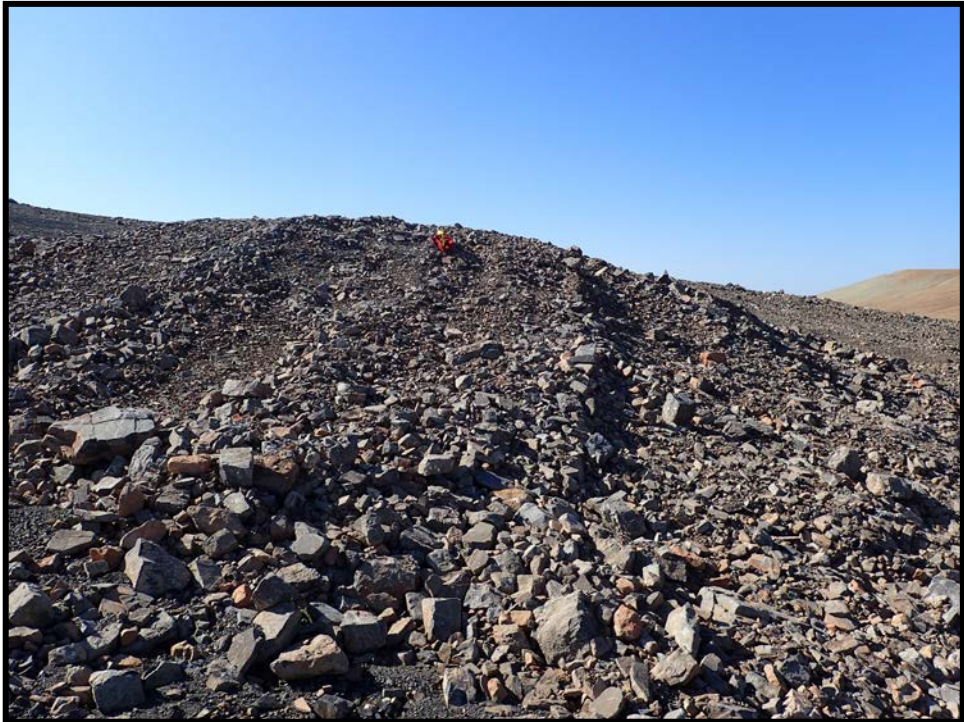
Photo 71. Shale Hill Raise—Mound over backfilled raise. No settlement has been observed.
