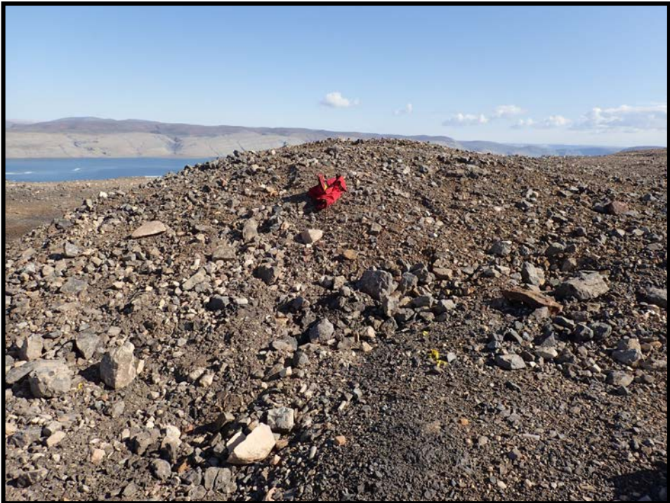
Photo 73. Oceanview West Raise— Mound over backfilled raise. No settlement has been observed.
