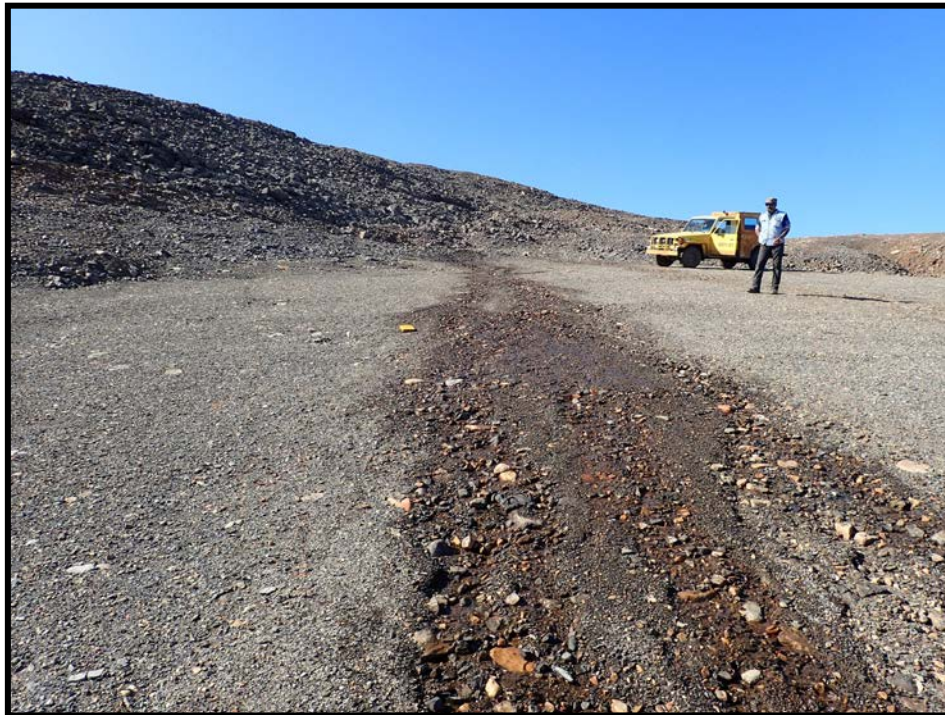
Photo 48. East Trench—Spring water running along surface of cover causing minor rill erosion
