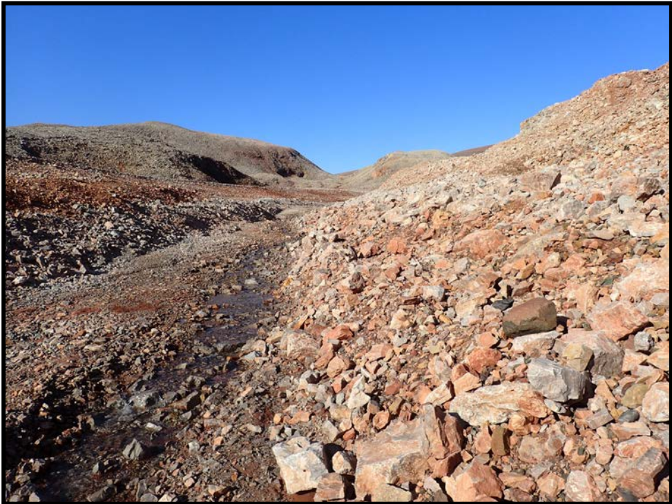
Photo 6. West Twin Dyke Spillway—Looking upstream along left bank of spillway. Note erosion scar approximately 1-2 m above base of spillway.
