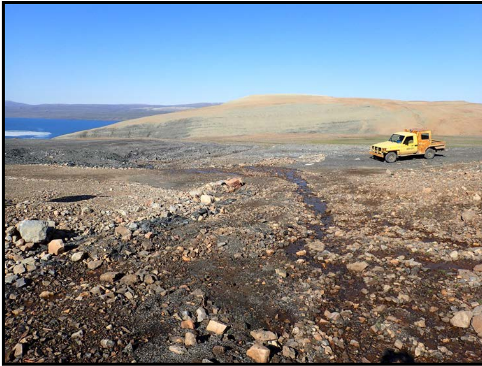
Photo 60. 17N Portal—Surface water running along east edge of portal cover.
