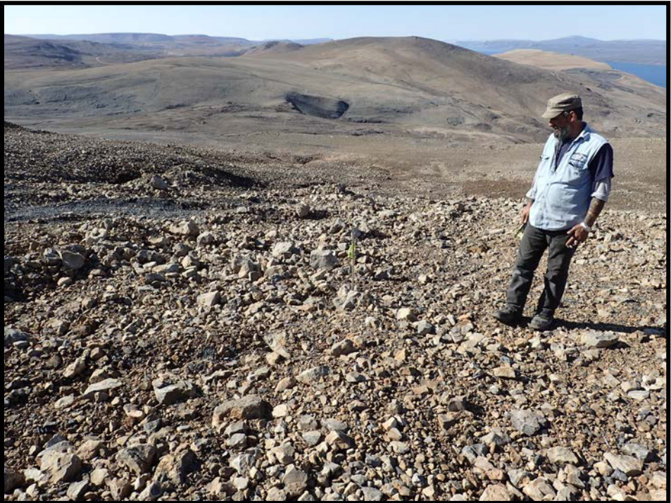
Photo 74. Area 14 Raise—Graded area above backfilled raise. Note stake with flagging denoting approximate location of raise.
