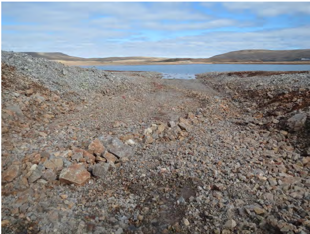
Photo 8. West Twin Dyke Spillway—Deposition of eroded material in bottom of spillway.
