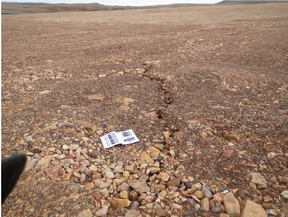
Photo 19. Surface Cell—Cracking in secondary N/S drainage swale. View looking north.
