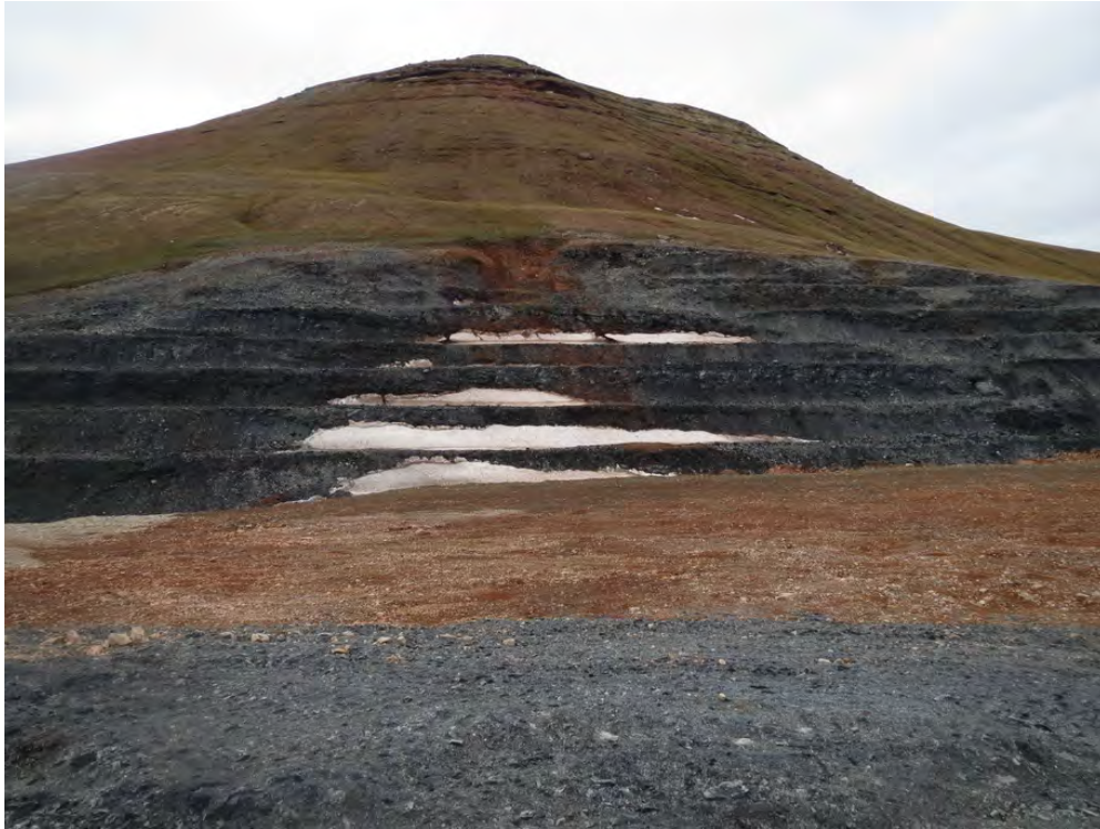
Photo 75. Mt. Fuji Shale Quarry—Note ongoing sloughing of bench faces reducing overall slope.
