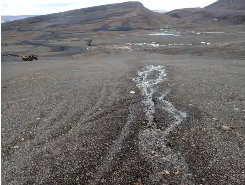
Photo 45. East Trench—Trench cover as seen from upslope edge. Note small flow of water on surface of cover causing minor rill erosion.
