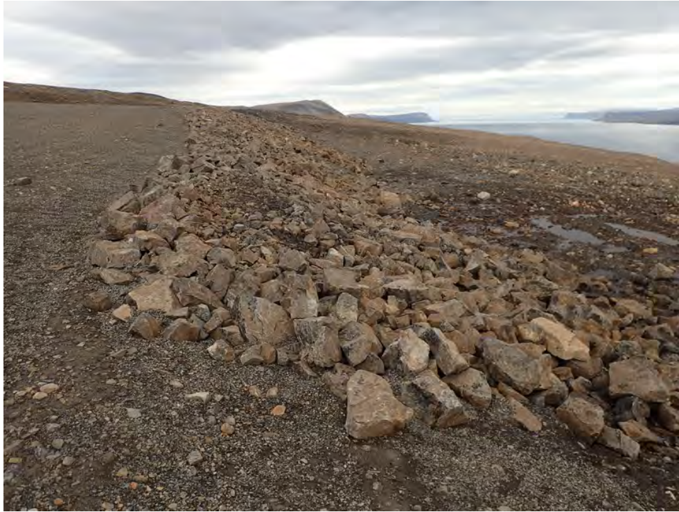
Photo 47. Oceanview Open Pit—Toe of cover system. Note seepage emerging at the bottom of toe.
