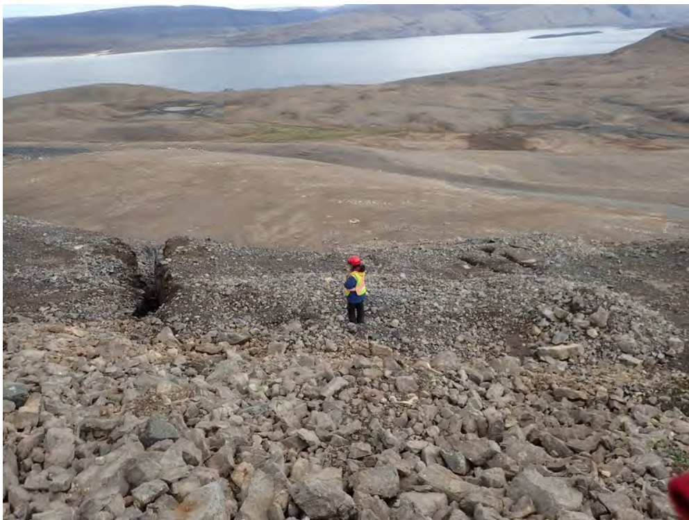
Photo 44. East Open Pit—Cracking in crown pillar. Similar condition to 2015.
