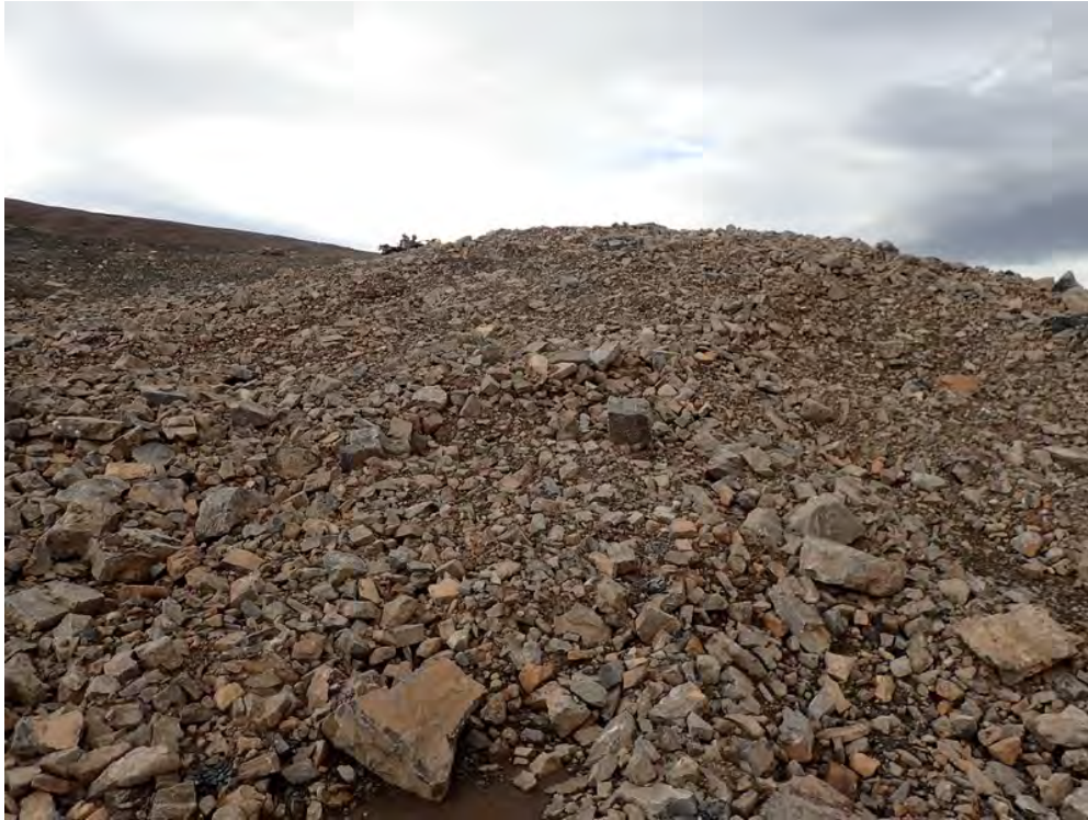
Photo 69. Shale Hill Raise—Mound over backfilled raise. No settlement has been observed.
