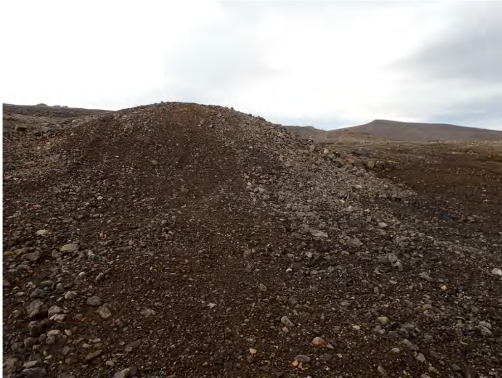
Photo 71. Oceanview West Raise— Mound over backfilled raise. No settlement has been observed.
