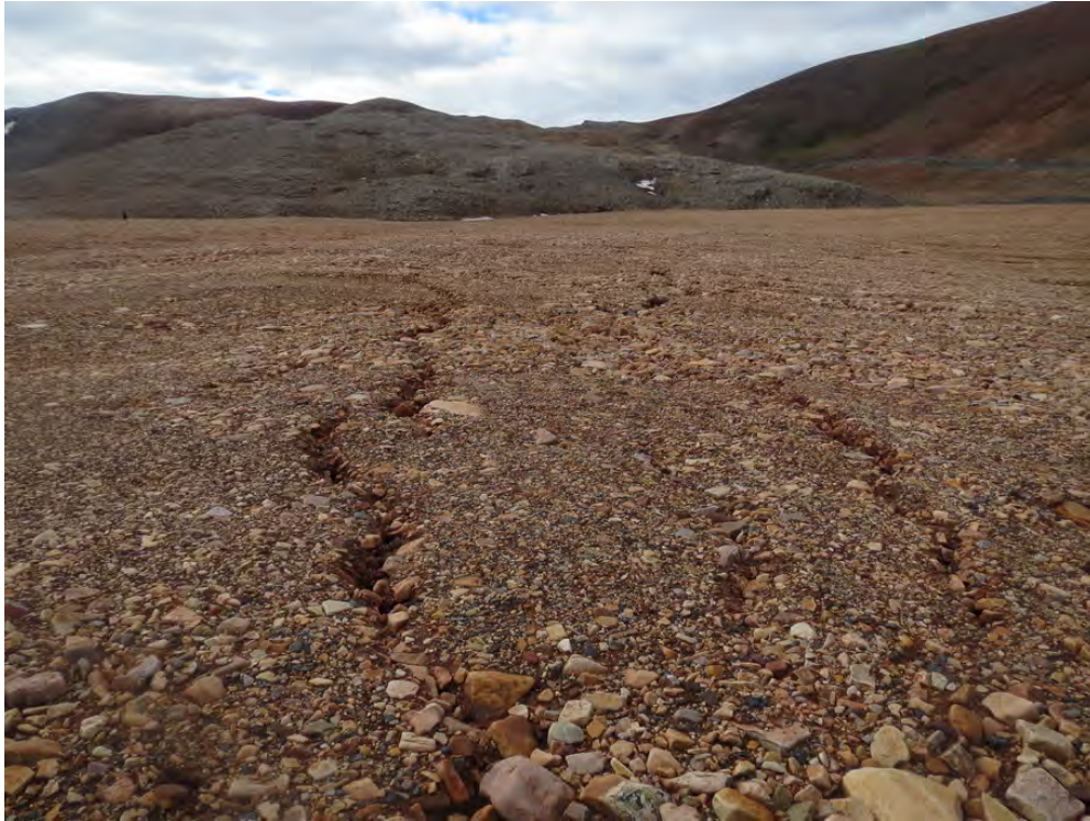
Photo 17. Surface Cell—Surface Cell cover system. Note cracking of surface of cover.
