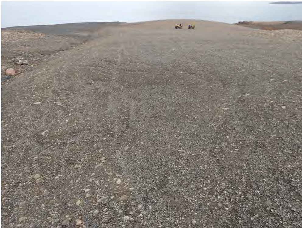
Photo 61. Oceanview Portal—Settlement area along west edge of cover. Note very little to no change in 10 years.
