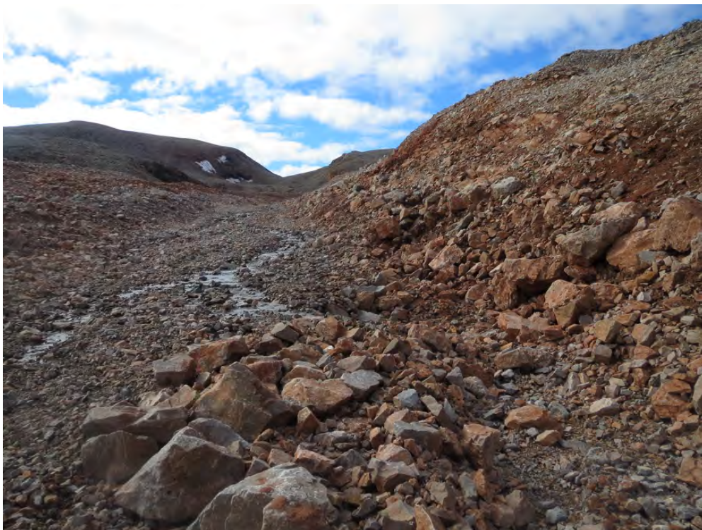
Photo 6. West Twin Dyke Spillway—Erosion along left bank of spillway.
