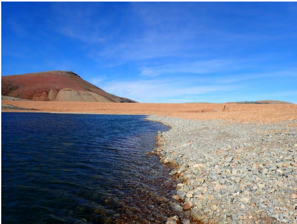
Photo 30. Toe of Test Cell Dyke— Looking west along armoured shoreline at toe of Test Cell Dyke.
