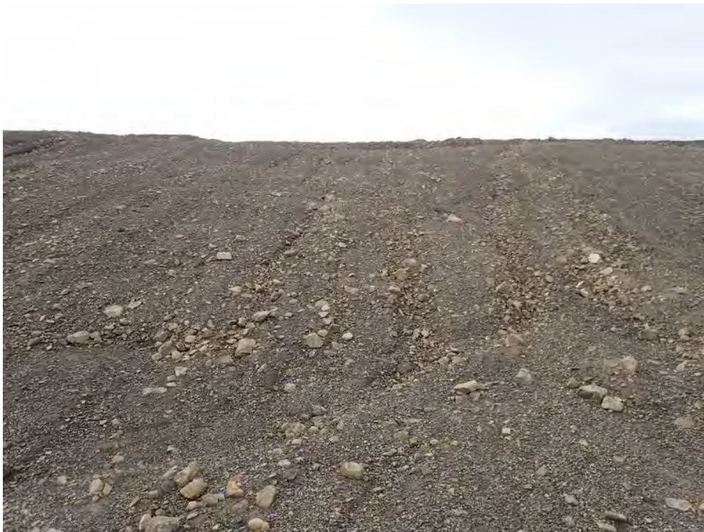
Photo 48. Oceanview Open Pit—Rill erosion along backslope. Note self armoring that is occurring.
