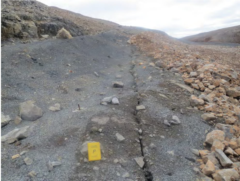
Photo 37. West Open Pit—Crack in crown pillar. No visual change in the 10 years since closure.
