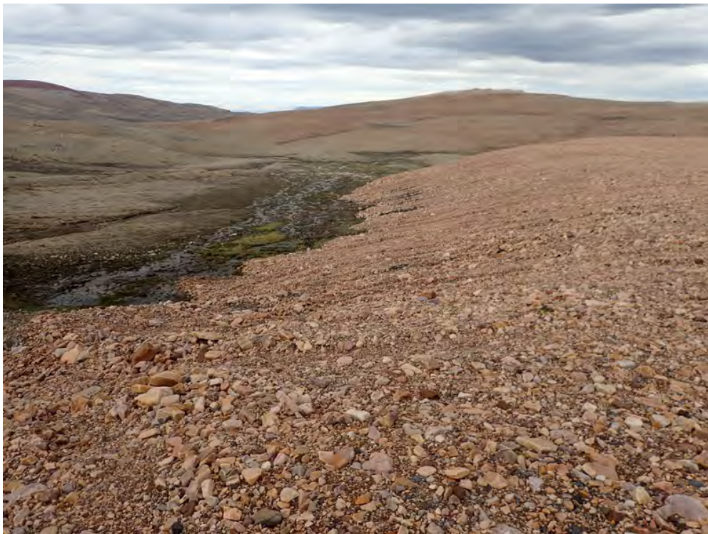
Photo 36. Landfill–Toe of landfill cover system. Note surface water flow along toe of cover.
