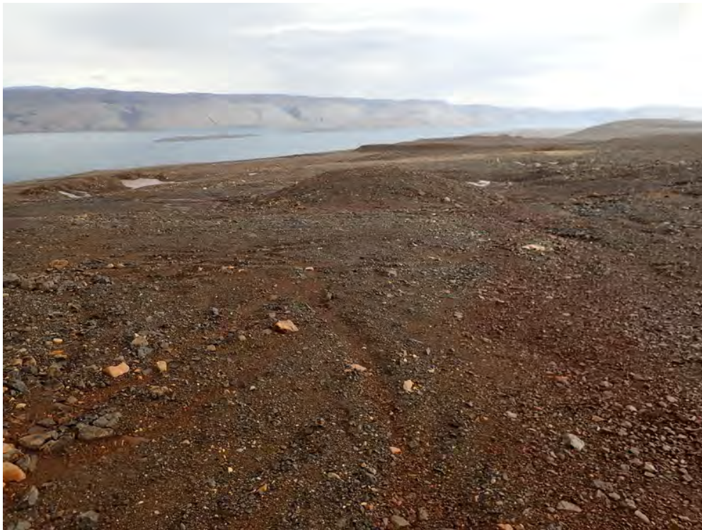
Photo 70. Oceanview East Raise—Mound over backfilled raise. No settlement has been observed.
