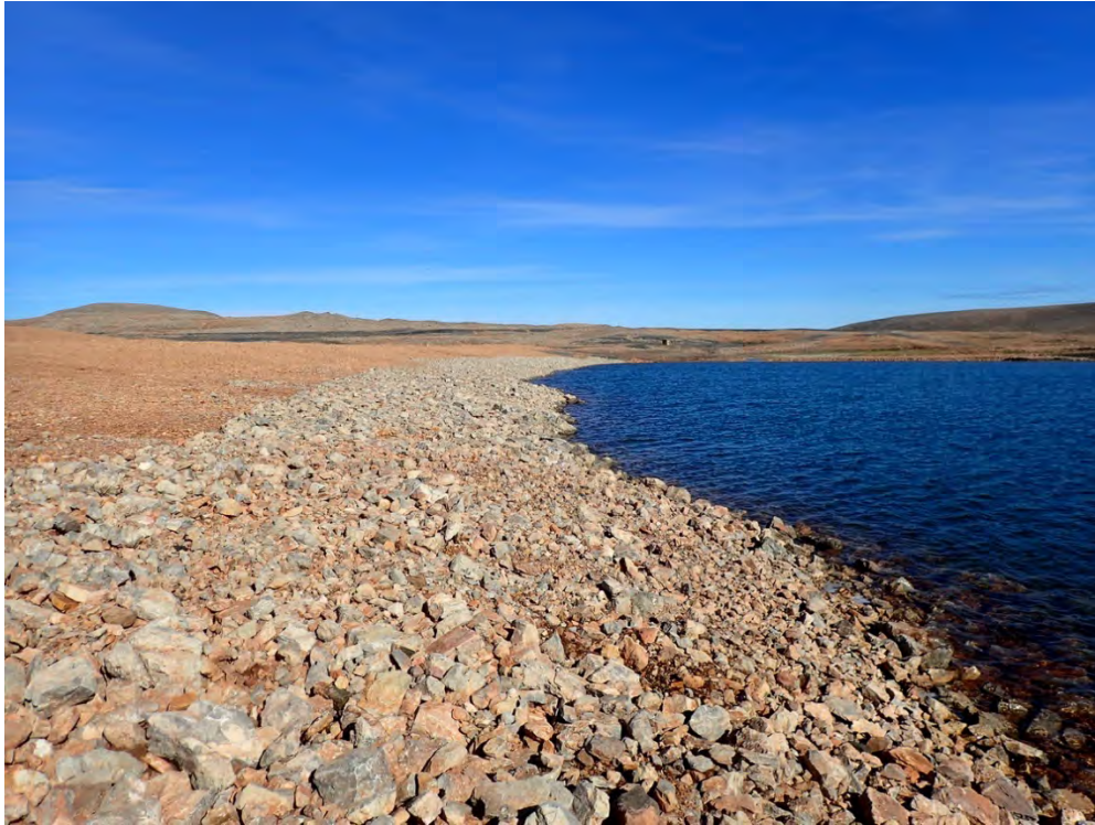
Photo 29. Toe of Test Cell Dyke—Looking north along armoured shoreline at toe of Test Cell Dyke.
