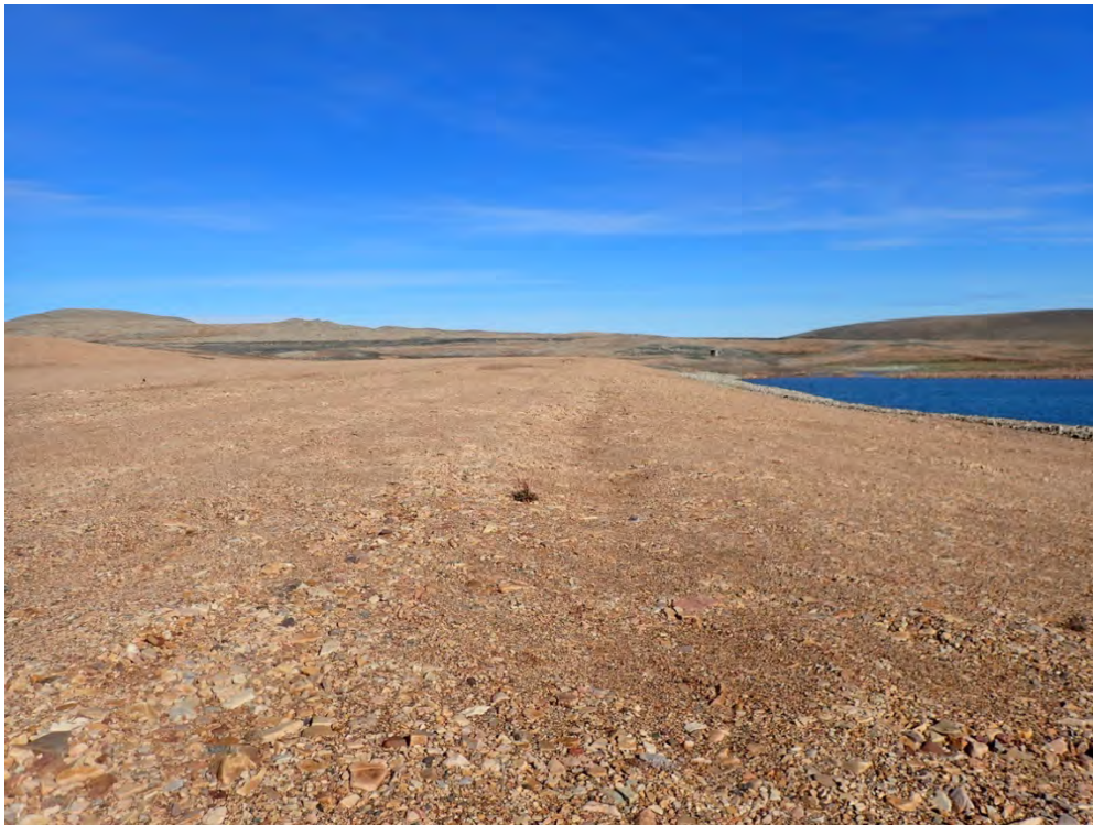
Photo 24. Test Cell—Settlement trough along north/south arm of Test Cell dike.
