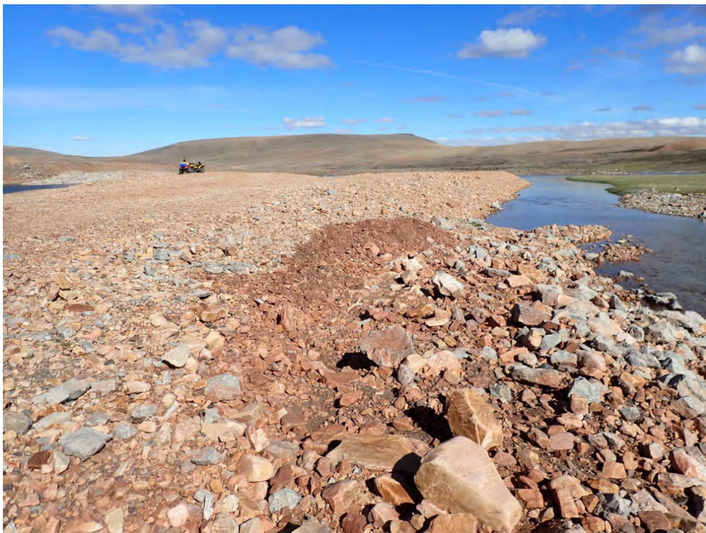
Photo 14. East Twin Creek Diversion Channel —Erosion along face of dyke.
