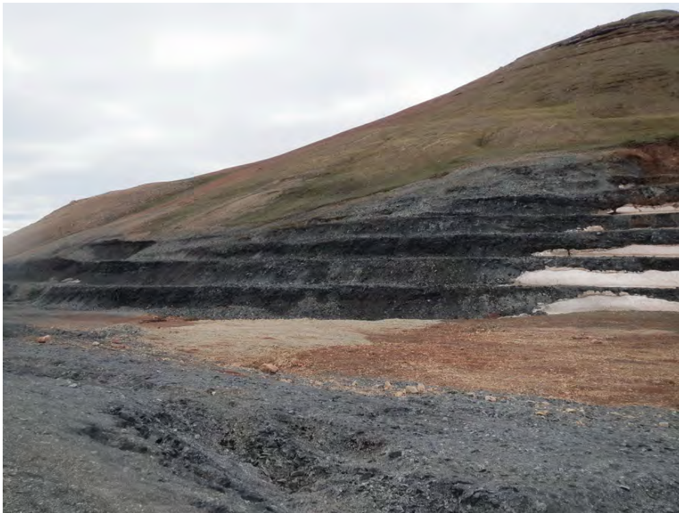
Photo 76. Mt. Fuji Shale Quarry—Note ongoing sloughing of bench faces reducing overall slope.
