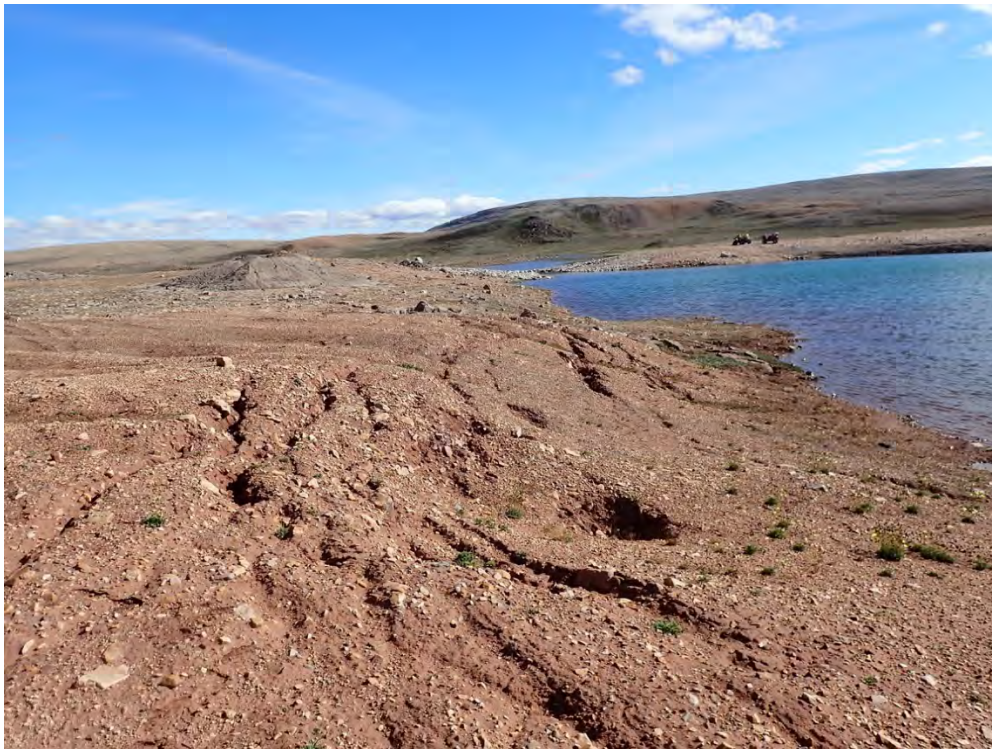
Photo 12. West Twin Lake Outlet Channel—Settlement and cracking along north edge of polishing pond.
