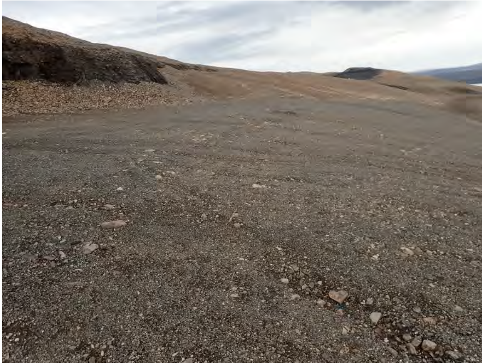
Photo 41. East Open Pit— At transition from flat to sloping upper surface of cover system. Note minor settlement and cracking.
