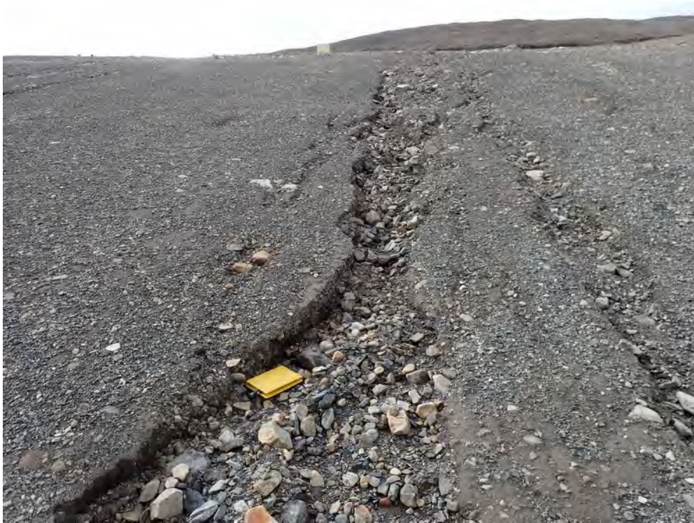
Photo 43. East Open Pit—Looking upslope along lower sloping face of cover. Note rill erosion.
