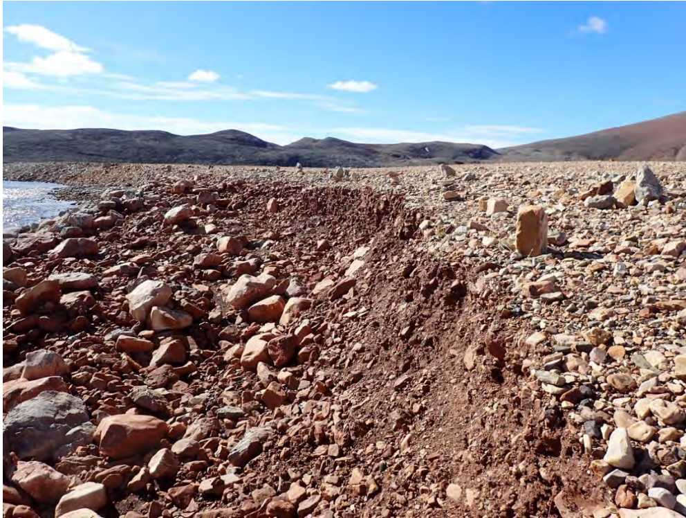
Photo 13. East Twin Creek Diversion Channel—Erosion along face of dyke.
