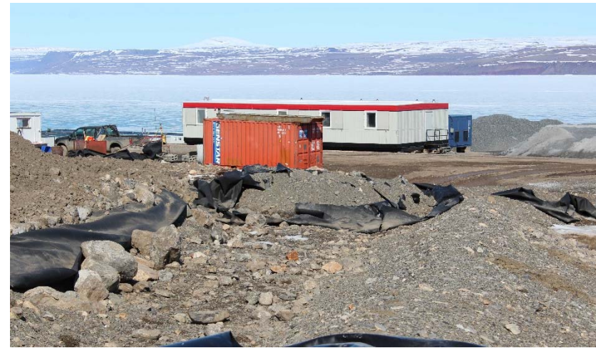
Photo 4: A stockpile of PHC contaminated soil was observed to have been placed to the east of treatment cell UTA5 on June 8, 2016. Facing north.
