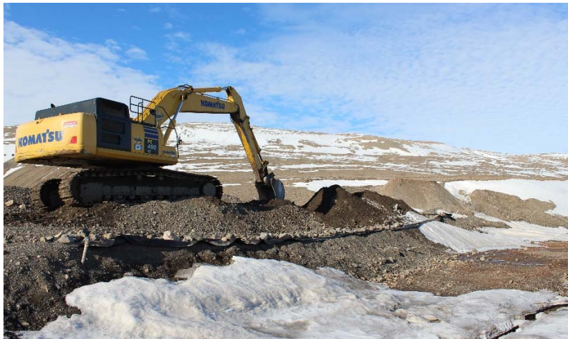
Photo 3: The soil in the UTA is being aerated in early June. Facing west.
