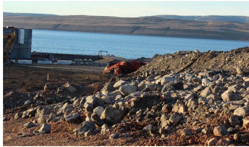
Photo 8: The liner was consolidated into a single stockpile at the LTA and covered with orange snow fencing to secure it in place over the winter. Facing north.
