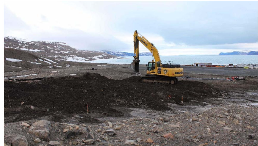
Photo 2: Biopiles with a height of approximately 1.5 m were re-established in the LTA in early June. Facing north.
