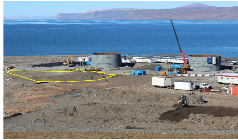
Photo 6: The stockpile of remediated soil is outlined in yellow. Closure samples were collected from the base of the LTA after the liner was removed. Facing north.
