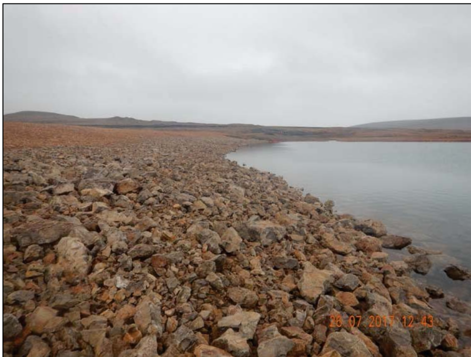
Photo 28. Test Cell – Armour along shoreline of N/S arm of TC Dyke.
