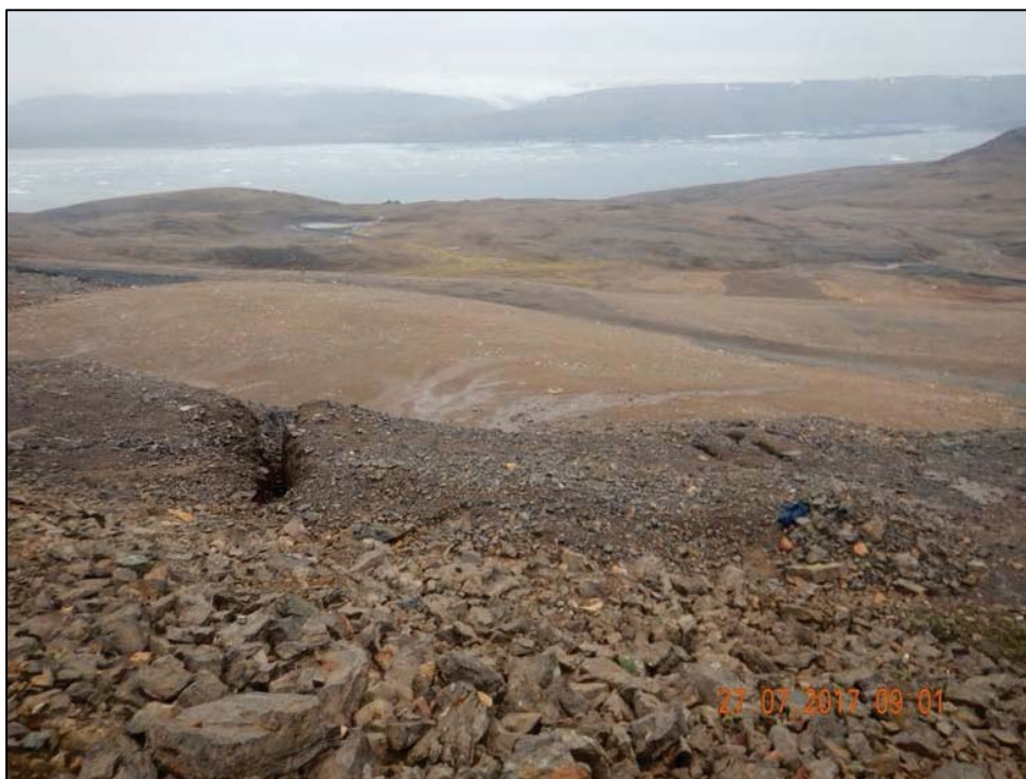
Photo 44. East Open Pit – Crack in crown pillar of EOP.
