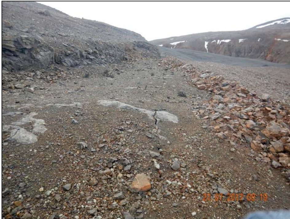
Photo 41. West Open Pit – Crack in crown pillar of WOP.
