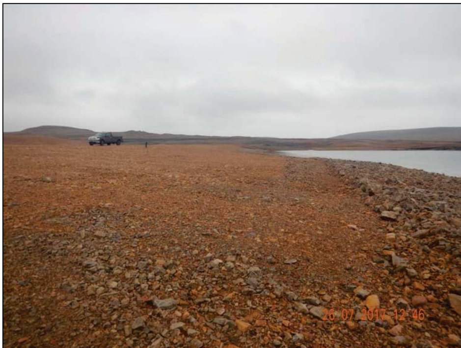
Photo 30. Test Cell – Sloping face of cover along outside face of N/S arm of TC Dyke.
