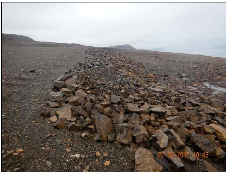
Photo 50. Oceanview Pit – Armoured face of slope at toe of cover system.
