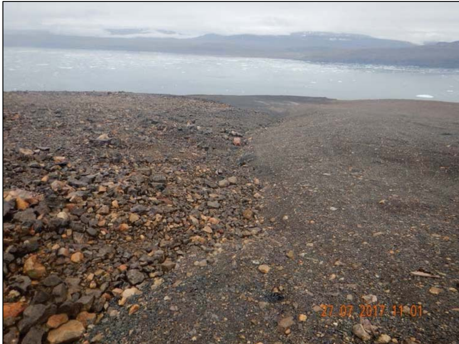
Photo 68. Oceanview Portal – West edge of portal cover. Note old settlement area not showing any signs of ongoing deformation.
