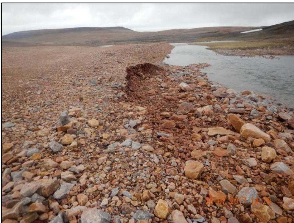
Photo 12. ETC Diversion Channel – Erosion area along left bank of diversion channel.
