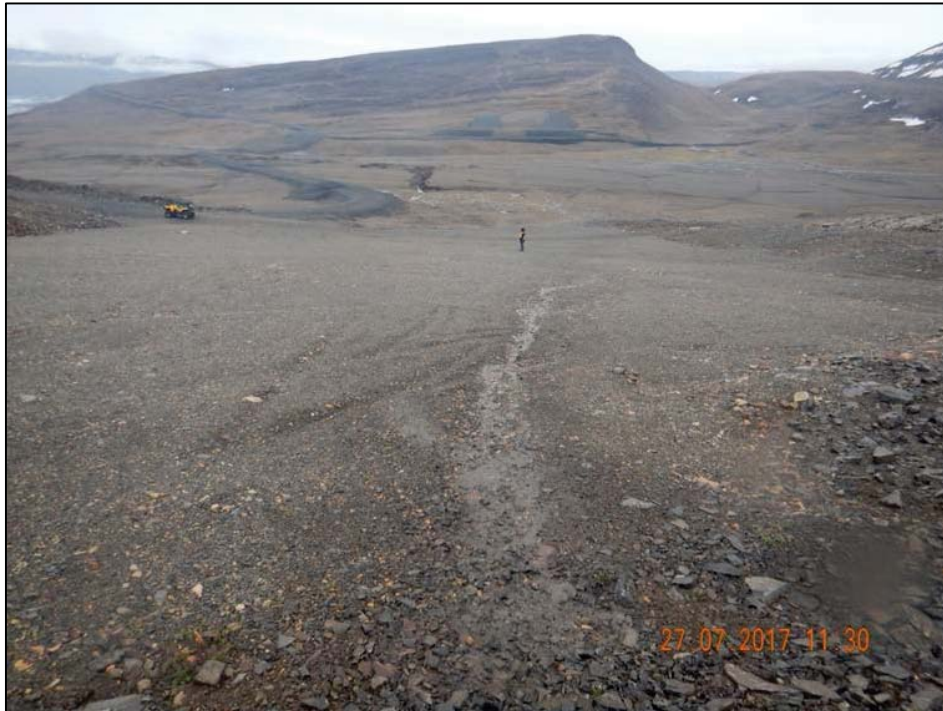
Photo 49. East Trench – Rill erosion on surface of cover system view looking downslope.
