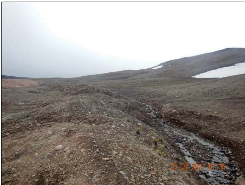
Photo 38. Landfill – Upslope diversion berm.
