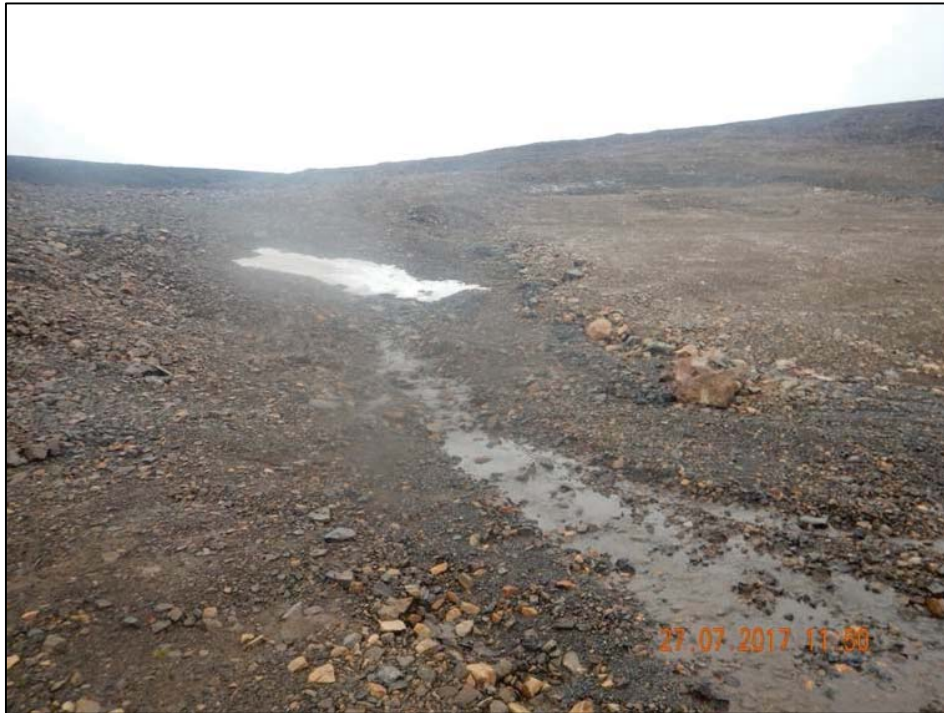
Photo 63. 17N Portal – Water running along east edge of portal cover.
