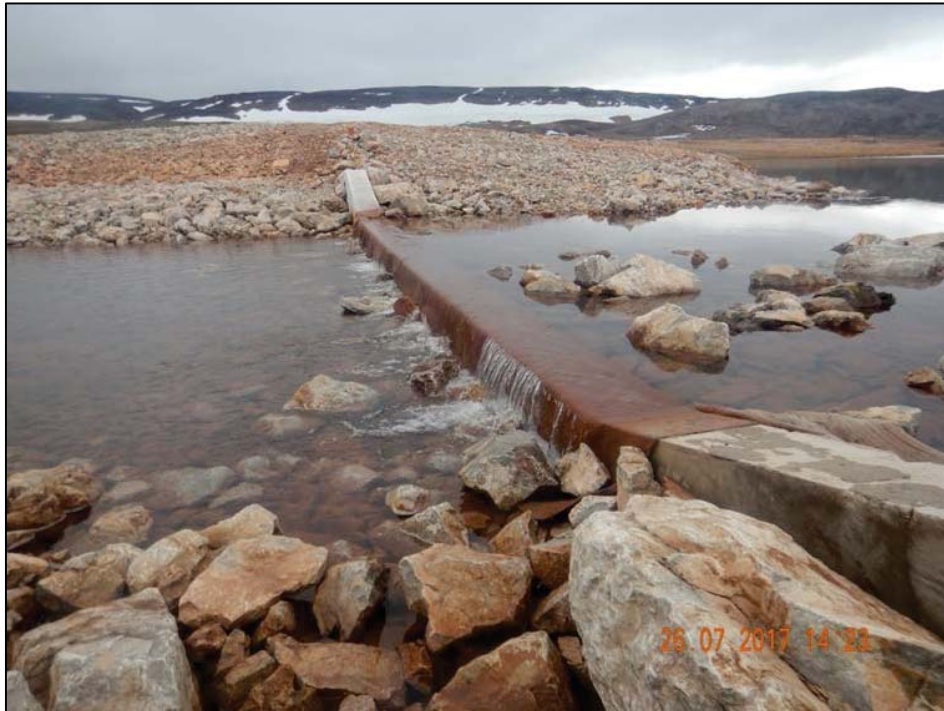
Photo 9. WT Outlet – Outlet wall. Note flow is approximately +4 cm.
