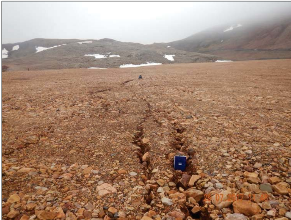
Photo 19. Surface Cell – Thermal cracking along edge of main swale.
