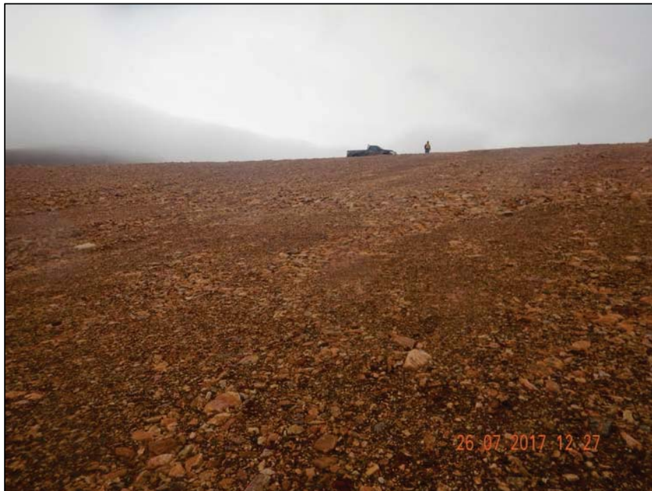
Photo 23. Surface Cell – Face of WT Dyke as seen from toe of dyke.
