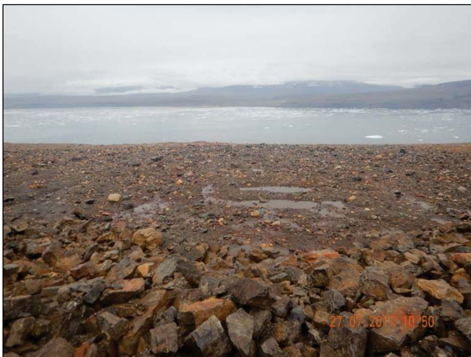
Photo 52. Oceanview Pit – Flow of water emerging from toe of cover system.
