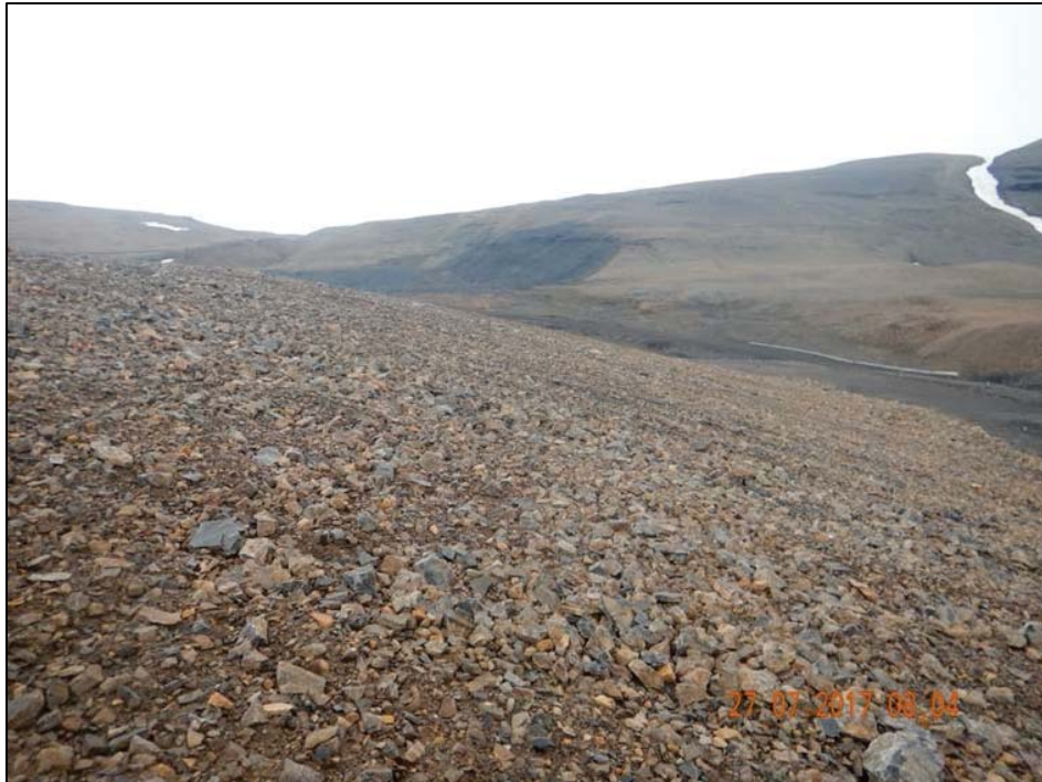
Photo 62. Industrial Complex – Sloping face of IC cover system.
