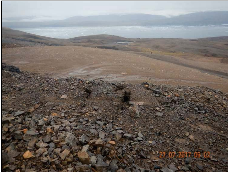
Photo 45. East Open Pit – Crack in crown pillar of EOP.
