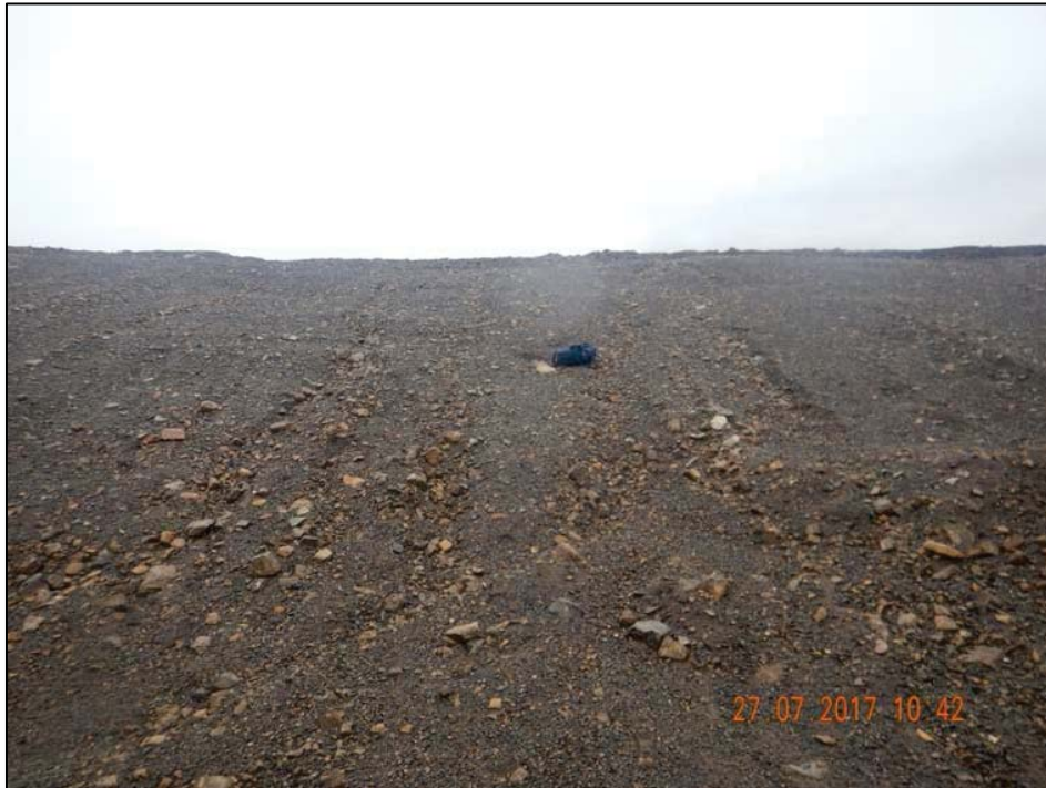
Photo 51. Oceanview Pit – Rill erosion along backslope of cover system.
