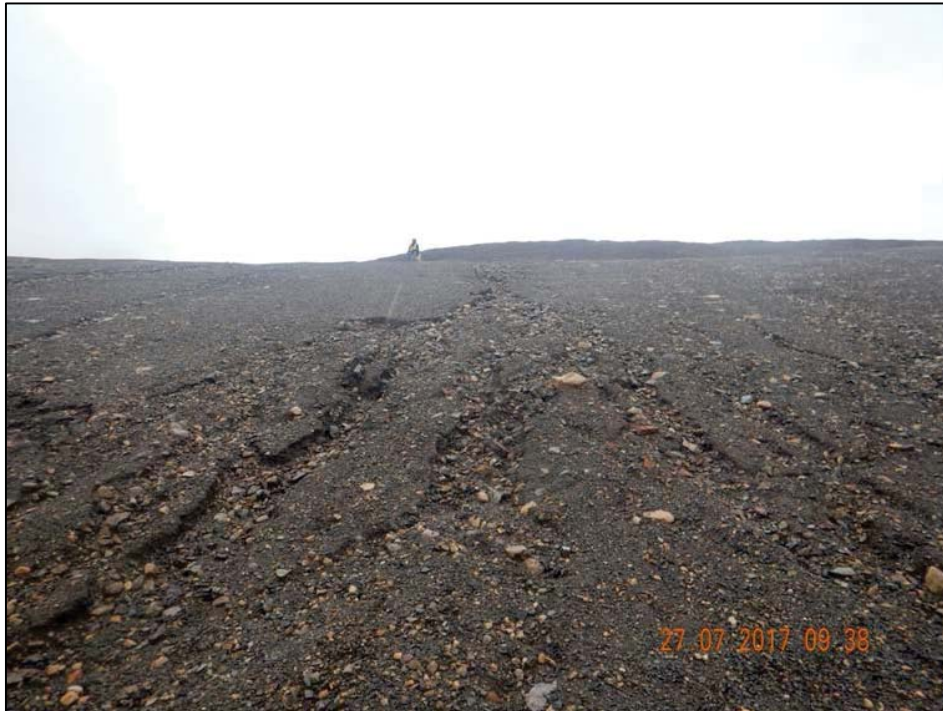
Photo 47. East Open Pit – Self armoured rill erosion channels along lower portion of EOP cover system.
