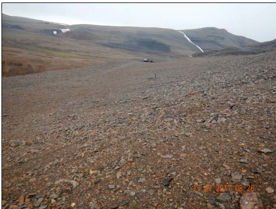
Photo 42. West Open Pit – Sloping face of WOP cover system.
