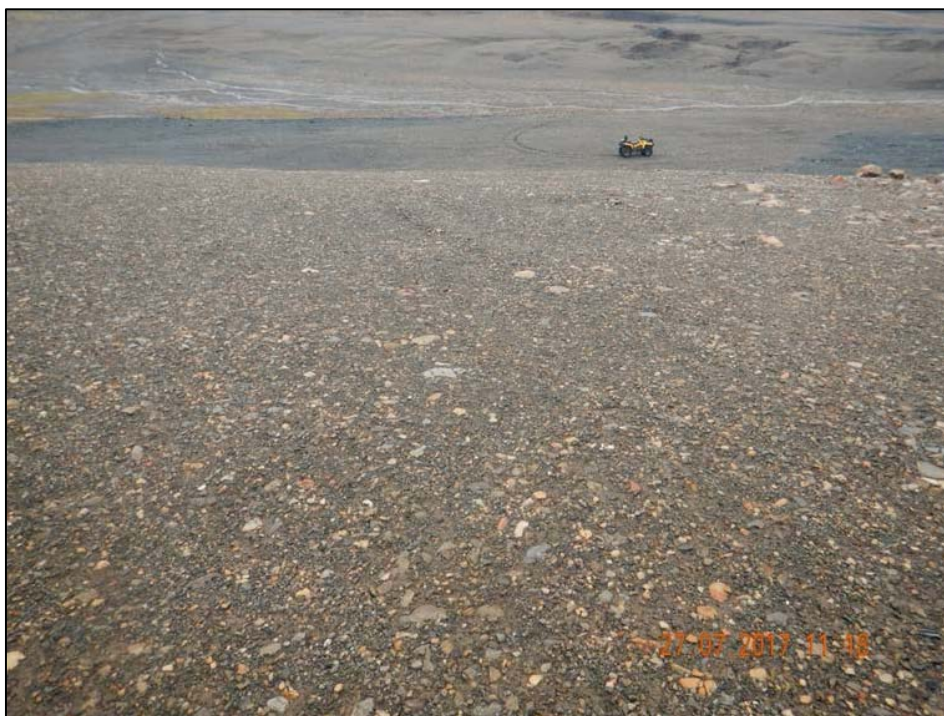
Photo 70. K-Baseline Portal – Lower sloping portion of portal plug cover.
