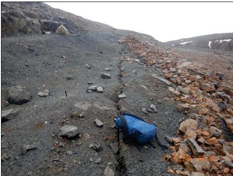
Photo 40. West Open Pit – Crack in crown pillar of WOP.
