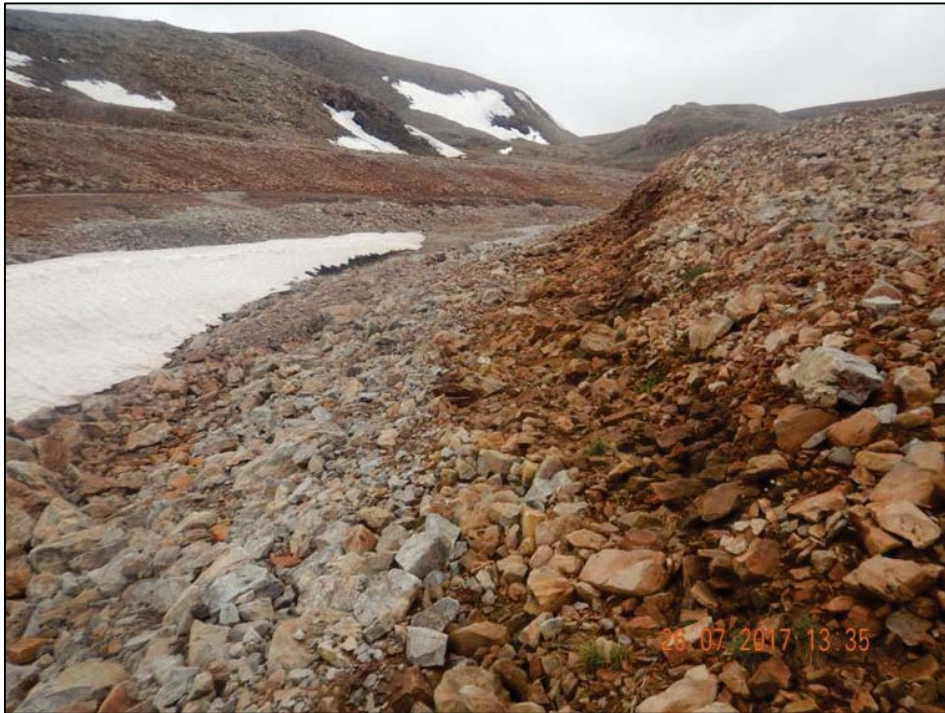
Photo 5. Spillway – Erosion along left bank of spillway. View looking upstream along left bank.
