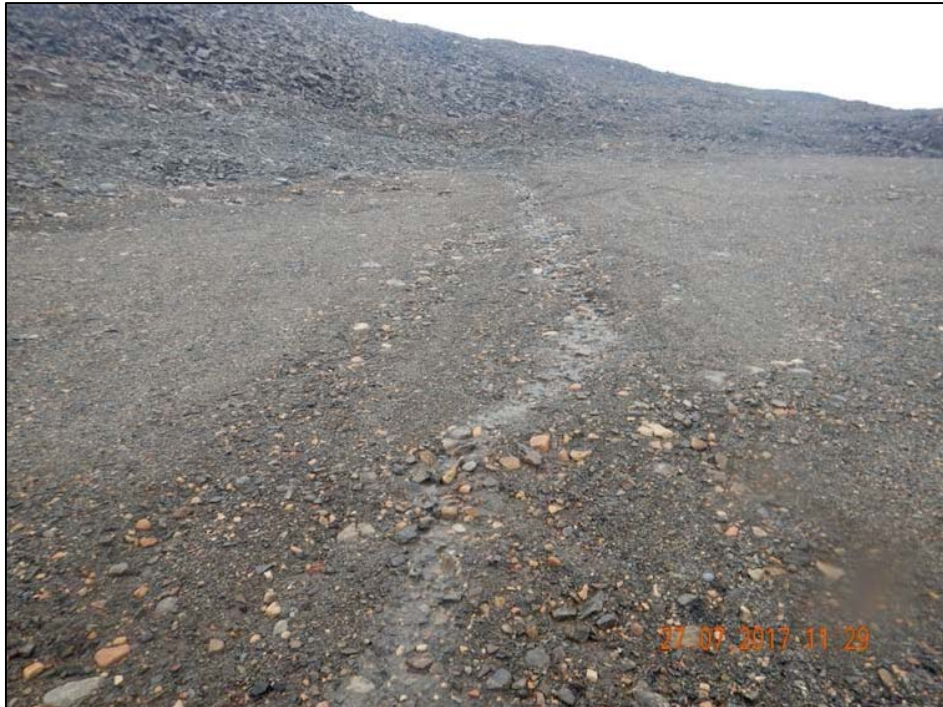
Photo 48. East Open Pit – Rill erosion on surface of cover system view looking upslope.
