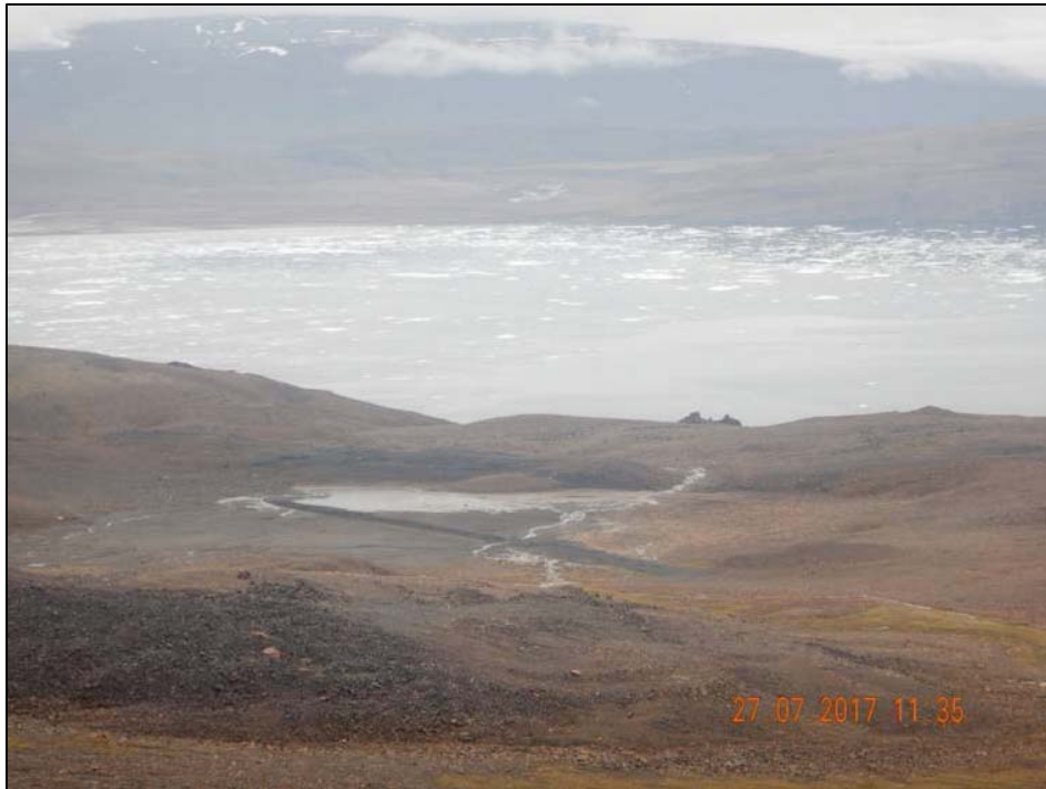
Photo 1. East Adit – Retention Pond. Note the infilling of the basin and flow through conditions.
