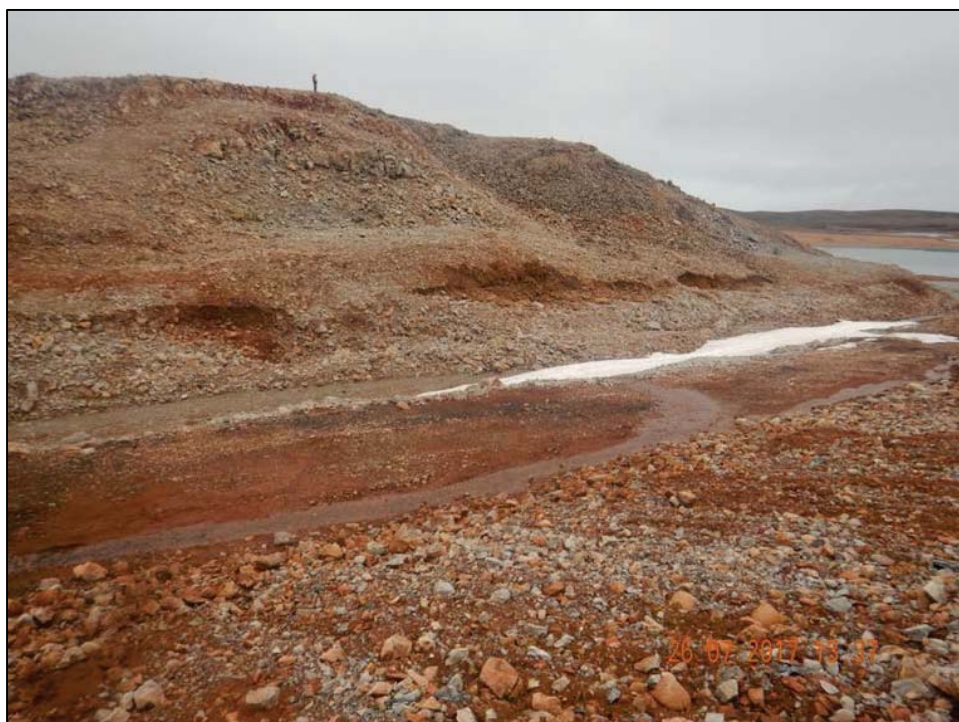
Photo 4. Spillway – View of erosion area along left bank of spillway as seen from crest of right bank.
