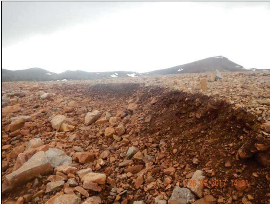
Photo 13. ETC Diversion Channel – Erosion area along left bank of diversion channel.
