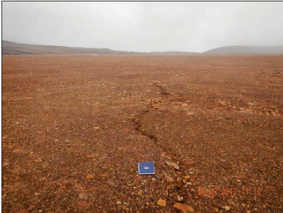
Photo 17. Surface Cell – Thermal cracking in southwest quadrant of Surface Cell cover system.
