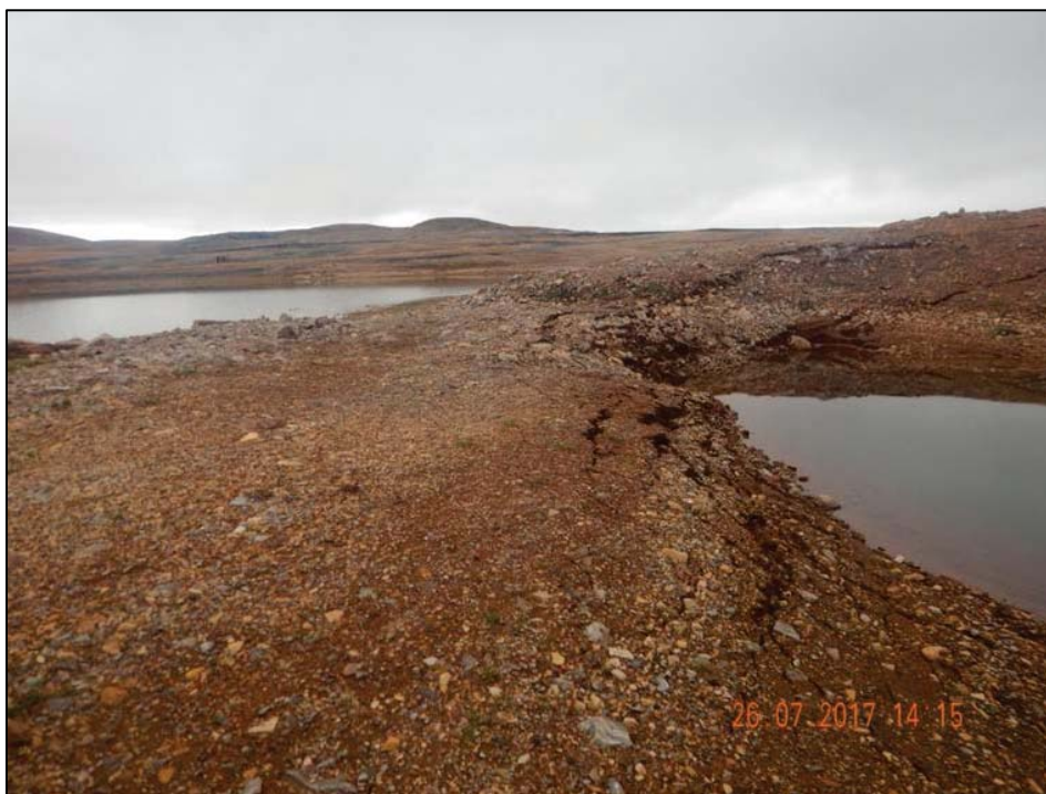
Photo 10. WT Outlet – Thermokarst/settlement area along north shoreline of remnant polishing pond.
