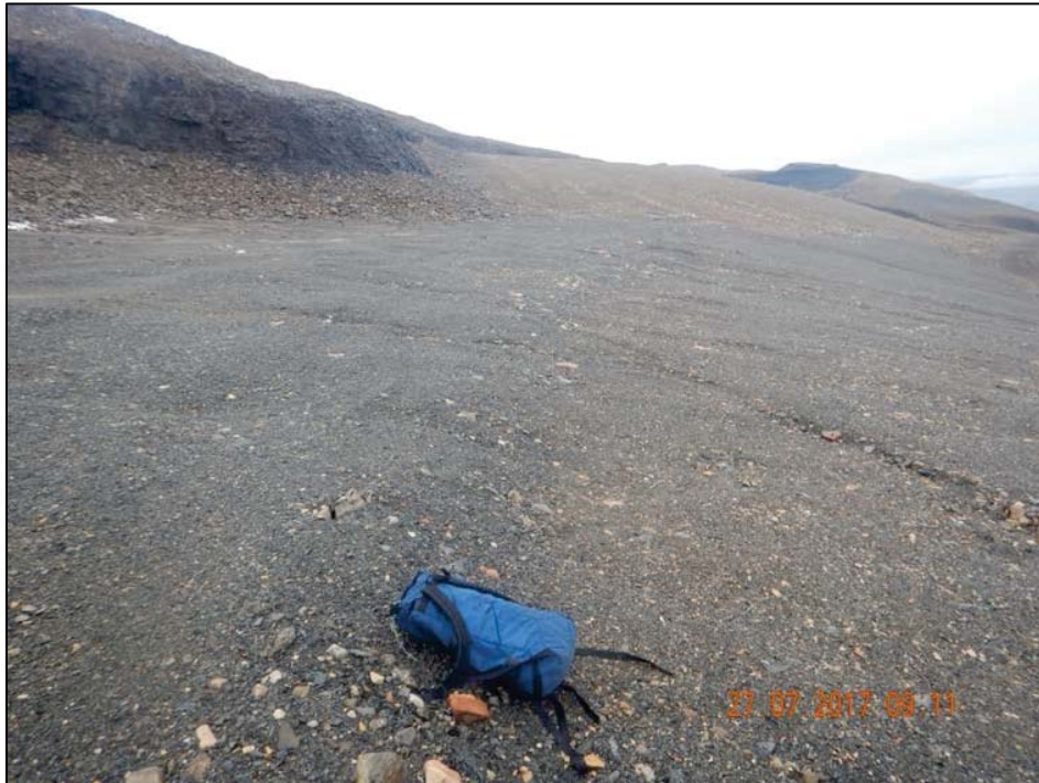
Photo 43. East Open Pit – Settlement trough along upper bench of cover system.
