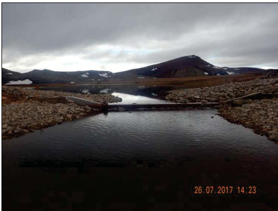
Photo 8. WT Outlet – Outlet wall. Note flow is approximately +4 cm.
