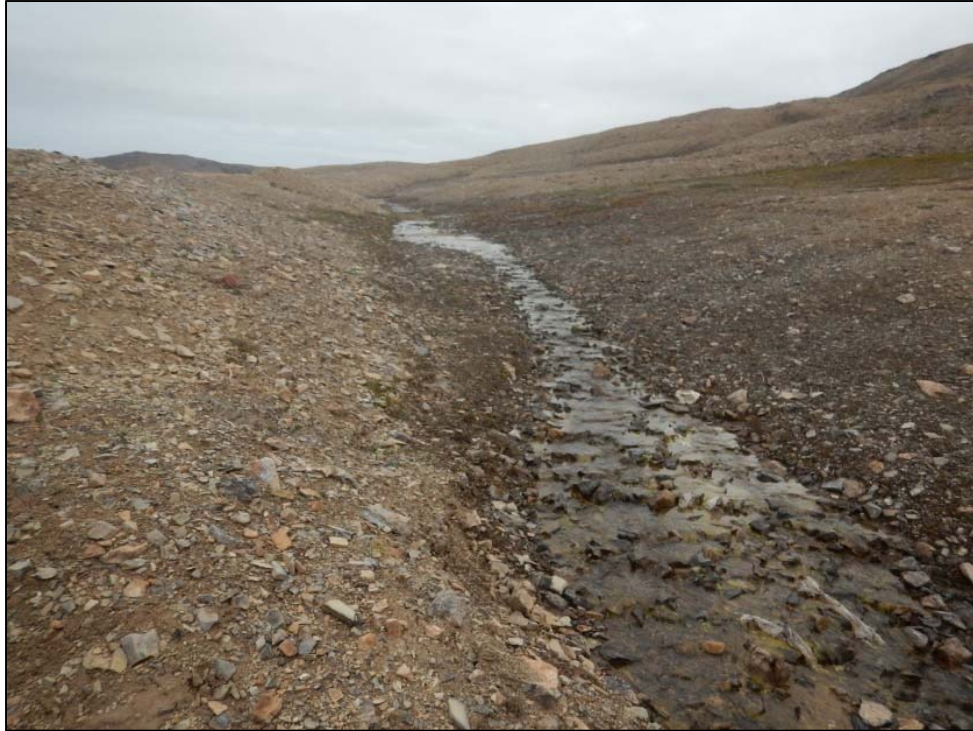
Photo 41. Landfill – Diversion berm upstream of the landfill.
