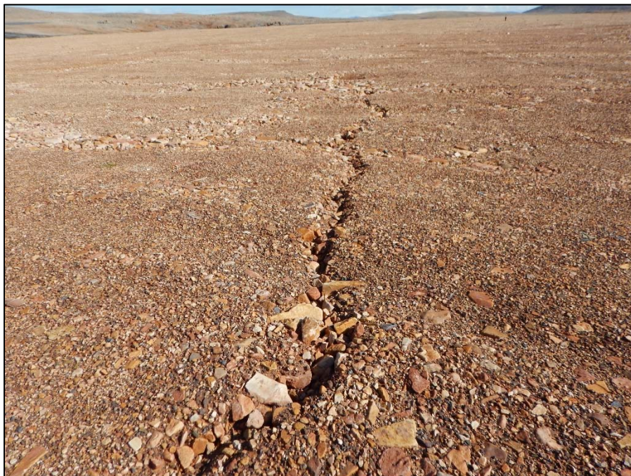
Photo 22. Surface Cell Cover System – Thermal cracking in the southwest quadrant of the Surface Cell cover system.
