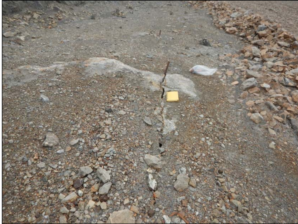
Photo 45. West Open Pit – Crack behind remnant highwall.
