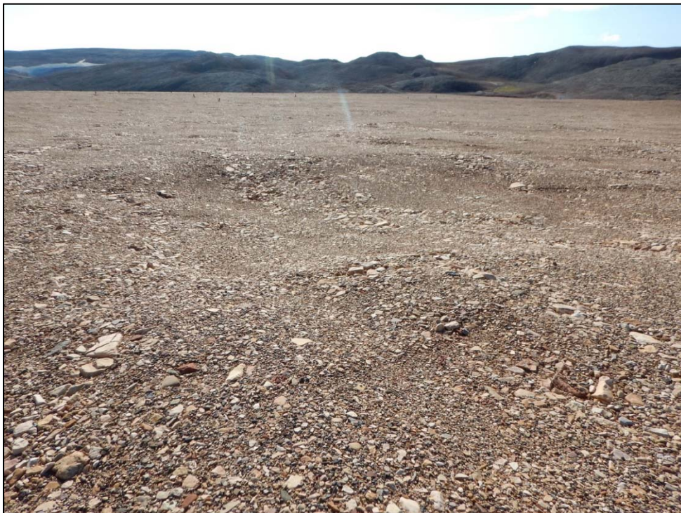
Photo 18. Surface Cell Cover System – Minor thermokarsting along main E-W drainage swale.
