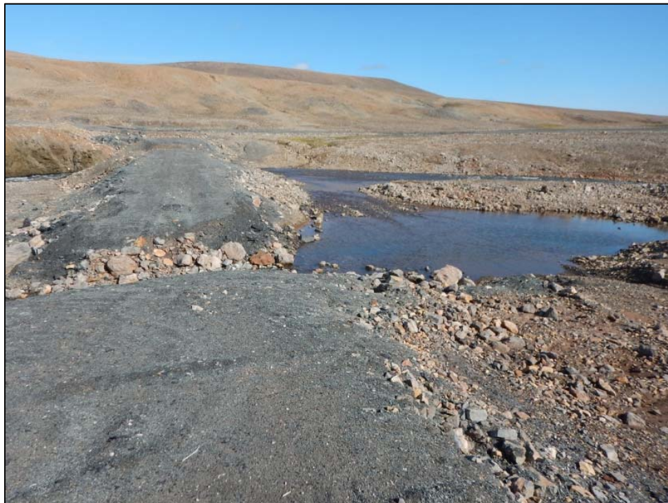
Photo 62. Upper Dump Pond – Breach in road to mill site.
