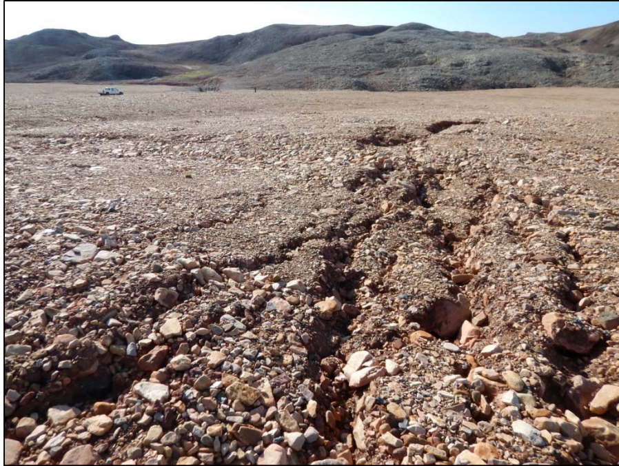
Photo 21. Surface Cell Cover System – Thermal cracking along the edge of the main swale.
