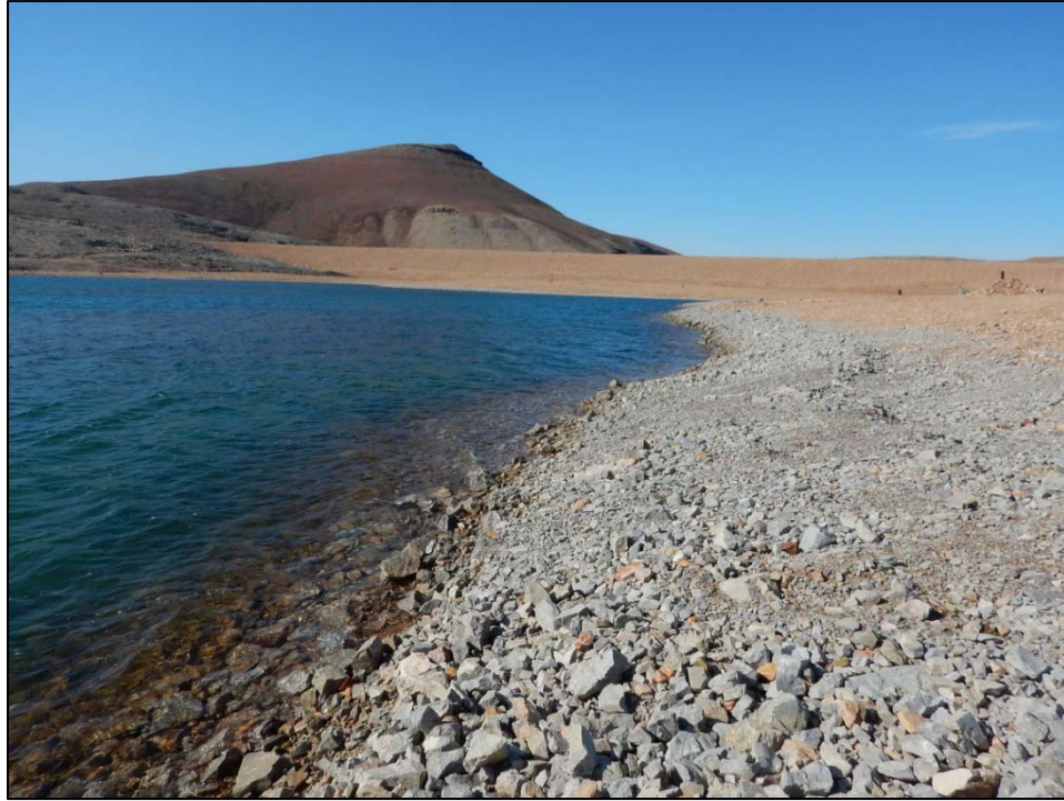
Photo 33. Test Cell Cover System – Erosion protection along the East Arm of the Test Cell Dyke, view looking northwest.
