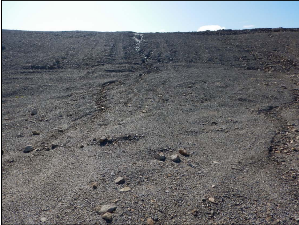
Photo 55. Oceanview Pit – Rilling on the south end of the cover system.
