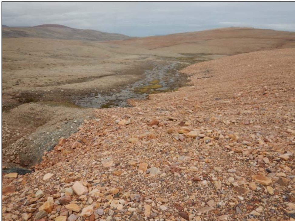
Photo 40. Landfill – Diverted water flowing around north side of cover system.
