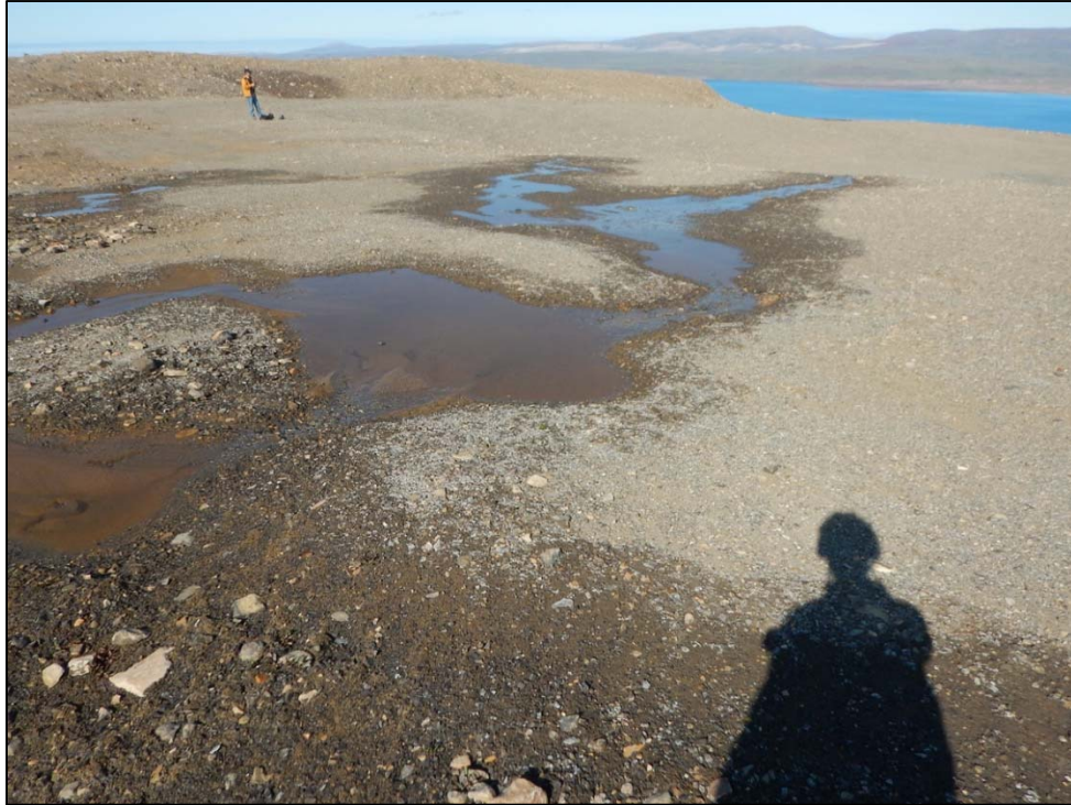
Photo 59. Oceanview Pit – Seepage flowing into the cover system from upstream.
