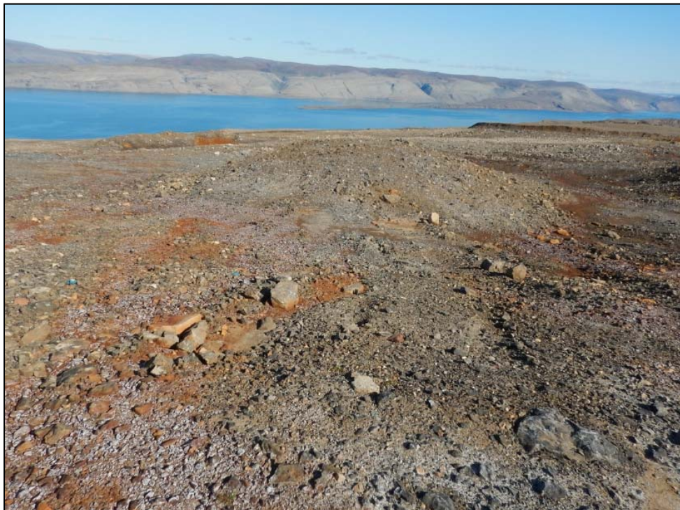
Photo 72. Oceanview East Raise – ARD staining around the plug and mound.
