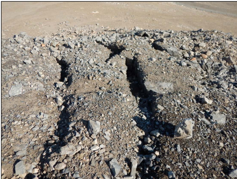
Photo 48. East Open Pit – Cracking in crown pillar.
