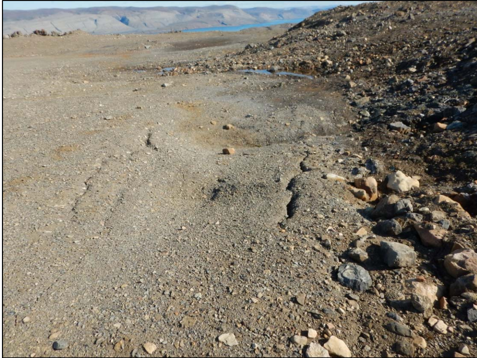
Photo 57. Oceanview Pit – Minor thermal cracking on south end of the cover.
