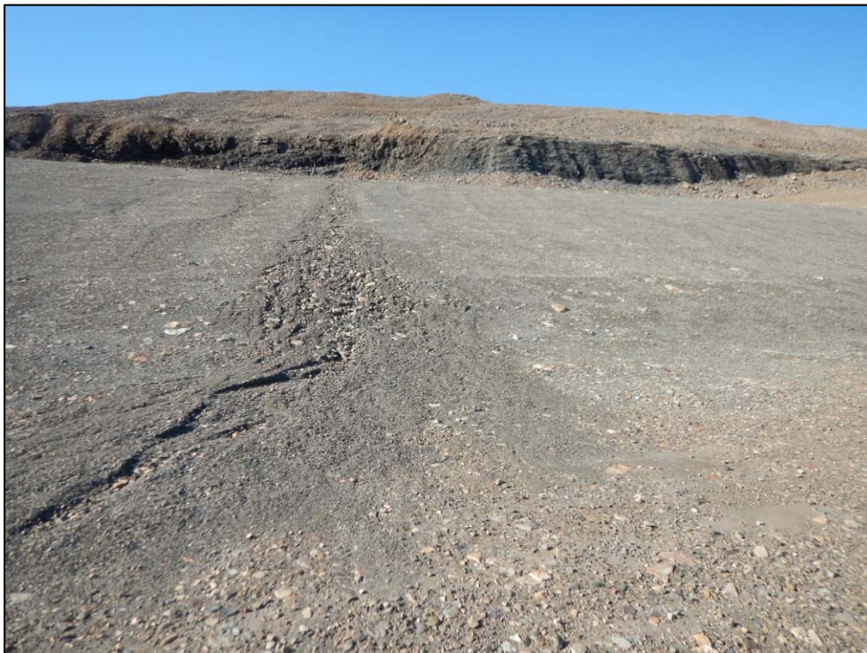
Photo 50. East Open Pit – Looking upslope at rilling on cover system. Note self-armouring.
