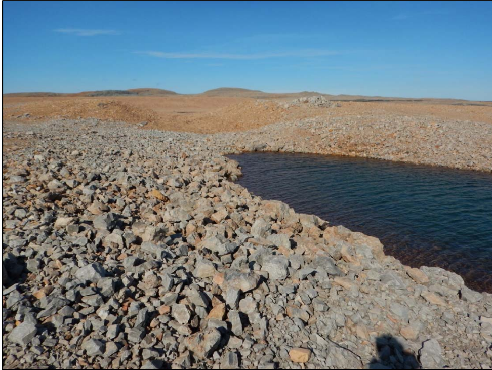
Photo 35. Test Cell Cover System – Outlet of breach in Test Cell Dyke.
