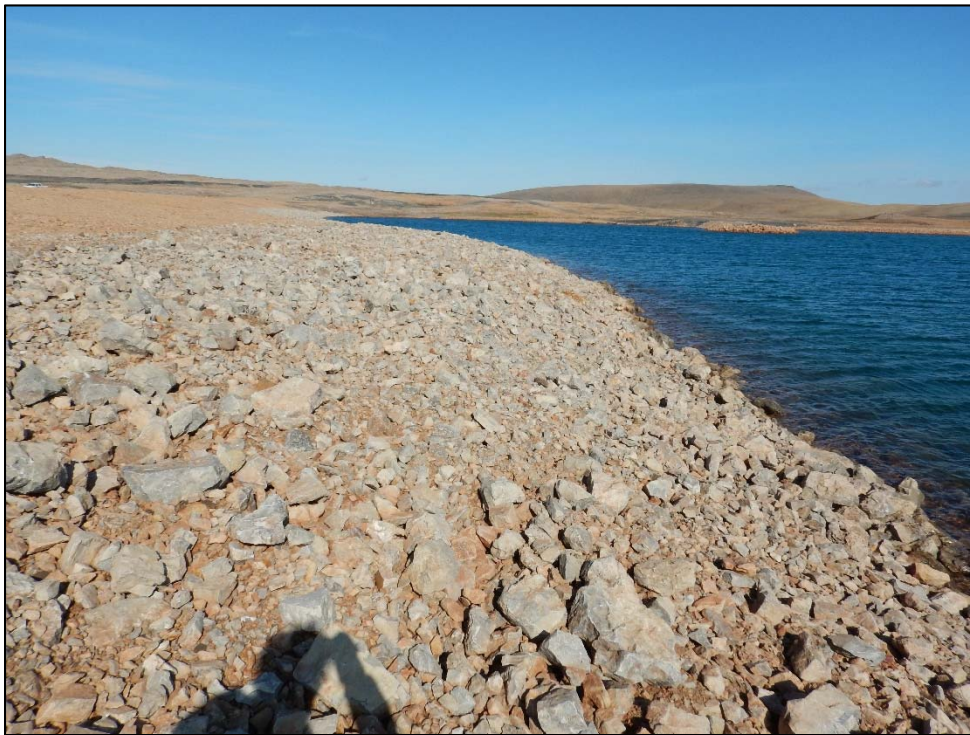
Photo 34. Test Cell Cover System – Erosion protection along the N/S arm of the Test Cell Dyke, view looking north.
