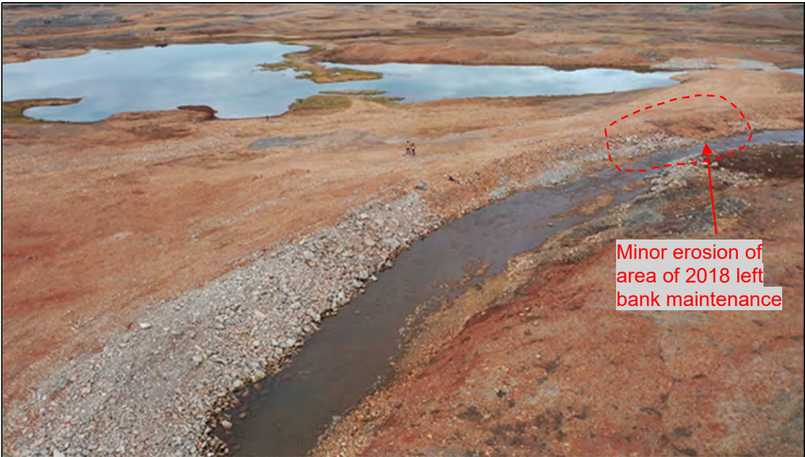
Photo 15. East Twin Creek Diversion – Overview, looking downstream from UAV. Note minor erosion near upper right.
