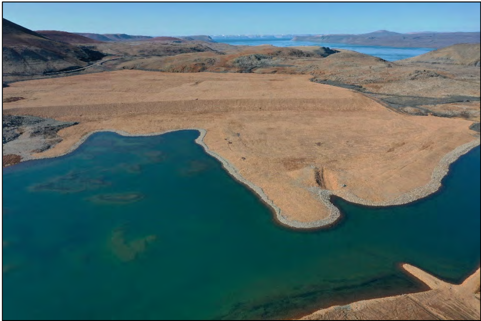
Photo 36. Test Cell Cover System – UAV overview of erosion protection along the toe of the Test Cell Dyke, view looking north.
