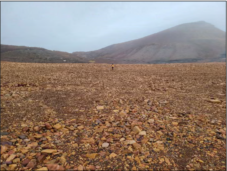
Photo 19. Surface Cell Cover System – Minor thermokarsting along main E-W drainage swale.
