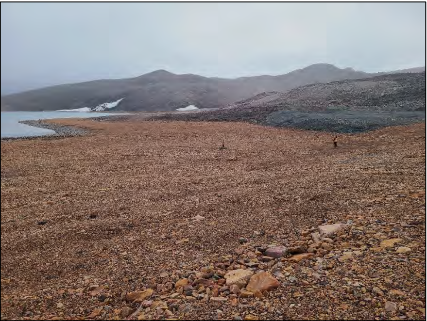
Photo 38. Toe of West Twin Dyke Tailings Cover – Note minor thermokarsting.
