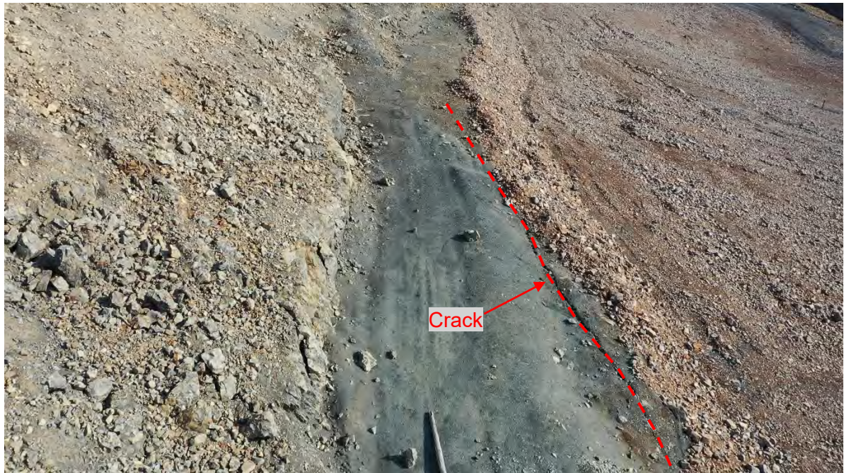
Photo 45. West Open Pit – Crack behind remnant highwall, as seen from above.
