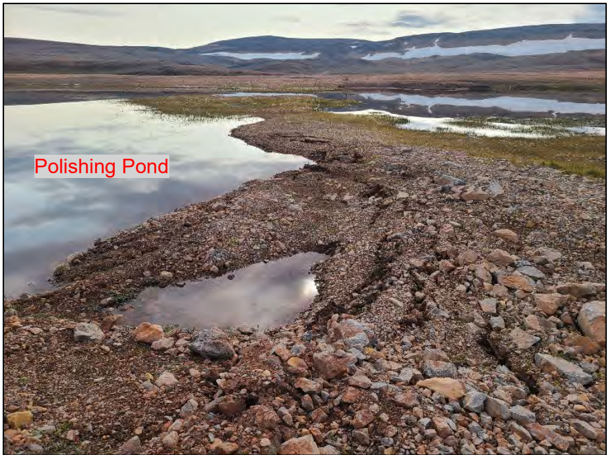
Photo 14. Polishing Pond – Thermokarsting around Polishing Pond.
