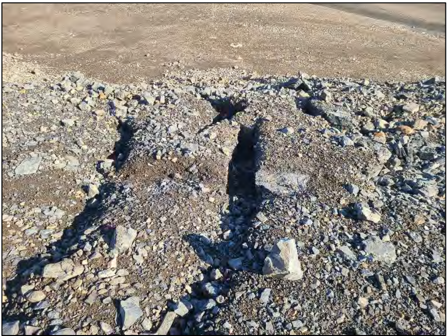
Photo 51. East Open Pit – Cracking in crown pillar.
