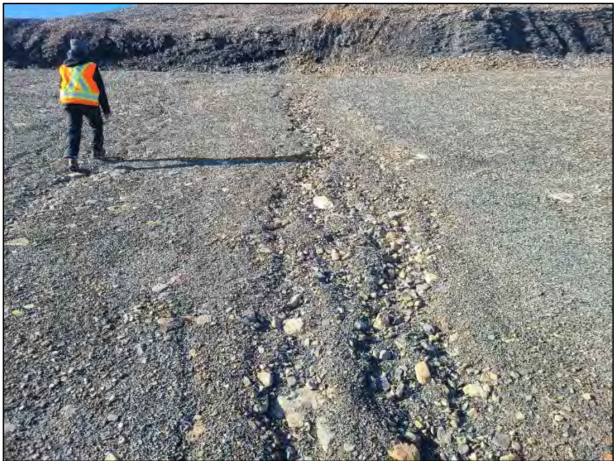
Photo 49. East Open Pit - Looking upslope at rilling on upper portion of cover. Note self-armouring.
