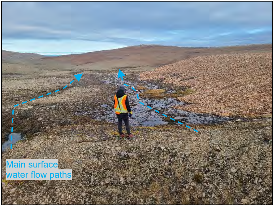
Photo 41. Landfill – Diverted water flowing around north side of cover system.
