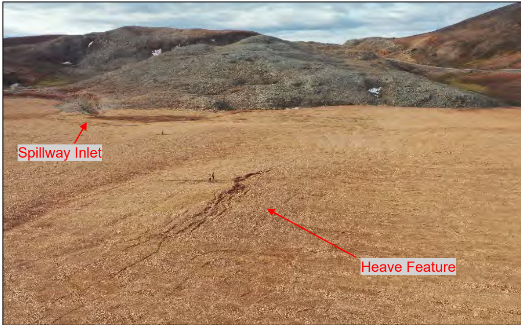
Photo 21. Surface Cell Cover System – Heave feature in the southwest quadrant of the Surface Cell cover system, as seen looking Southwest
