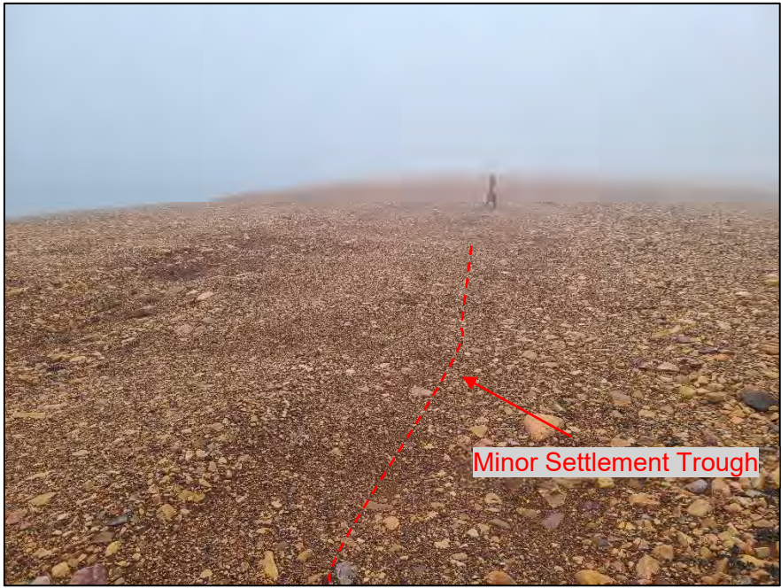
Photo 29. Test Cell Cover System – Minor settlement trough along N/S arm of Test Cell Dyke.
