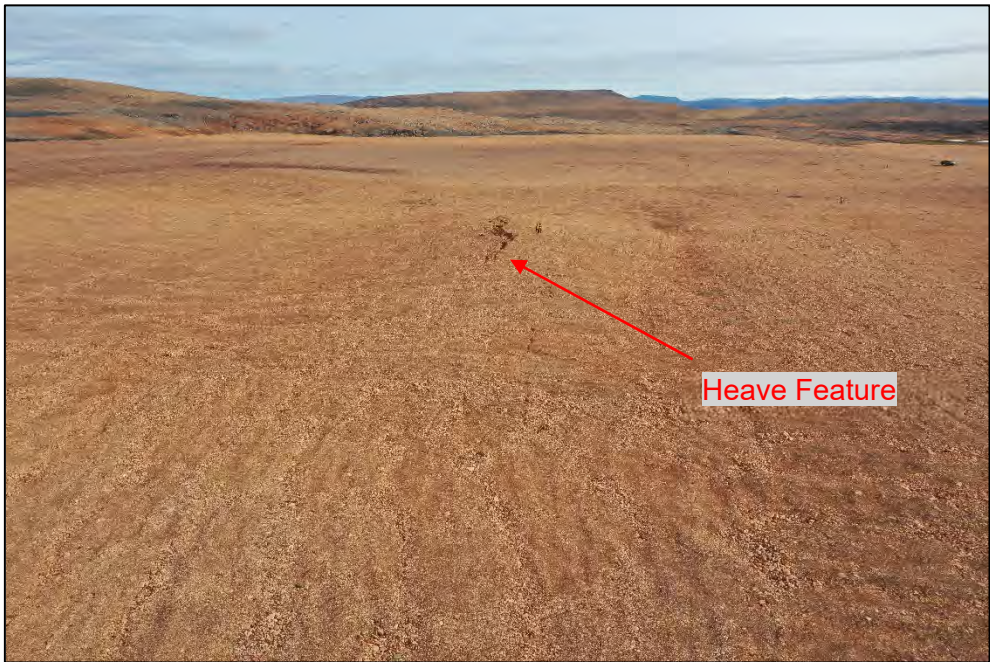
Photo 22. Surface Cell Cover System – Heave feature in the southwest quadrant of the Surface Cell cover system, as seen looking Northeast from UAV.
