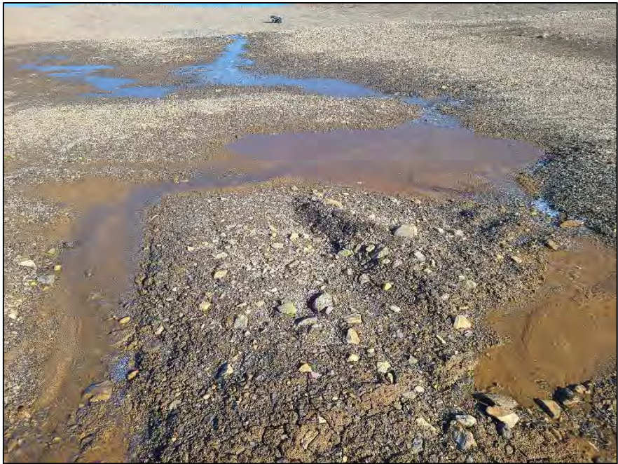
Photo 56. Oceanview Pit – Minor seepage flowing into the cover system from upslope, as seen from the ground.
