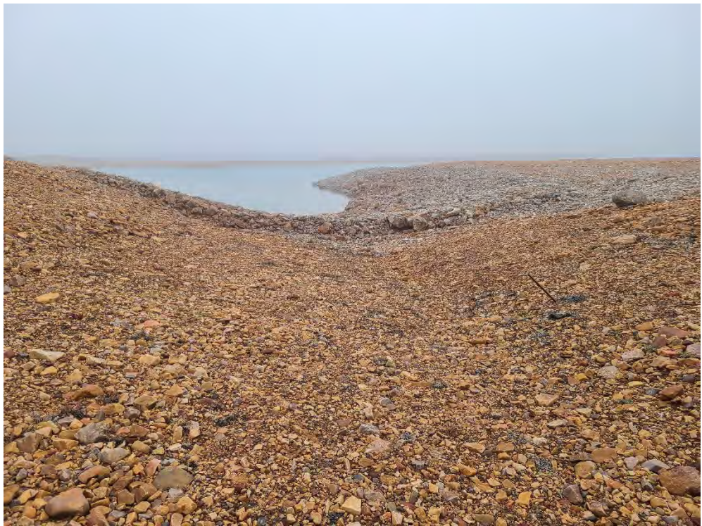
Photo 34. Test Cell Cover System – Outlet of breach in Test Cell Dyke.
