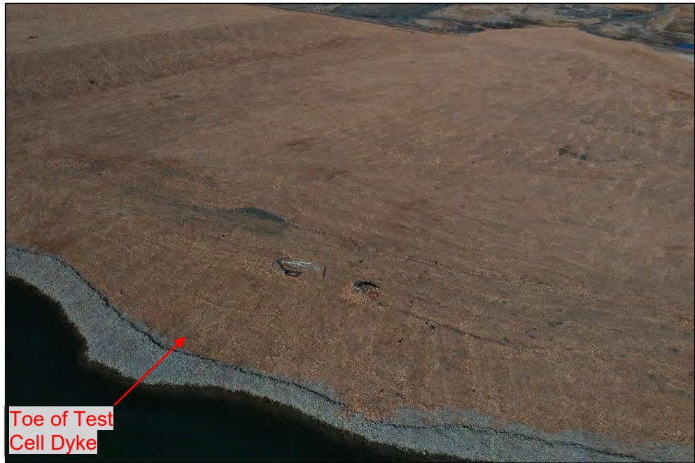
Photo 33. Test Cell Cover System – Toe of the test cell dyke.
