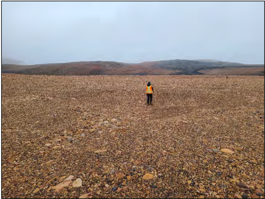
Photo 18. Surface Cell Cover System – Minor thermokarsting along main N-S drainage swale.
