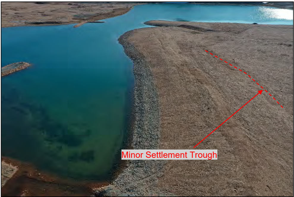
Photo 30. Test Cell Cover System – N/S arm of Test Cell Dyke, as seen from UAV. Note minor settlement trough.
