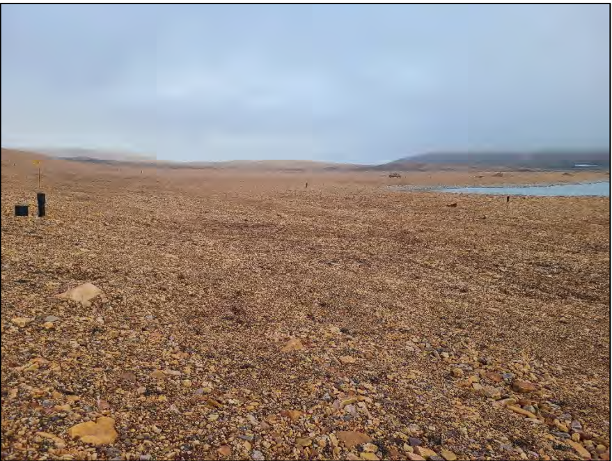
Photo 39. Toe of West Twin Dyke Tailings Cover – Note minor thermokarsting.
