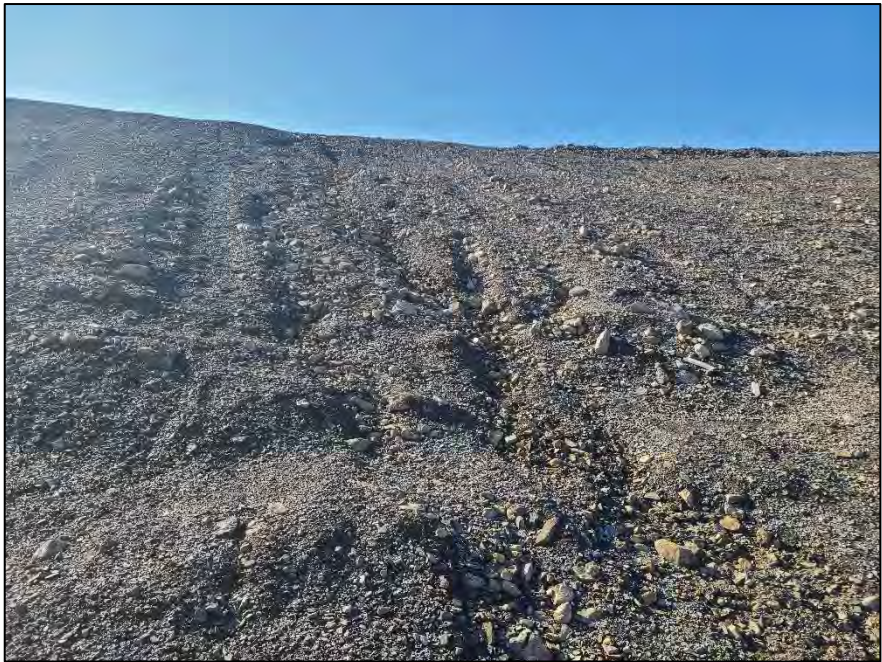
Photo 55. Oceanview Pit – Rilling on the south end of the cover system. Note self-armouring.
