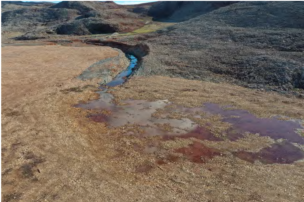
Photo 3. West Twin Dyke Spillway – Small headpond at spillway inlet as seen from UAV.
