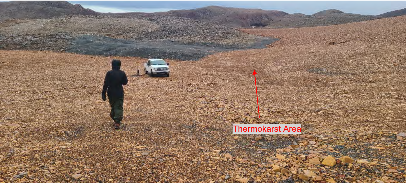
Photo 40. Toe of West Twin Dyke Tailings Cover – Note minor thermokarsting, looking south.
