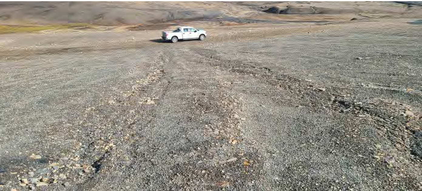
Photo 52. East Open Pit - Looking downslope at rilling on upper portion of cover. Note self-armouring.
