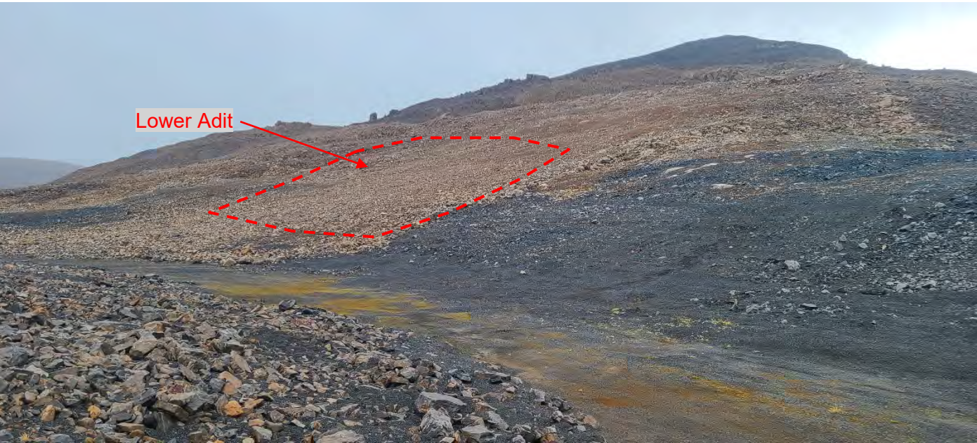
Photo 71. Lower Adit – Sloping face of cover system as seen from UAV.
