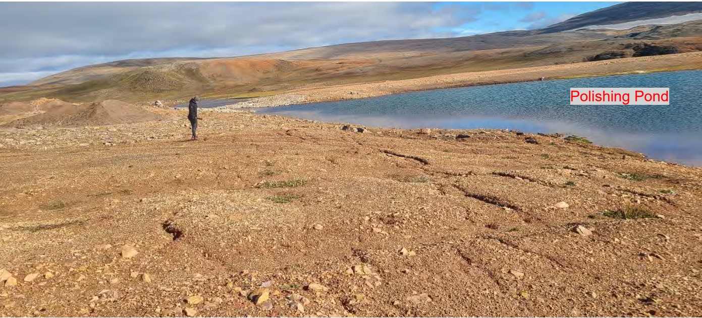
Photo 13. Polishing Pond – Thermokarst cracking along the north side of the Polishing Pond.
