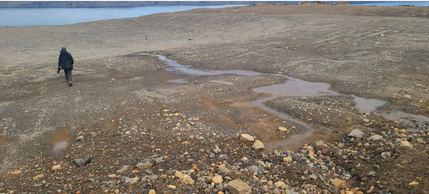
Photo 59. Oceanview Pit – Minor seepage flowing onto the cover system from upslope, as seen from the ground.
