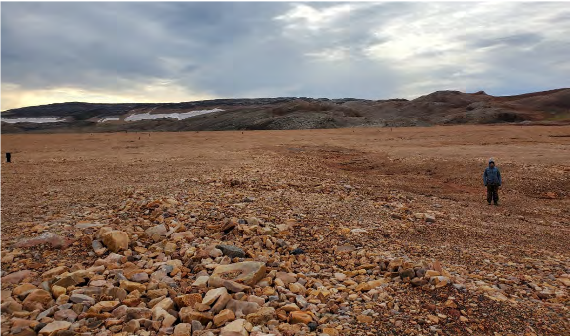
Photo 18. Surface Cell Cover System – Minor thermokarsting along main E-W drainage swale.
