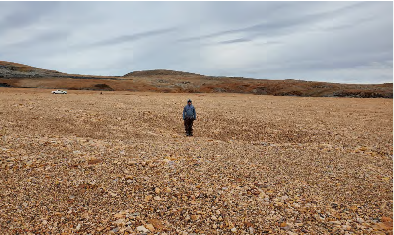
Photo 17. Surface Cell Cover System – Minor thermokarsting along main N-S drainage swale.
