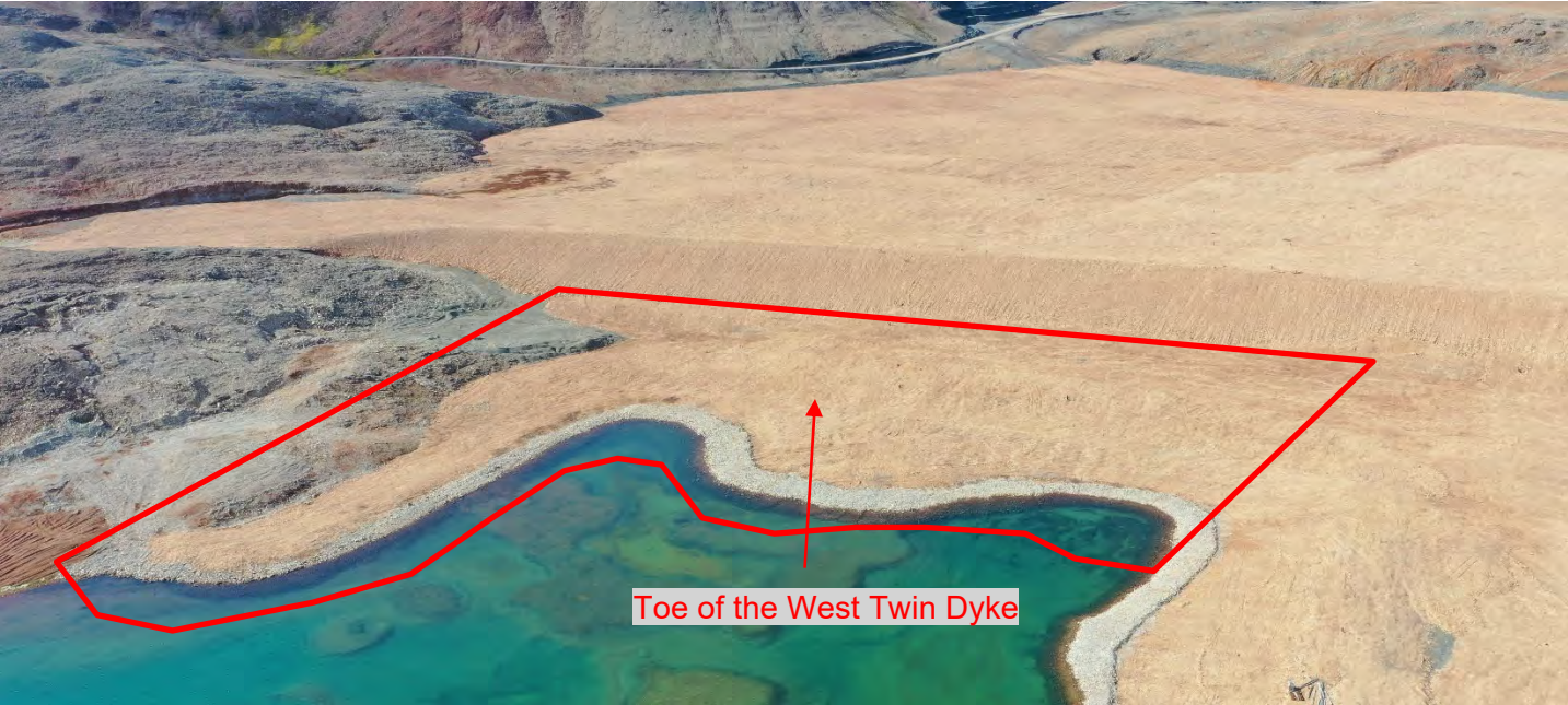
Photo 39. Toe of West Twin Dyke Tailings Cover – Overview as seen from UAV.
