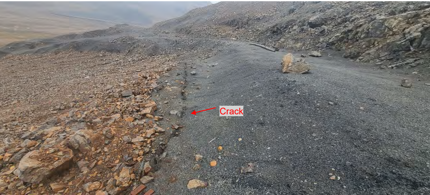
Photo 48. West Open Pit – Crack behind remnant highwall.
