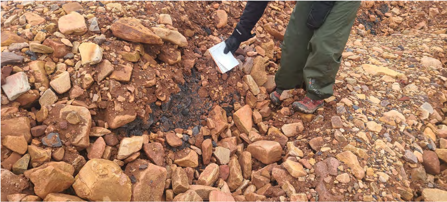
Photo 23. Surface Cell Cover System – Exposed shale within the cracking at the crest of the heave feature (0.3 m in thickness).
