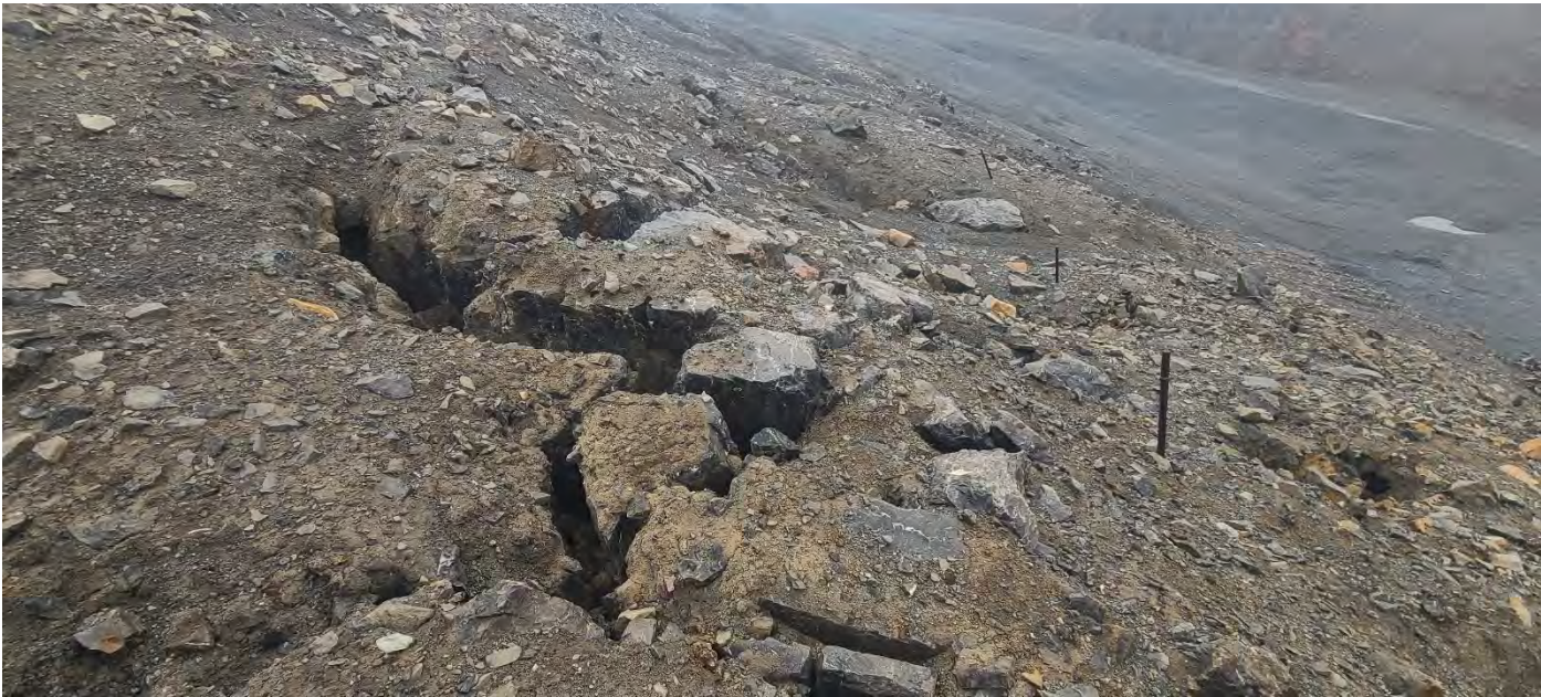
Photo 49. West Open Pit – Tension cracking and deformation adjacent to the east of the edge of the West Open Pit cover system.
