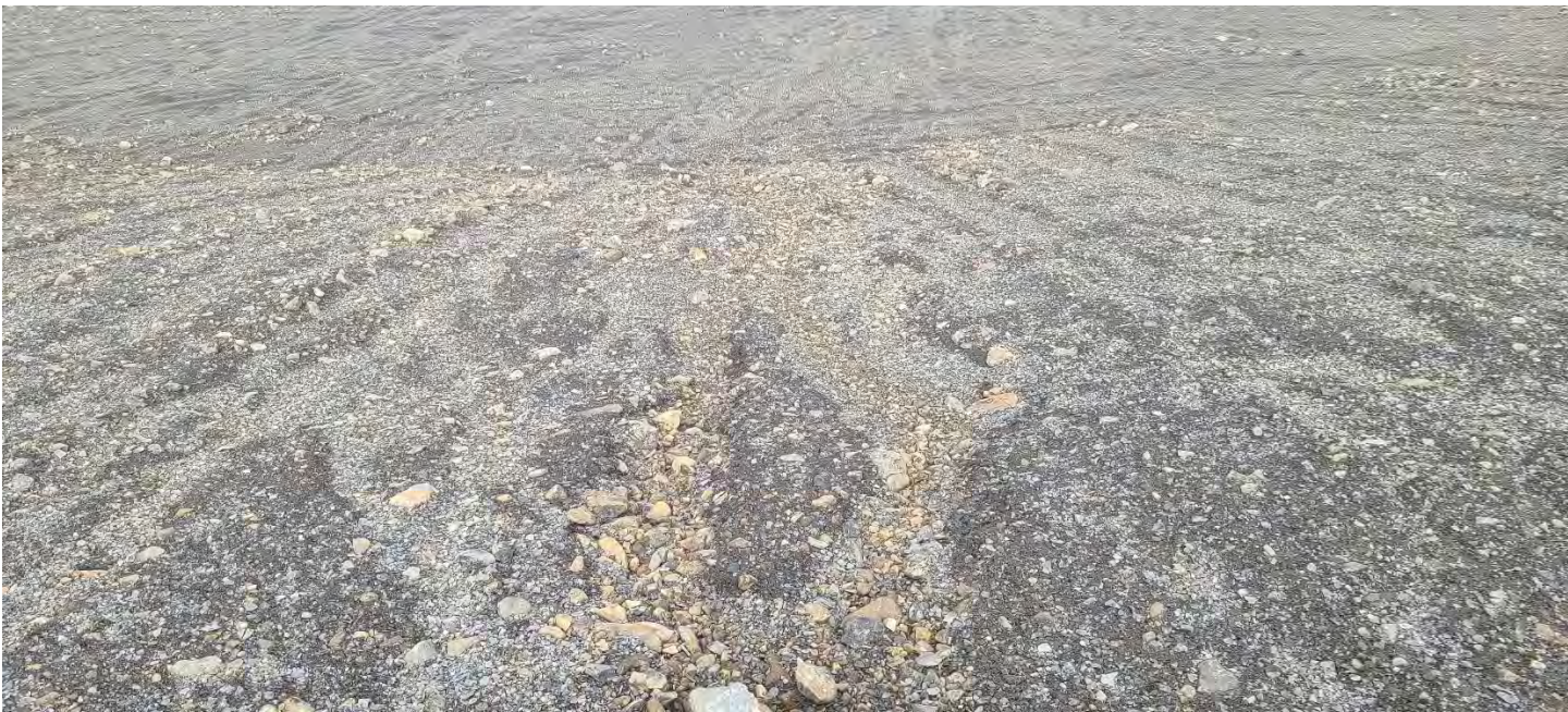
Photo 58. Oceanview Pit – Rilling on the south end of the cover system. Note self-armouring.
