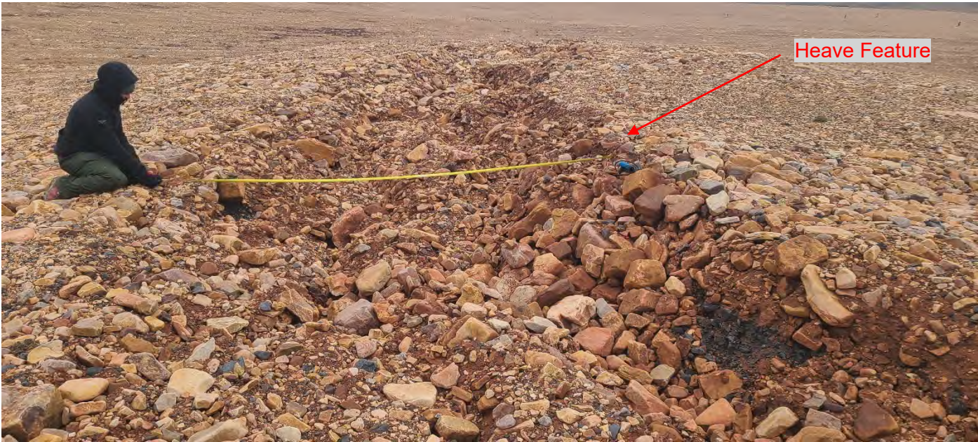
Photo 22. Surface Cell Cover System – Maximum crack width at the crest of the heave feature (2.8 m wide, 0.6 m deep).
