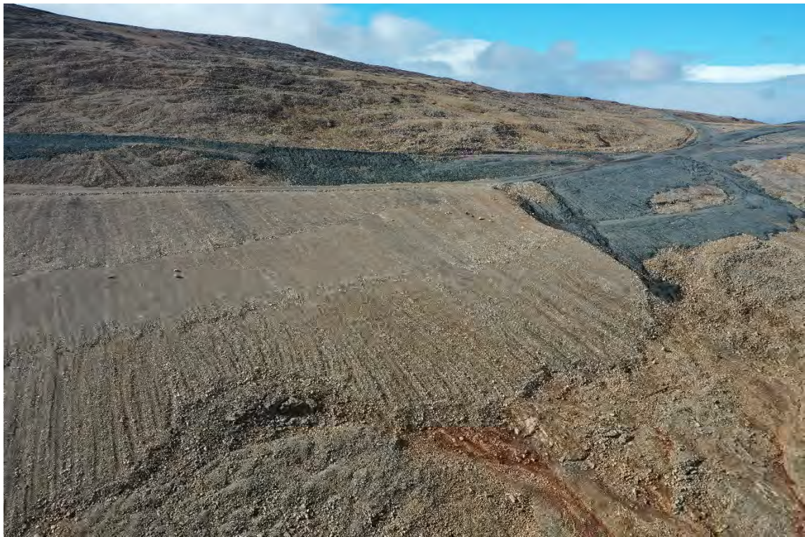
Photo 56. East Open Pit – Overview of western portion of the cover system, as seen from UAV.
