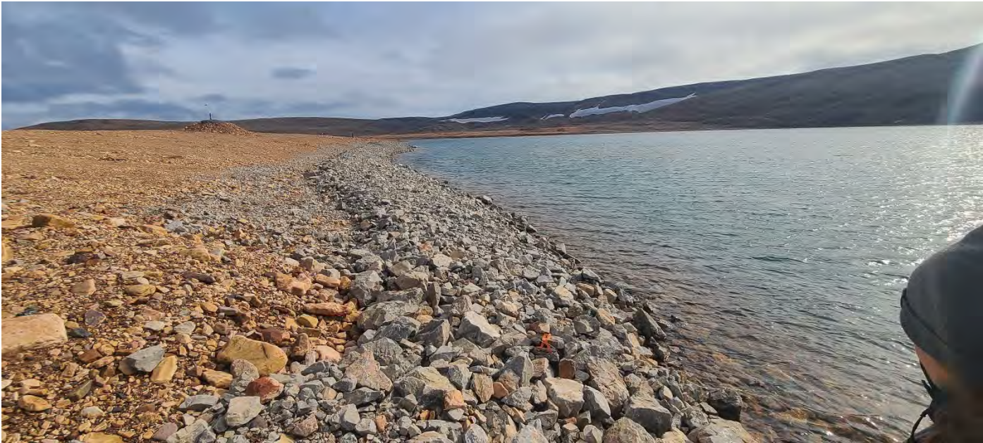
Photo 36. Test Cell Cover System – Erosion protection along the toe of the Test Cell Dyke, view looking East.
