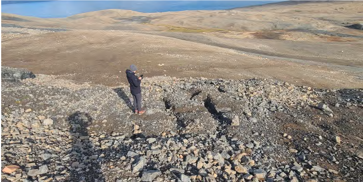
Photo 54. East Open Pit – Cracking in crown pillar.
