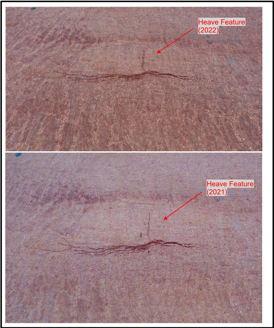
Photo 21. Surface Cell Cover System – Heave feature in 2022 (above) and 2021 (below), looking northeast.
