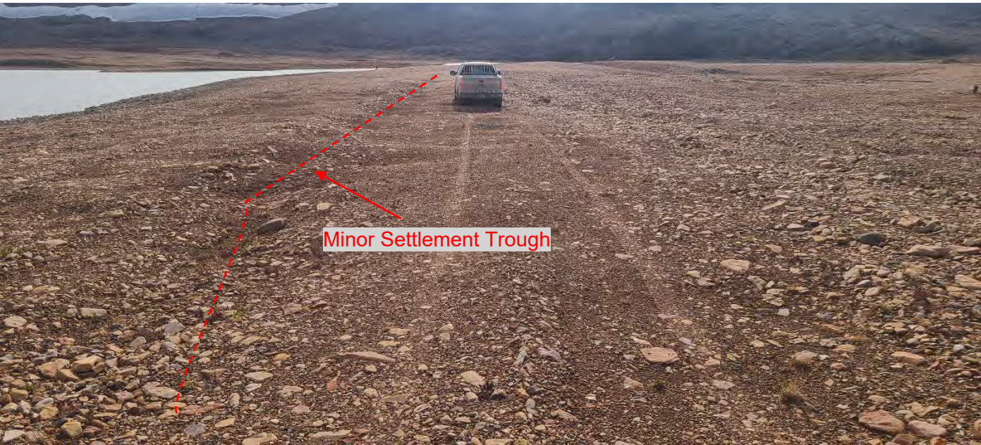
Photo 30. Test Cell Cover System – Minor settlement trough along N/S arm of Test Cell Dyke.
