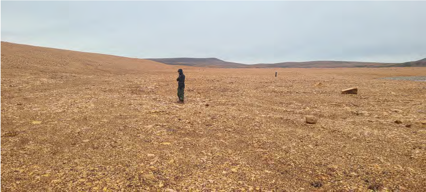
Photo 41. Toe of West Twin Dyke Tailings Cover – Note minor thermokarsting, looking North.
