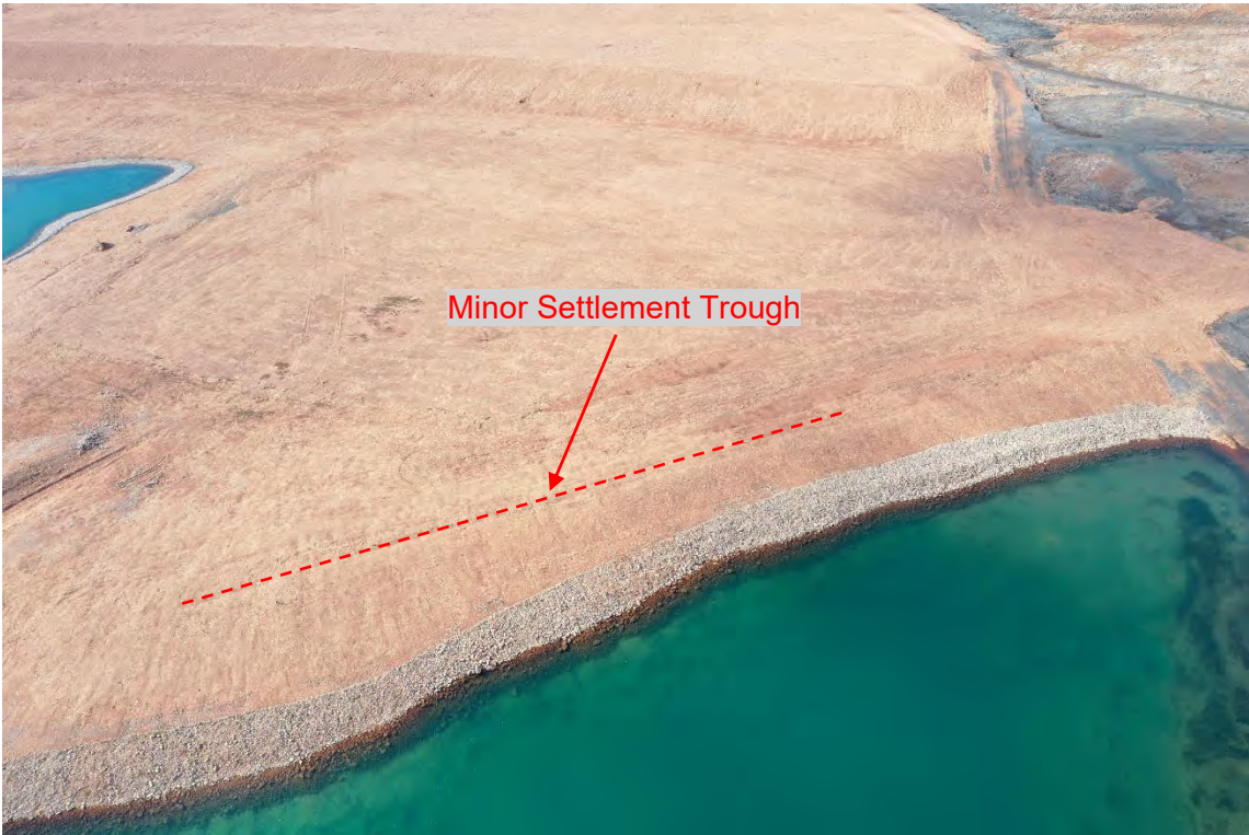
Photo 31. Test Cell Cover System – N/S arm of Test Cell Dyke, as seen from UAV. Note minor settlement trough.
