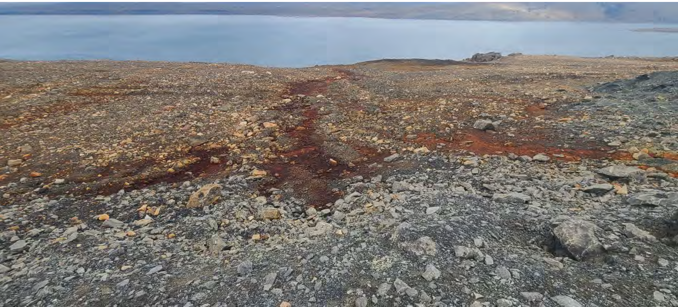
Photo 60. Oceanview Pit – Staining at toe of cover. No seepage was observed during the inspection.
