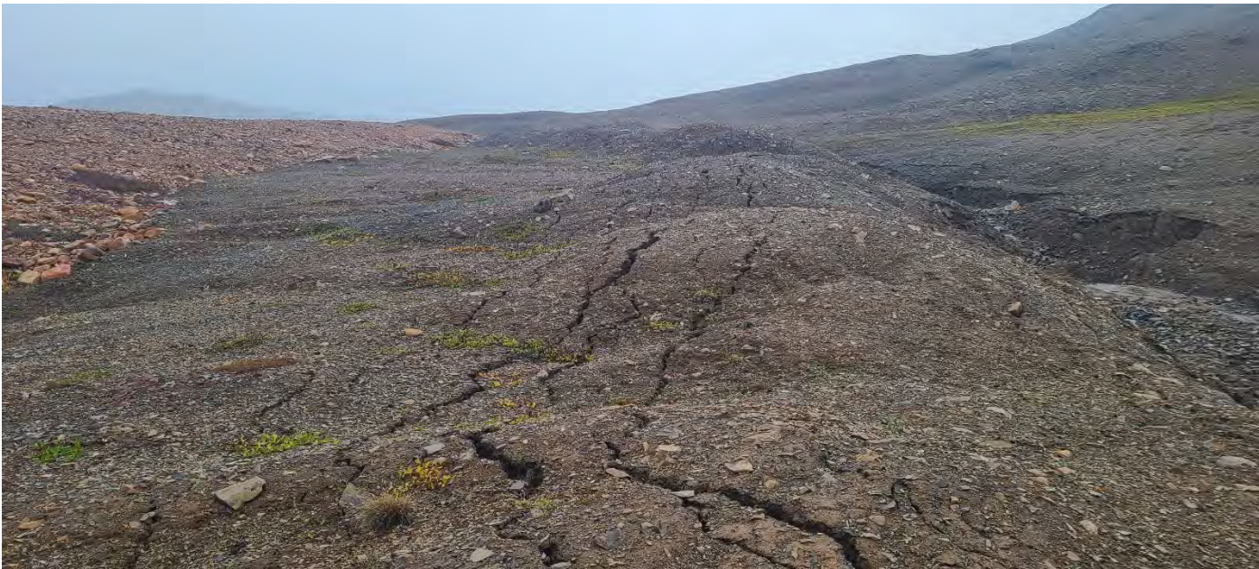
Photo 46. Landfill – Thermokarst cracking encroaching on the southwest corner of the cover system.
