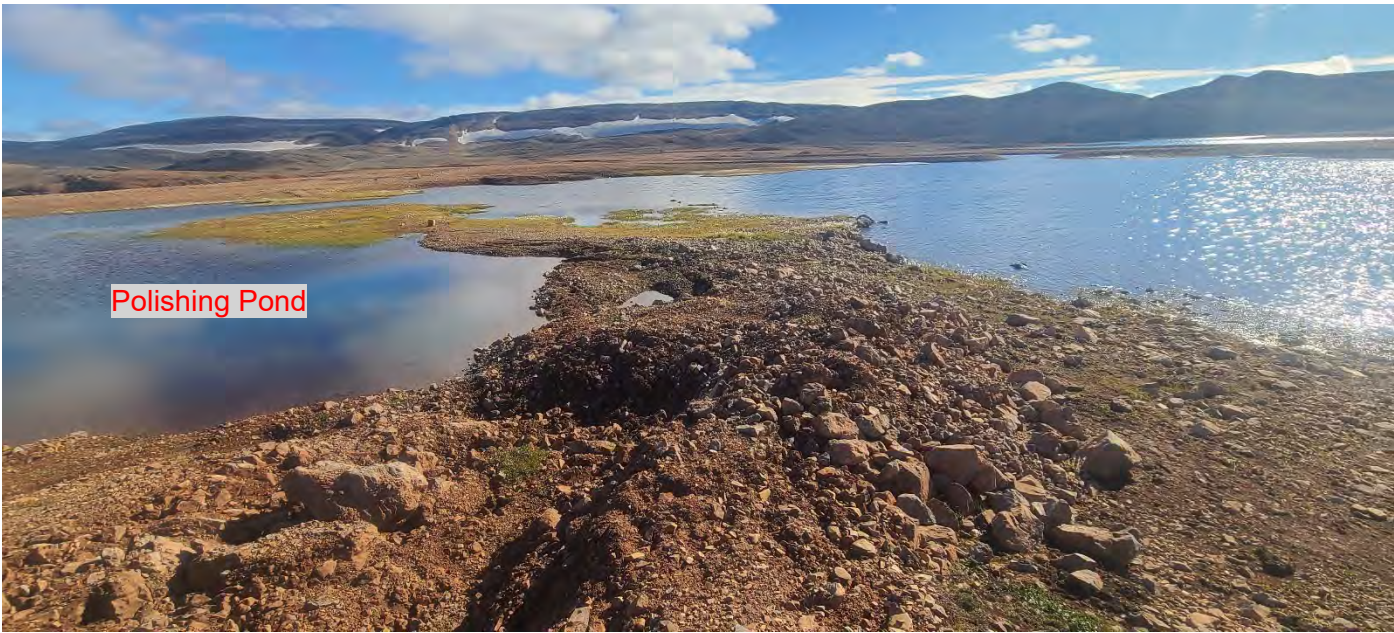
Photo 12. Polishing Pond – Thermokarsting around Polishing Pond, looking south.
