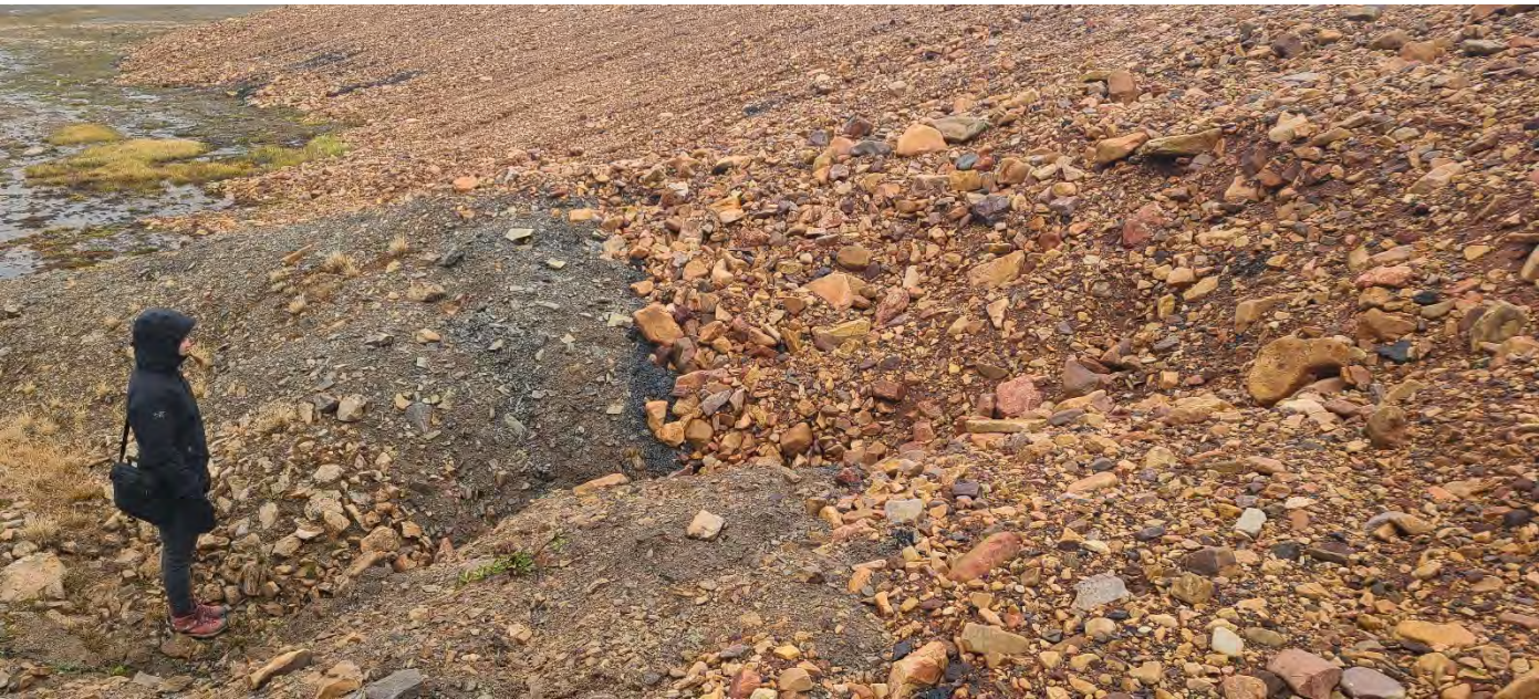
Photo 44. Landfill – Thermokarst encroaching on the southwest corner of the cover system. View looking north.
