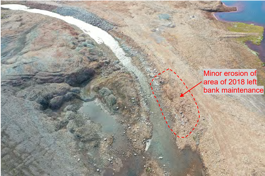
Photo 14. East Twin Creek Diversion – Overview, looking downstream from UAV. Note minor erosion near upper right.
