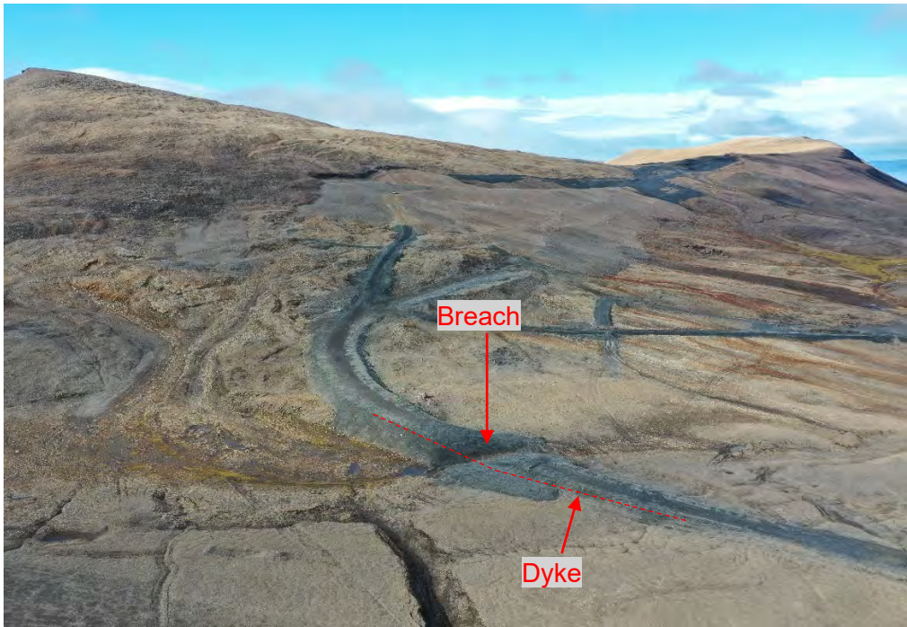
Photo 2. East Adit Treatment Facility - Breach in treatment pond as seen from UAV.
