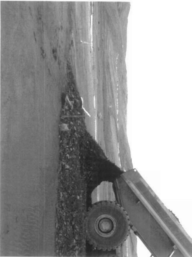
23-Jul-04 Photo 035 WTDA End dumping for constructing the test fill at north end of Surface Cell.
