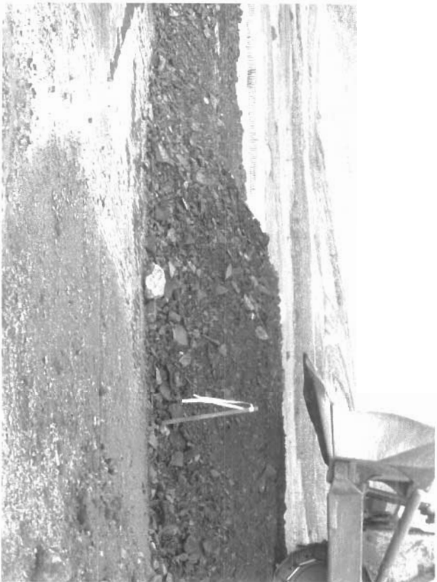
23-Jul-04 Photo 044 WTDA Constructing the top 0.5 m lift of the test fill.
