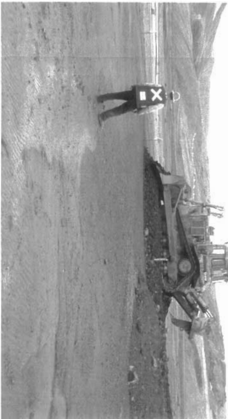
23-Jul-04 Photo 034 WTDA Constructing test fill at the Surface Cell. Note the pad is being advanced by a D8 dozer in 0.5 m lifts.
