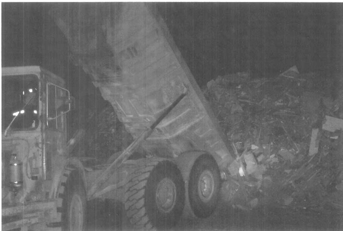
Demolition debris from the town site demolition being dumped underground in the 10 block storage area.
