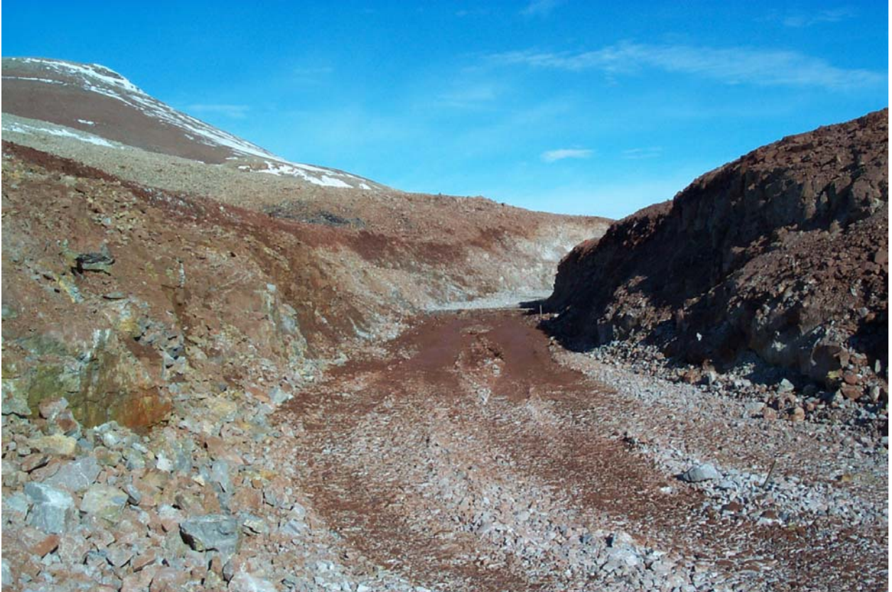
Newly Constructed Spillway from the Surface Cell to West Twin Reservoir
