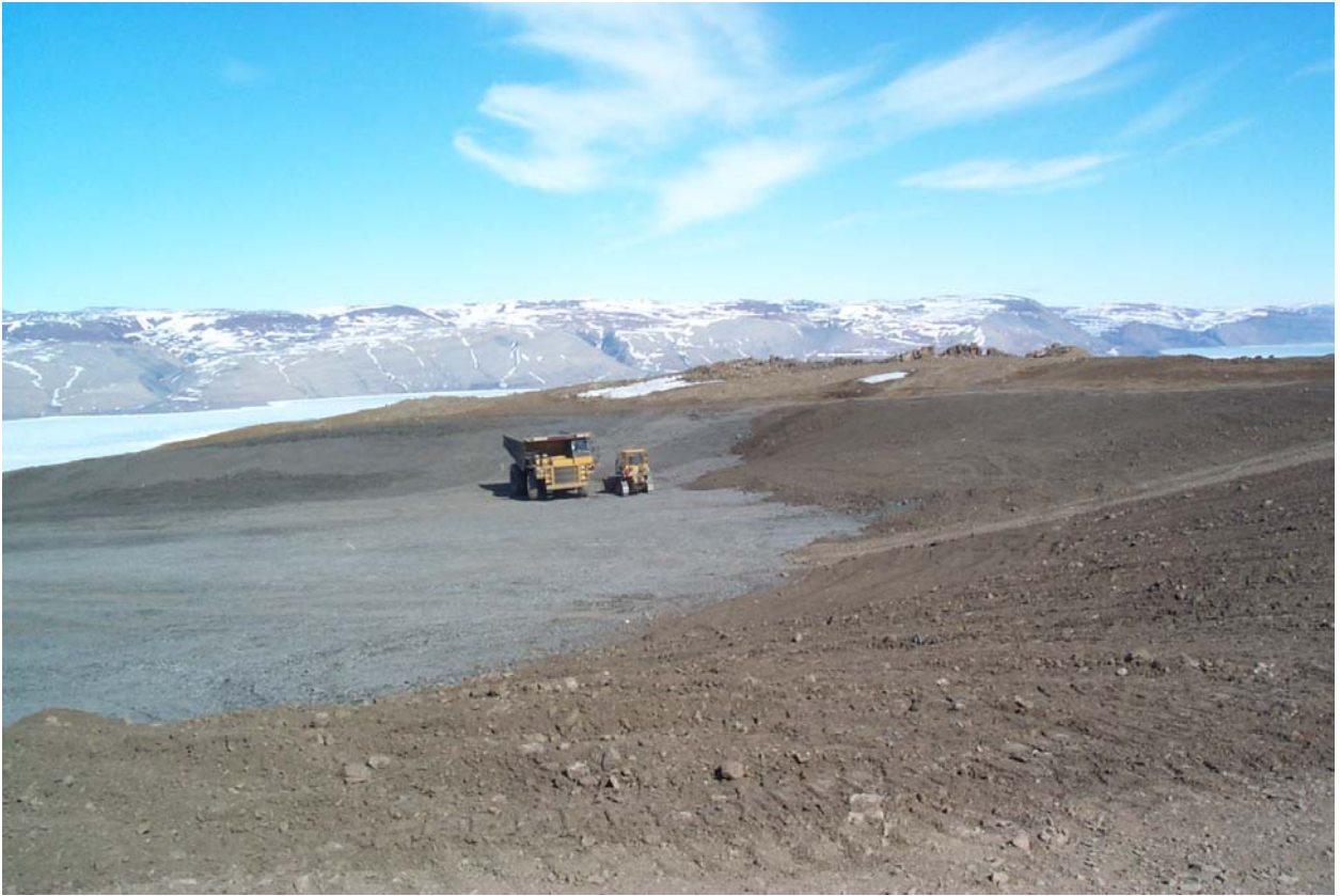
Sand and Gravel Cover in progress at the Ocean View Pit
