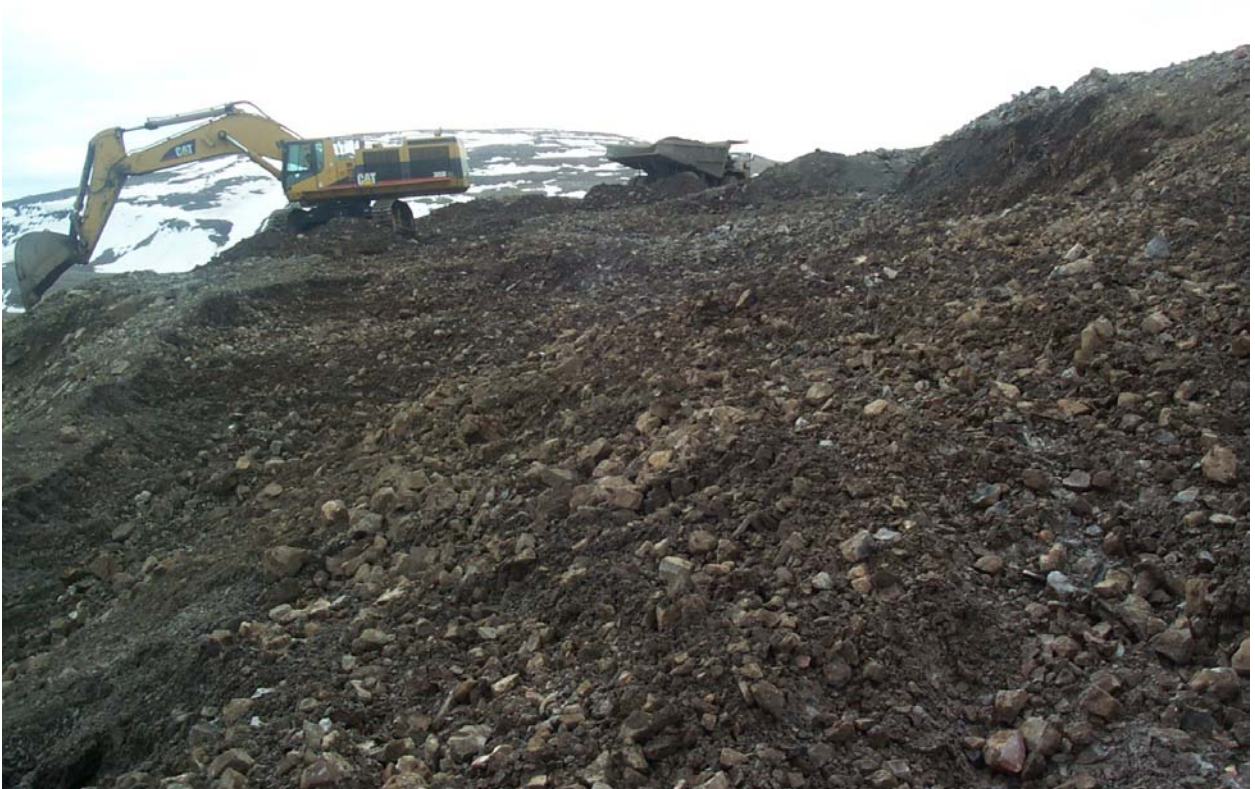
Excavating the East Pit waste rock pile down to original ground
