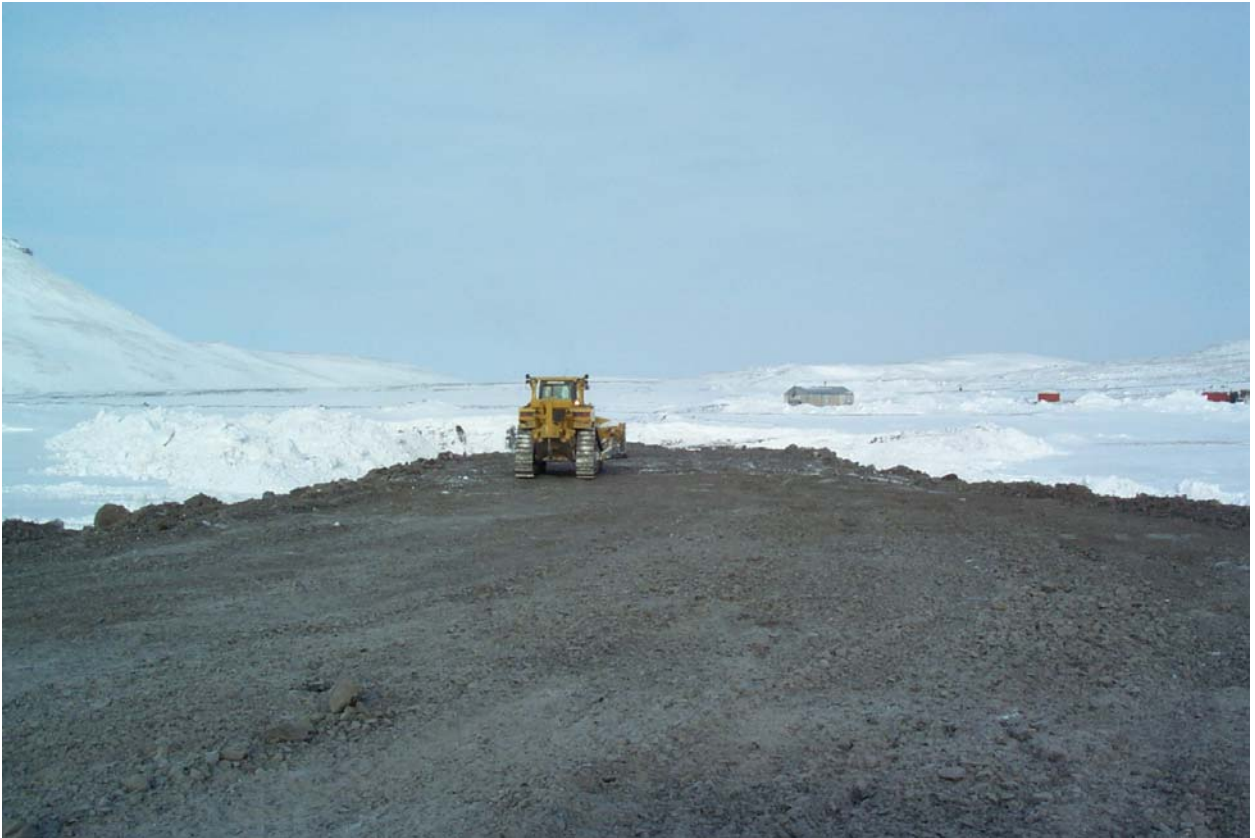
Haulage Road Construction from The East Twin Quarry to the West Twin Deposition Area
