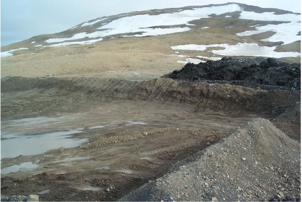
Landfarm excavated and ready for recontouring
