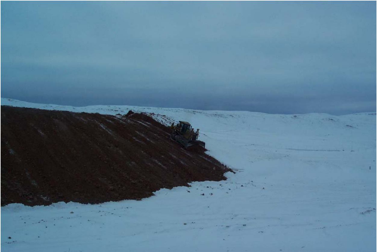
Finishing touches on the sand and gravel armouring at the Landfill site
