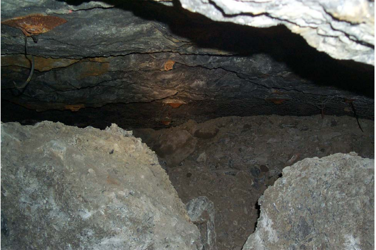
Backfill placed inside the mine opening adjacent to the West Open Pit
