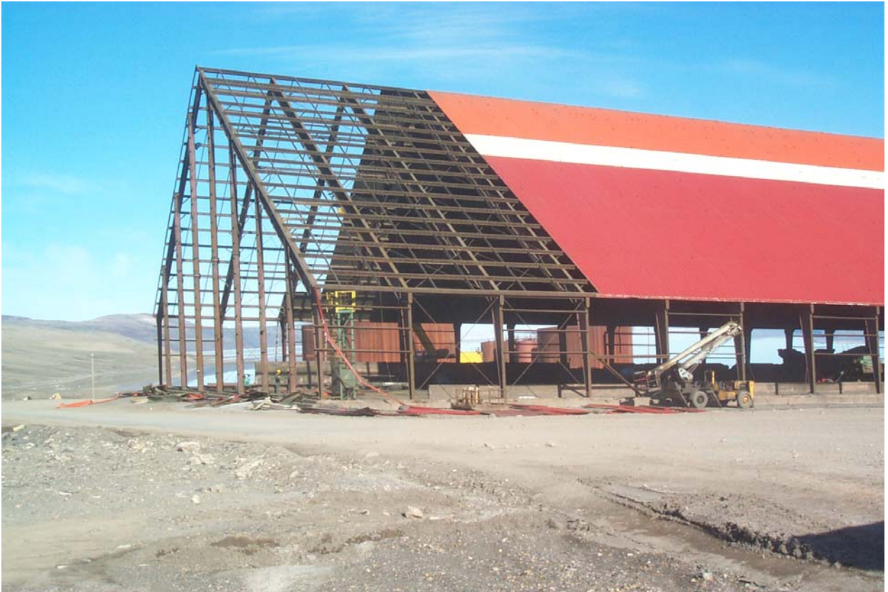
Concentrate Shed with portions of the exterior cladding removed
