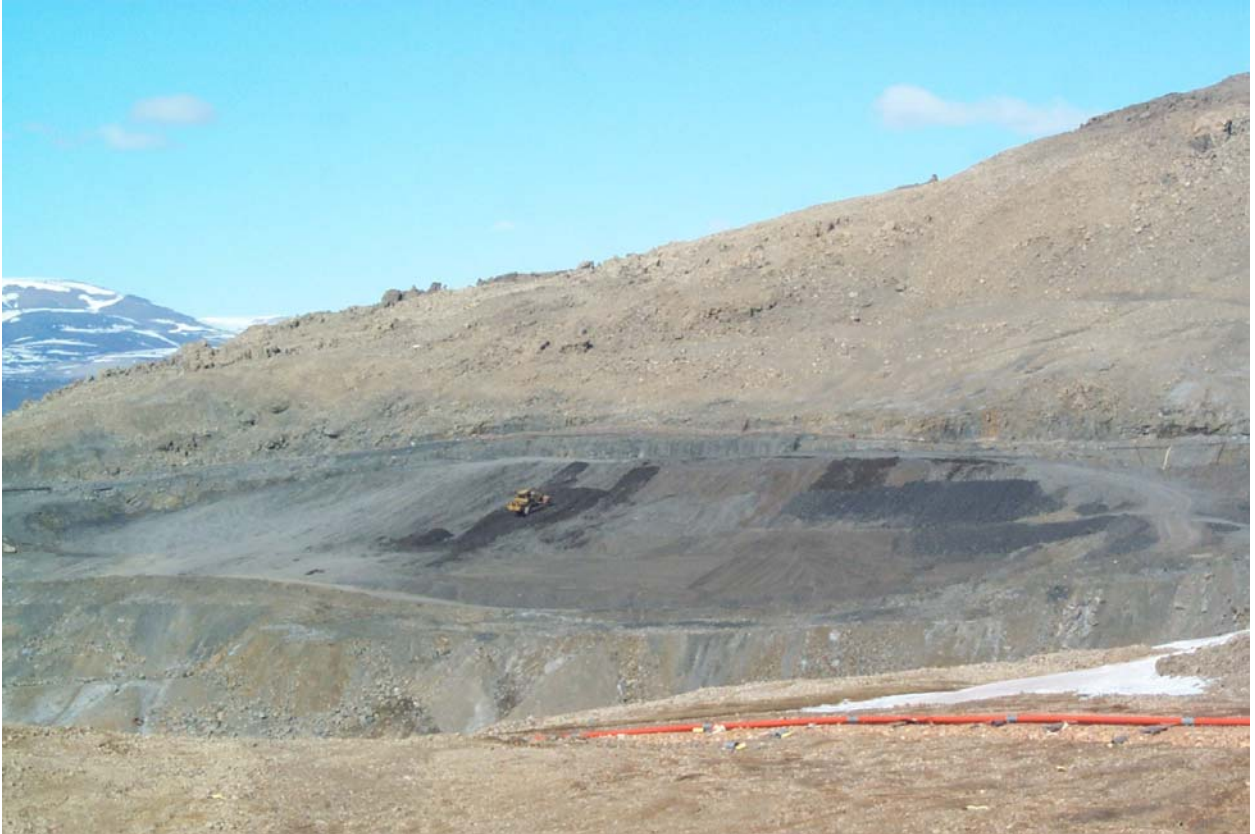
Shale cover for the West Open Pit nearing completion
