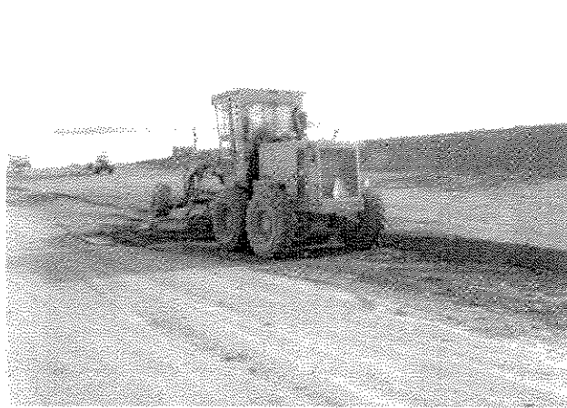
Scraping up metal contaminated soil
