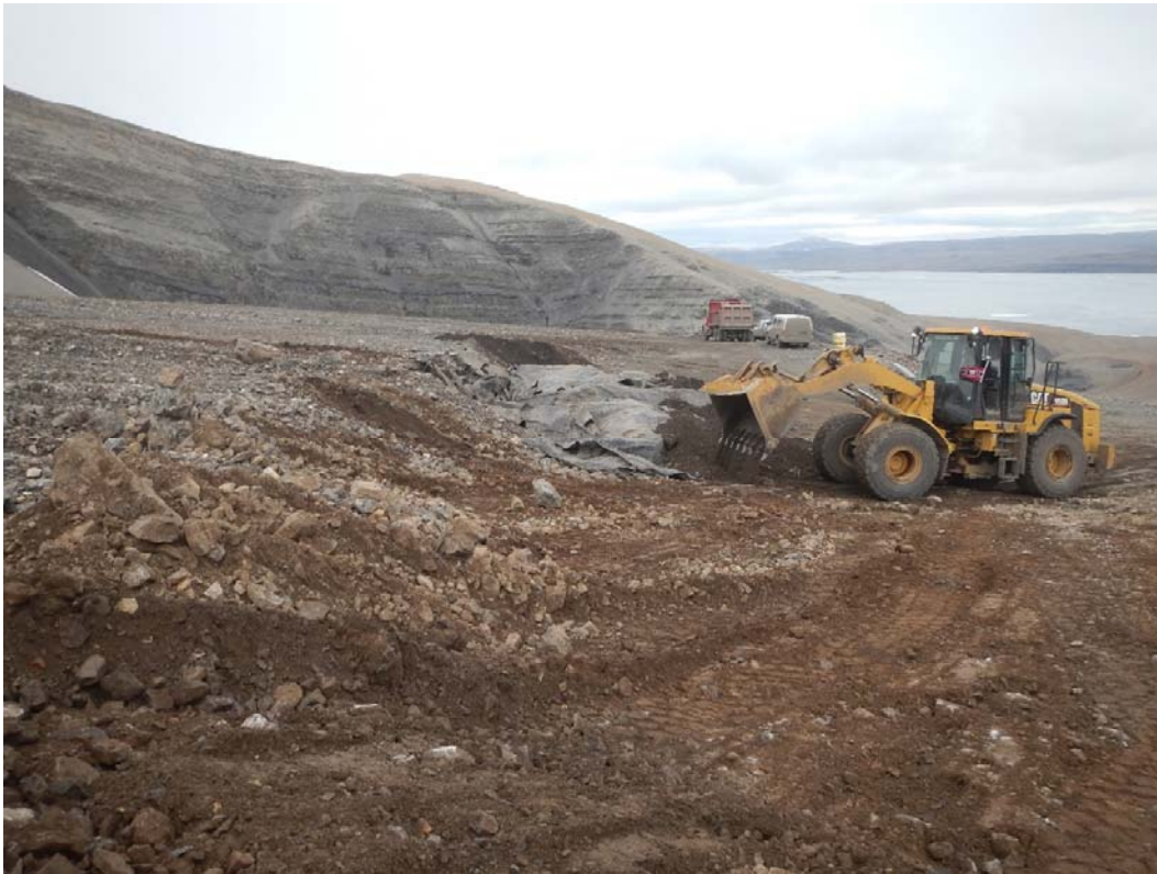
Photo 3: Landfill cover construction progressing from the middle toward the east. Photo looking north-west.
