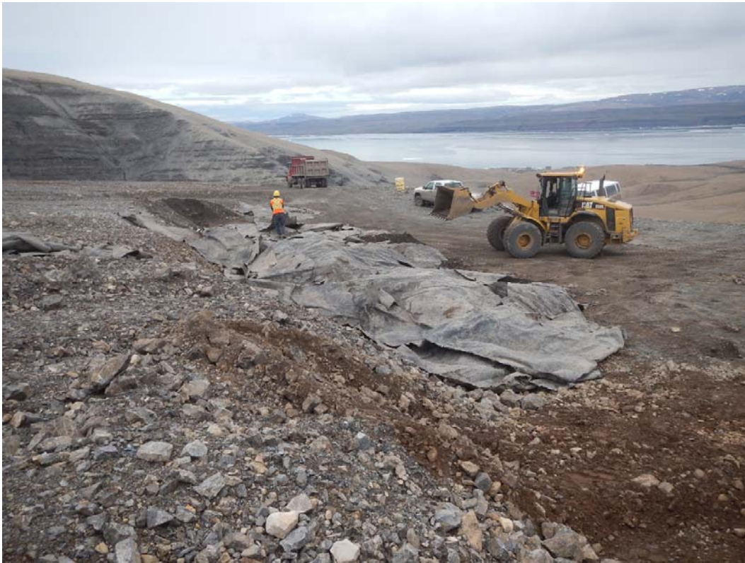
Photo 1: Large pieces of liner were stretched out over the waste in the landfill and the edges were backfilled with cover material to weigh them down. Photo looking north-west.
