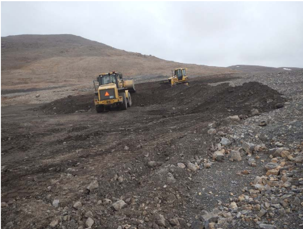
Photo 4: The upstream side of the landfill was covered by pushing the unconsolidated cover material with a dozer. Photo looking south-east.
