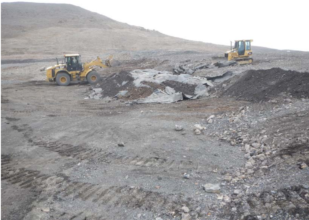
Photo 2: The outer slope of the landfill was covered with cover material relocated using the loader from the west edge of the landfill. Photo looking east.
