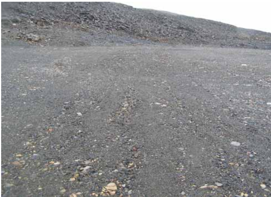
Photo 40 Very minor rill erosion attributed to constant seepage on surface of East Trench cover. Similar to what was observed in 2008.
