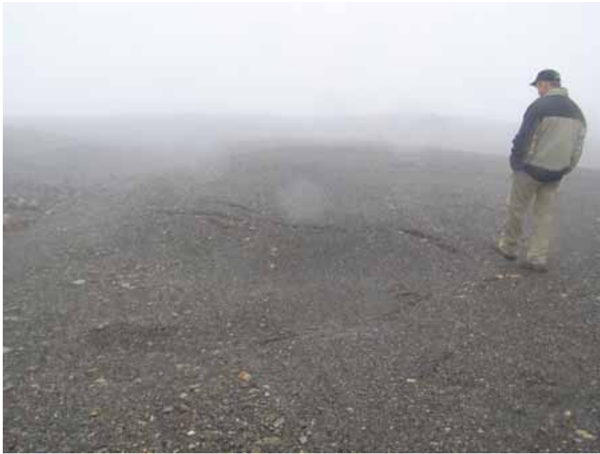
Photo 51 Settlement depression at the southwest corner of the Oceanview Portal cover. Note that the depression does not appear to have progressed since 2008.
