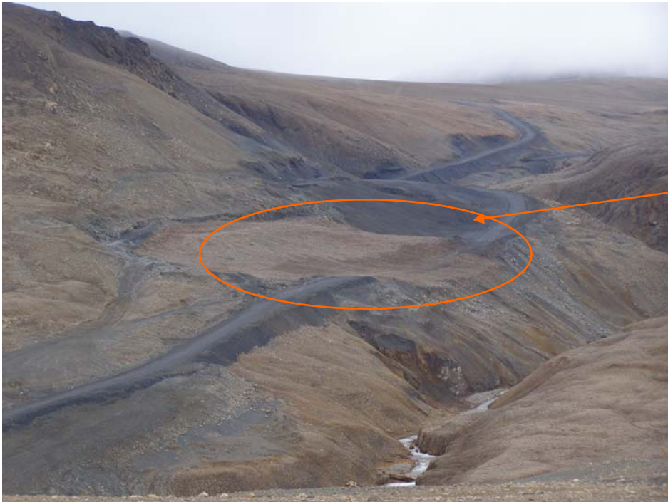
Photo 31 West Open Pit waste rock cover as seen from Stol Port. Note that the road has been armoured over.
