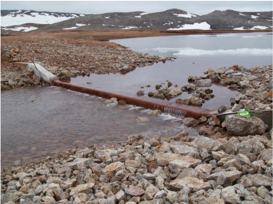
Photo 12 West Twin Outlet Wall in mid-August 2009.
