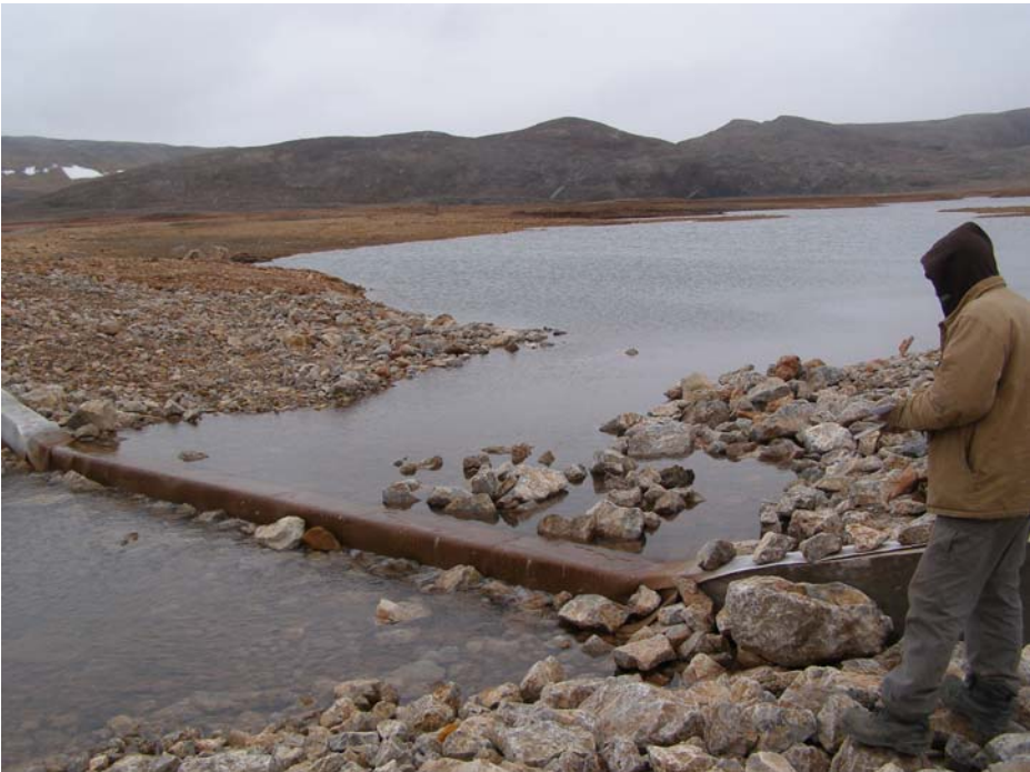
Photo 11 West Twin Outlet Wall in mid-August. Note water is flowing over the wall.
