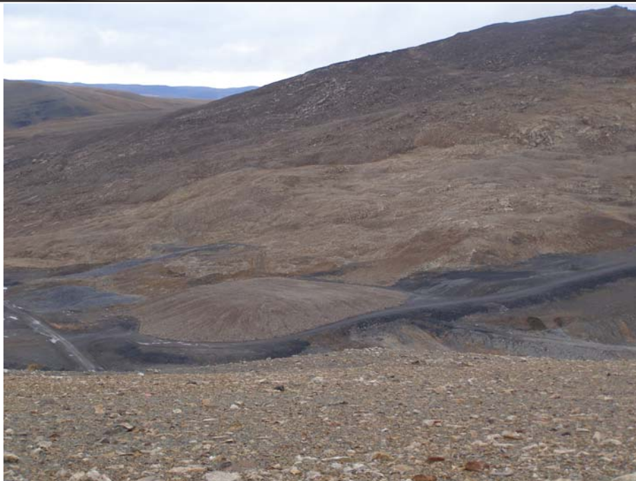
Photo 47 Industrial Complex cover as seen from Stol Port. Note that this cover was completed over metals contaminated soil and the original foundation during the summer of 2008.
