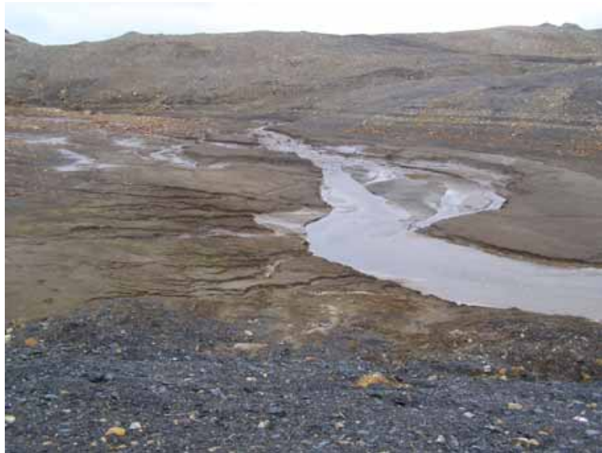
Photo 2 East Adit Treatment Pond. Channelized sediments in the bottom of the East Adit treatment pond.
