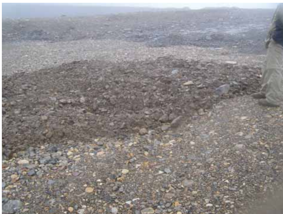
Photo 50 Backfilled thermokarst feature in 17N Portal Cover. Note that it is continuing to show signs of surficial disturbance.
