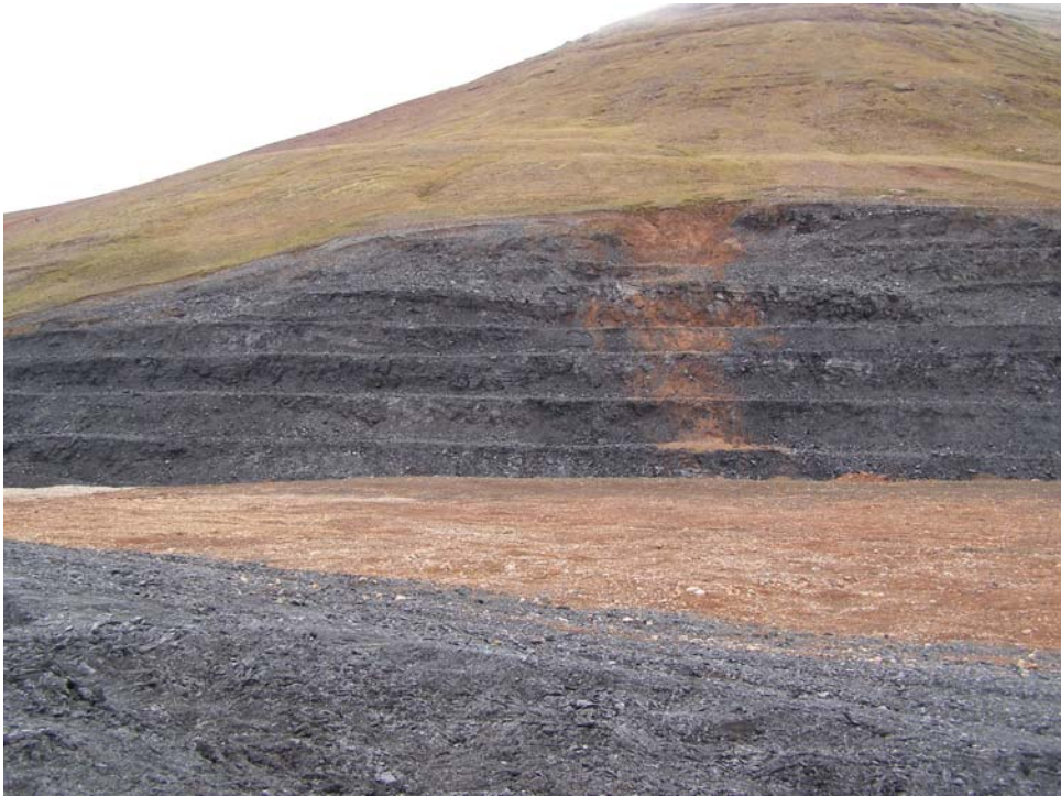
Photo 64 Mt. Fuji shale borrow area. Note the natural cover material is falling down from above over the benches.
