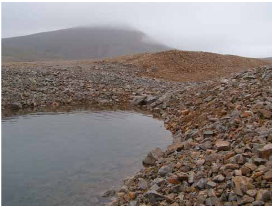
Photo 22 Rip rapped Test Cell outlet. Note riprap extended below water line.
