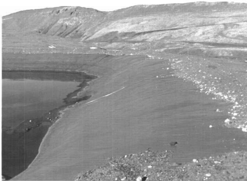
Photo 154 shows a view of the eastern berm of the Upper Dump Pond. The liner is quite wrinkled but some fill has been placed on top in an attempt to anchor the liner better.
