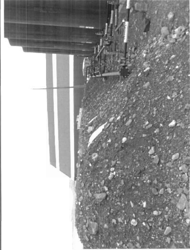
Photo 270 shows a new berm that was placed along a portion of the north berm. This new lift appears to be approximately 1.2 to 1.4 m high.
