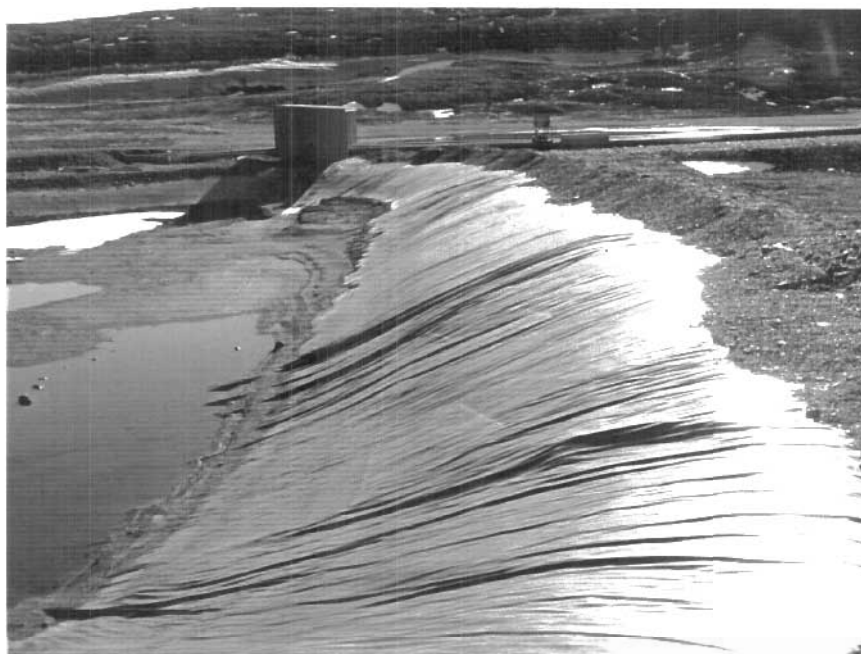
Photo 157 shows a view along the top of the western berm of this dump pond. No signs of cracking of the liner were noted. No signs of berm settlements or cracking or seepage at its downstream end have been noted either.
