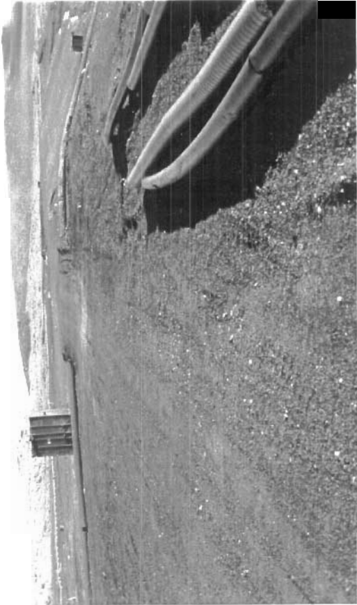
Photo 45 shows a view of the crest looking towards the north. Some minor pot holes are evident near the north limit of the spare pipes.
