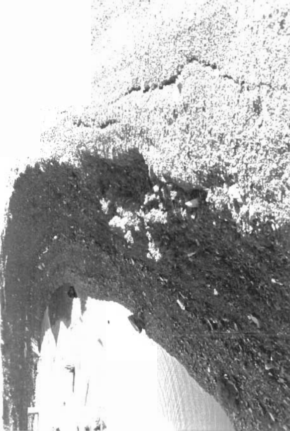
Photo 93 shows a view of the inside edge of the dike. This portion was the more recent fill placed to close the gap between the N-S and E-W portions of the Test Cell dikes. These cracks are the result of the oversteepened nature of the fill placed in this portion of the dike.
