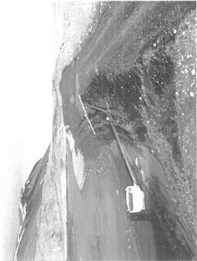
Photo 202 shows a view of the upstream side of the dike. Note the multiple beach lines and the appearance of the steepened upper section of the dike face .
