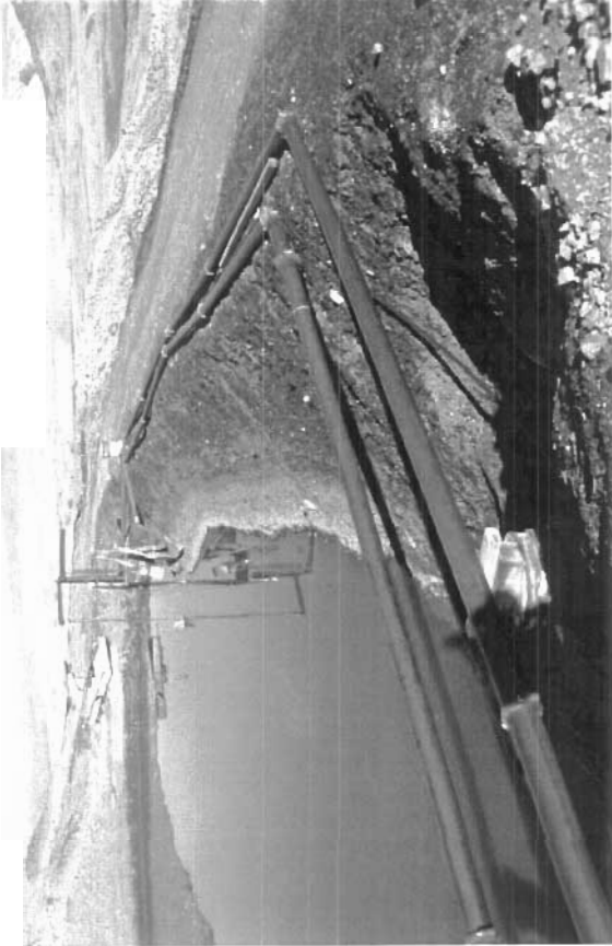
Photo 182 is a view of the crest of the Treatment Pond Dike. Pipeline used to pump water for lime treatment. Note the lighter coloured fill that has been recently placed on the crest.
