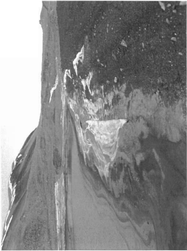
Photo 207 shows a view of the GCL which was previously placed on the upstream side of the dike. The top of the liner has dropped somewhat and needs to be re-installed. In the background of the photo can also be seen that some of the GCL has been caught by the wind and needs to be re-installed properly.
