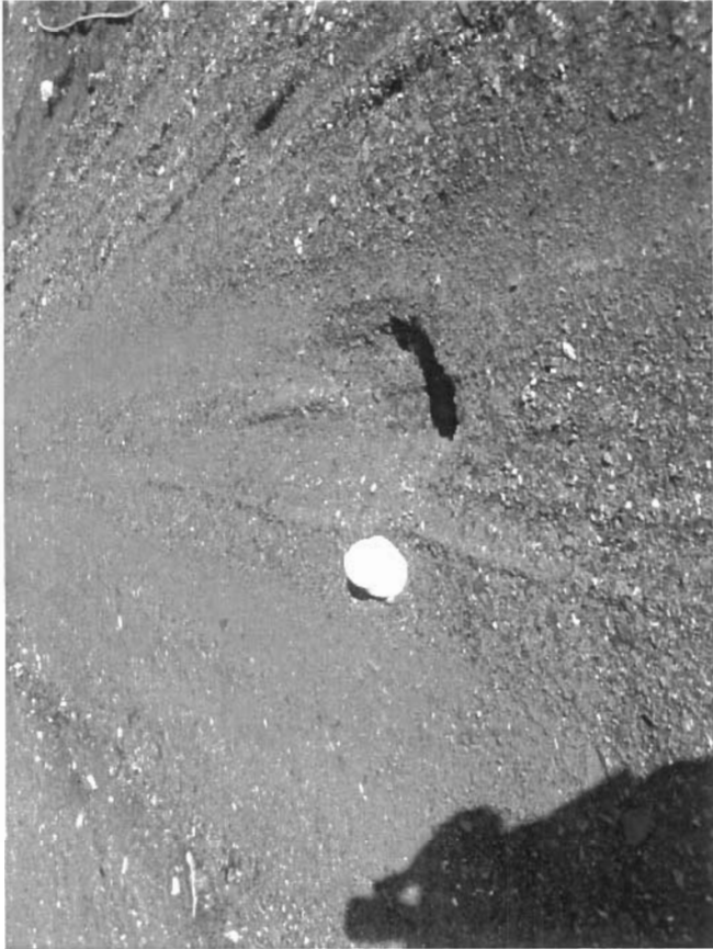
Photo 104 shows a view of a small sinkhole located in the crest of the Test Cell Dike.
