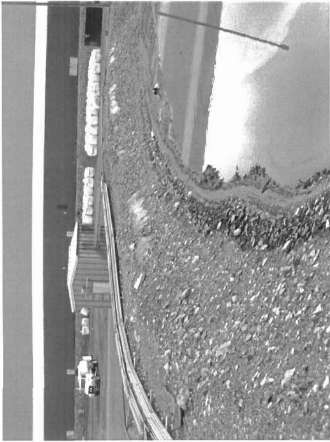
Photo 275 shows the dike crest, the retained pond and the exposed geomembrane liner (which does not appear to have any major cuts).
