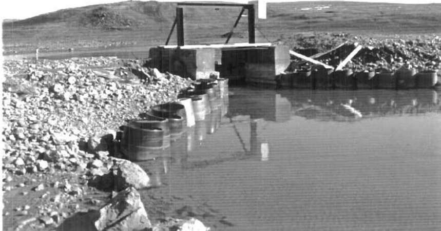
Photo 113 shows the decant spillway structure at the outlet of the polishing pond. There's a steel gate within five valves within the concrete structure that allows water to be decanted from the pond. This photo shows the erosion on the sides of wing walls of the concrete structure.
