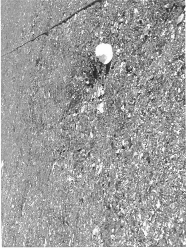
Photo 44 shows a view of some small settled areas just behind the hard hat. These are located some 3 metres down the downstream slope from the crest elevation. This photo was taken near the water discharge lines.
