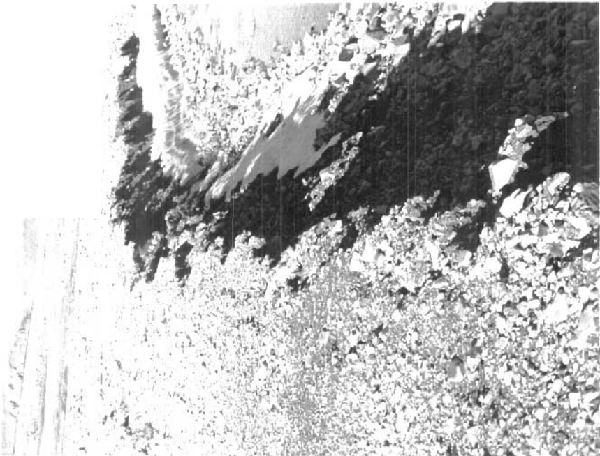
Photo 144 shows a close up view of the crest of the Diversion Dike. There is cracking occurring due to erosion on this side of the dike. Hence, some repairs and riprap will be required to prevent the erosion from getting worse.
