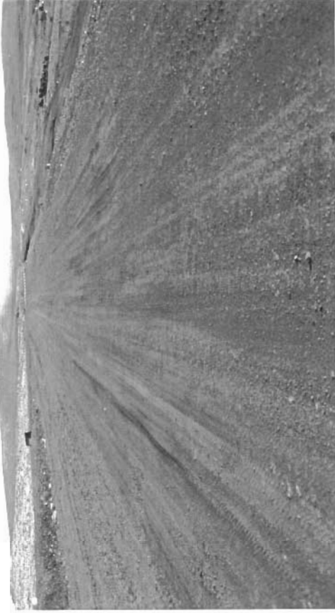
Photo 64 shows a view of the crest of the northern portion of this dike. In general, the surface is in good condition, although some minor pot holes are evident at this location.
