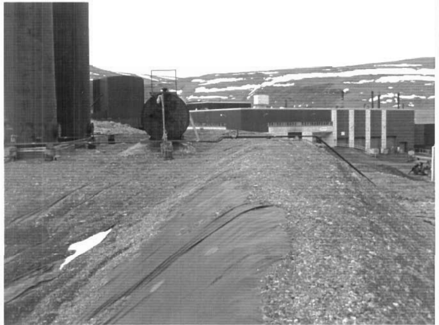
Photo 238 is a view of the exposed liner along the west berm. No cuts or tears were observed from this location.
