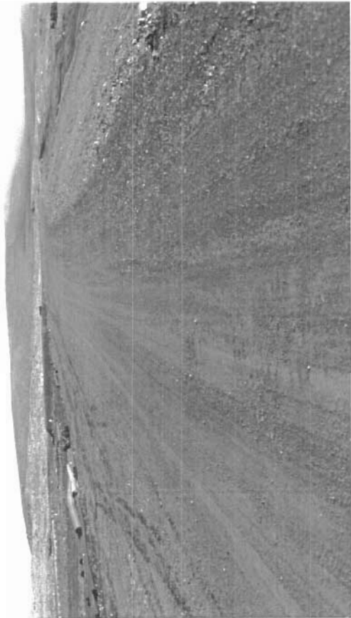
Photo 59 shows a view of the upstream crest looking towards the north abutment. No signs of significant settlement or deformation.
