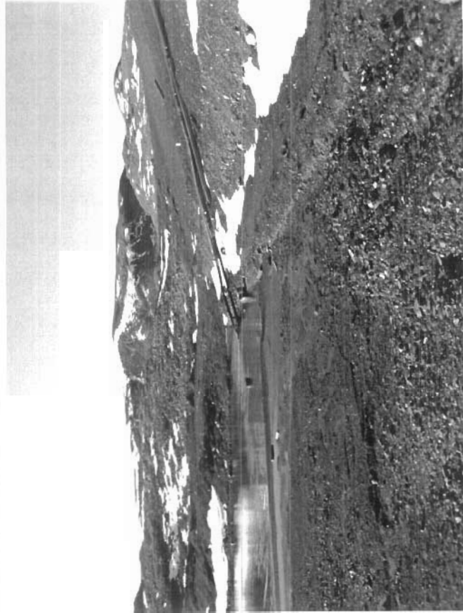
Photo 77 is a view along the toe. In the mid ground can be seen the lines which discharge water from the Surface Cell into the Reservoir. In addition, the initial placement of shale covering can also be seen over some tailings at the toe .
