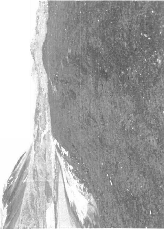
Photo 206 shows the undulating nature of the shale fill that was previously placed on the upstream face of the dike. Note the settlement troughs and cracking.
