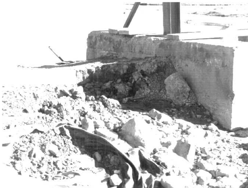
Photo 114 shows a close up view of the erosion that has occurred on the left wing wall. This needs to be repaired and then riprap should be placed on the upstream side to prevent future erosion.
