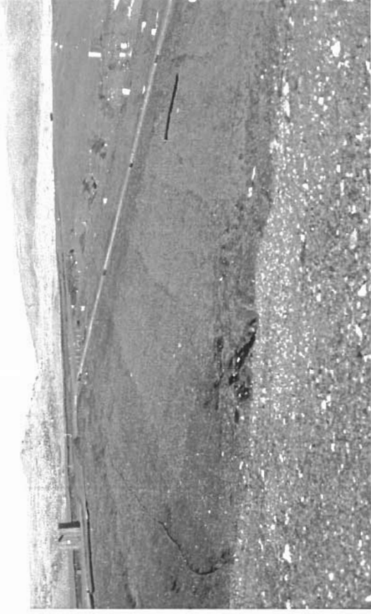
Photo 35 shows a view of the contact between the dike embankment fill and the native ground rising to the right at the south abutment. There are no wet spots or signs of seeping water. Note that some settlement of the fill has occurred where it was placed to smooth the benched appearance.
