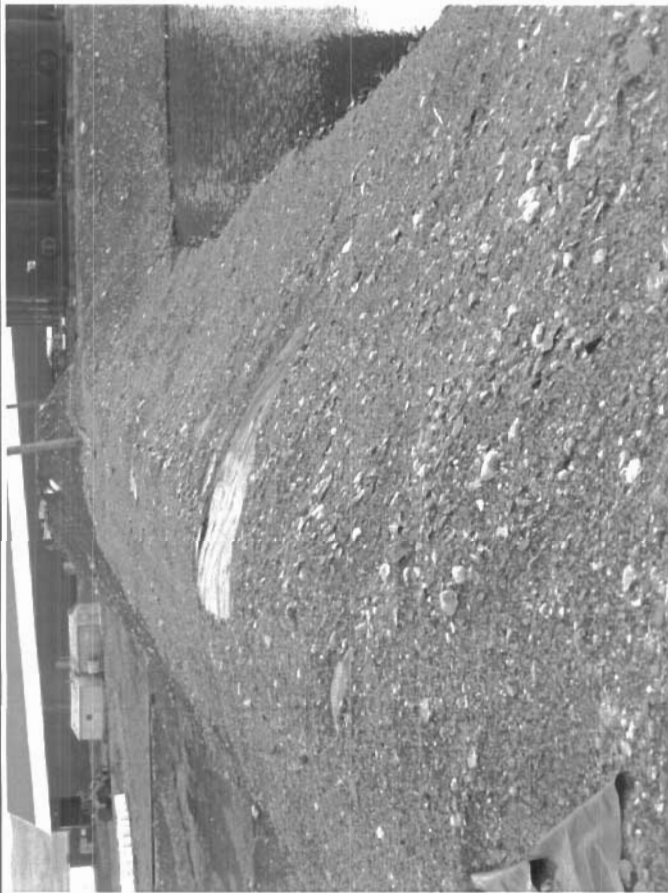
Photo 267 shows the crest of the north berm. There are several locations where the liner is exposed.
