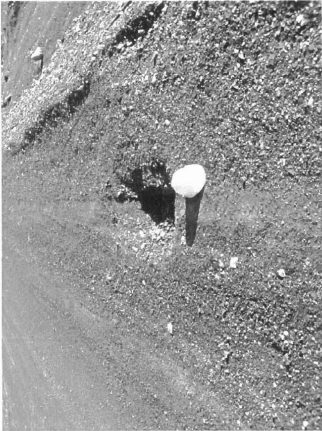
Photo 55 shows a sink hole located in the crest of the dike, above the portion of the dike that remains benched.
