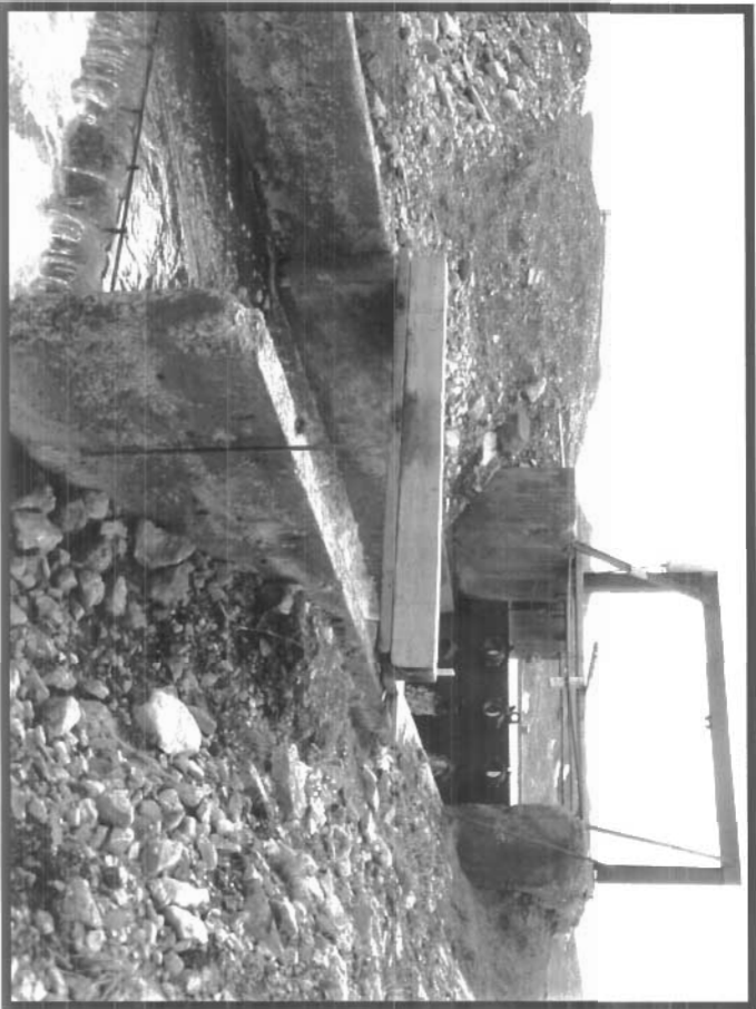
Photo 116 is of the Polishing Pond Outlet structure. Note the flow is only occurring from the middle and bottom valves.
