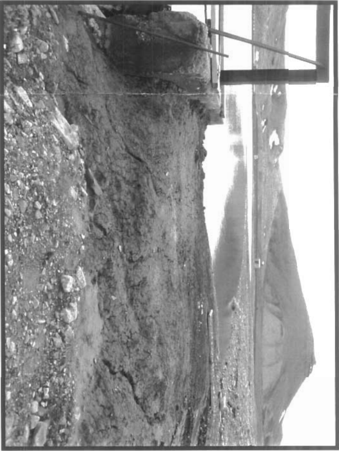
Photo 118 is of the north side of the of Polishing Pond Outlet structure. Note the erosion around the concrete observed last year has been repaired by placing additional marine silt and clay.
