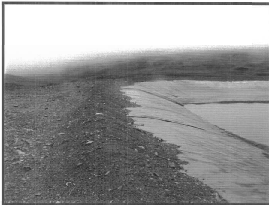
Photo 31 is of the shale and native ground material holding down the liner.
