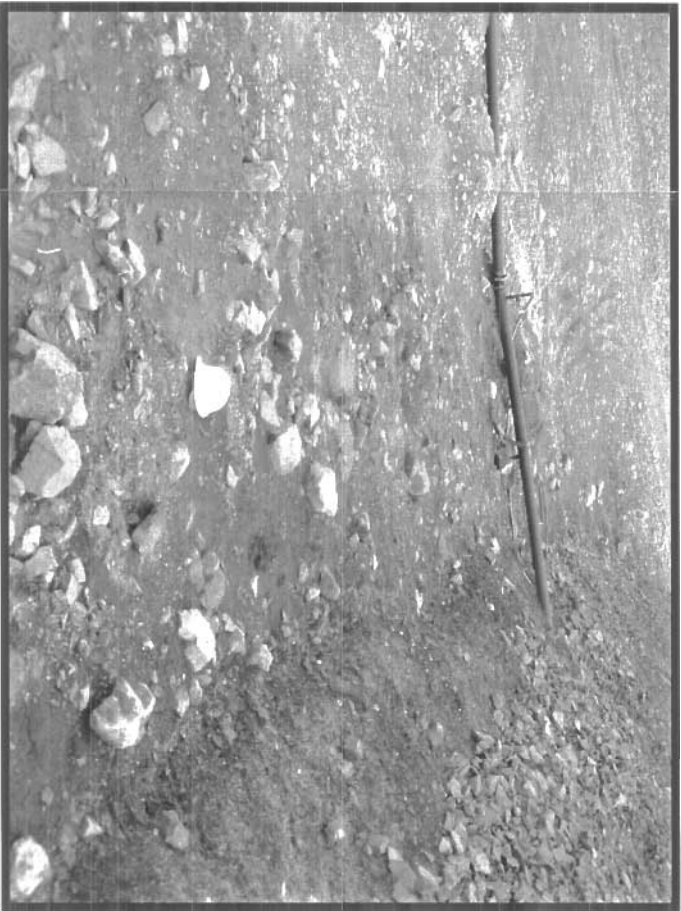
Photo 140 is a view of the downstream face of the dike at the centre of the dike. Note the wet area near the toe of the dike (by the hardhat). This may indicate seepage beneath the dike at this location.
