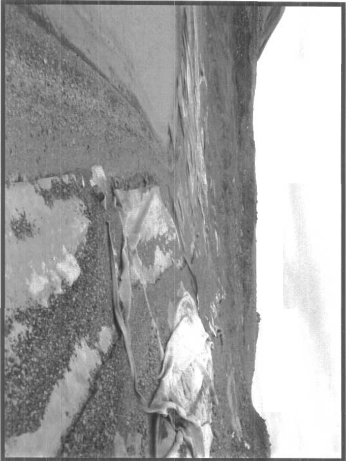
Photo 136 is a view of the northwest corner of the treatment pond. Note the ruffled nature of the liner.
