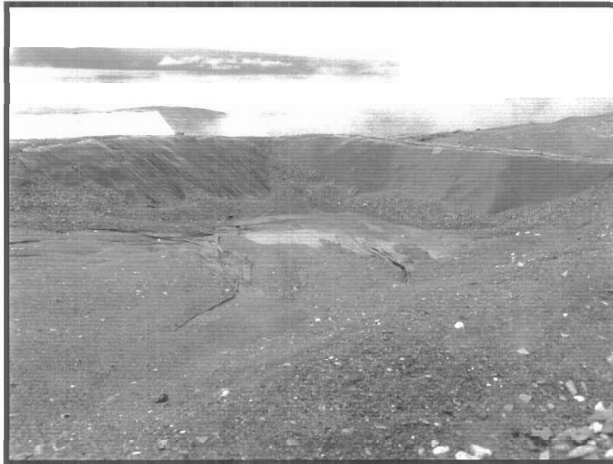
Photo 10 is taken towards the north end of the Tank Farm in the water collection pit. Note that there is currently approximately 50 centimeters of water in the deepest spot collected in the bottom of this pit.
