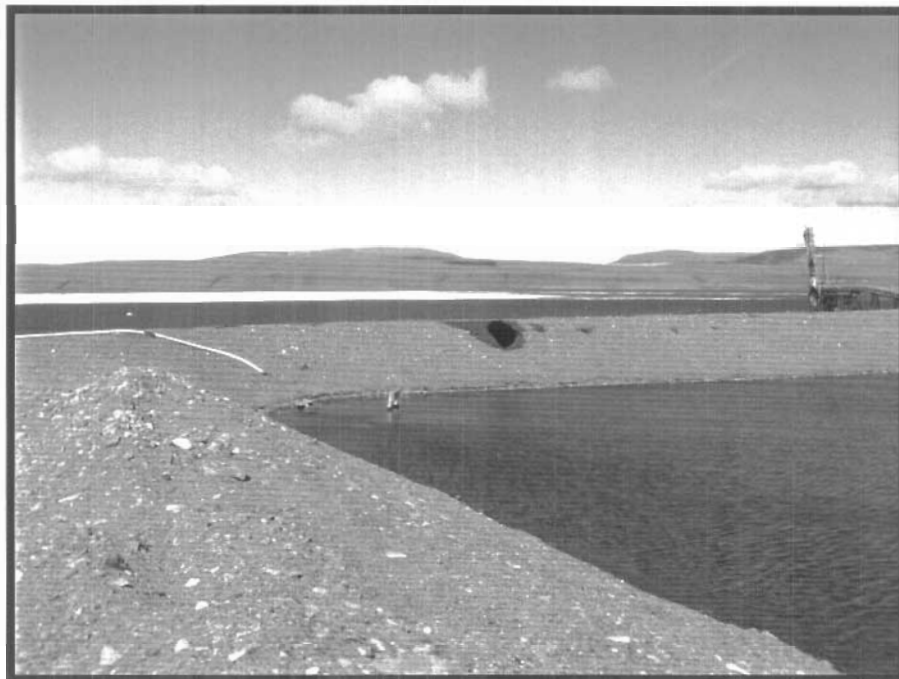
Photo 52 is taken looking towards the northwest corner of the containment berm. It is an area where the liner is exposed. As can be seen it has been repaired at some point in the past. The depth of water within the pond is approximately 50 cm.
