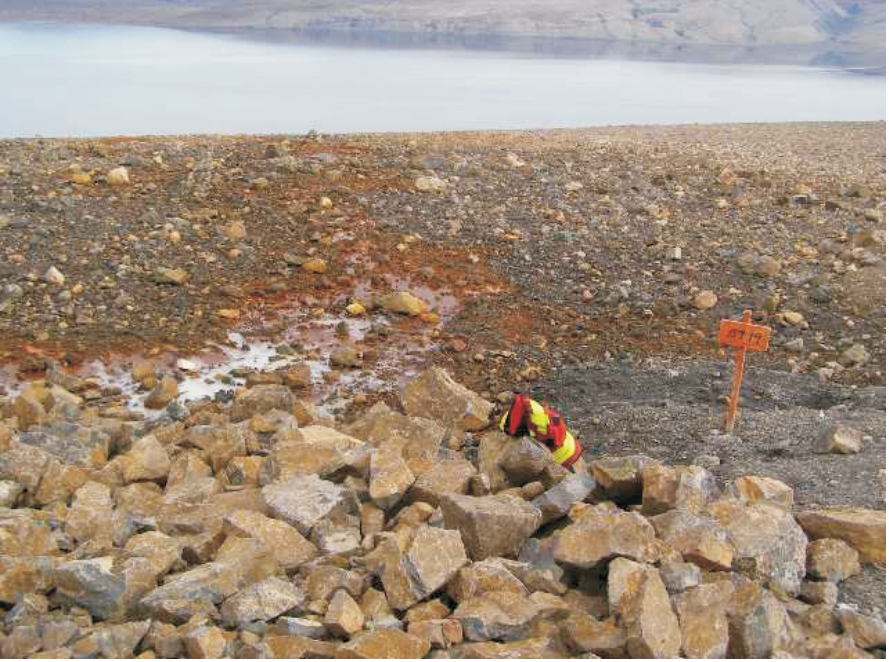
Photo 52 Seepage at toe of Oceanview Open Pit Waste Rock cover.
