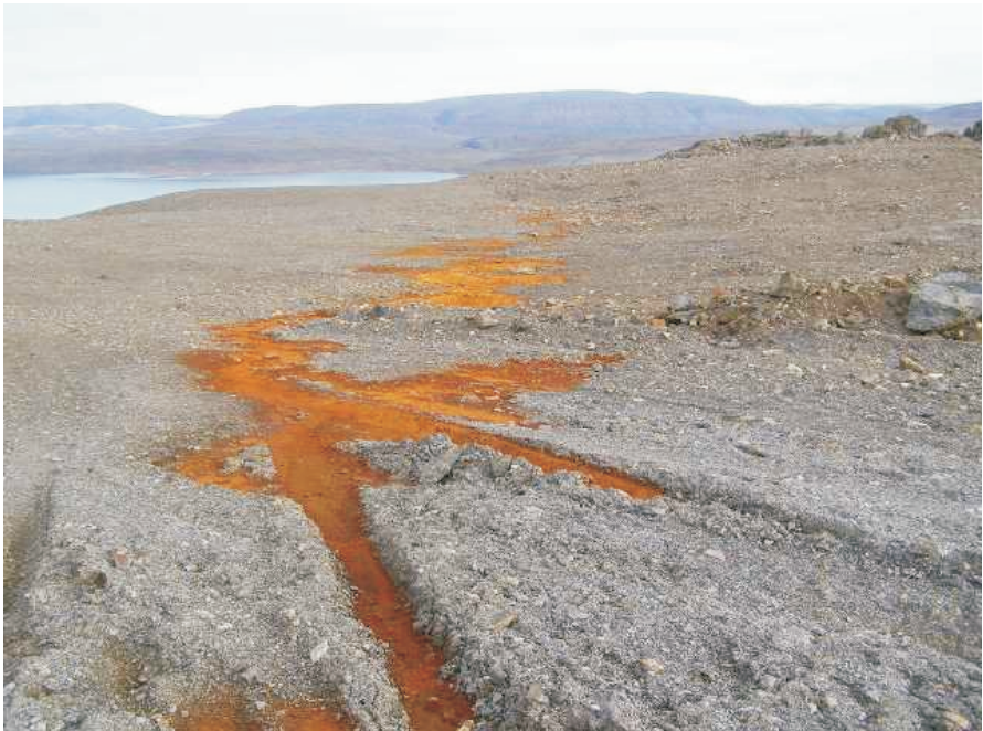
Photo 53 ARD running along east edge of Oceanview Open Pit Waste Rock cover. Note source is upslope of pit.
