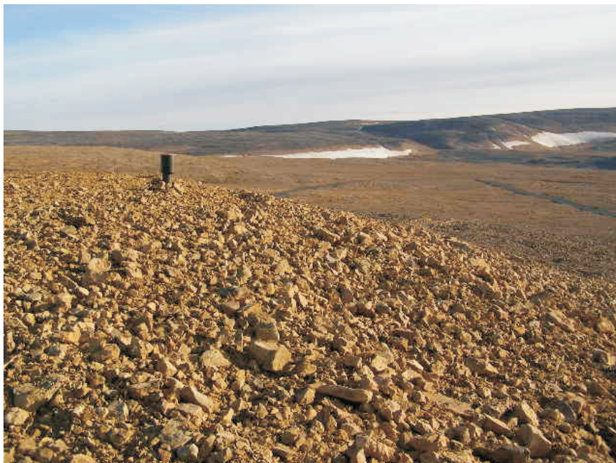
Photo 56 Face of Area 14 waste rock cover. Note location of frost gauge and proximity to edge of cover.
