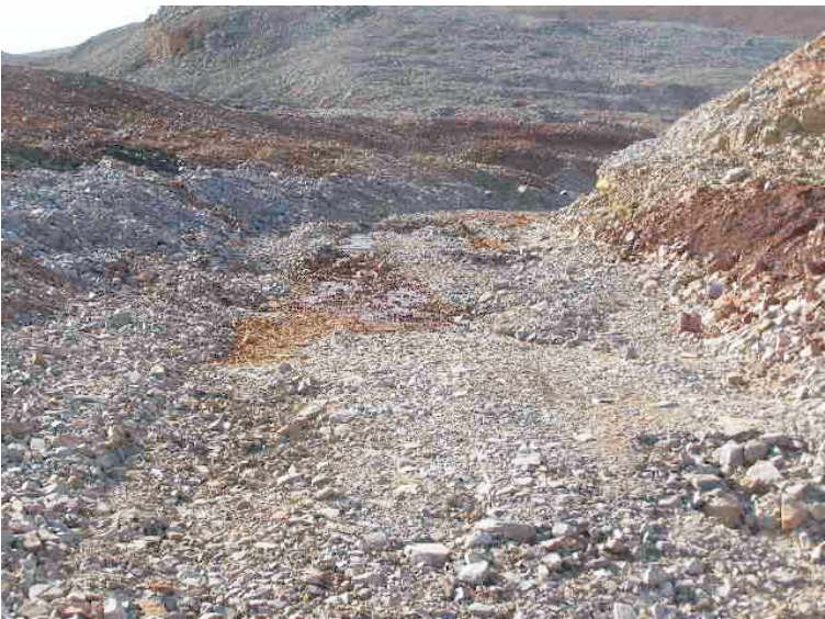
Photo 13 Undulating spillway bottom downstream of access ramp. View looking up gradient.
