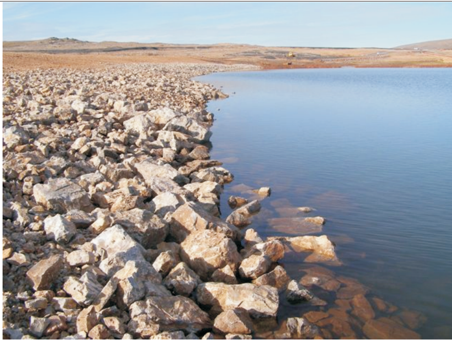
Photo 33 Riprap along shoreline at toe of Test Cell Dike.
