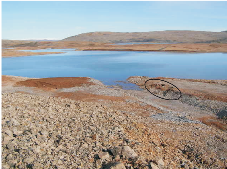
Photo 12 Spillway outlet. Note thermokarsting (circled) along right bank.
