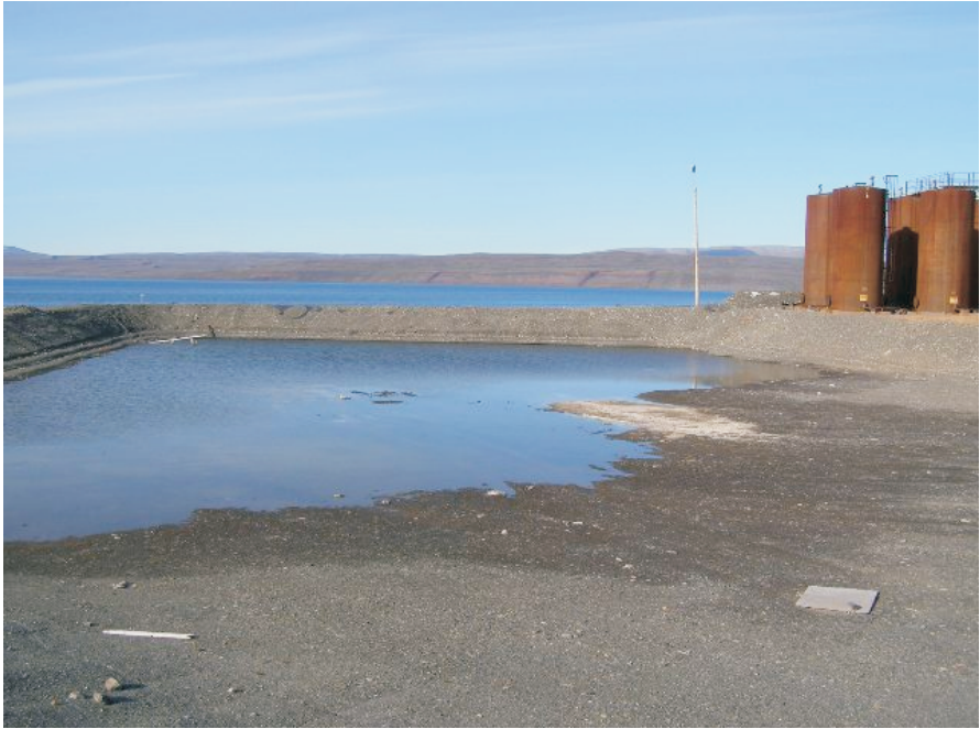
Photo 7 Water in seepage collection pond.
