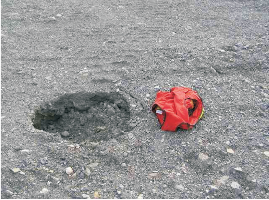
Photo 54 Sinkhole located near north end of Oceanview Open Pit Waste Rock cover.
