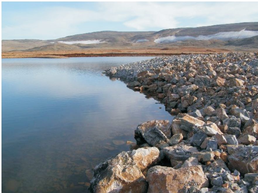
Photo 34 Riprap along shoreline at toe of Test Cell Dike.
