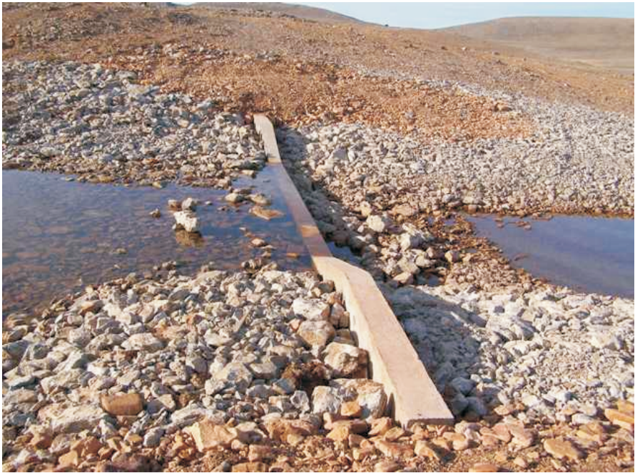
Photo 15 Concrete wall at West Twin Outlet Channel.
