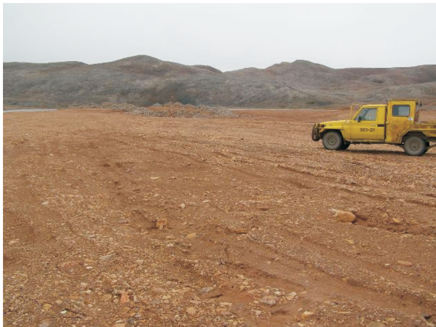
Photo 32 Surface of crest of north/south arm of Test Cell Dike. Note undulations.
