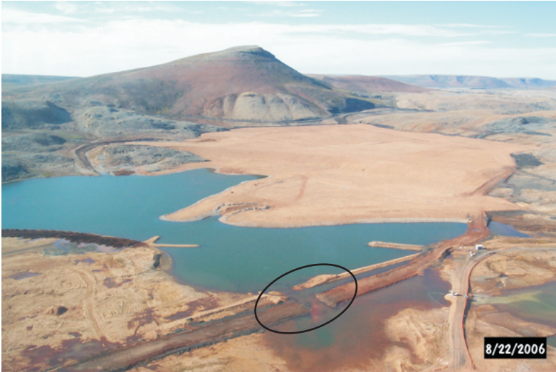
Photo 30 Surface Cell and Test Cell covers. Note breach of rockfill baffle and haul road (in circle).
