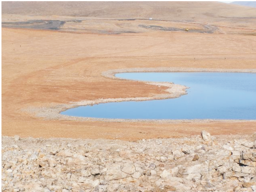
Photo 35 Riprap along shoreline at toe of West Twin Dike.
