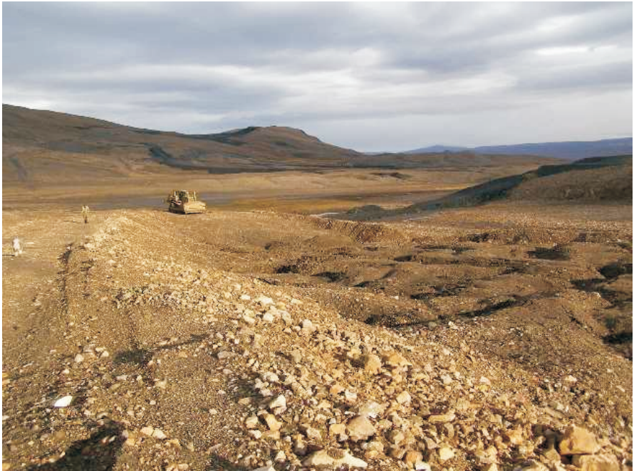
Photo 75 D8 dozer at Kuhulu Lake Road deposit. Note thermokarsting on the right.
