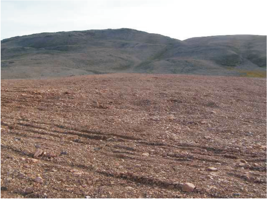
Photo 38 Surface of Landfill cover. Note undulations and loose surface.
