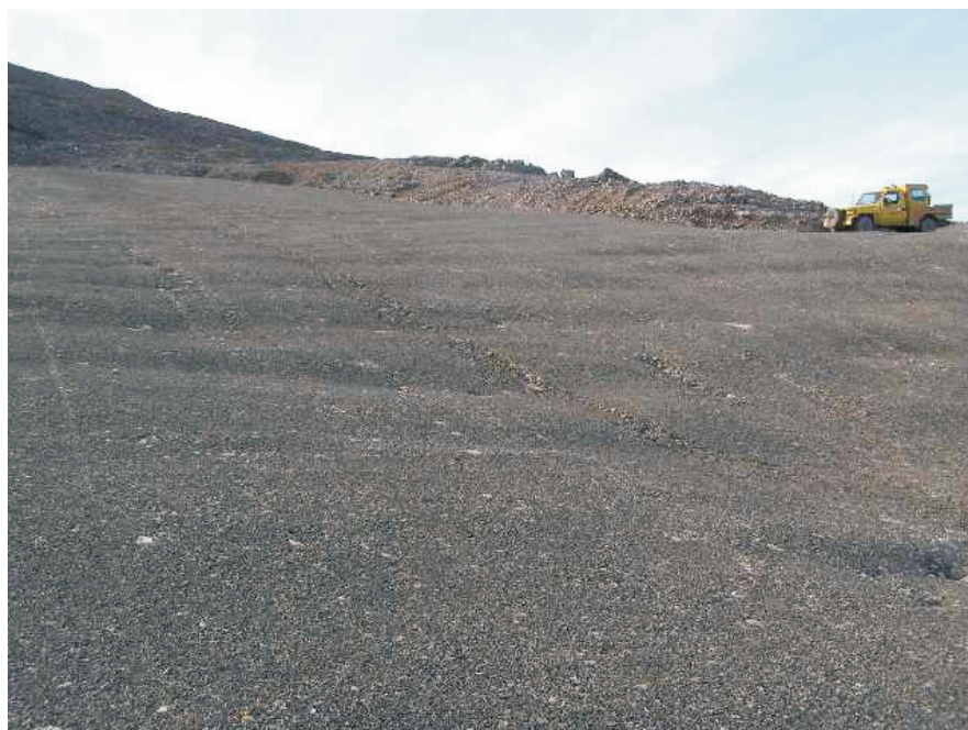
Photo 50 East Trench cover armour surface.
