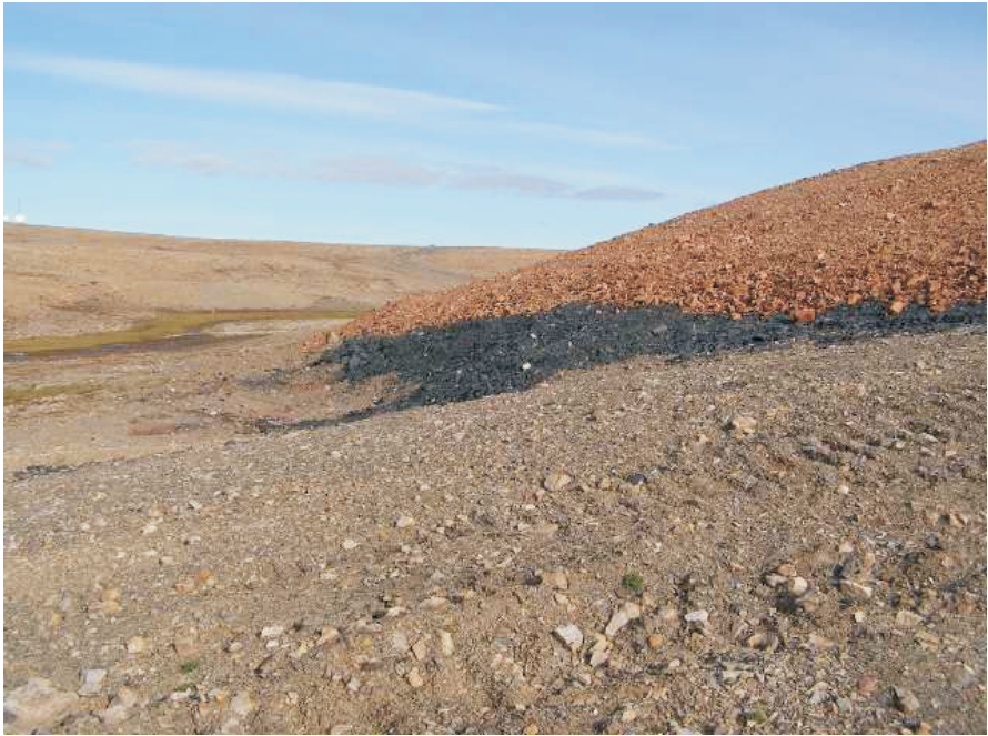
Photo 37 Toe of Landfill cover on west face. Note uncovered shale at toe.
