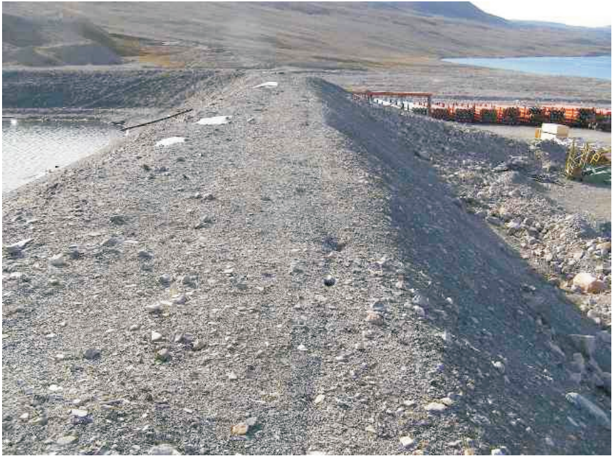
Photo 5 Main tank farm seepage collection berm on the downhill side.
