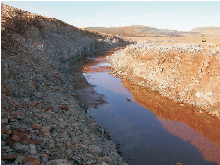
Photo 9 Water running in spillway between inlet and access ramp.
