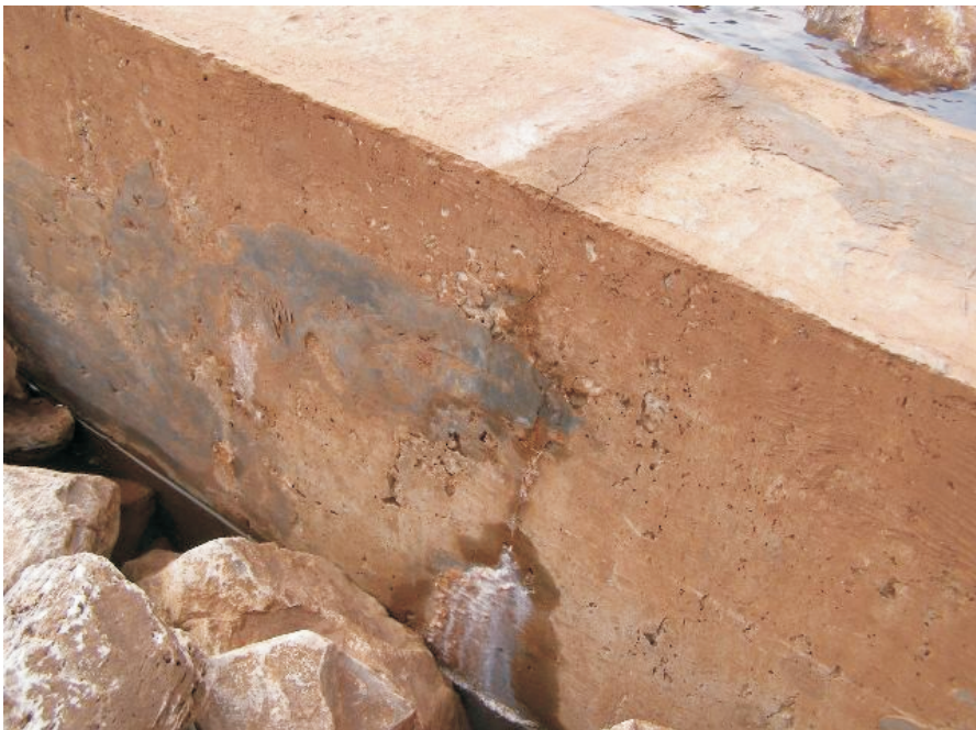
Photo 18 Crack in concrete wall in West Twin Outlet Channel.
