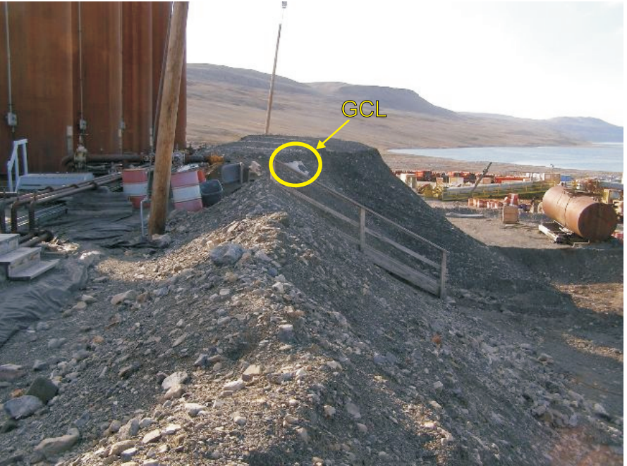
Photo 8 Seepage collection berm. Note a portion has been excavated during removal of hydrocarbon contaminated soils, and exposed the underlying GCL.
