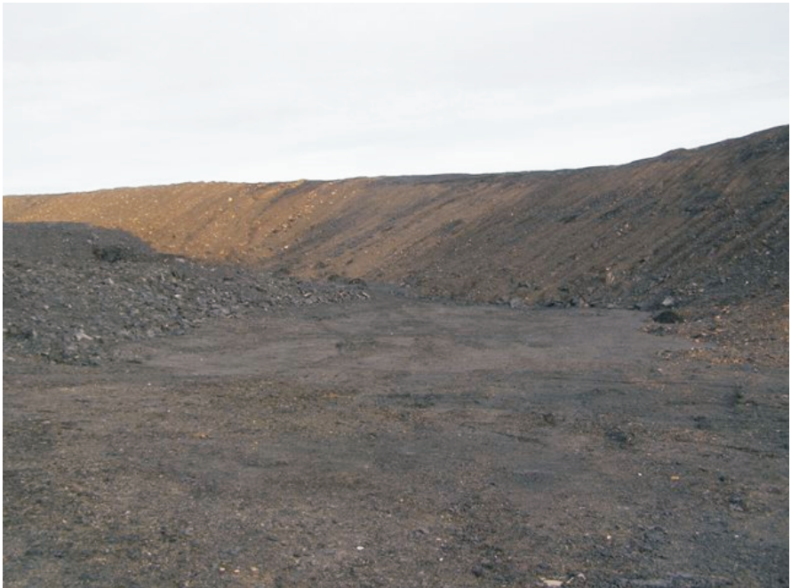
Photo 71 Re-sloped face of Shale Hill borrow area.
