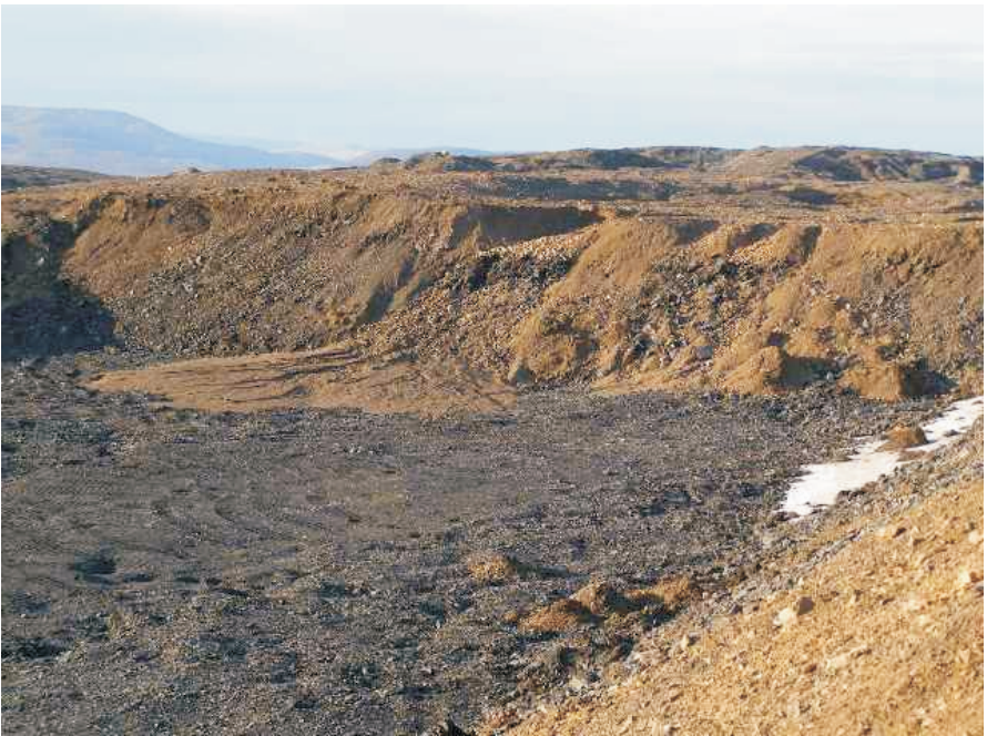
Photo 70 Erosion occurring at north end of Area 14 borrow area.
