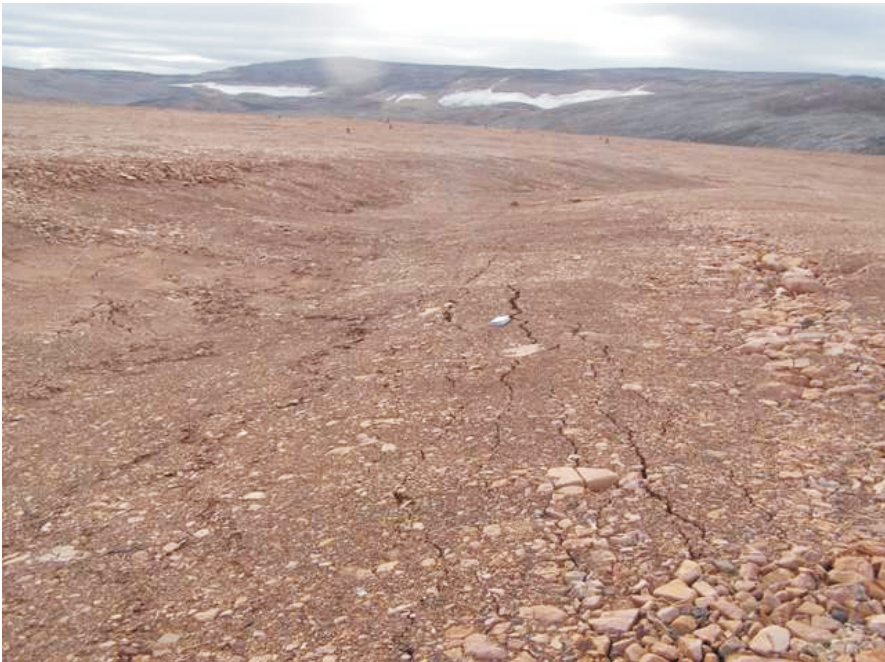
Photo 22 East/West drainage swale at Surface Cell. Note cracking along slopes.
