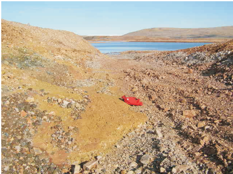
Photo 14 Weathered diabase debris cone in spillway bottom.
