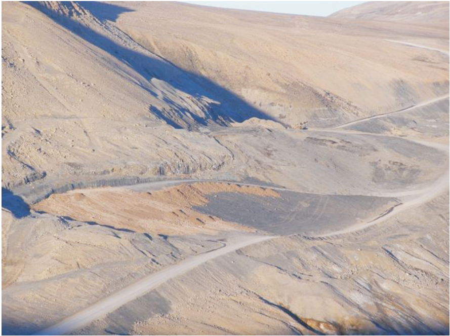
Photo 41 West Open Pit waste rock cover as seen from Stol Port. View looking east. Note armouring still in progress.
