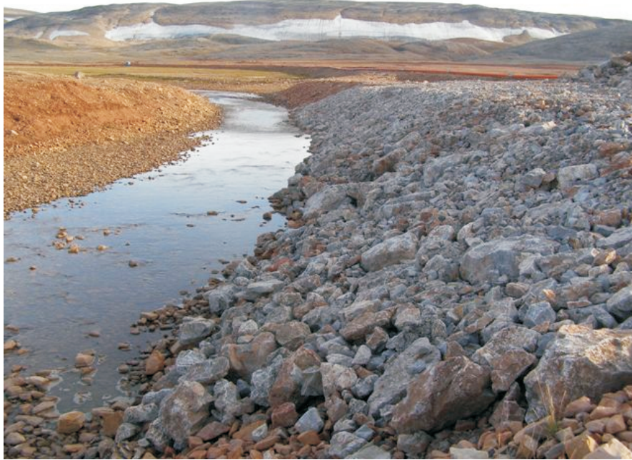
Photo 19 Riprapped face along East Twin Creek Diversion Berm. View looking upstream.
