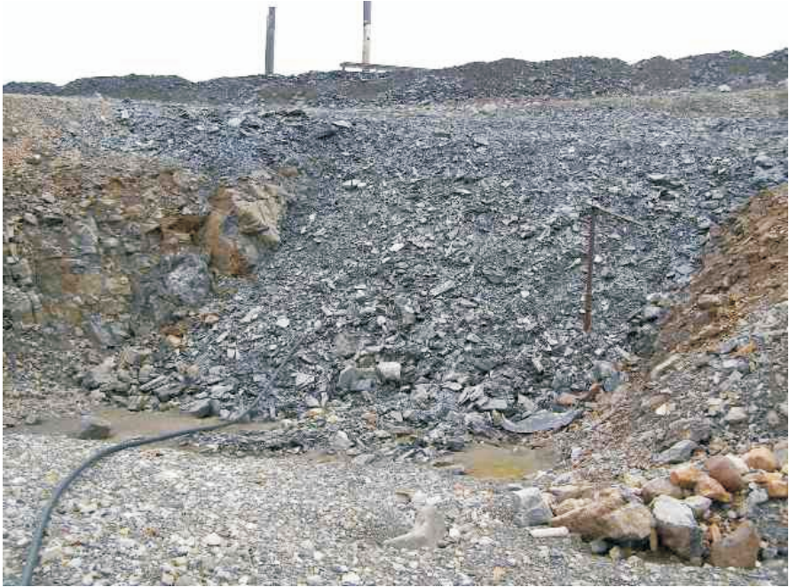
Photo 80 Plug for portal beneath Mill.
