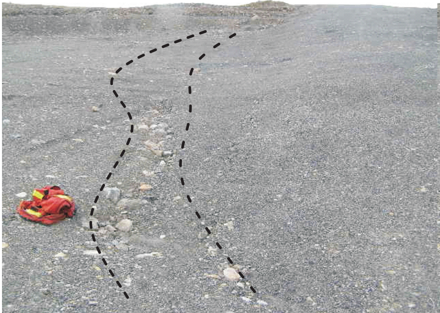
Photo 62 Edge of Oceanview Portal cover. Note minor erosional channel beginning to develop along edge of portal cover.
