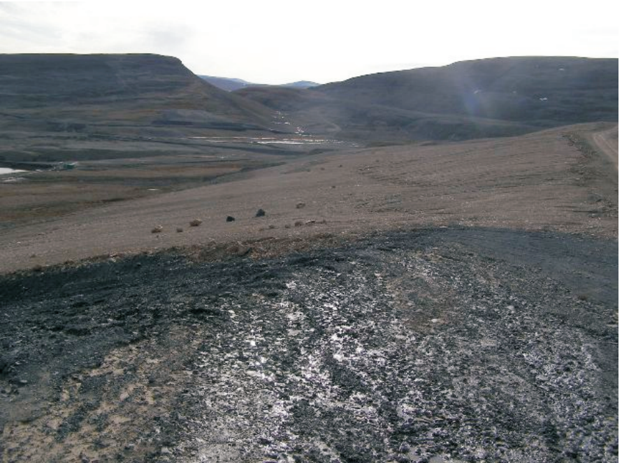
Photo 47 Erosion occurring at west end of East Open Pit cover where armour surface transitions into re-sloped shale surface below road.
