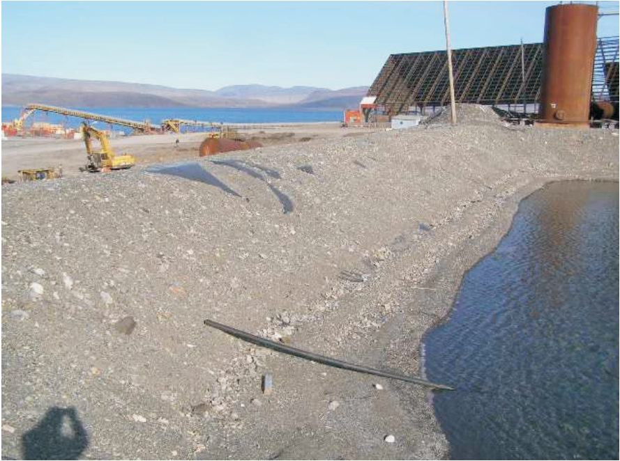
Photo 6 Main tank farm seepage collection berm. Note exposed liner.
