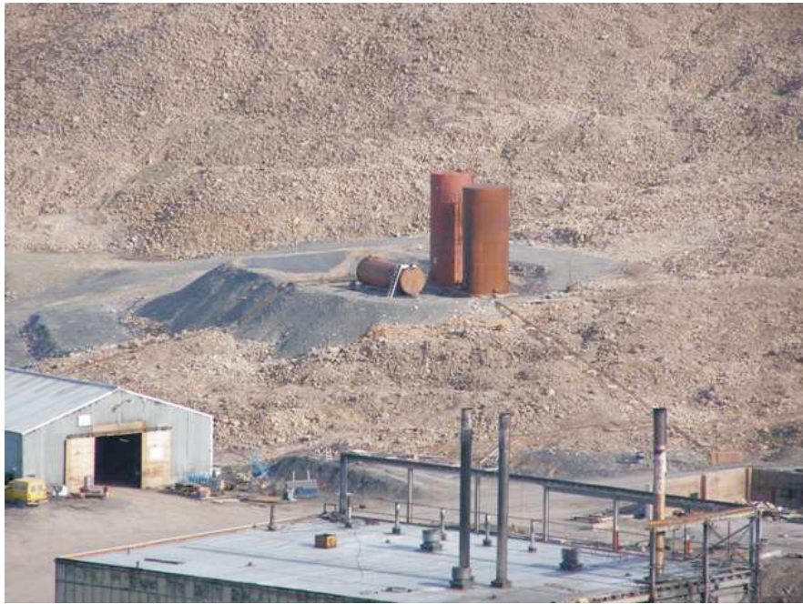
Photo 3 Day tank farm and seepage collection berm.
