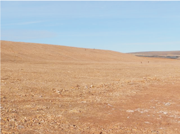
Photo 31 Test Cell tailings cover at toe of West Twin Dike.
