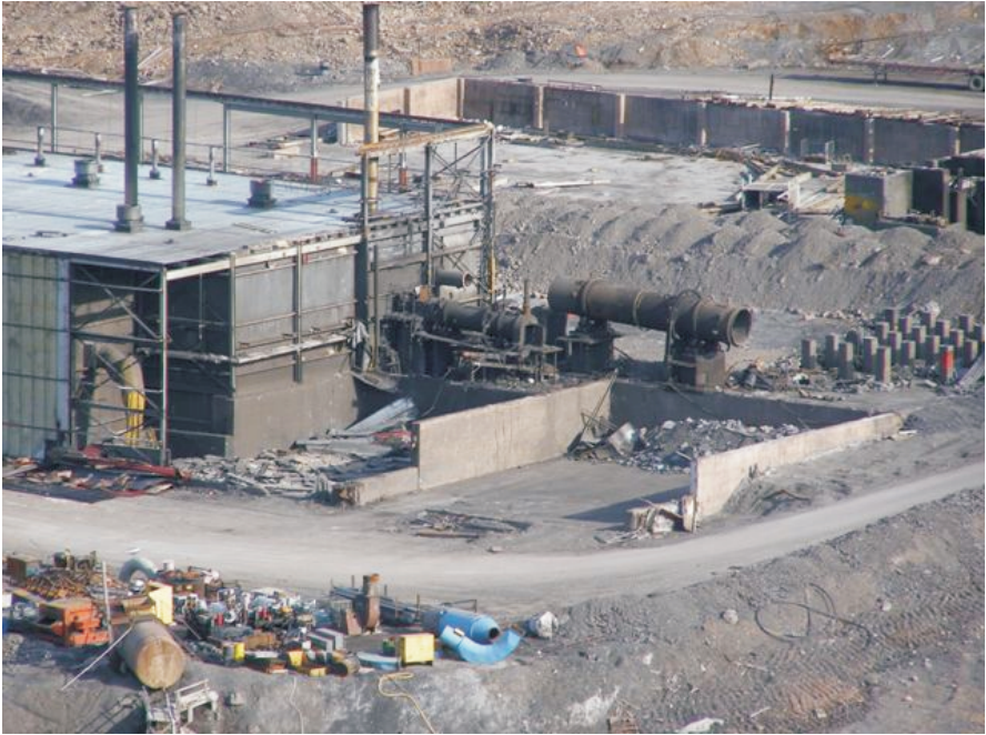
Photo 78 Mill foundation. Note soil backfill being placed.
