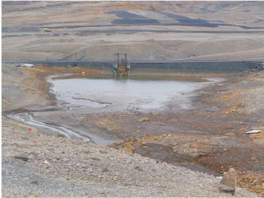
Photo 1 East Adit Treatment Pond and Dike. Note the low water level in the pond.
