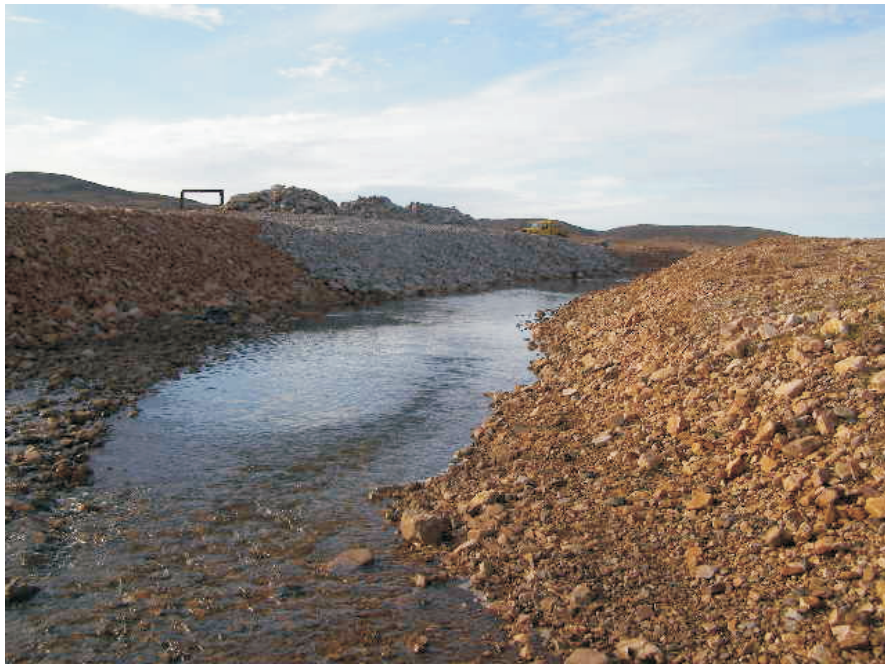
Photo 20 Riprapped face along East Twin Creek Diversion Berm. View looking downstream.
