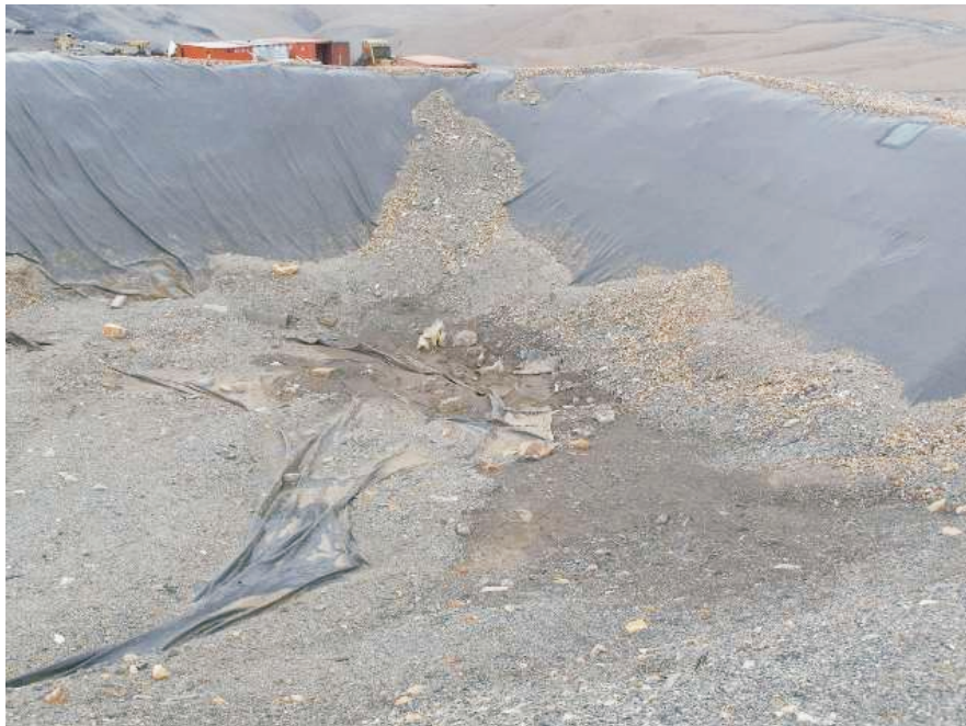
Photo 4 Day tank farm seepage collection berm. Note there is no water in the cell and the disturbed liner in the corner.
