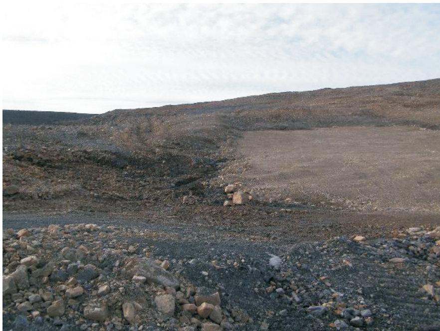
Photo 58 Seepage area at northeast corner of 17 North Portal cover.
