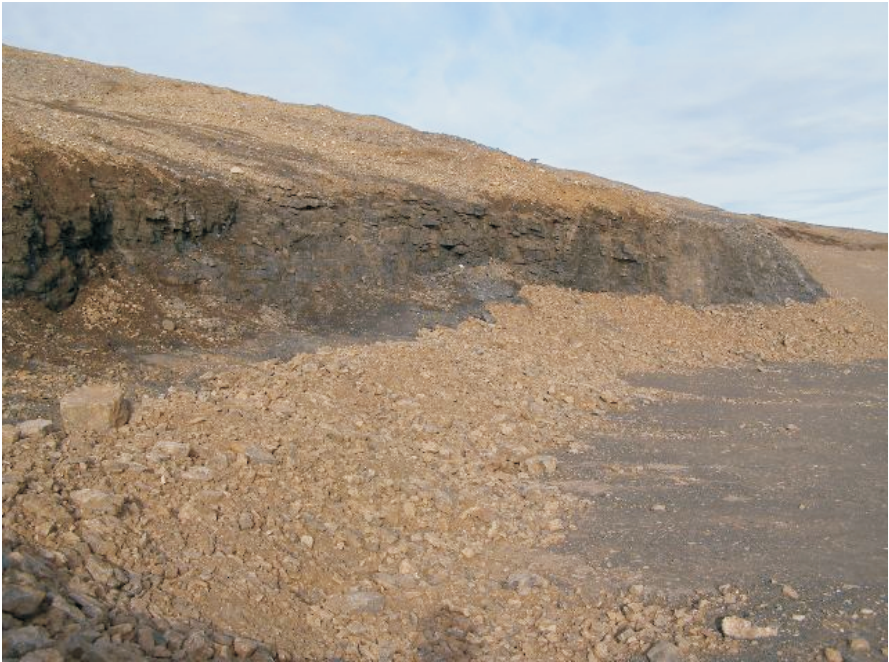
Photo 46 Armour rock along base of remnant highwall of East Open Pit.
