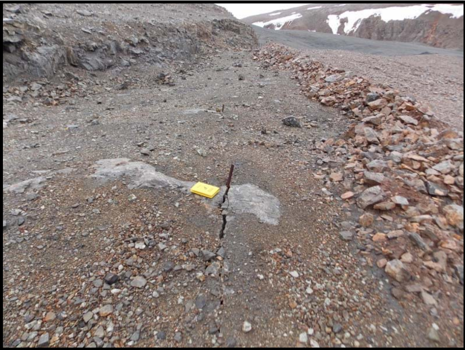
Photo 34. West Open Pit—Crack in crown pillar.
