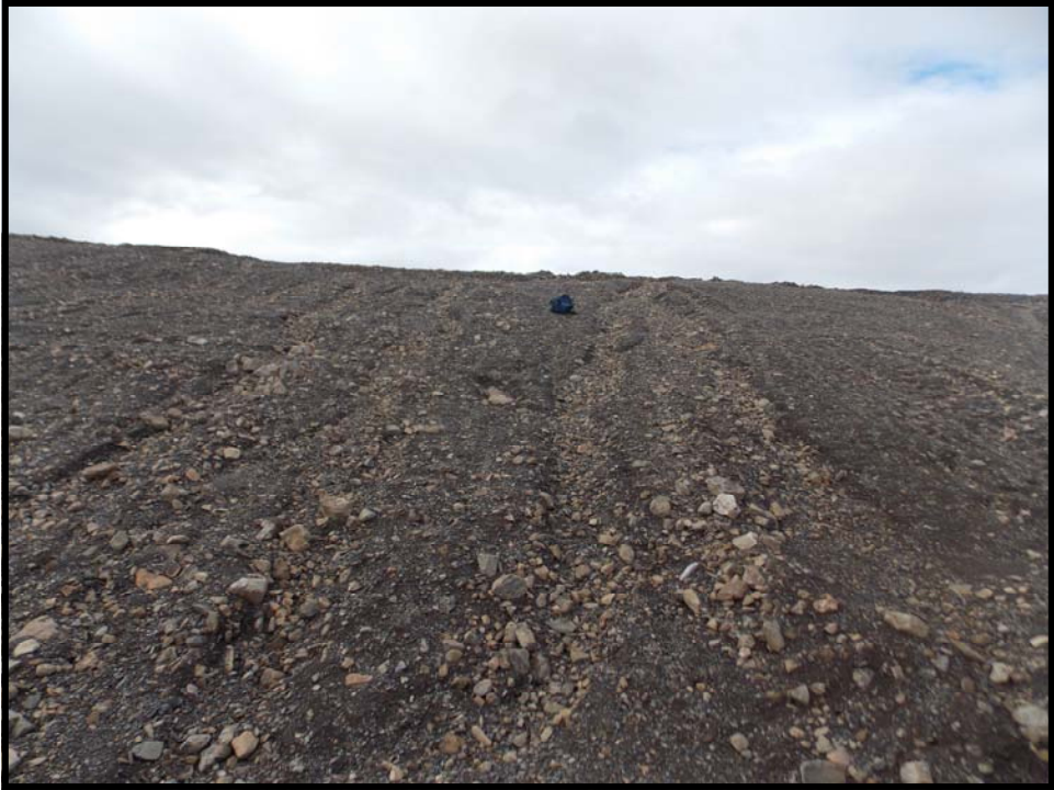
Photo 42. Oceanview Open Pit—Rill erosion along sloping face of cover at SW corner of pit.
