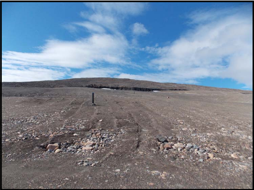
Photo 39. East Open Pit—Looking upslope along surface of cover. Note minor rill erosion.
