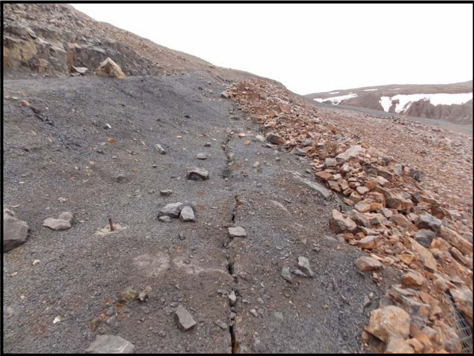
Photo 33. West Open Pit—Crack in crown pillar.
