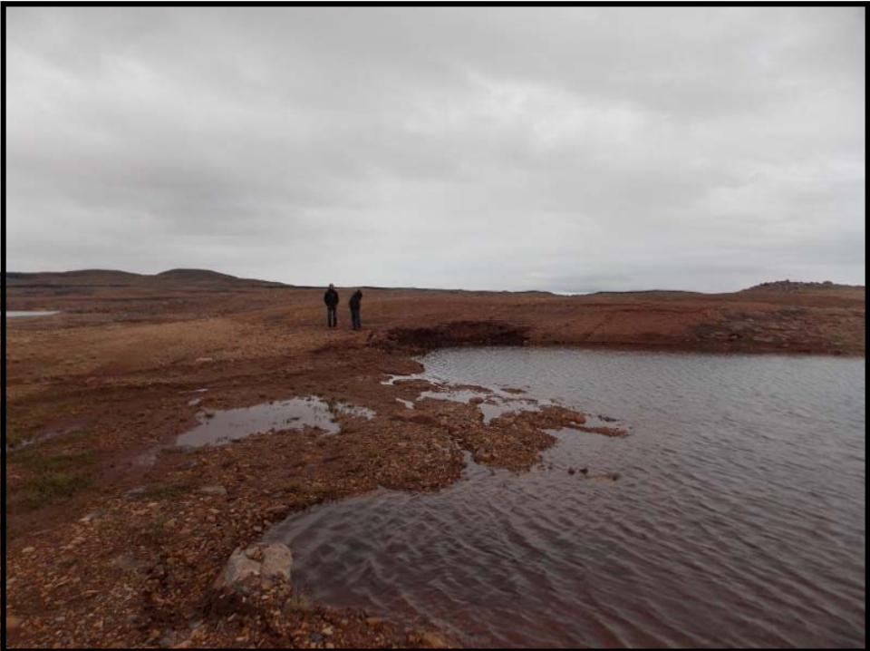
Photo 11. West Twin Outlet Channel—Slumping and thermokarst along shoreline of polishing pond.
