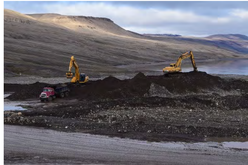
Photo 4: Relocating the stockpile from Area 2 to the concrete pad (August 14, 2014).
