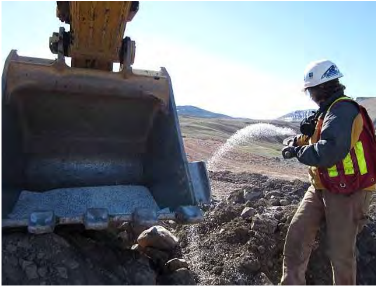
Photo 14: Nutrient amendment application process.
