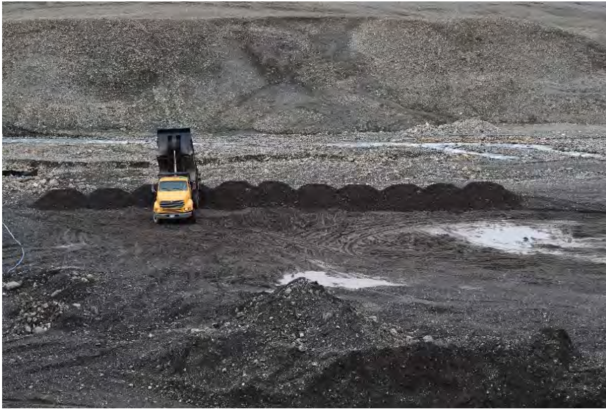
Photo 7: Relocation of remediated soil to the former secondary containment area.
