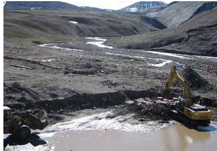
Photo 6: Waste concrete being placed in Area 4 (July 12, 2014).
