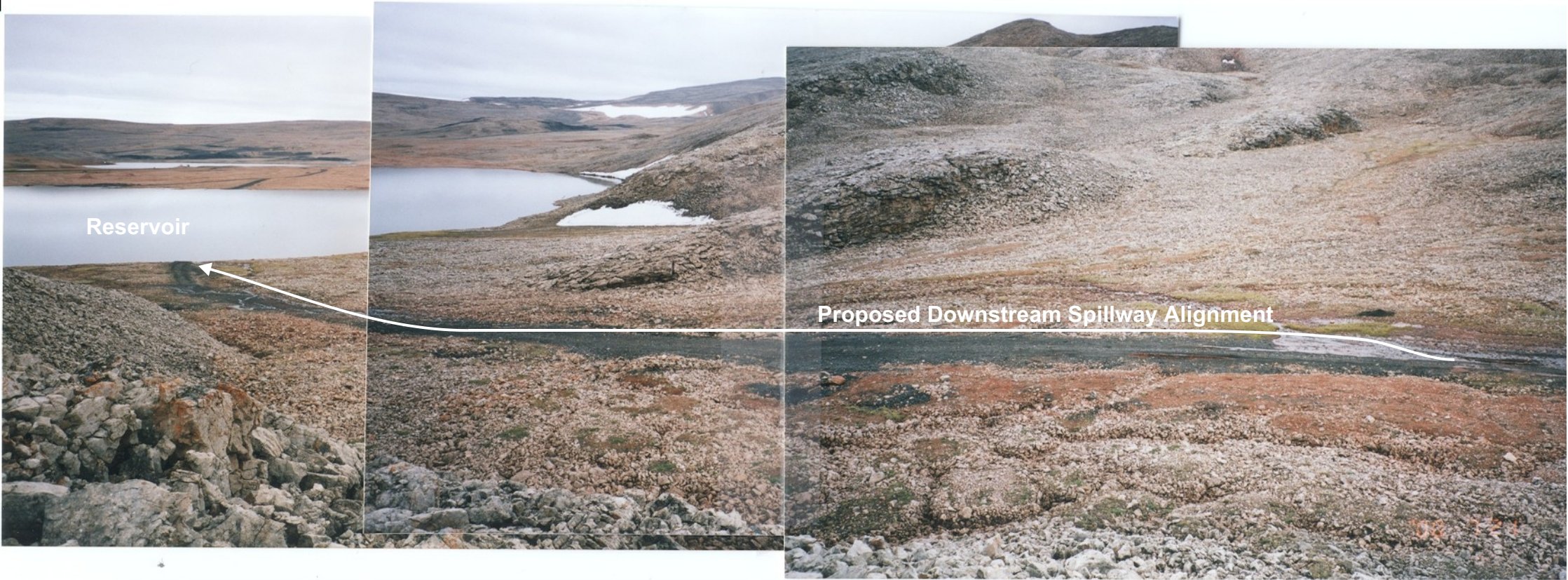
Photo #5 (left) View of downstream portion of proposed spillway alignment from the top of dolostone bedrock outcrop at the south abutment.
