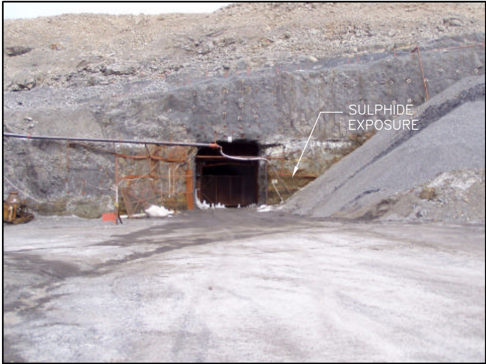
FRONT VIEW OF 00 PORTAL (JULY 2004). NOTE: SULPHIDE EXPOSURE ON HIGHWALL.
