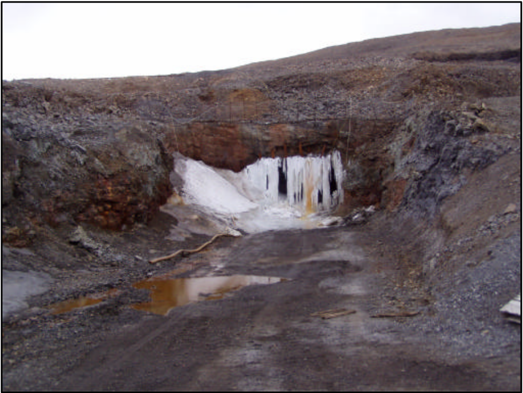
VIEW OF 88 PORTAL (JULY 2004). NOTE: CATCH FENCE ABOVE AND ICE BUILD UP AT ENTRANCE.
