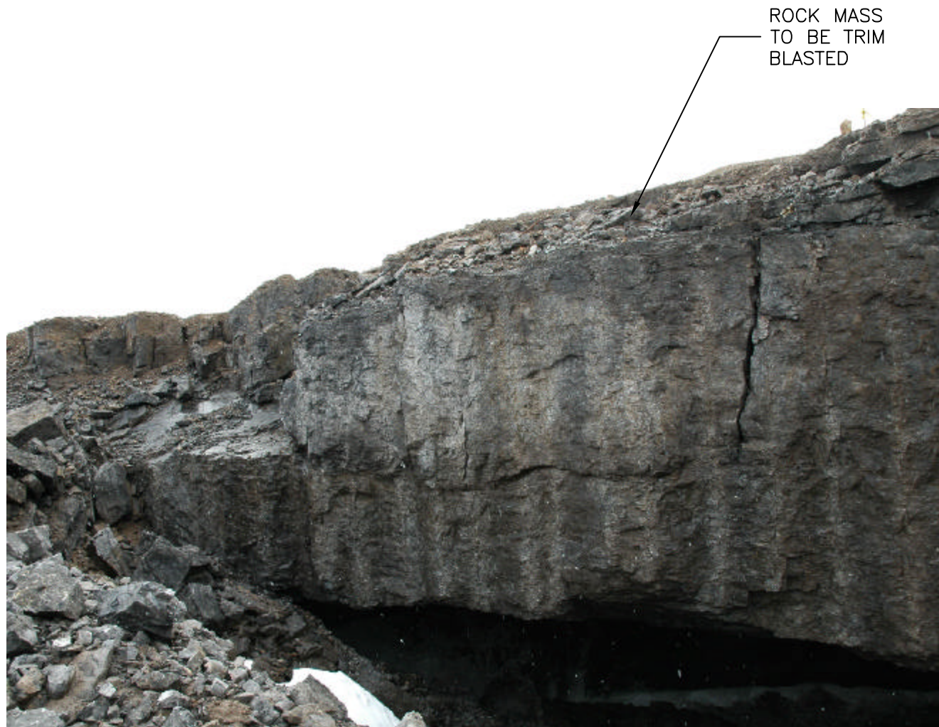
PHOTO 3 (SEPTEMBER 2004) TAKEN FROM TOP OF DEBRIS PILE LOOKING SOUTHWEST. VIEW OF ROCK BLOCK ON HEADWALL EXHIBITING DILATED JOINTS.
