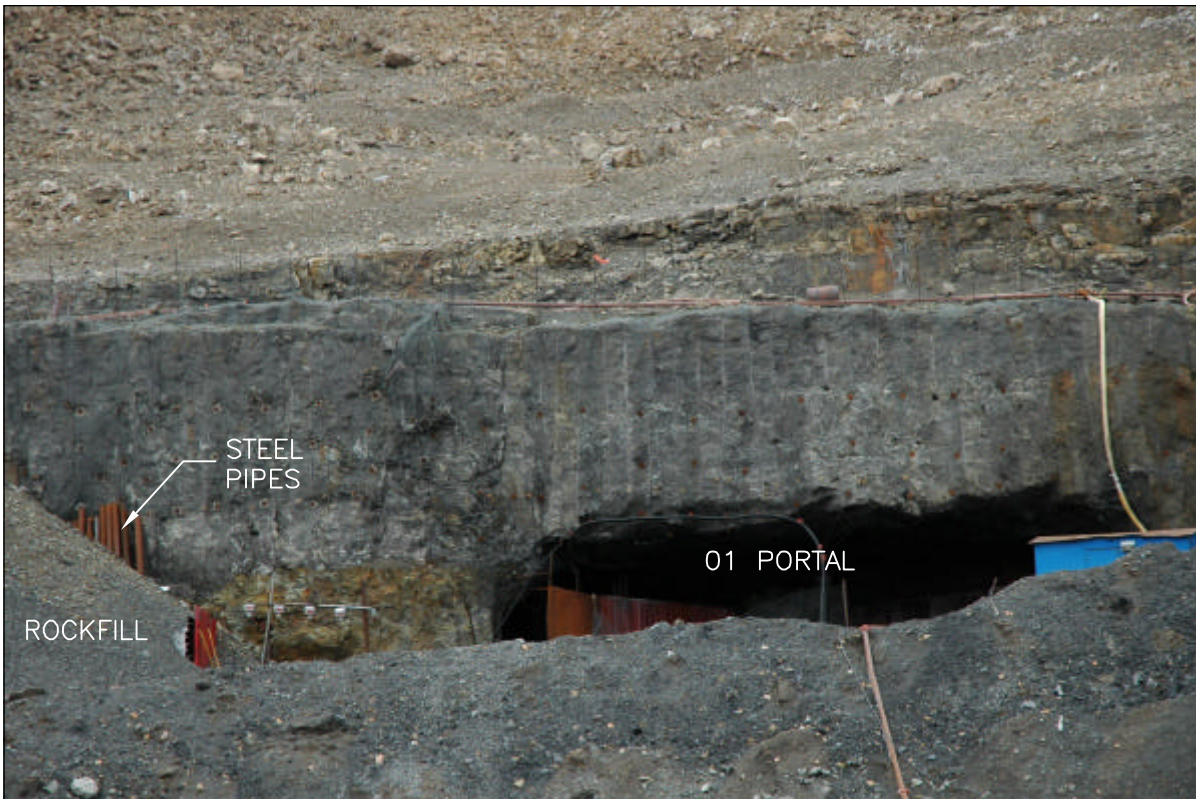
PHOTO 3 – JULY 2004 (VIEW LOOKING NORTH) ROCKFILL PLACED AGAINST STEEL PIPES LAID AGAINST THE OUTSIDE OF WEST OPEN PIT HIGHWALL ADJACENT TO 01 PORTAL.
