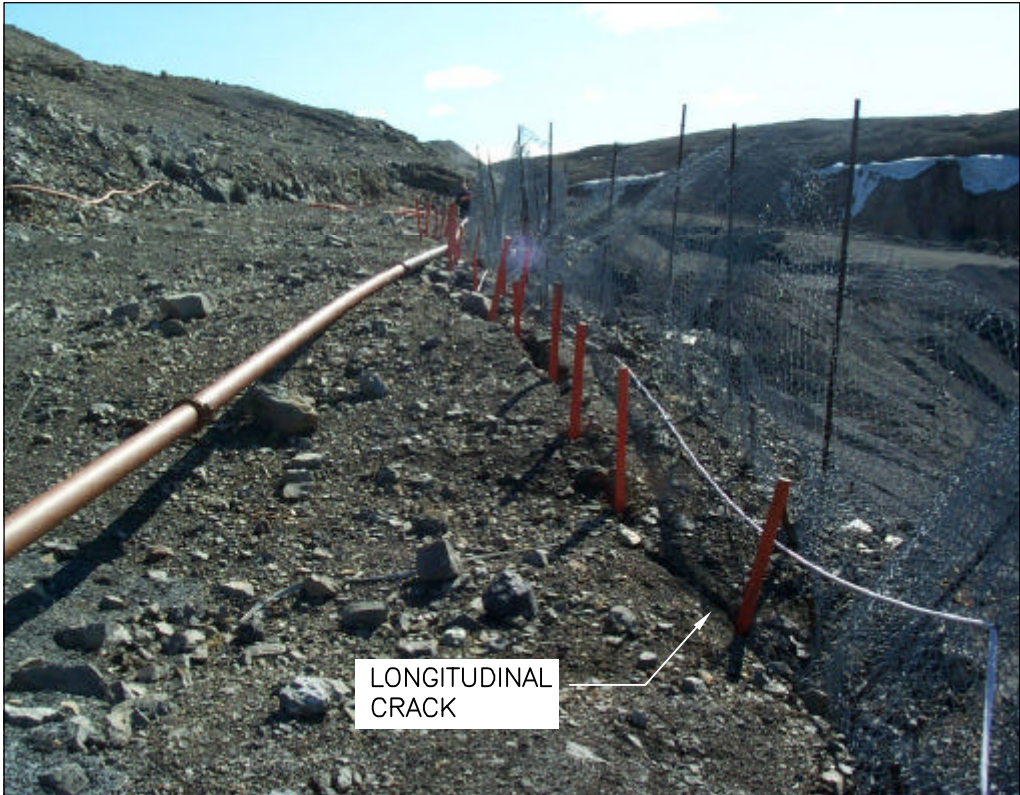
PHOTO 2 – JULY 2004 (VIEW LOOKING EAST) BENCH ABOVE WEST OPEN PIT HIGHWALL. NOTE THE LONGITUDINAL CRACK RUNNING PARALLEL TO THE HIGHWALL MARKED OUT BY ORANGE STAKES.
