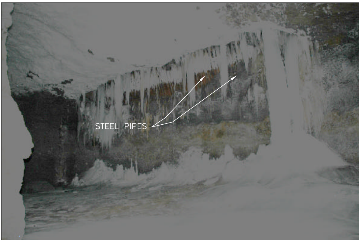
PHOTO 4 – SEPTEMBER 2004 (VIEW LOOKING SOUTH) VIEW OF REMOVED PORTION OF RIB PILLAR FROM UNDERGROUND. NOTE THE STEEL PIPES VISIBLE BY THE FROST COVER ON THE PIPES NEAR THE TOP OF THE EXCAVATION. THE PIPES RETAIN THE ROCKFILL PLACED AGAINST THE OUTSIDE FACE OF THE HIGHWALL.
