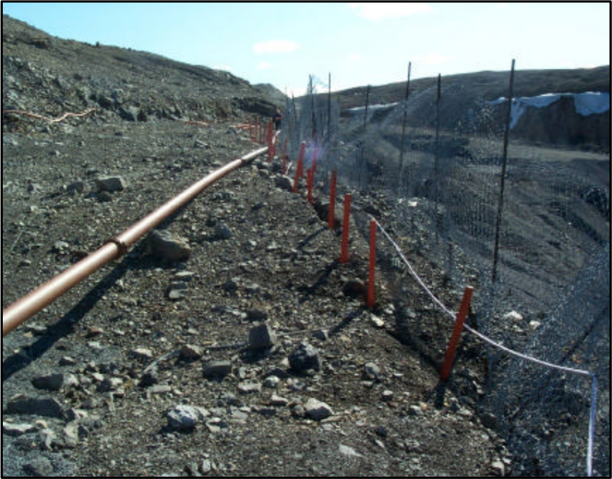
CRACK IN BENCH ABOVE HIGHWALL MARKED BY ORANGE STAKES (JULY 2004).
