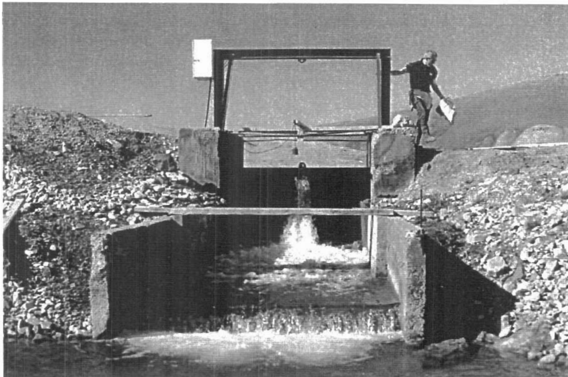
Photo 6 The effluent discharge weir from the West Twin Lakes tailings area.
