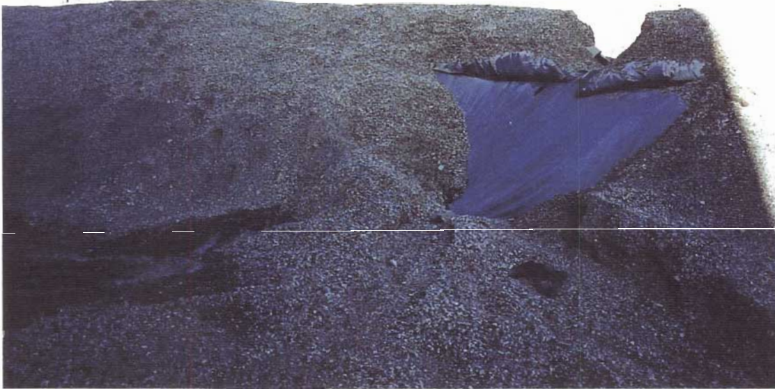
Exposed section of tank farm on internal face of east limb of perimeter containment dyke showing location of tear near internal toe, looking approximately northeast, August 1, 2000.
