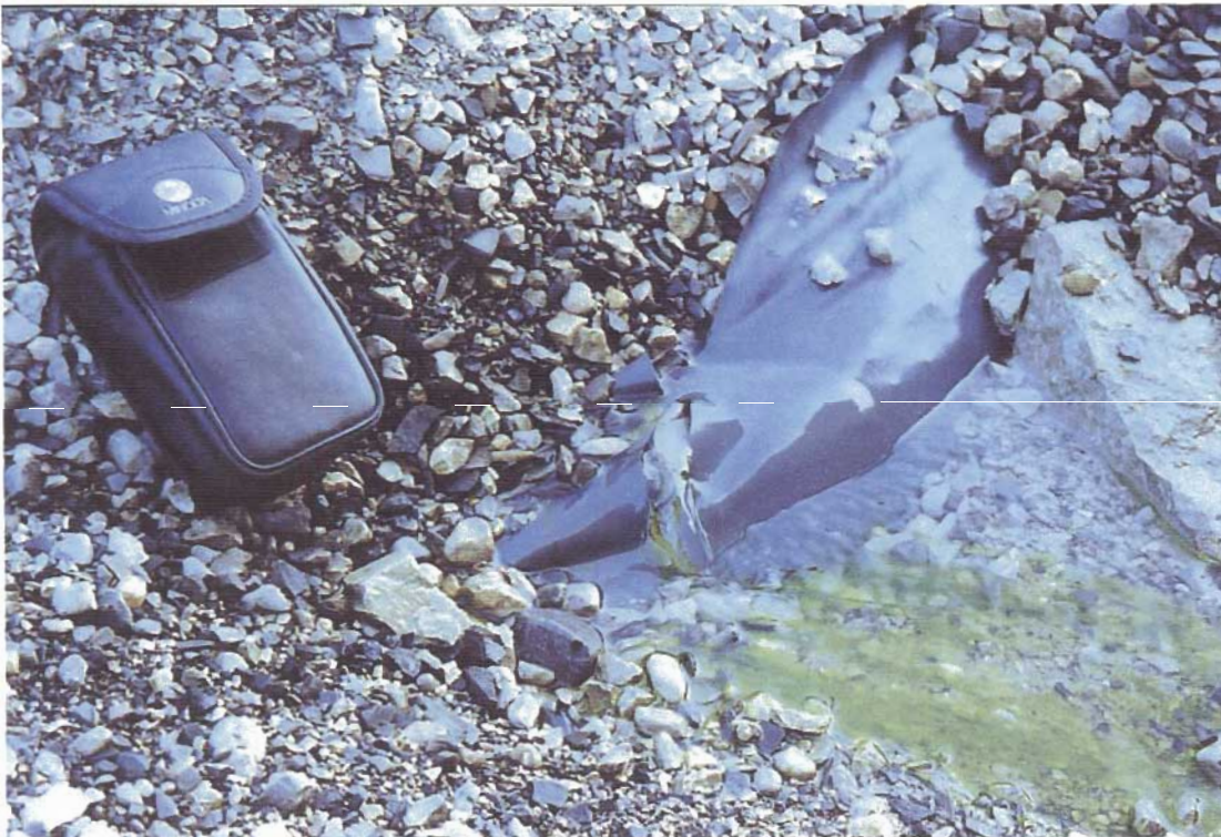
Water inflow through tear in tank farm liner near internal toe of east limb of perimeter containment dyke, August 1, 2000.
