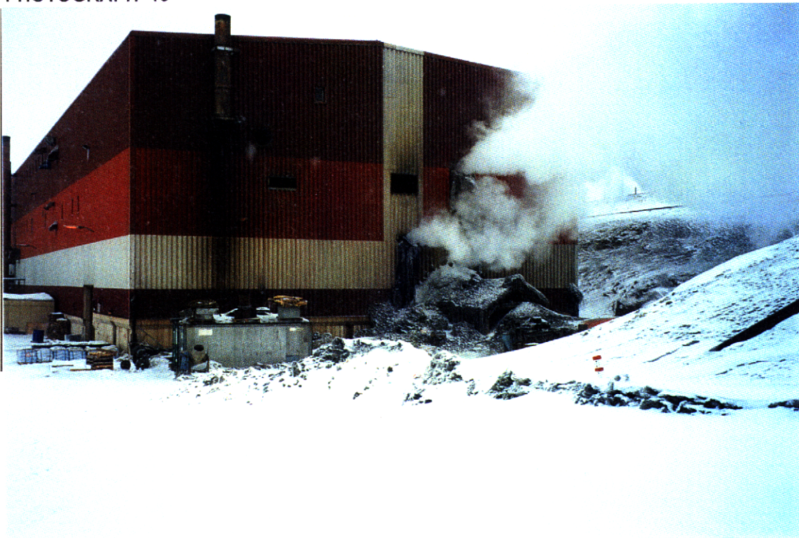
Dryer Exhaust At Rear Of Mill (lead/zinc concentrate dust on snow).
