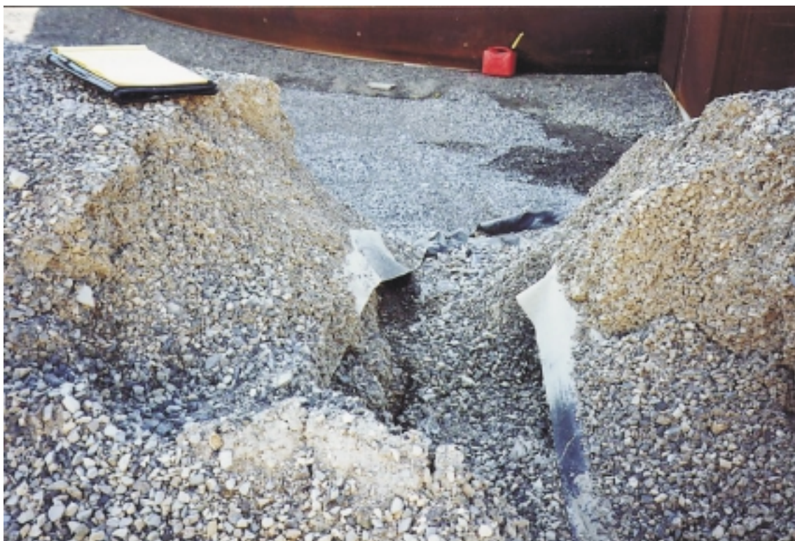
Erosion of crest perimeter containment dyke on east limb showing separated liner sections and exposed soil, August 1, 2000.
