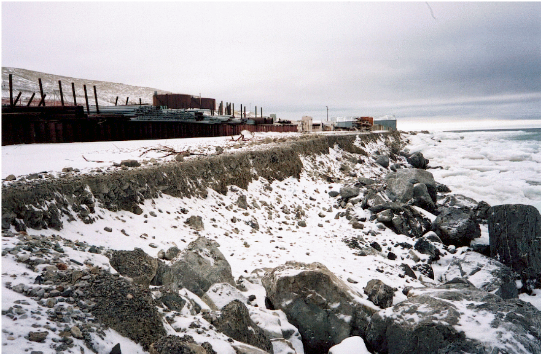
Photograph No. 17: View of shoreline looking south at Station 1100 N. The riprap is failing and the bank behind the riprap is eroding. Some larger pieces of mine rock are in the order of 900 mm cube size, and are deteriorating rapidly due to freeze/thaw cycles. (August 19, 2000).
