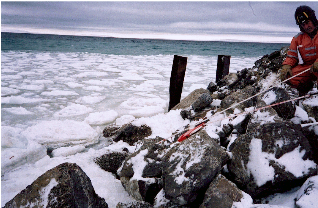
Photograph No. 22: View of shoreline looking north at Station 800 N. This is the southern extent of the riprap and is immediately south of the H-Piles at the temporary dock. (August 19, 2000).
