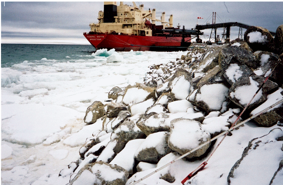
Photograph No. 14: View of shoreline looking north at Station 1200 N. New riprap has been placed between here and the dock in the last 2 years, and has a mean size of about 300 mm. (August 19, 2000).
