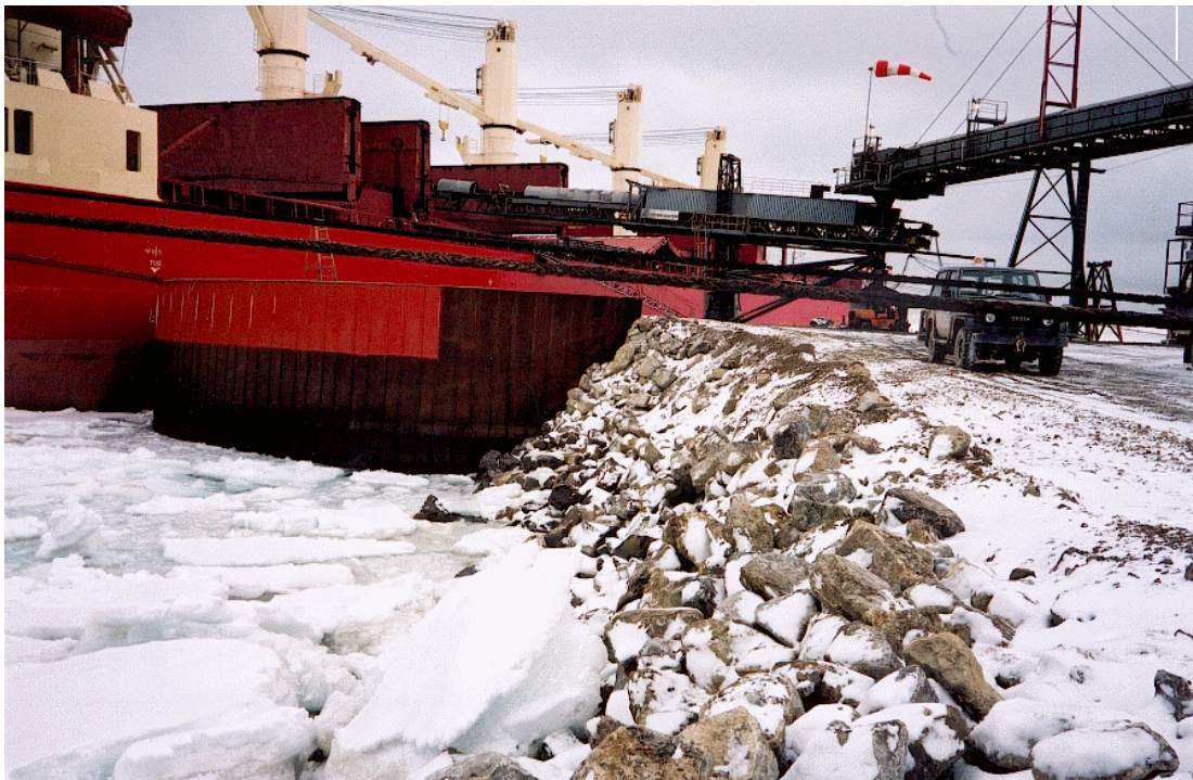
Photograph No. 12: View of shoreline looking north at Station 1300 N. New riprap has been placed in this area in the last 2 years. (August 19, 2000).
