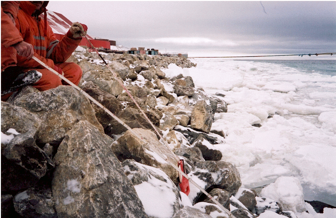
Photograph No. 13: View of shoreline looking south at Station 1300 N. This area has the largest size rock produced from the Little Red Dog Quarry and used as riprap, with a mean size in the range of about 400 mm to 500 mm. (August 19, 2000).
