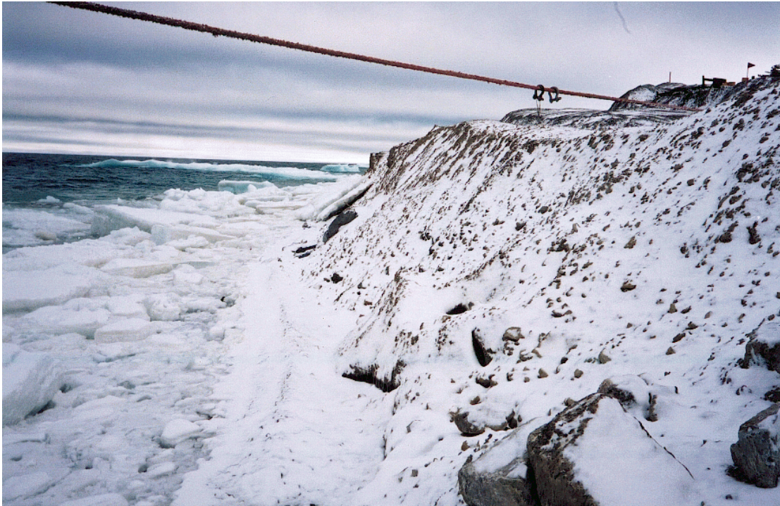
Photograph No. 10: View of shoreline looking north at Station 1500 N. The shoreline to the north of 1500 N is fill comprised of material with about 300 mm minus material. (August 19, 2000).
