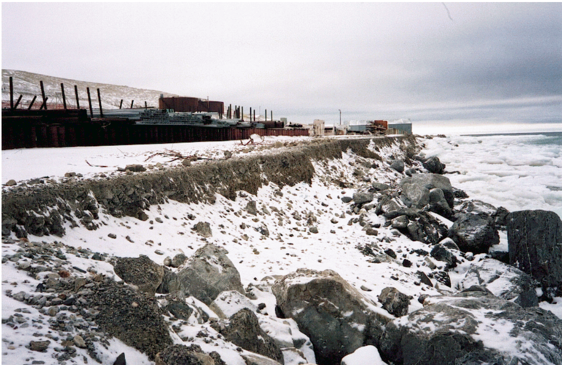
Photograph No. 17: View of shoreline looking south at Station 1100 N. The riprap is failing and the bank behind the riprap is eroding. Some larger pieces of mine rock are in the order of 900 mm cube size, and are deteriorating rapidly due to freeze/thaw cycles. (August 19, 2000).
