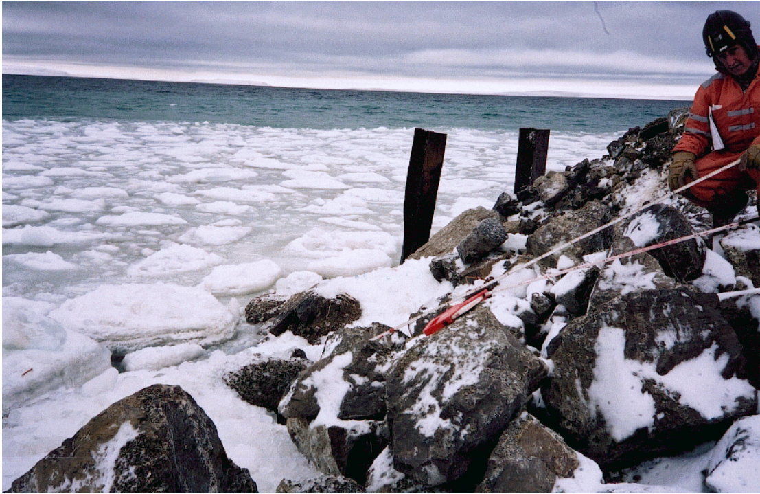
Photograph No. 22: View of shoreline looking north at Station 800 N. This is the southern extent of the riprap and is immediately south of the H-Piles at the temporary dock. (August 19, 2000).
