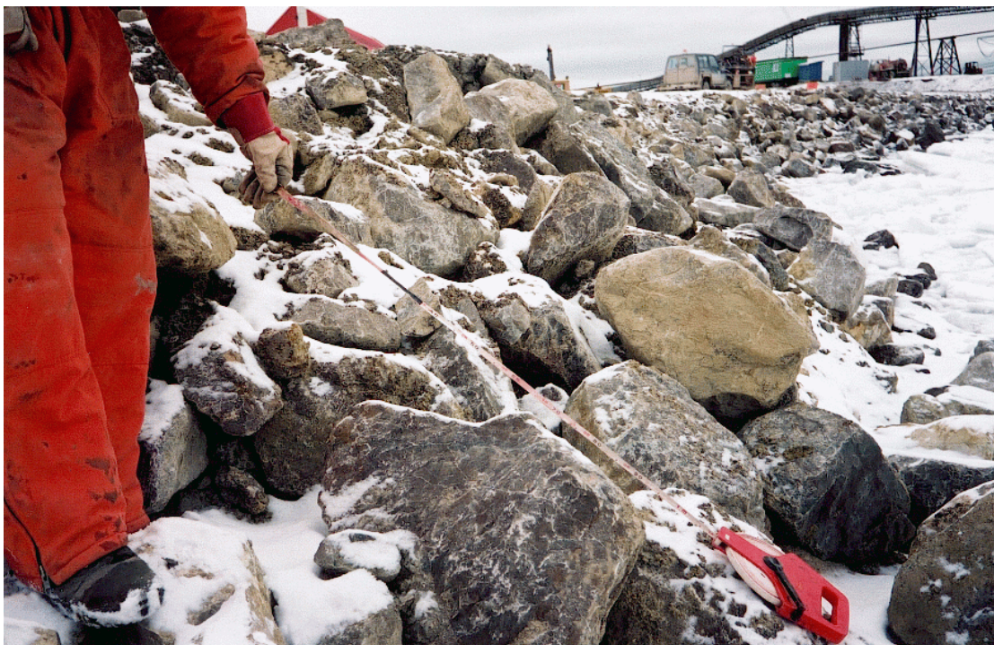
Photograph No. 11: View of shoreline looking south at Station 1500 N. The shoreline is covered with rip rap to the south of Station 1500 N, with a mean size of about 300 mm (August 19, 2000).
