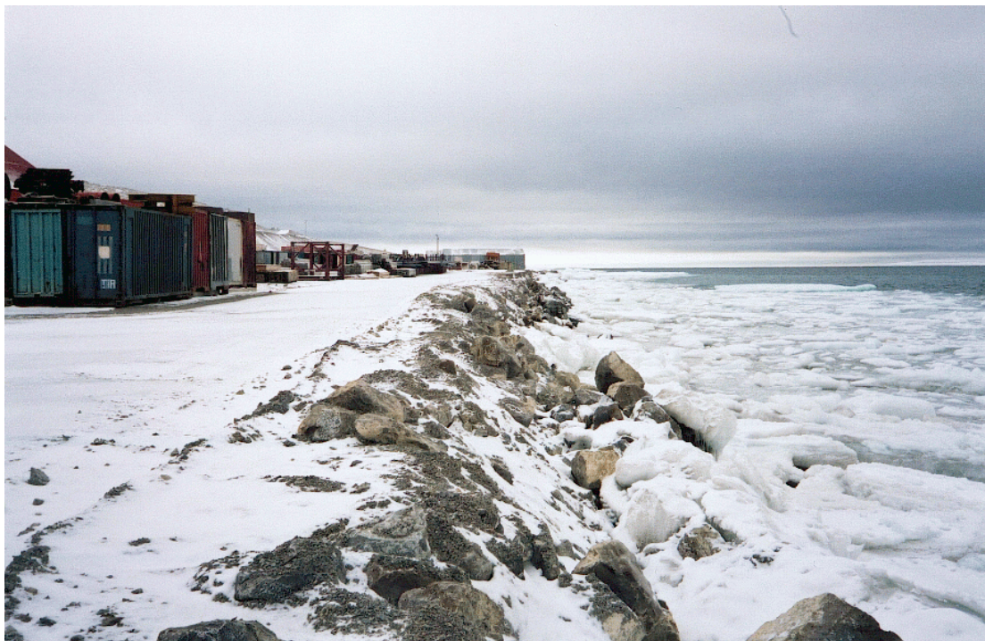
Photograph No. 15: View of shoreline looking south at Station 1200 N. It has been more than two years since riprap has been placed south of Station 1200 N. (August 19, 2000).
