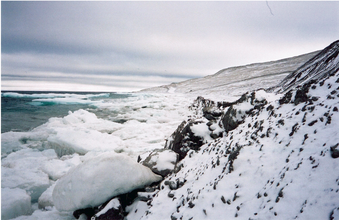
Photograph No. 8: View of shoreline looking north at Station 1600 N. The fill is about a 300 mm minus material, with a mean size of 25 mm. (August 19, 2000).
