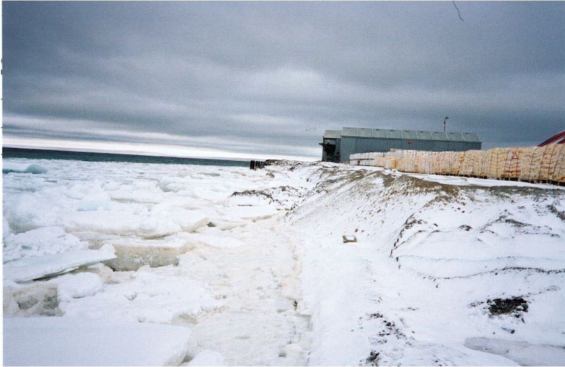
Photograph No. 24: View of shoreline looking north at Station 700 N. The beach is comprised of natural material at this location, with some regrading of the top of the bank to form a flat storage area. (August 19, 2000).
