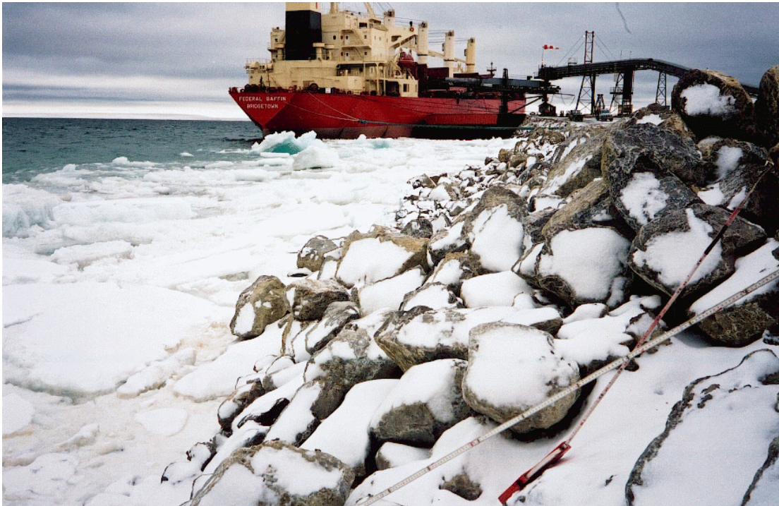
Photograph No. 14: View of shoreline looking north at Station 1200 N. New riprap has been placed between here and the dock in the last 2 years, and has a mean size of about 300 mm. (August 19, 2000).
